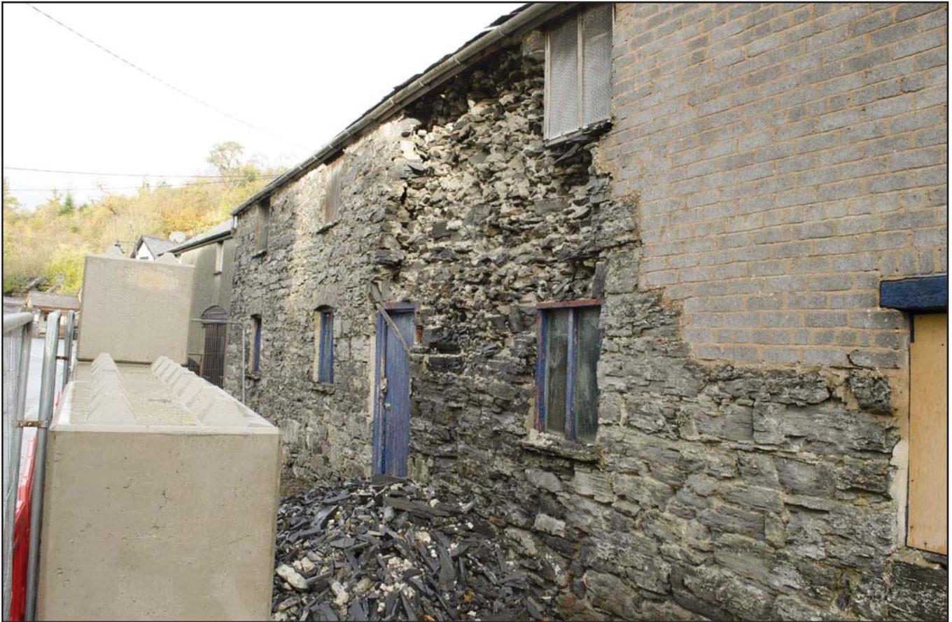
Plate 39: Partially collapsed roadside façade of Block C; scale not used; view from SSE (archive reference: G2750\_008).
