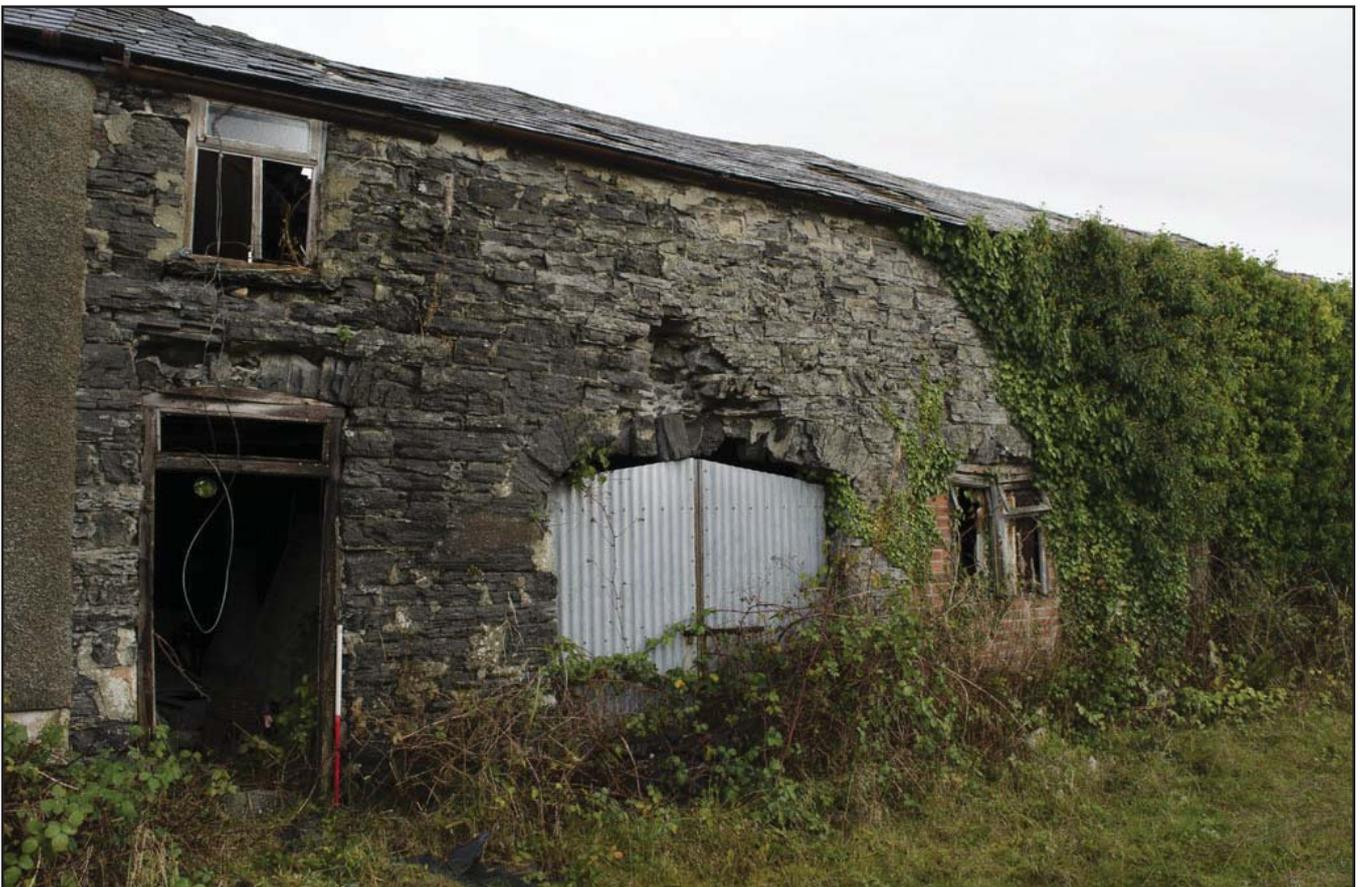
Plate 4: Block A, close up of southwest face with structural damage; scale 1x1m; view from SW (archive reference: G2750\_016).
