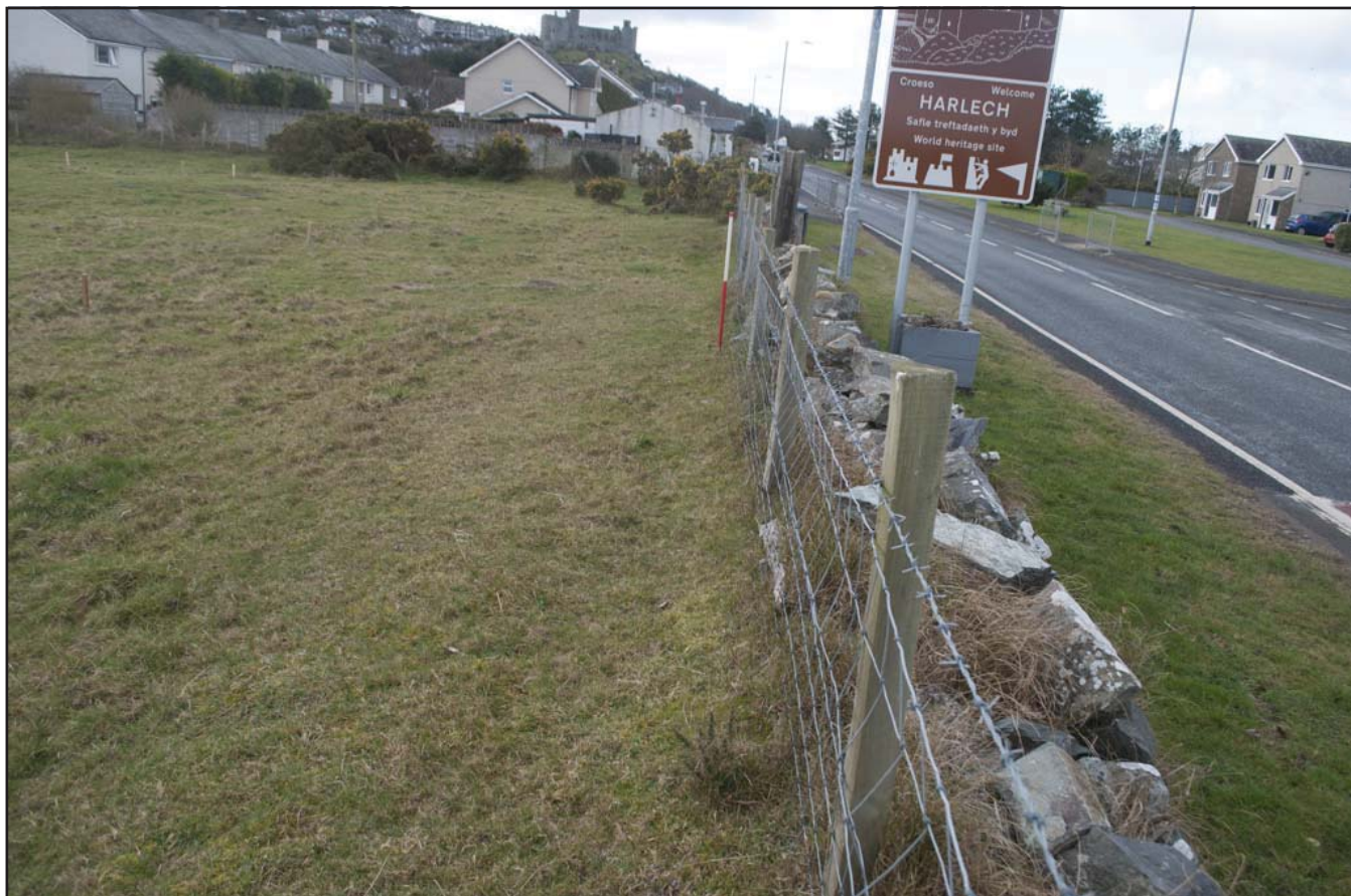
Plate 7: View along the western low drystone wall alongside the road boundary (0.6 m high); scale 1m; view from NE (archive reference: G2759_07).
