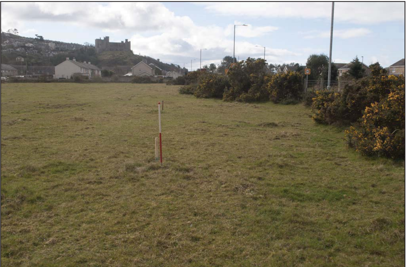
Plate 16: View along the pegs of the marked out services; scale 1m; view from N (archive reference: G2759_16).
