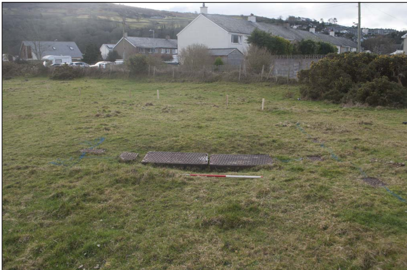
Plate 9: View of services within the development plot; scale 1m; view from NW (archive reference: G2759_09).
