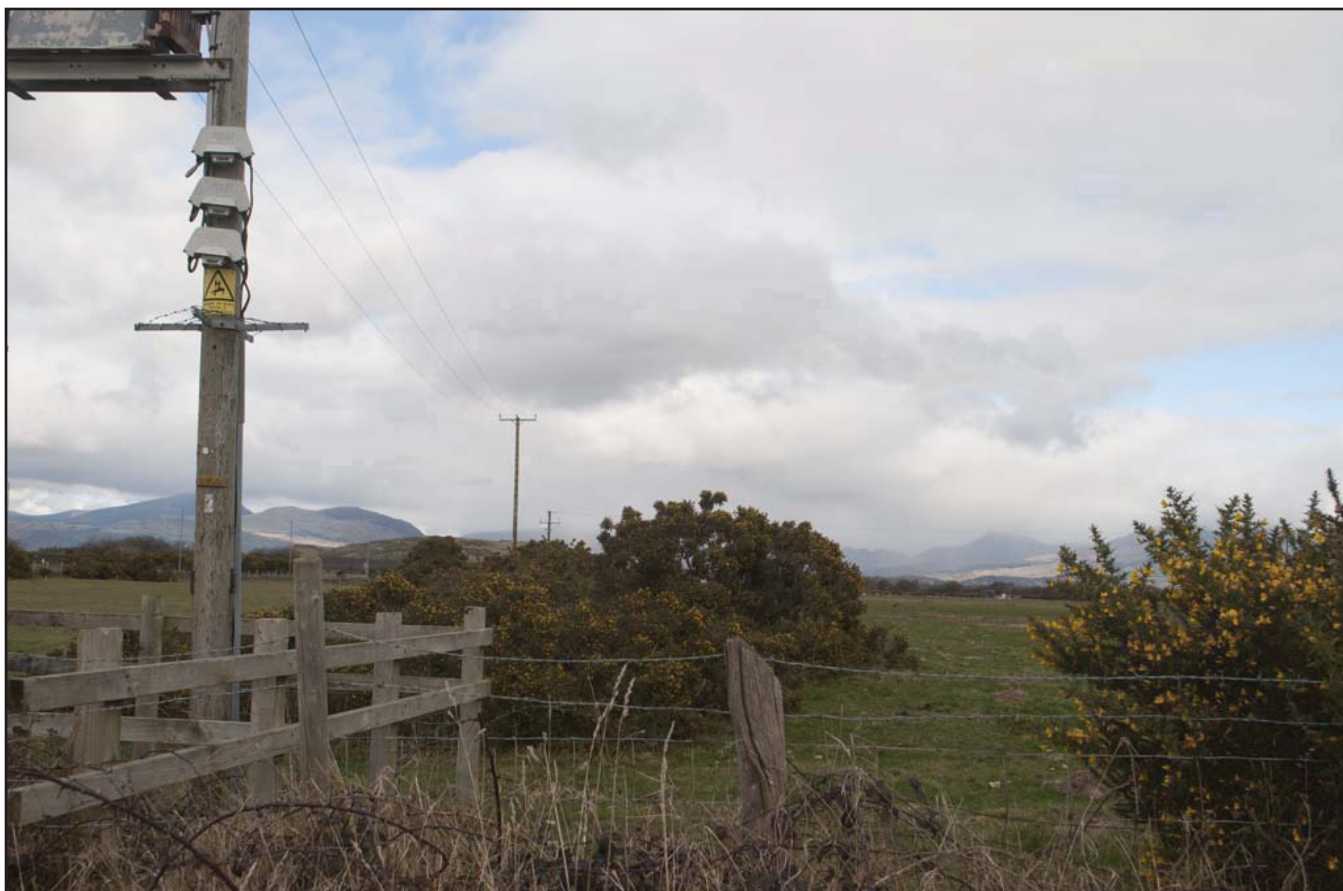
Plate 22: View of gorse covered embankment from the public footpath; scale not used; view from SSE (archive reference: G2759_22).
