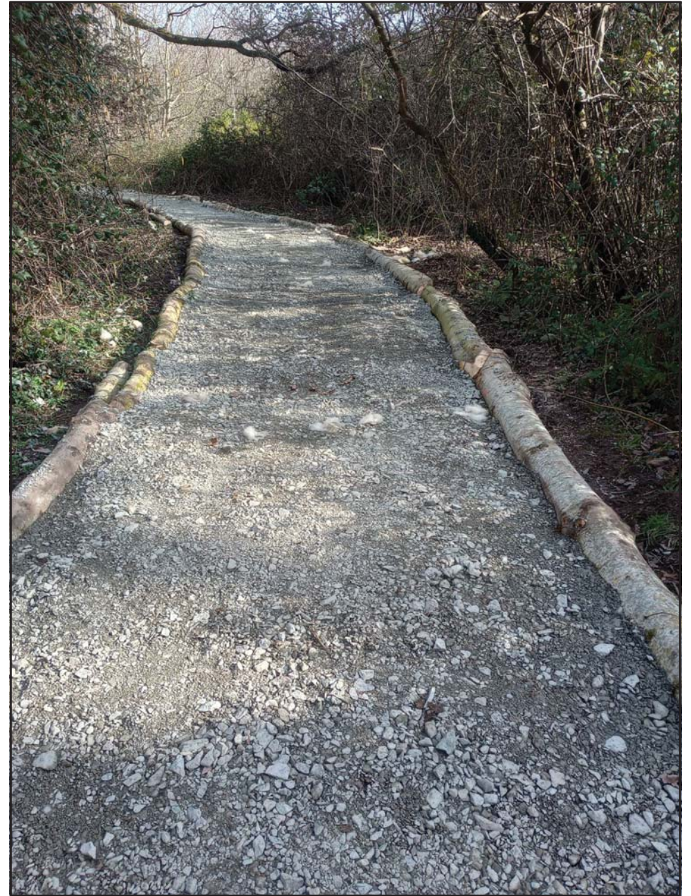
Plate 08: Footpath #1 showing stone laid for the path (archive reference: G2771_13).
