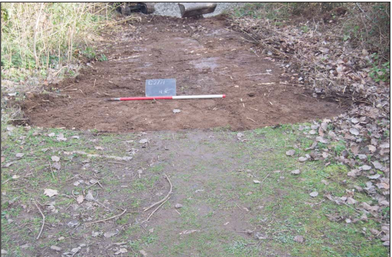
Plate 06: View of footpath #2 on the north eastern side of the castle after shallow scrape of soil removed; scale: 1x1m (archive reference: G2771_08).
