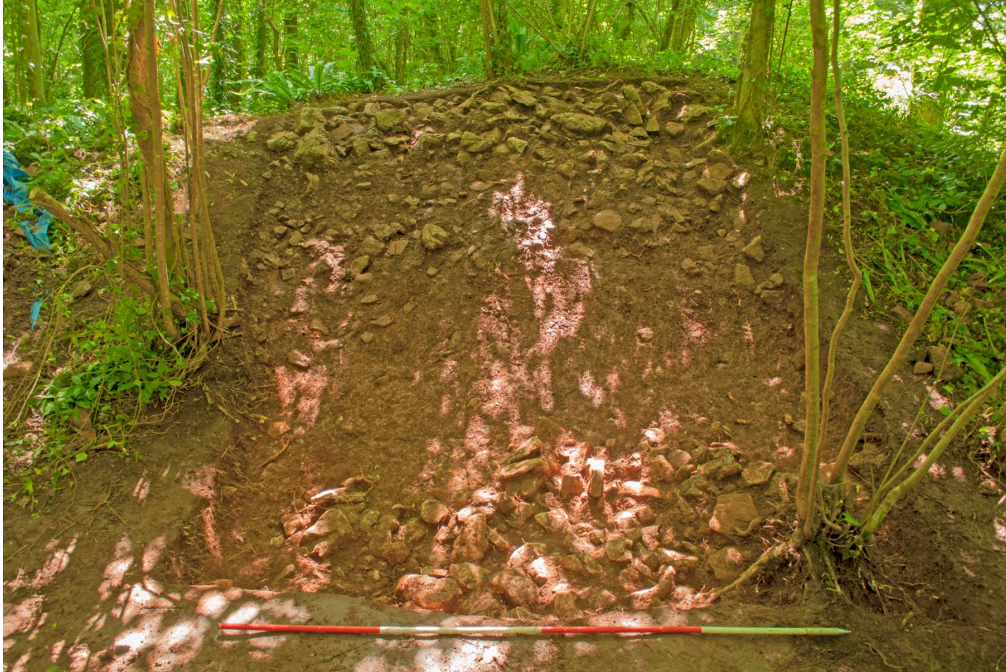
Figure 10: North-east facing side of bank B following removal of topsoil and leaf litter (900), showing rubble capping of bank (901) and upper ditch fill (904). (2m scale).
