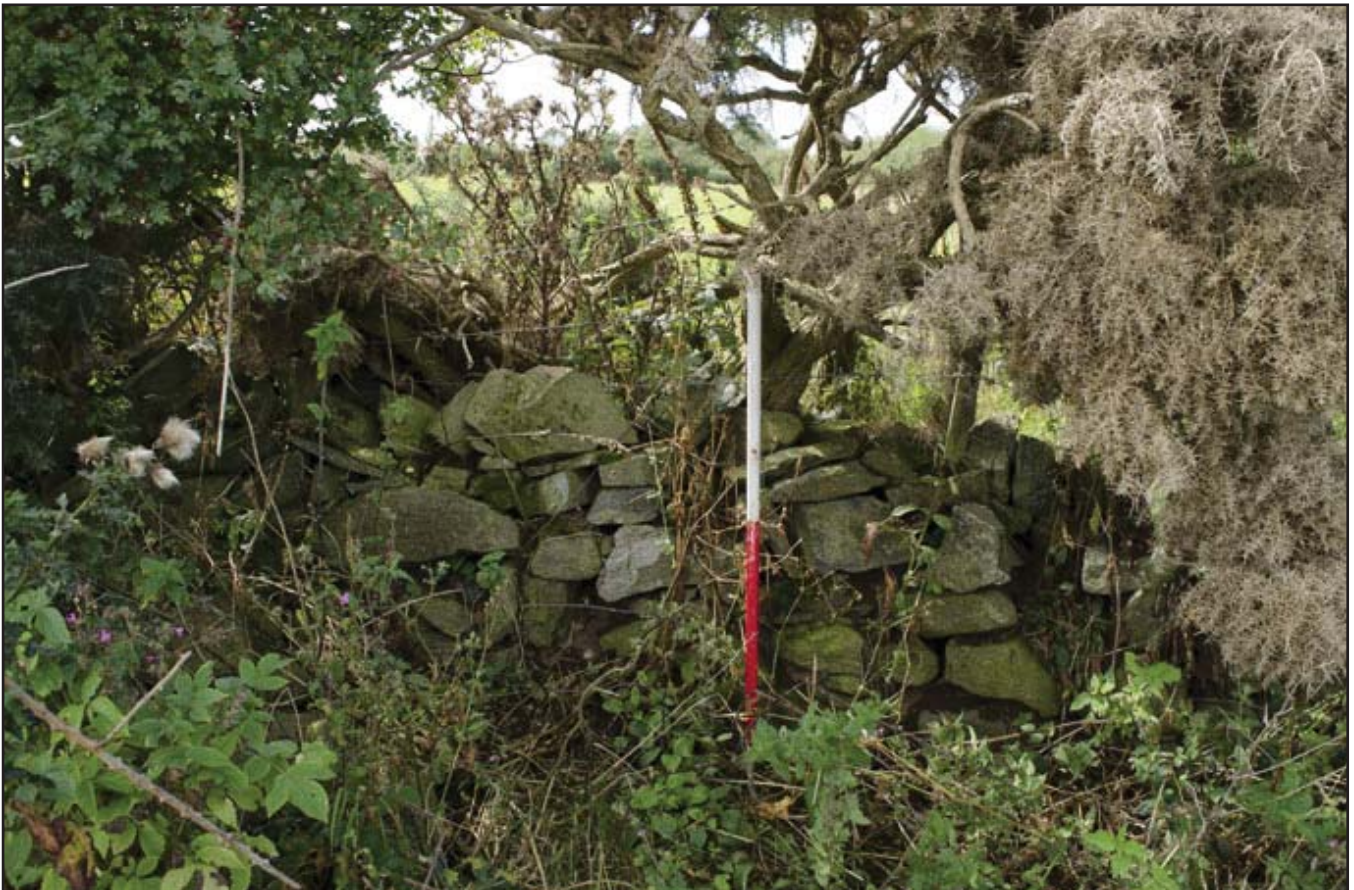
Plate 42: Dilapidated drystone wall between Fields 4 & 5; scale 1x1m; view from ENE (archive reference: G2739_040).
