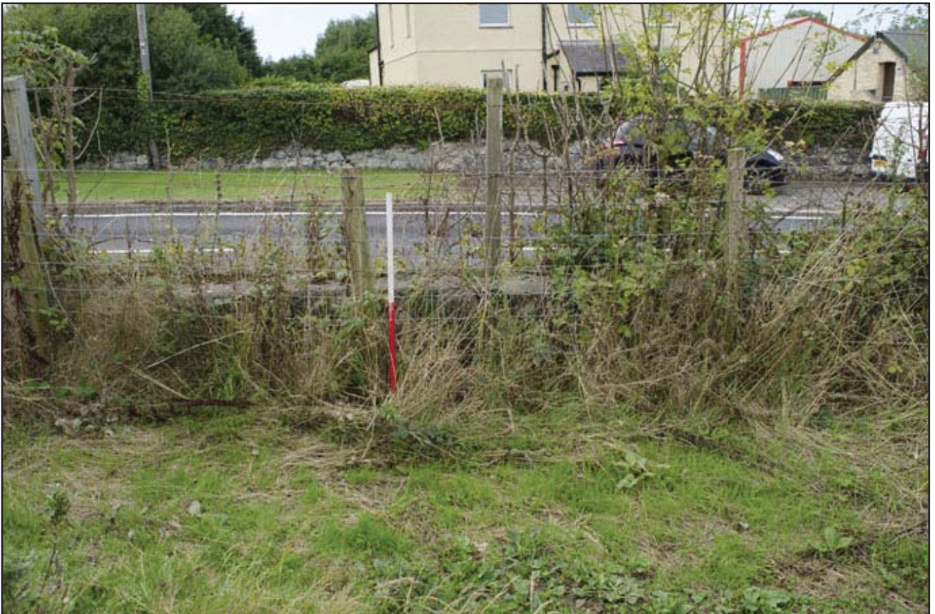
Plate 50: Low stone and concrete wall and post and wire fence; scale 1x1m; view from NE (archive reference: G2739_048).
