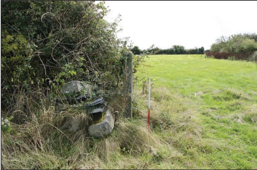
Plate 37: Concrete gate post and access Field 3 & 4; scale 1x1m; view from NW (archive reference: G2739_035).
