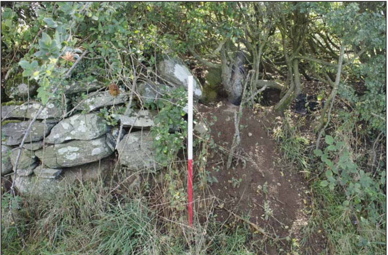
Plate 32: Boundary between drystone wall of Field 3 and clawdd of Field 2; scale 1x1m; view from NW (archive reference: G2739_030).
