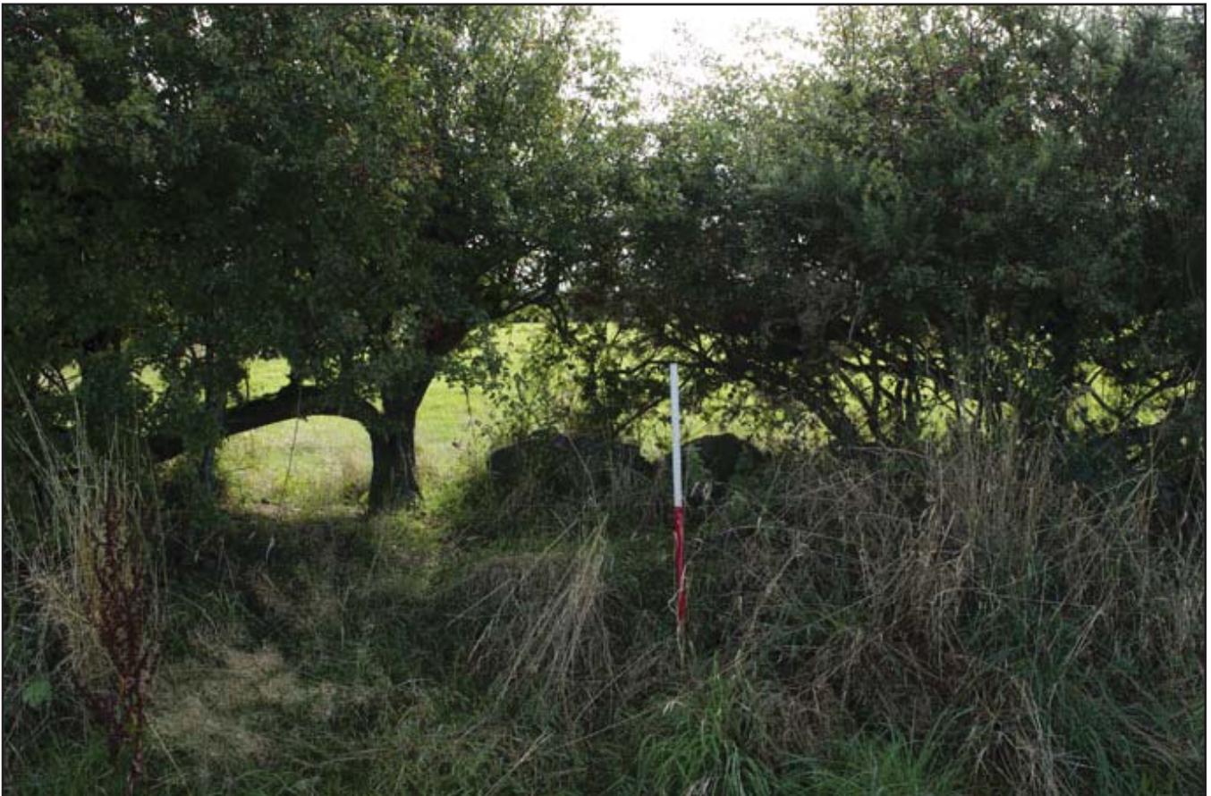
Plate 34: Tumbled clawdd and hedgerow boundary between fields 3 & 4; scale 1x1m; view from WNW (archive reference: G2739_032).
