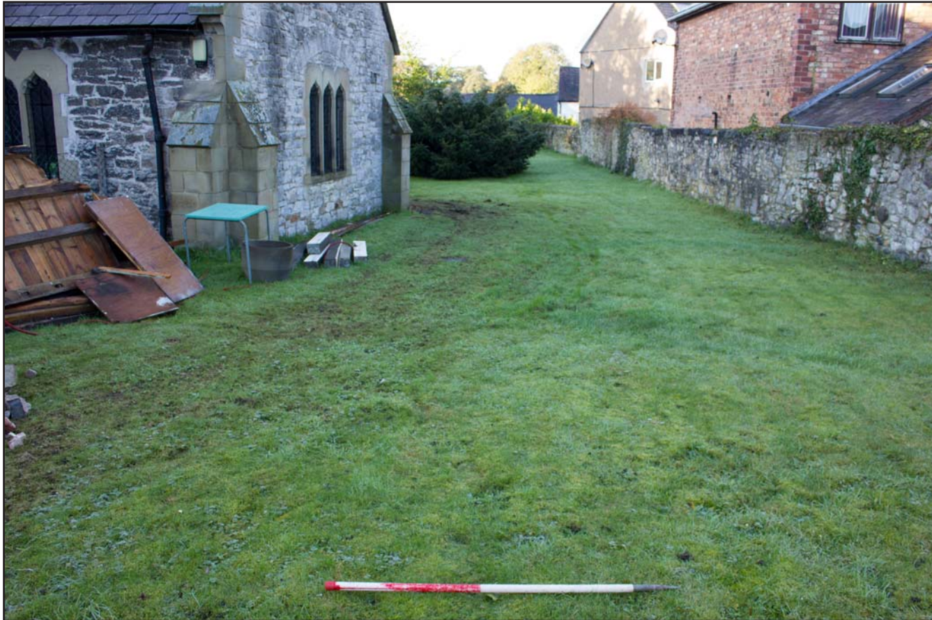
Plate 31: Pre excavation shot of drainage route to the north of St. Asaph Parish Church, St. Asaph, Denbighshire - from the east - scale 1m
