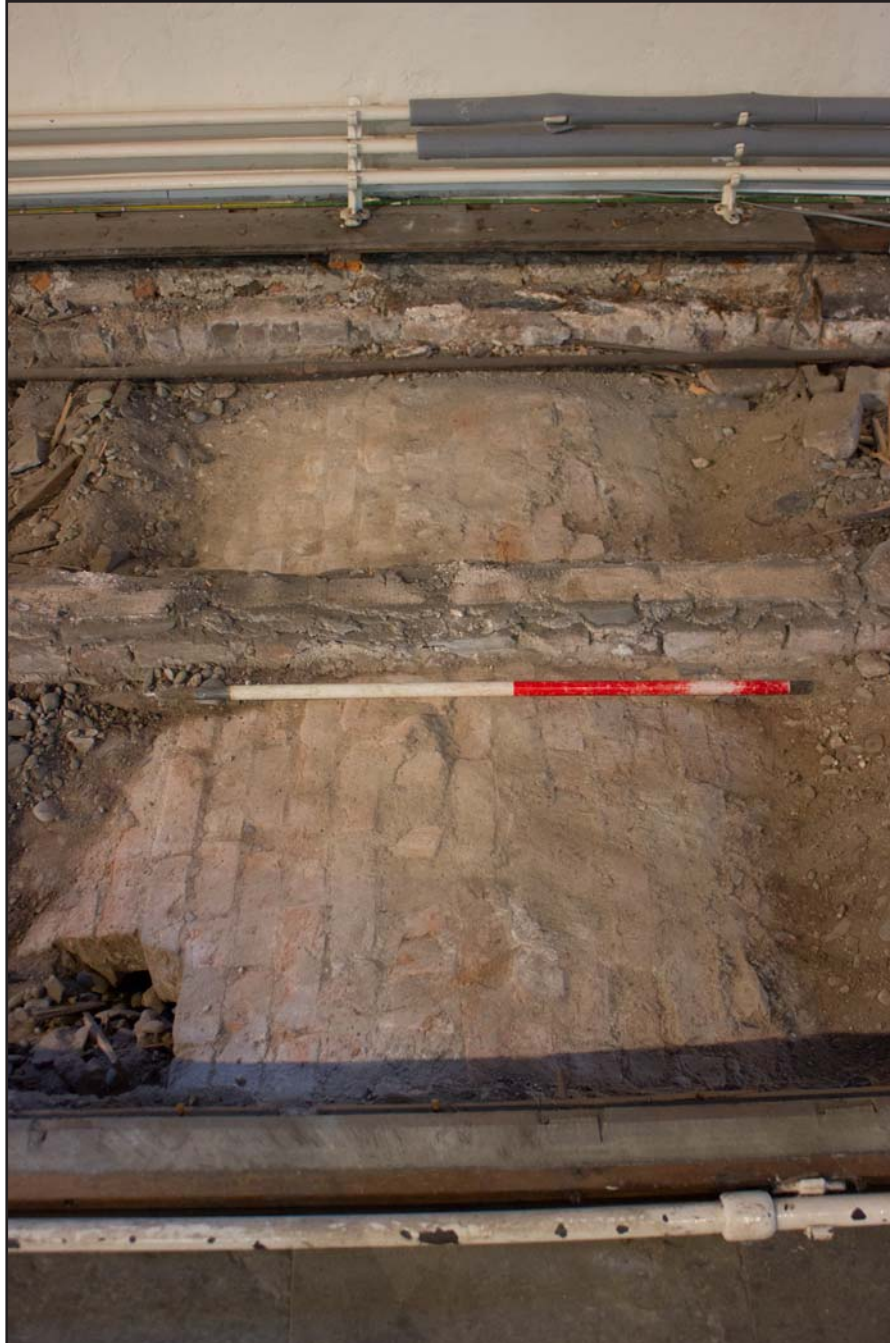
Plate 17: Second brick vault found below northern floor at St. Asaph Parish Church, St. Asaph, Denbighshire - from the south - scale 1m
