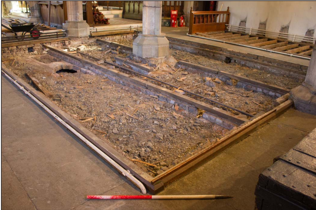
Plate 14: Floor removed in centre of church - from the southeast - scale 1m
