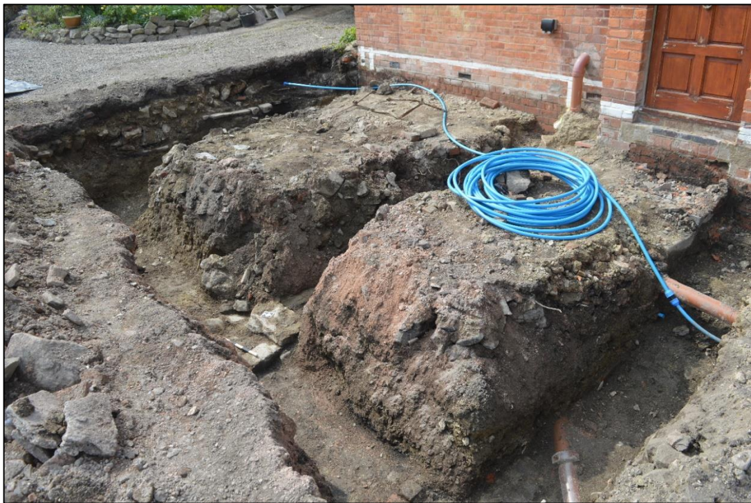
Fig. 5: Excavated footings viewed from the north-east. Photo CPAT 4638-0012
