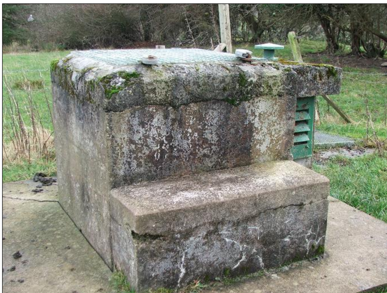
Plate 22. Detailing view of entrance stack leading into main subterranean bunker of Llandrindod Wells ROC UGMP prior to demolition (photograph by Mark Russell, taken 2007)
