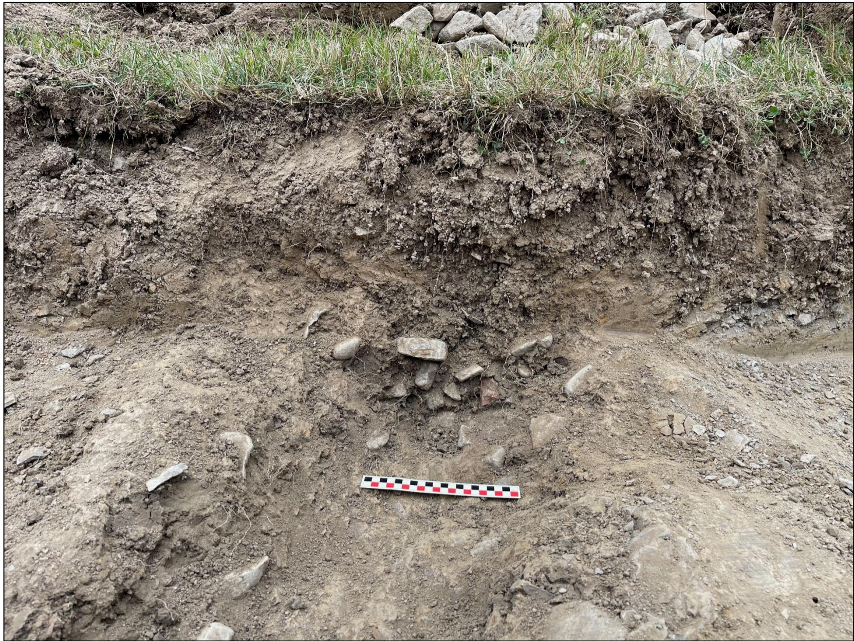
Plate 7. North facing view of land drain [207] cutting natural deposits (203) and (204) (in Trench 2)
