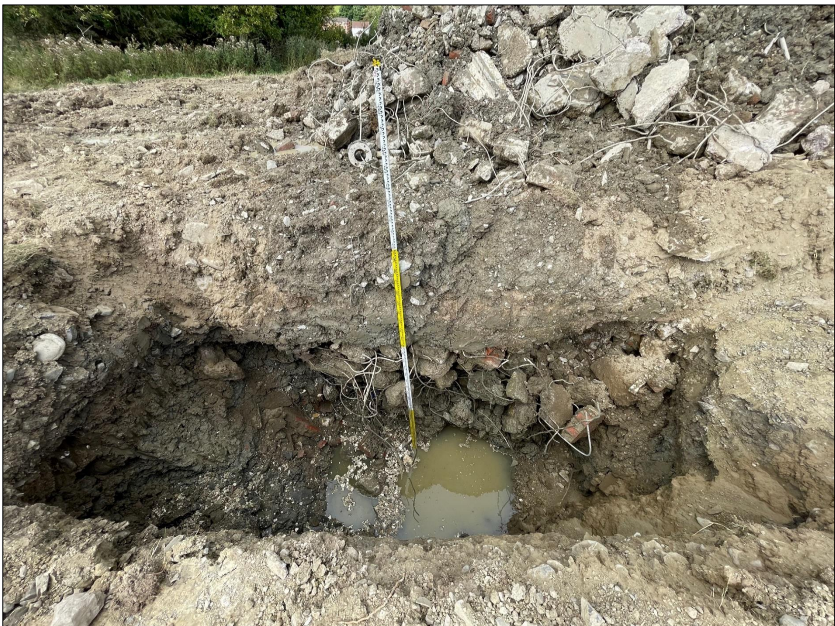
Plate 16. East facing view of fill (402) within cut [401] (in Trench 4a)
