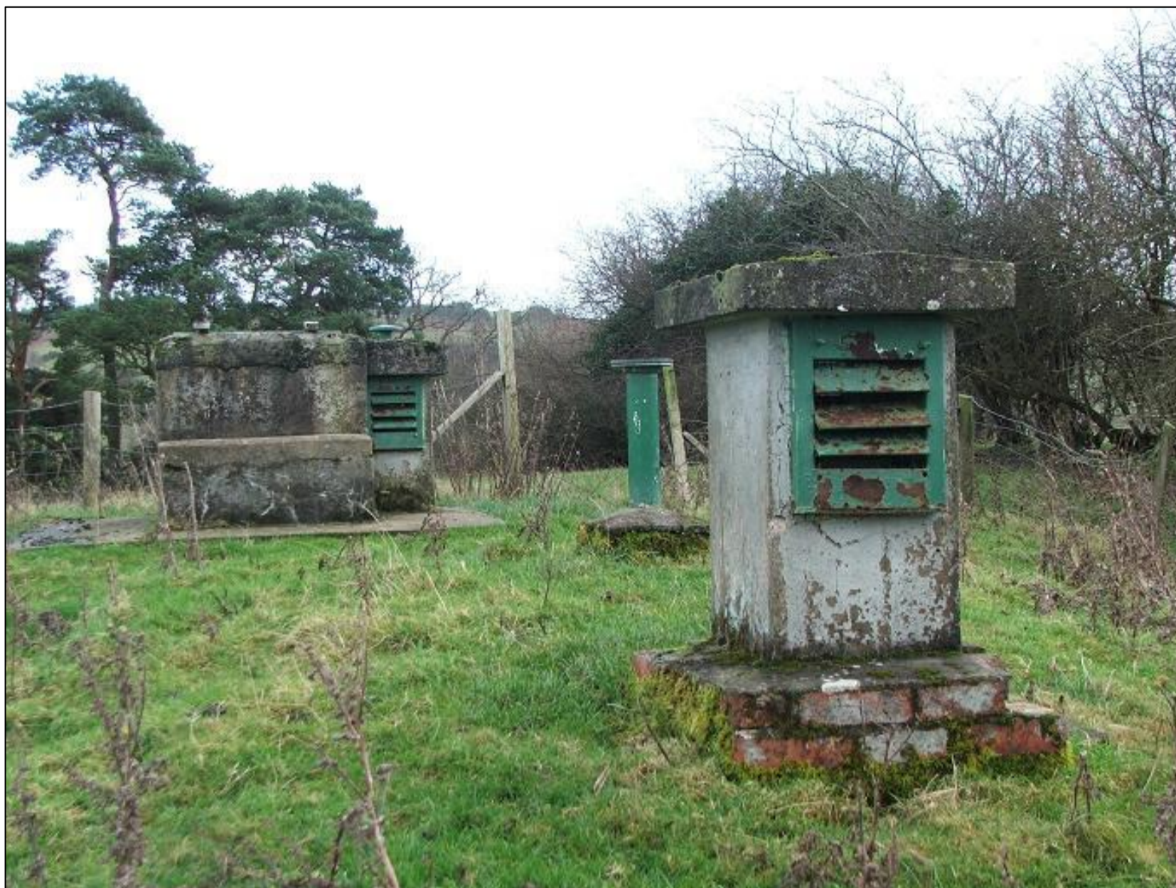
Plate 21. South facing view of surviving elements of the Llandrindod Wells ROC UGMP prior to demolition (photograph by Mark Russell, taken 2007)
