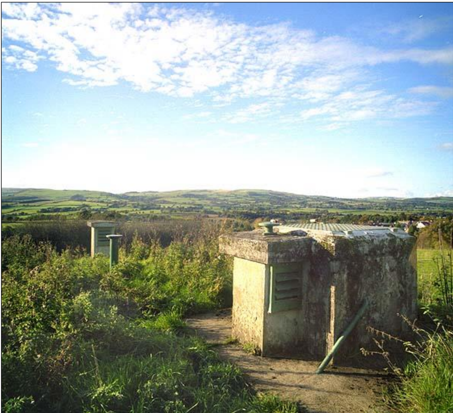
Plate 20. Northwest facing view of surviving elements of the Llandrindod Wells ROC UGMP prior to demolition (unknown date, although post-1991) (photograph by Nick Catford)
