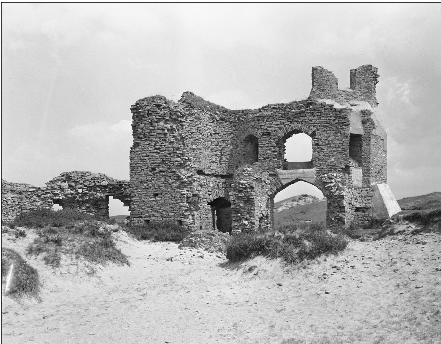
Plate 19 – View of the Gatehouse interior June 1941 (Archive No. 6351162) with 1923-4 concrete repairs. © Crown Copyright: Royal Commission on the Ancient and Historical Monuments of Wales.
