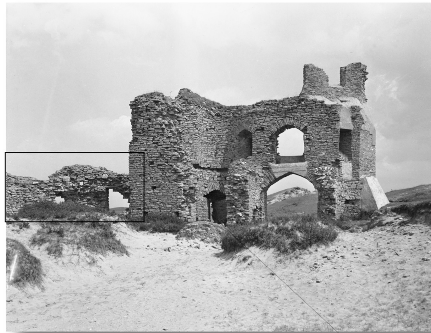
Significant area of curtain wall masonry collapse post-1952.
