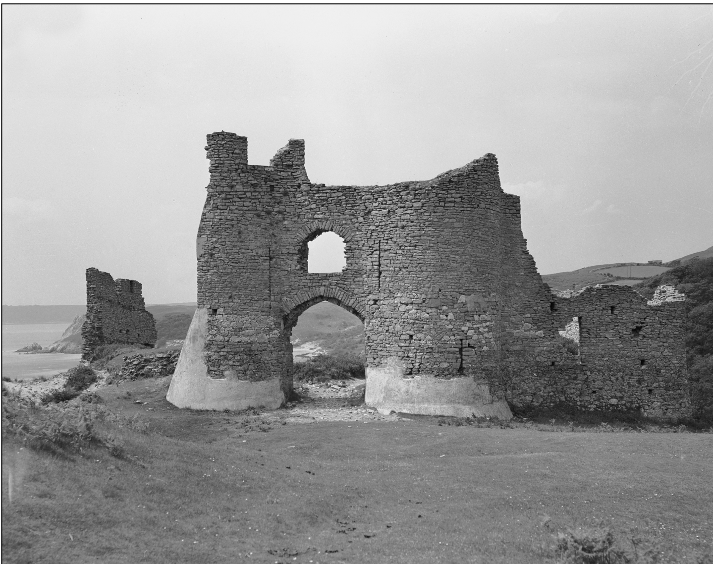
Plate 18 – View of the Gatehouse June 1941 (Archive No. 6351166) with 1923-4 concrete repairs. © Crown Copyright: Royal Commission on the Ancient and Historical Monuments of Wales.
