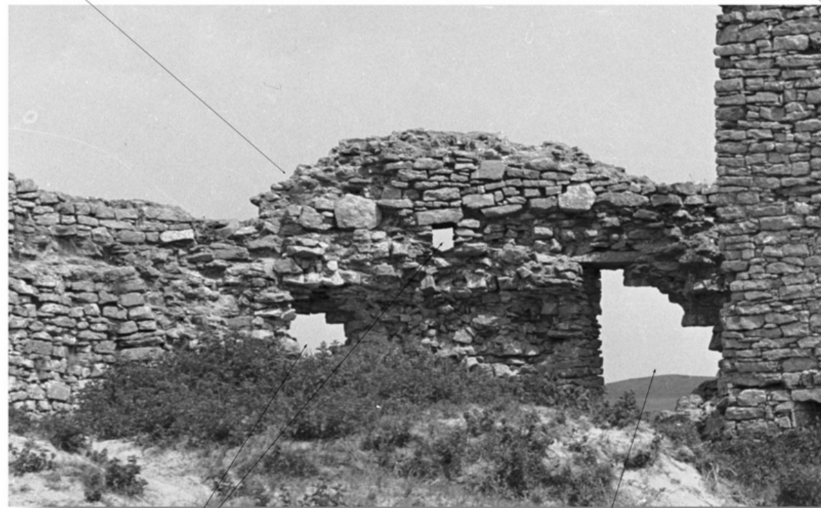
Significant area of curtain wall masonry collapse post-1952.
