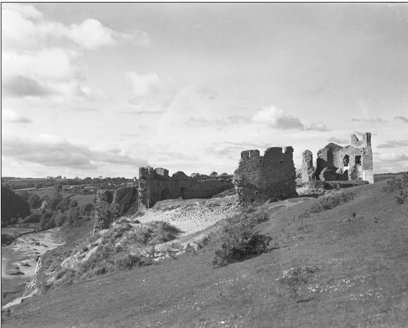
Plate 21 – View of the Pennard Castle, south and north curtain walls, square tower and gatehouse interior June 1941 (Archive No. 6351170) with 1923-4 concrete repairs. © Crown Copyright: Royal Commission on the Ancient and Historical Monuments of Wales.
