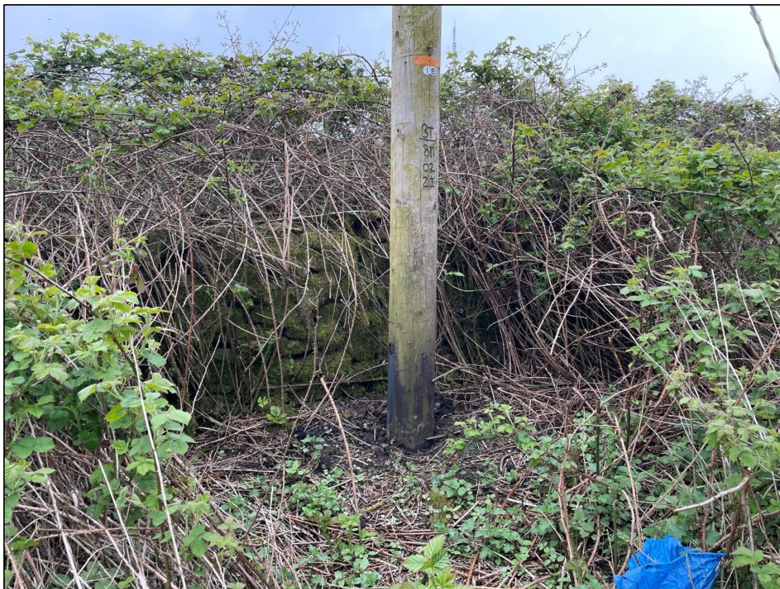
Plate 43. Existing telegraph pole on proposed power line route respecting the extant stone wall field boundary between Maesteg Golf Club and Cwmcerwyn Farm.
