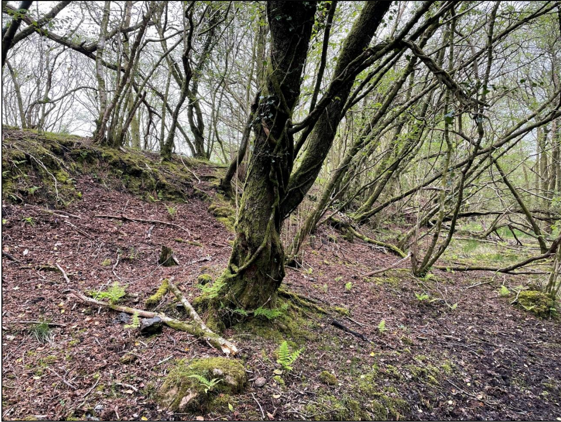
Plate 49. E facing view of Cwmceryn Tramway/ Port Talbot Railway (HA3) embankment adjacent to the proposed power line route.
