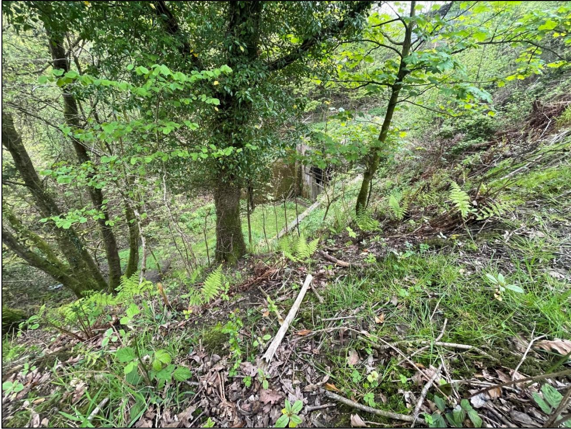
Plate 45. SW facing view of Cwmceryn Tunnel eastern entrance (HA34).
