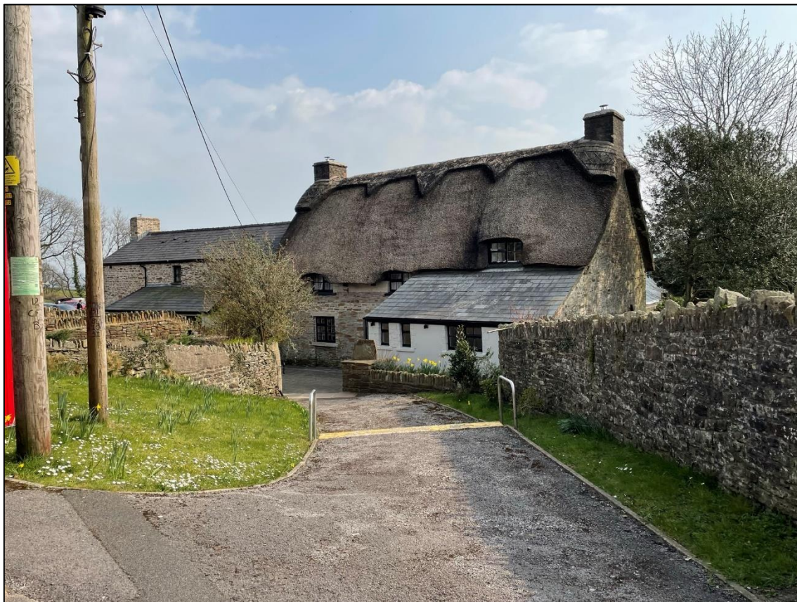
Plate 70. SE facing view of Old House Inn, Llangynwyd (HA44)
