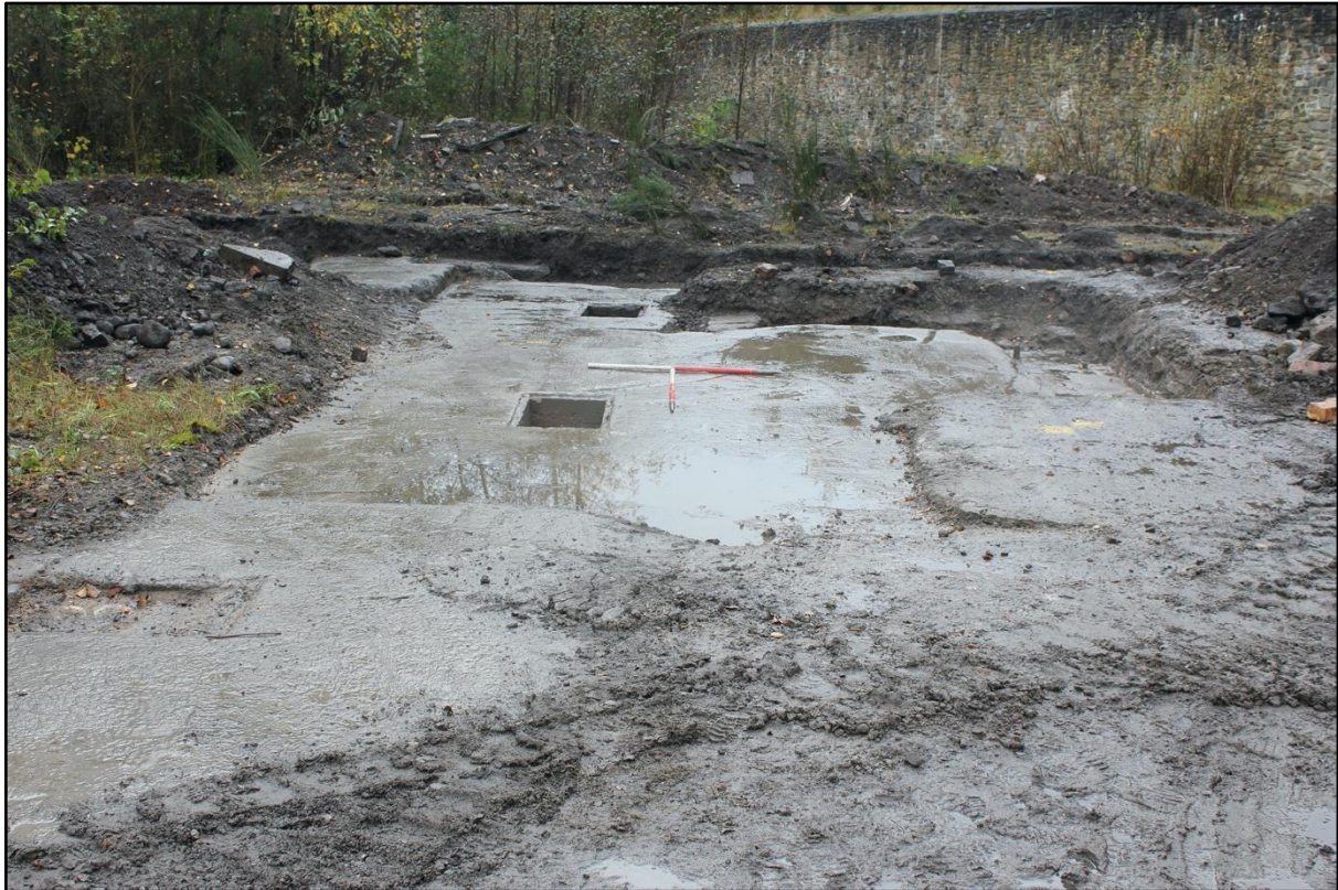
Plate 47. South facing view of Trench 5
