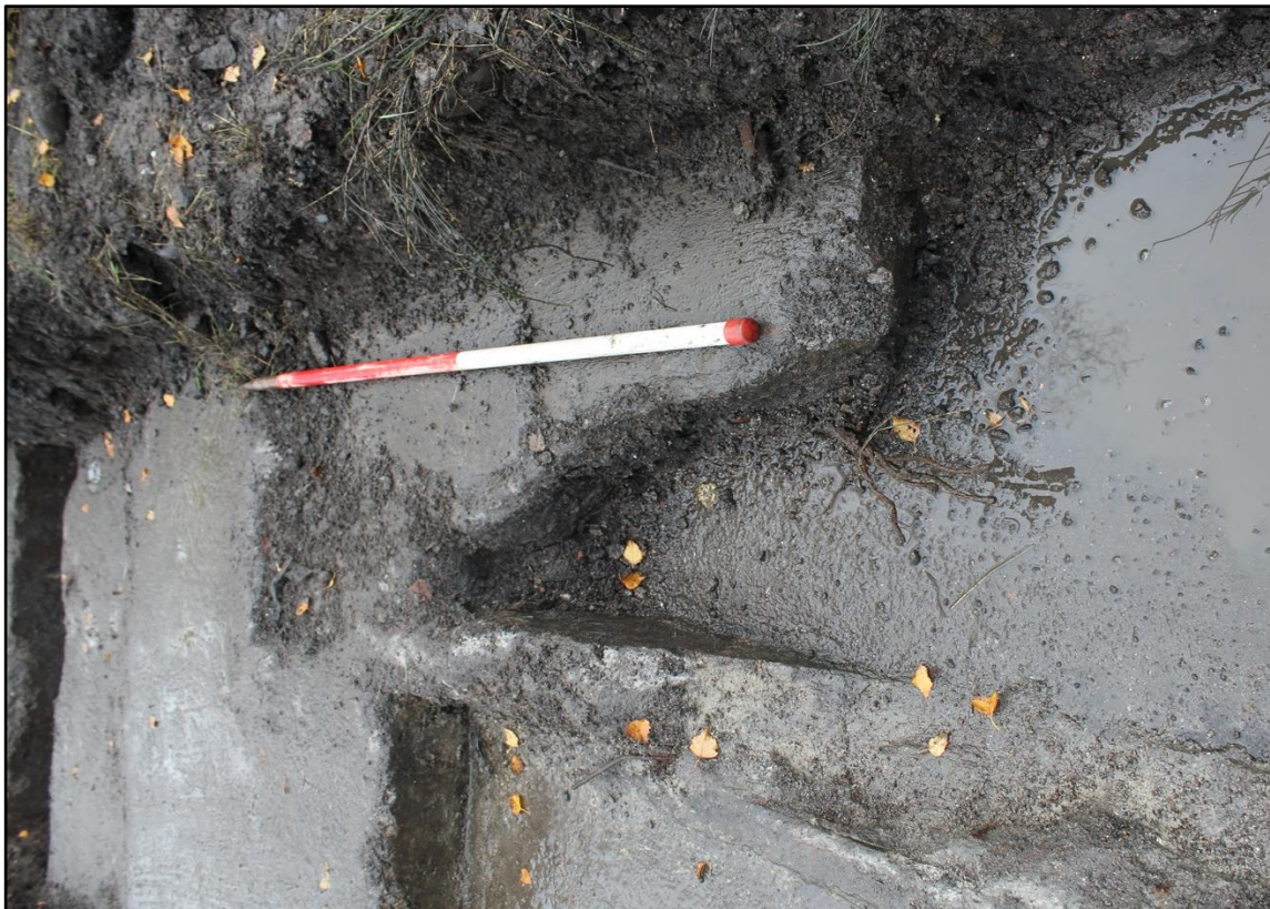
Plate 68. Electric cable entry into machine base [615] (view east)
