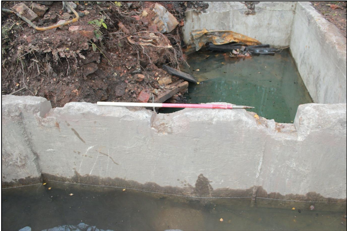
Plate 11. Eastern wall of hot well [141] in Trench 1 (view west)
