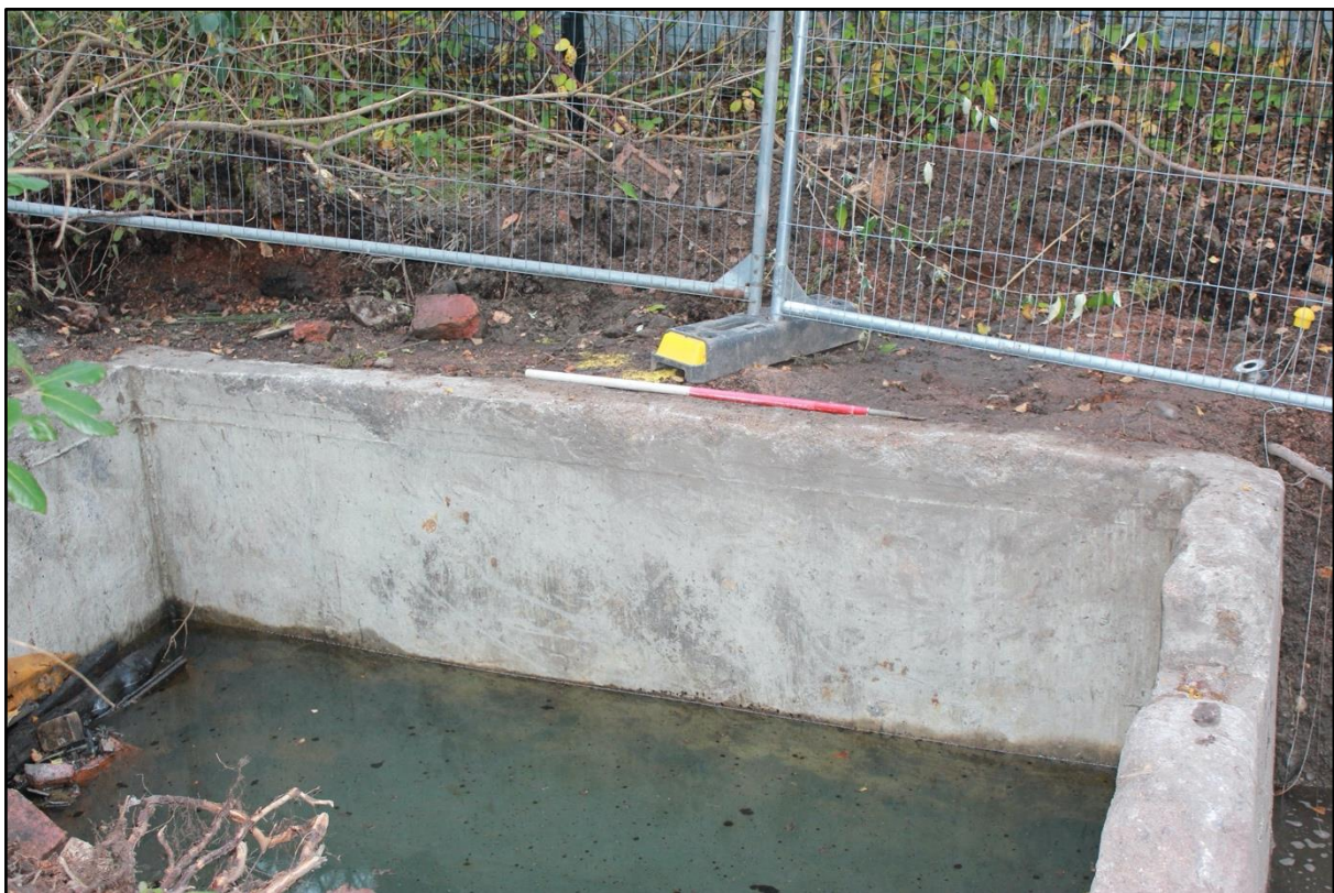
Plate 14. Northern wall of hot well [141] in Trench 1 (view north)
