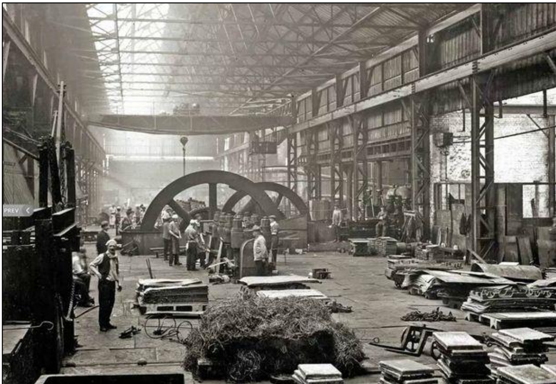
Plate 86. 20 th century photograph depicting the line of operations within the Hafod Plate Mill (copyright West Glamorgan Archives)
