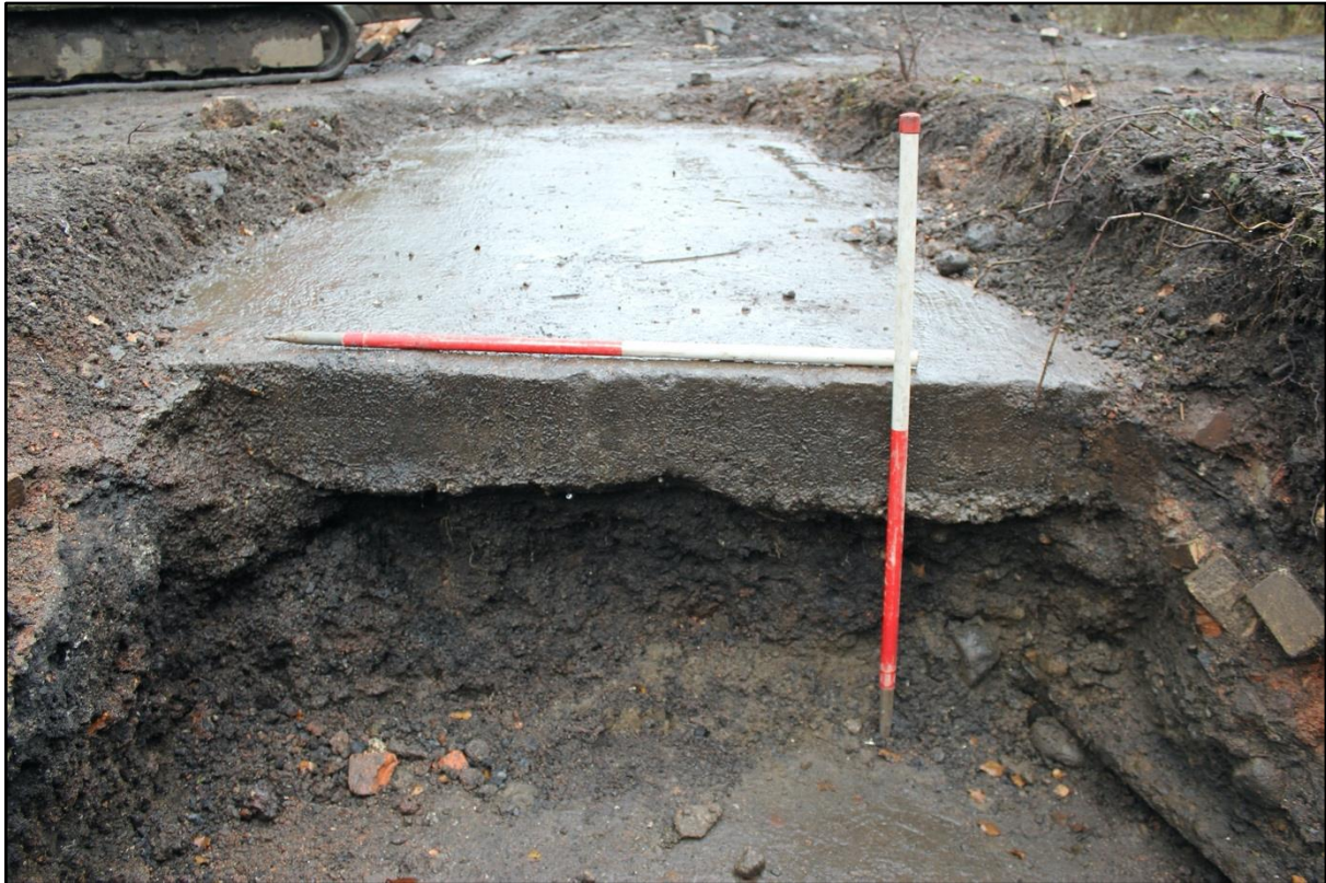
Plate 33. Concrete [302] overlying deposit (326) in Trench 3 (view southwest)
