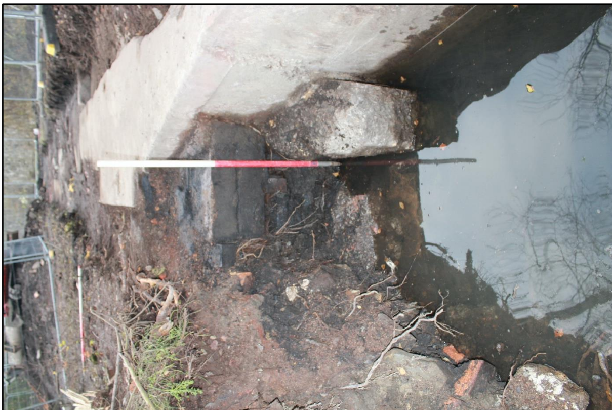
Plate 10. Culvert [115] in Trench 1 (view southwest)
