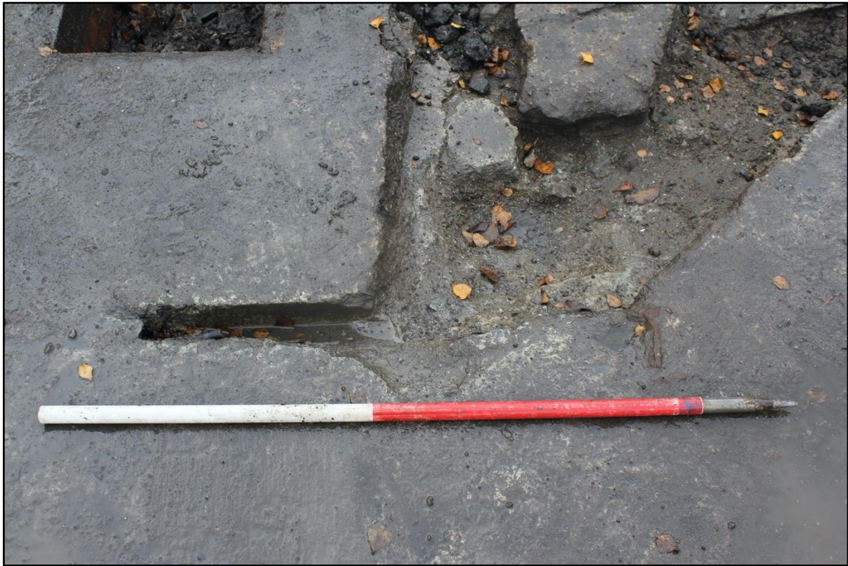
Plate 51. Cable inlet incorporated into machine base [504] and RSJ [511] in Trench 5 (view south)
