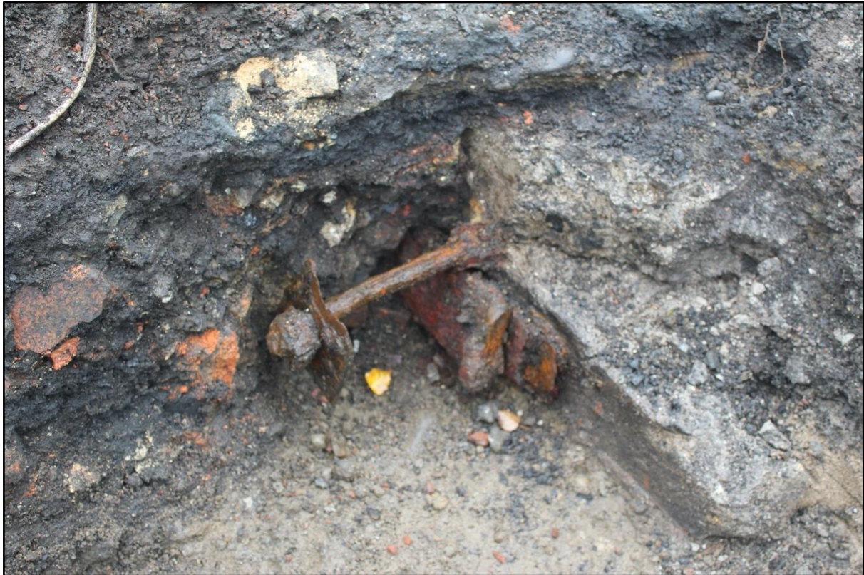
Plate 63. Close-up view of tie bar and anchor plate incorporated into wall [612] in Trench 6 (view southeast)
