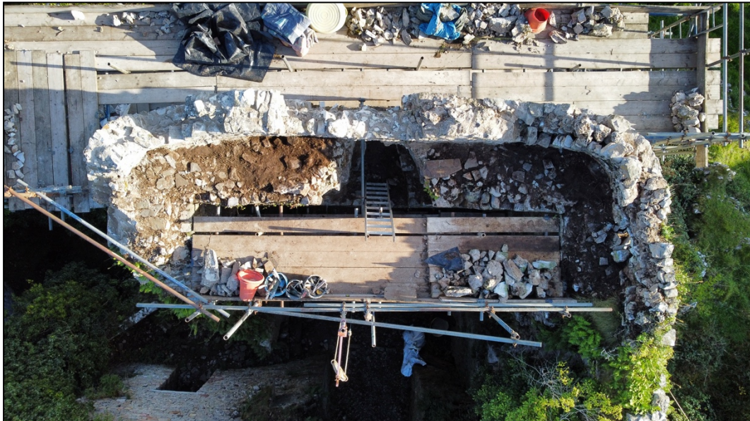
Plate 12. Gatehouse during masonry conservation and following archaeological investigation. Nadir view.
