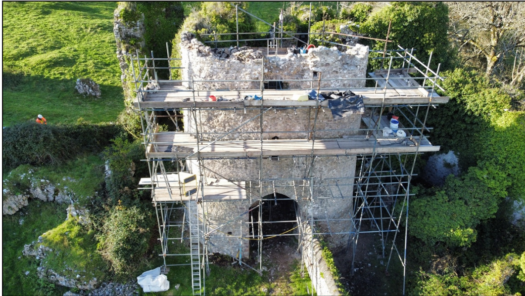
Plate 13. Gatehouse during masonry conservation and following archaeological investigation. View to NW.
