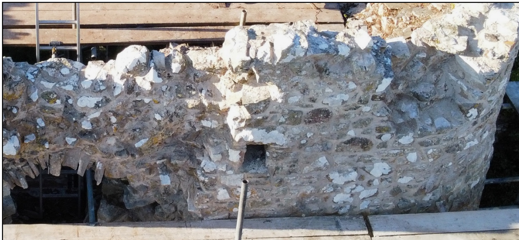
Plate 6. Wall Walk Drain [006] (NE side), view to NW.
