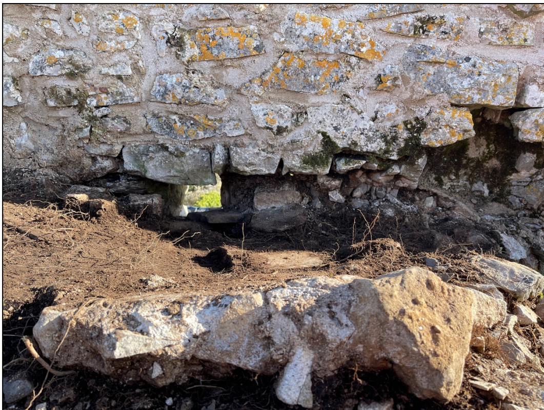
Plate 5. Wall Walk Drain [006] (NE side), view to SE following archaeological investigation.
