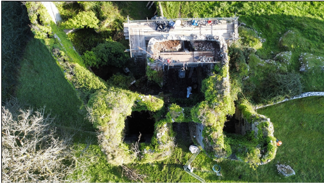
Plate 11. Gatehouse during masonry conservation and following archaeological investigation. Nadir view.
