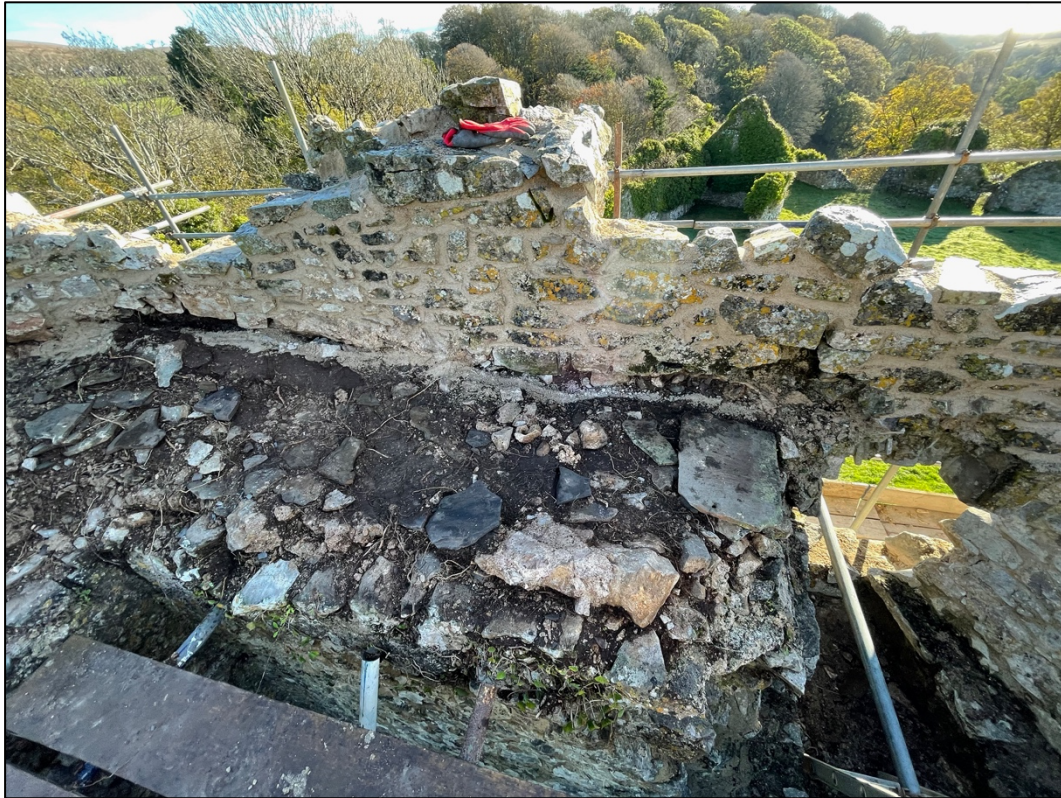
Plate 2. Wall walk (NE side) along the south eastern internal wall of the gatehouse during masonry conservation and prior to archaeological investigation.
