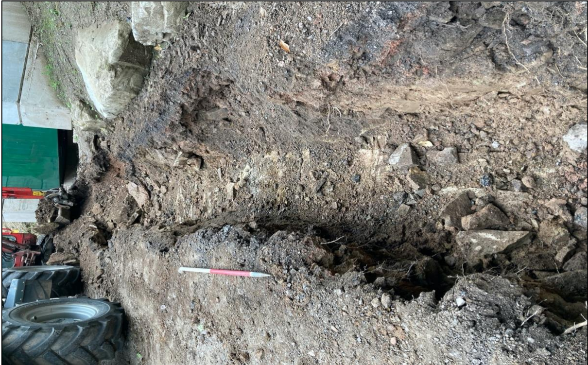
Plate 13. Excavations along trackway leading to newly installed substation (view southeast)
