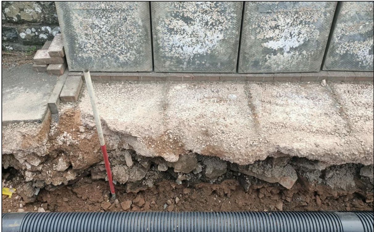
Plate 9. Excavation through bus stop on northern side of A466 (south-facing section).
