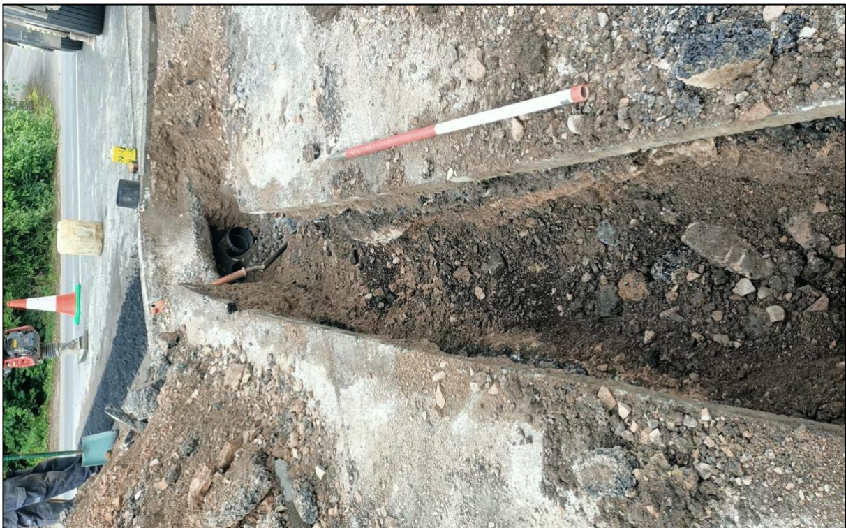
Plate 4. Excavations through pavement on north side of A466 (view east)
