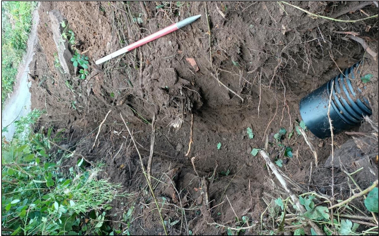
Plate 3. North-facing view of excavations within Abbey Farm
