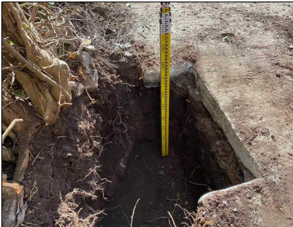
Plate 6. Test Pit 6 (view southwest)
