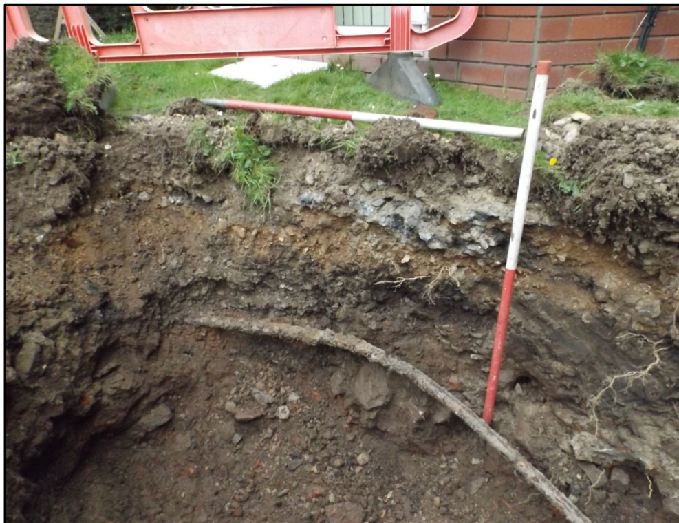
Plate 4. South-facing section of northern end of excavation area, showing concrete (010) below topsoil (001)
