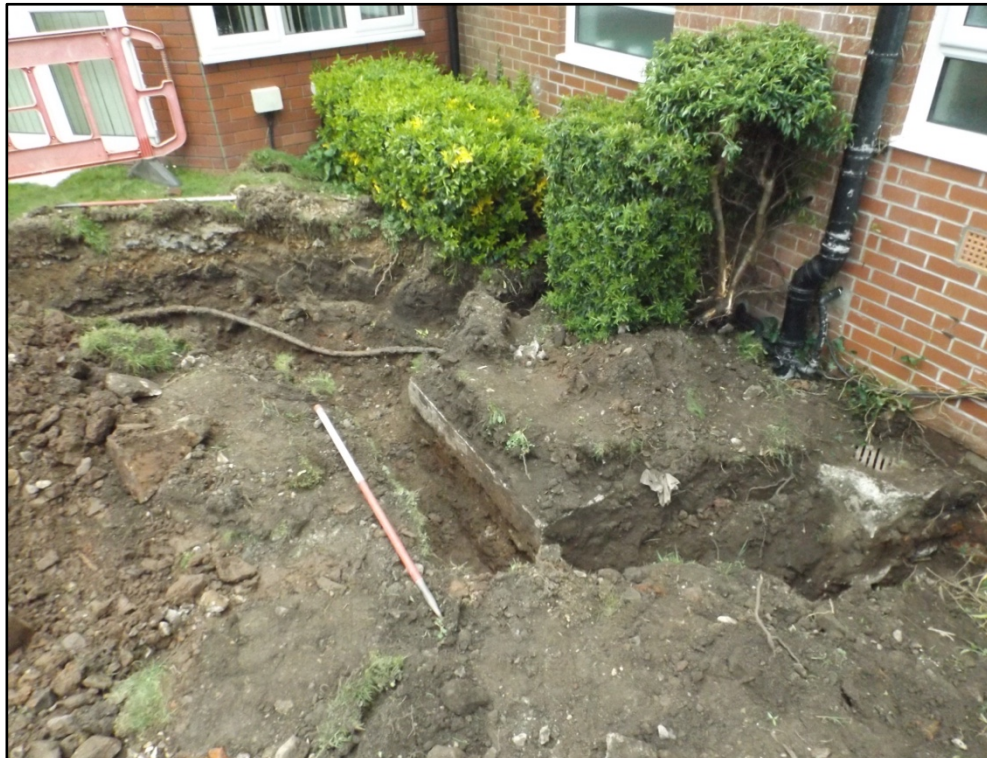
Plate 7. Plan view of excavation area (view northeast)
