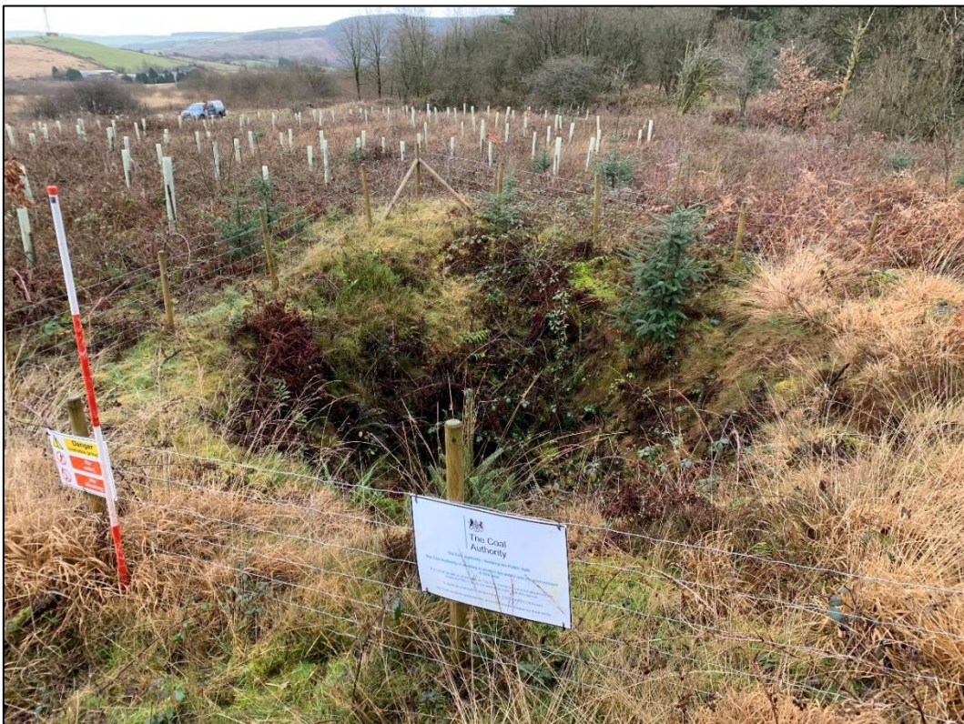
Plate 56. Air shaft on site of Ton-hir Colliery complex (HA02).
