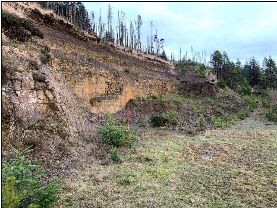
Plate 64. Northeast facing view of quarrying on site of Garn-wen Quarry (HA26) .
