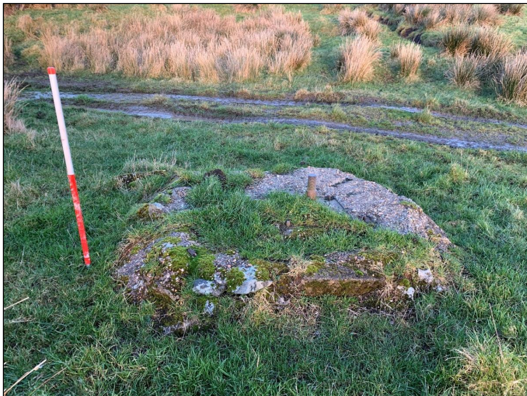
Plate 49. Concrete machine base with fixing bolts, possibly for winding gear, on site of extractive activity on Foel Trawsnant (SW of track) (HA47).
