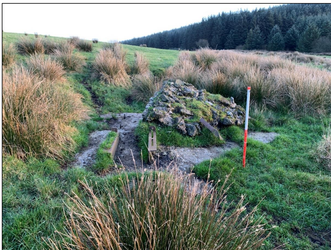
Plate 50. Remains of concrete structure with fixing bolts and steel brackets, possibly related to winding gear, on site of extractive activity on Foel Trawsnant (NE of track) (HA47).
