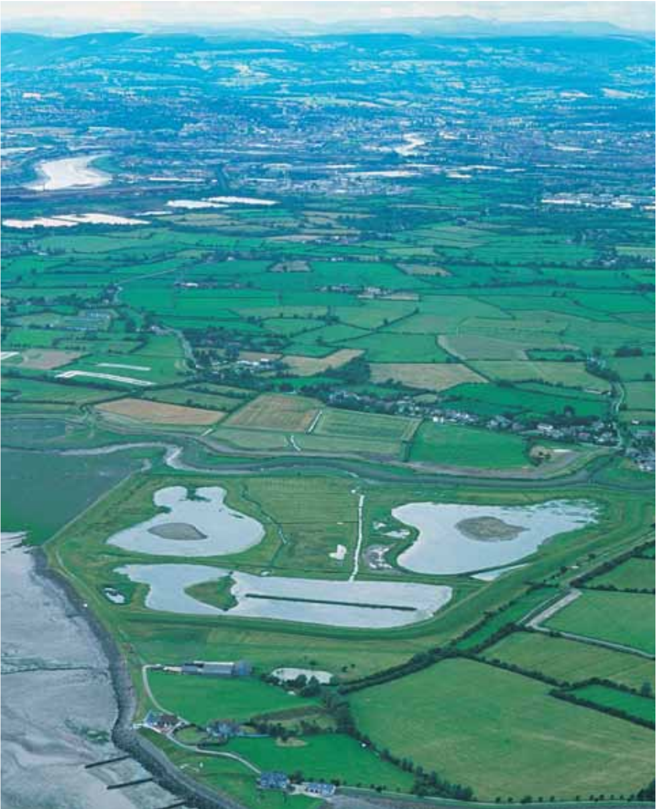
An aerial view of the lagoons and reedbeds of the Gwent Levels Wetland Reserve created to replace habitats lost when the Cardiff Bay Barrage was constructed. The reserve has been successfully integrated into the pattern of the Gwent Levels historic landscape (© RCAHMW).
