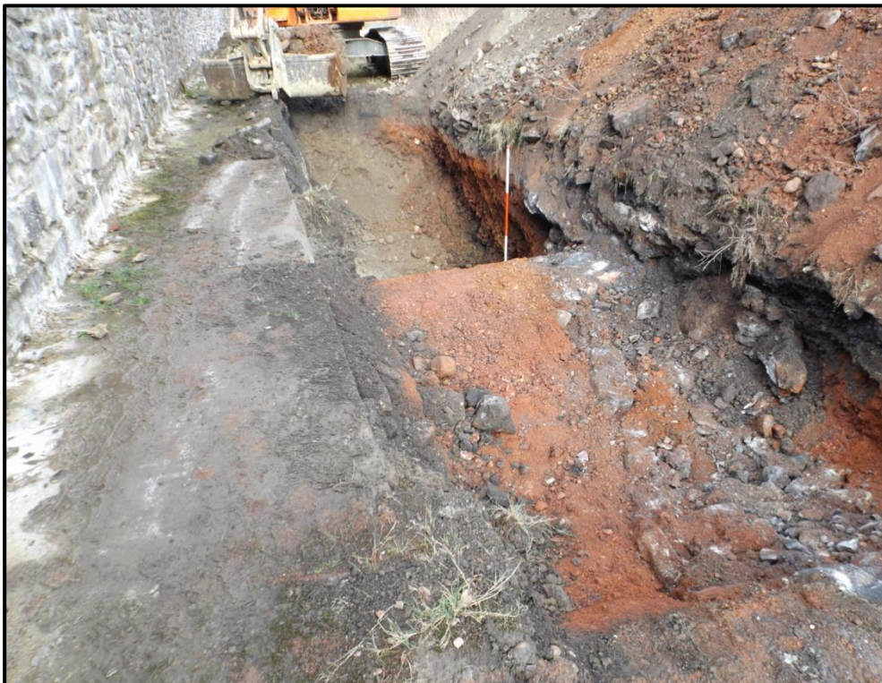
Plate 26. Cut [1206] and fill (1204) in Trench 12 (view north)
