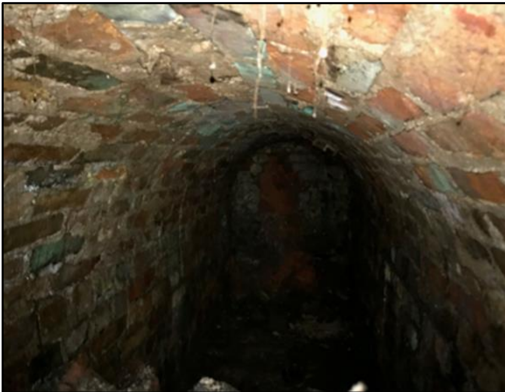
Plate 10. View of interior of culvert [309] in Trench 3
