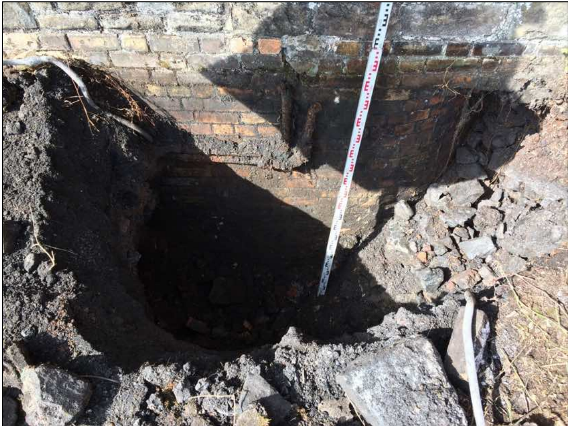
Plate 31. North East facing section of Test Pit 16 showing Porter's Lodge foundations and earlier wall [1602] with its curved feature to the right of the picture.
