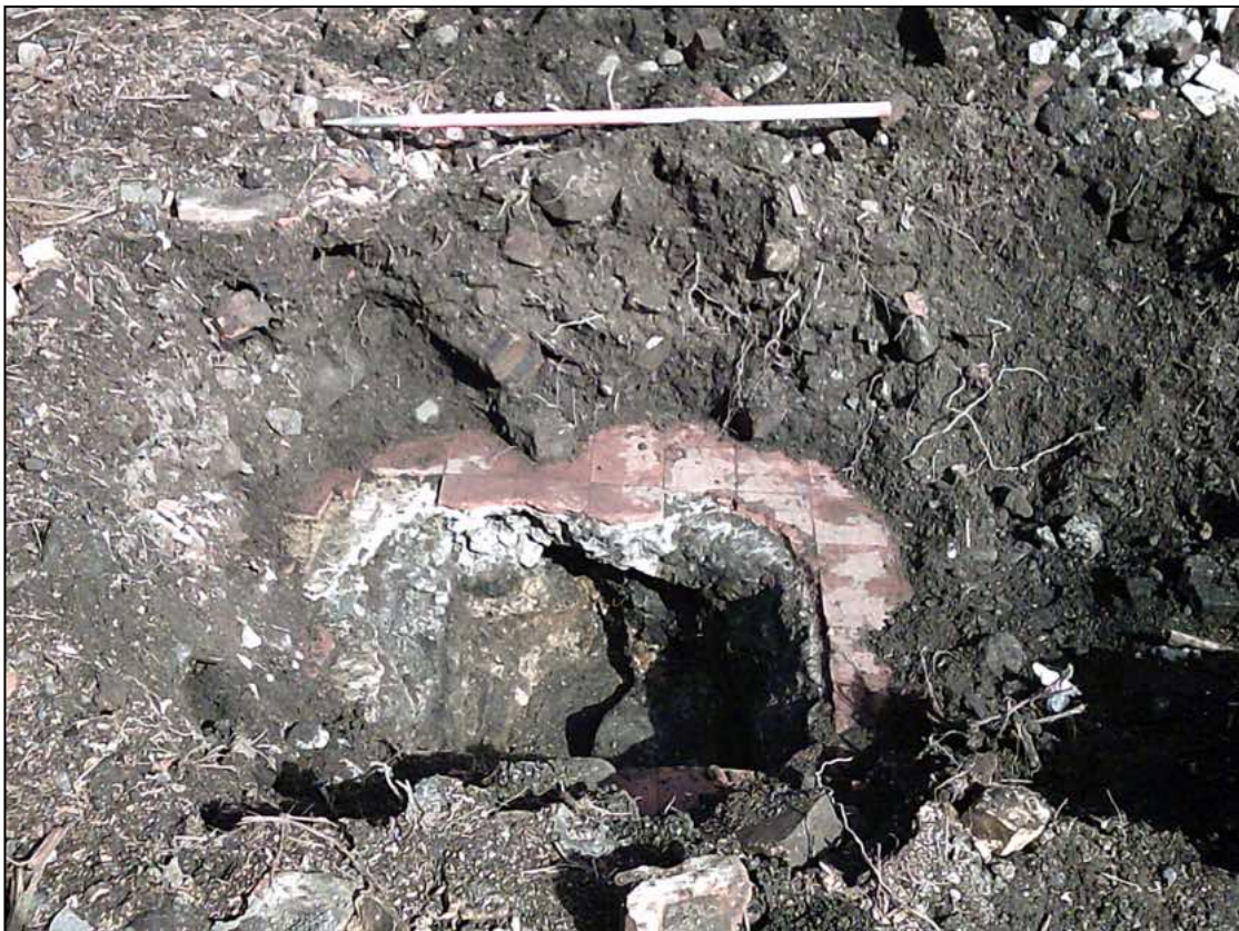
Plate 6. South facing section of Test Pit 2 showing quarry tile floor [202] and masonry structure [205].
