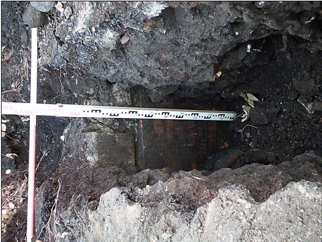
Plate 23. East facing section of Test Pit 14 showing the west wall of the weighbridge [1404] and concrete kerb [1303]. Also showing demolition rubble infill deposit (1402).
