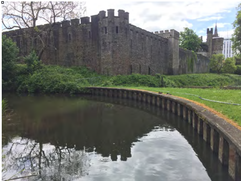
Plate 4. View to SE of Bute Dock Feeder Canal (01682.28s) as it turns east from Bute Park to the development area utilising Cardiff Castle's moat.
