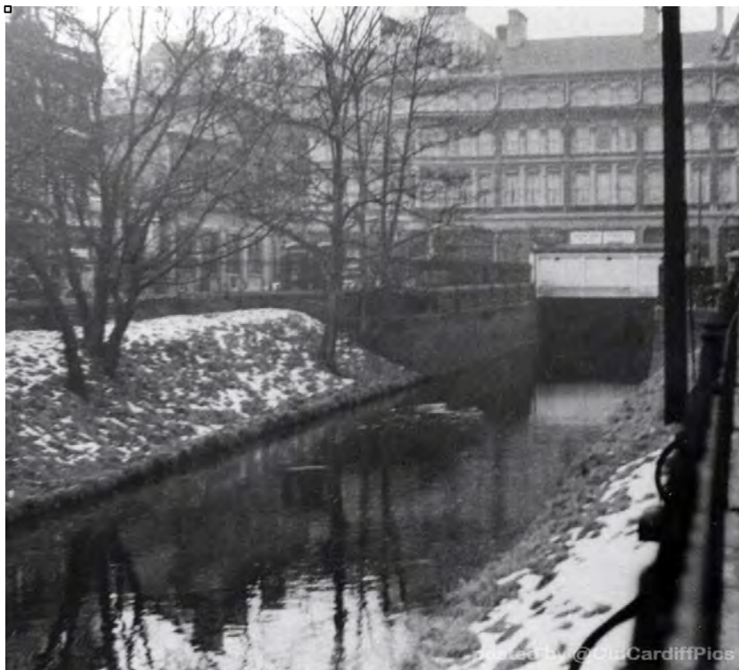
Plate 6. View to N of Bute Dock Feeder Canal (01682.28s) canalised under Park Hotel, with Edward and Pembroke Terraces either side.
