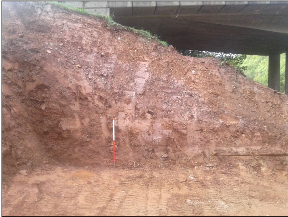
Plate 7. E facing section of Reduced Area 1 in Area A (view W).
