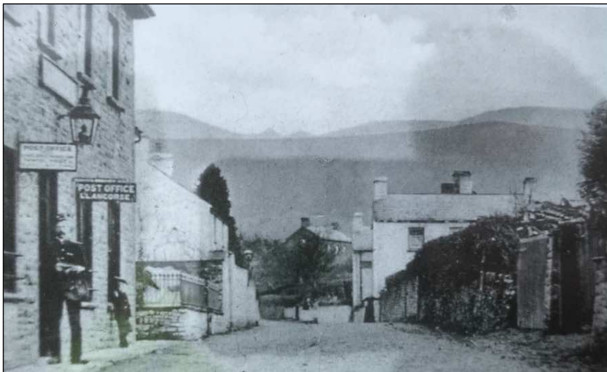
Plate 1. Postcard (1890s) showing main road to Bwlch through Llangorse with the old Post Office to the left and the development area to right.
