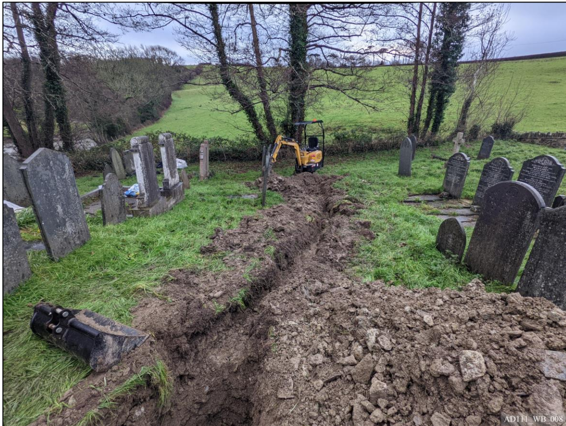
Plate 8 – View south, showing extent of excavations.
