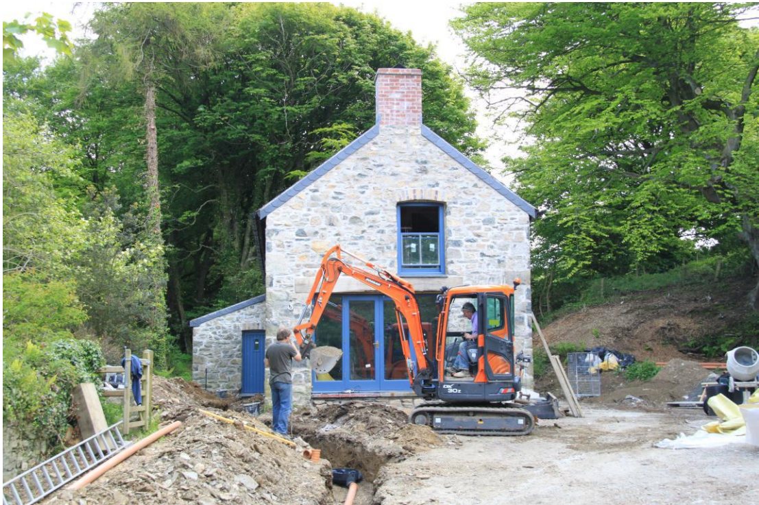
Plate 69 - AD010-D3-022 - View towards Former Coach House showing location of service trench 2.
