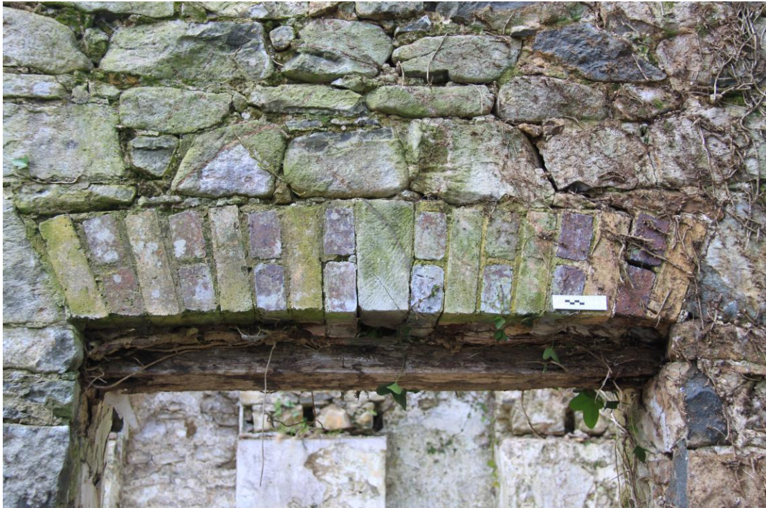
Plate 14 - AD010-BR-014 - Yellow and red brick flat segmental arch to door head, north elevation.
