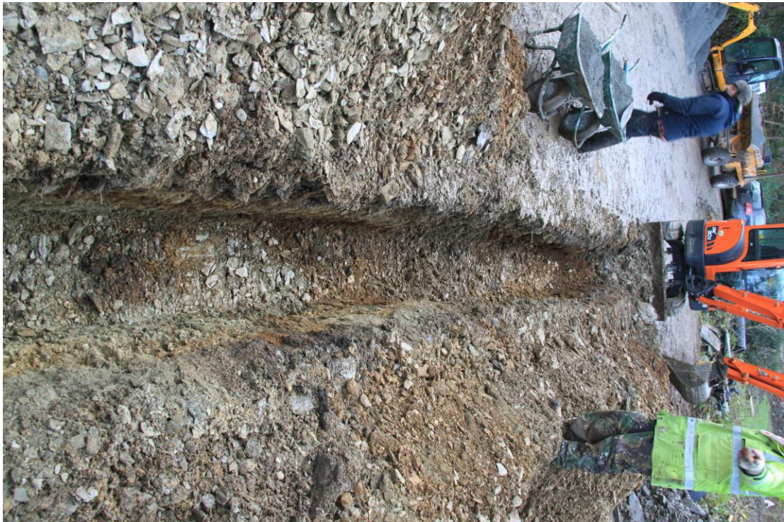
Plate 57 - AD010-D1-010 - Service trench 1 at west end of Former Coach House.
