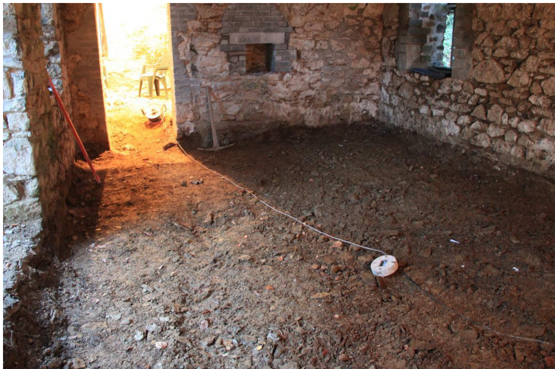
Plate 49 - AD010-D1-002 - Internal excavations for poring of concrete slab, view east.
