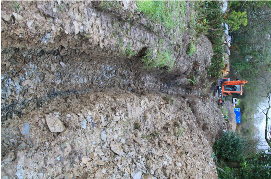
Plate 53 - AD010-D1-006 - Service trench 1 passing Castle Mill.
