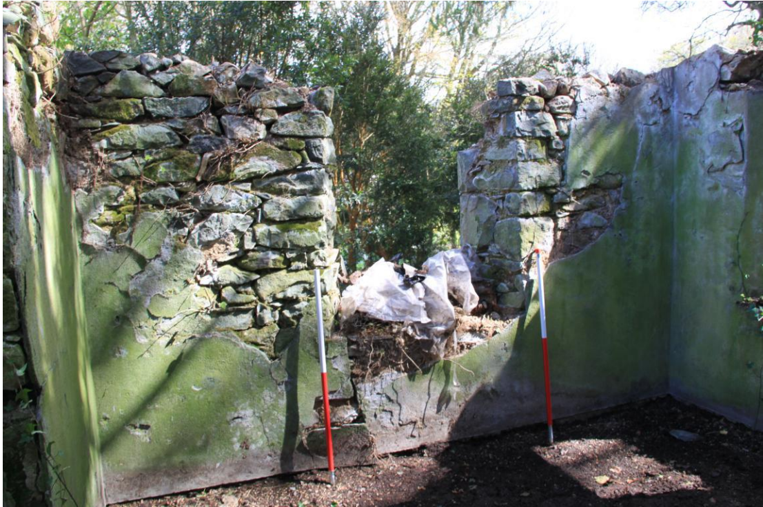
Plate 35 - AD010-BR-035 - Internal view of Extension B towards the north.
