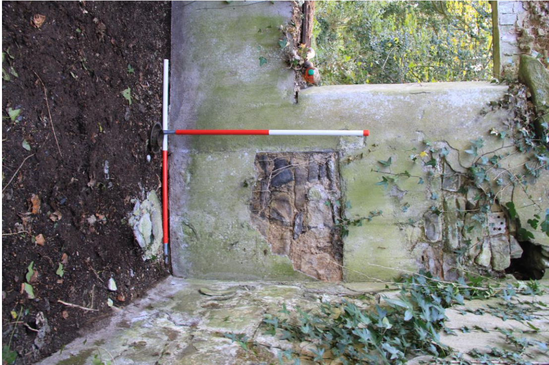
Plate 33 - AD010-BR-033 - Blocked fireplace, Extension B internal, east wall.
