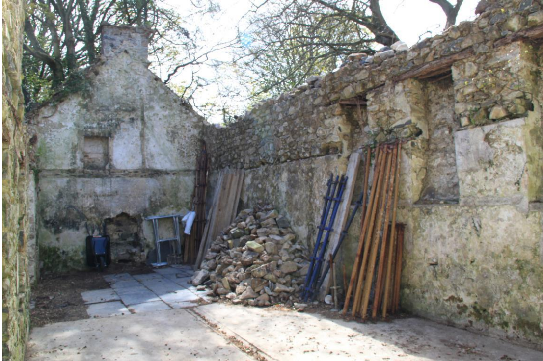
Plate 21 - AD010-BR-021 - Internal of Former Coach House view towards the east.
