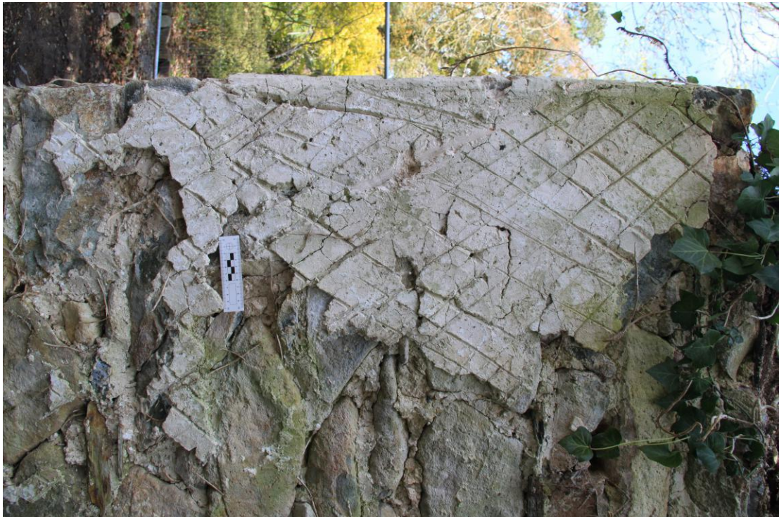
Plate 26 - AD010-BR-026 - Scoring to plaster base coat, internal north wall, Former Coach House.
