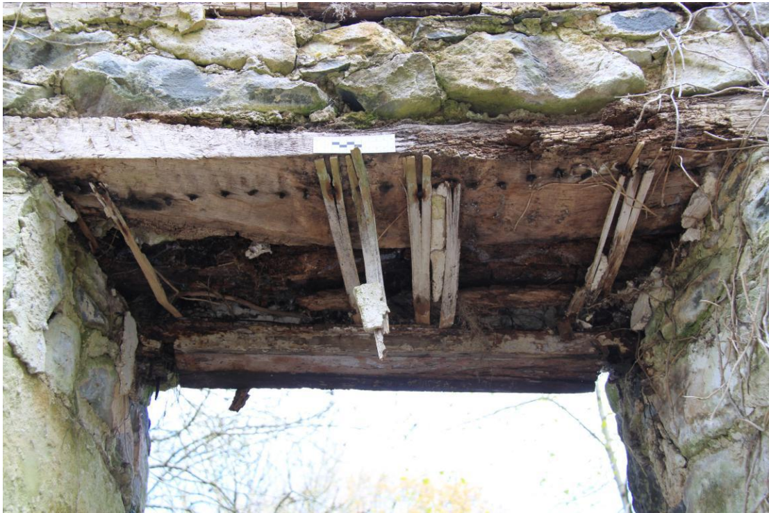
Plate 17 - AD010-BR-017 - Oak window lintel, internal, north wall.
