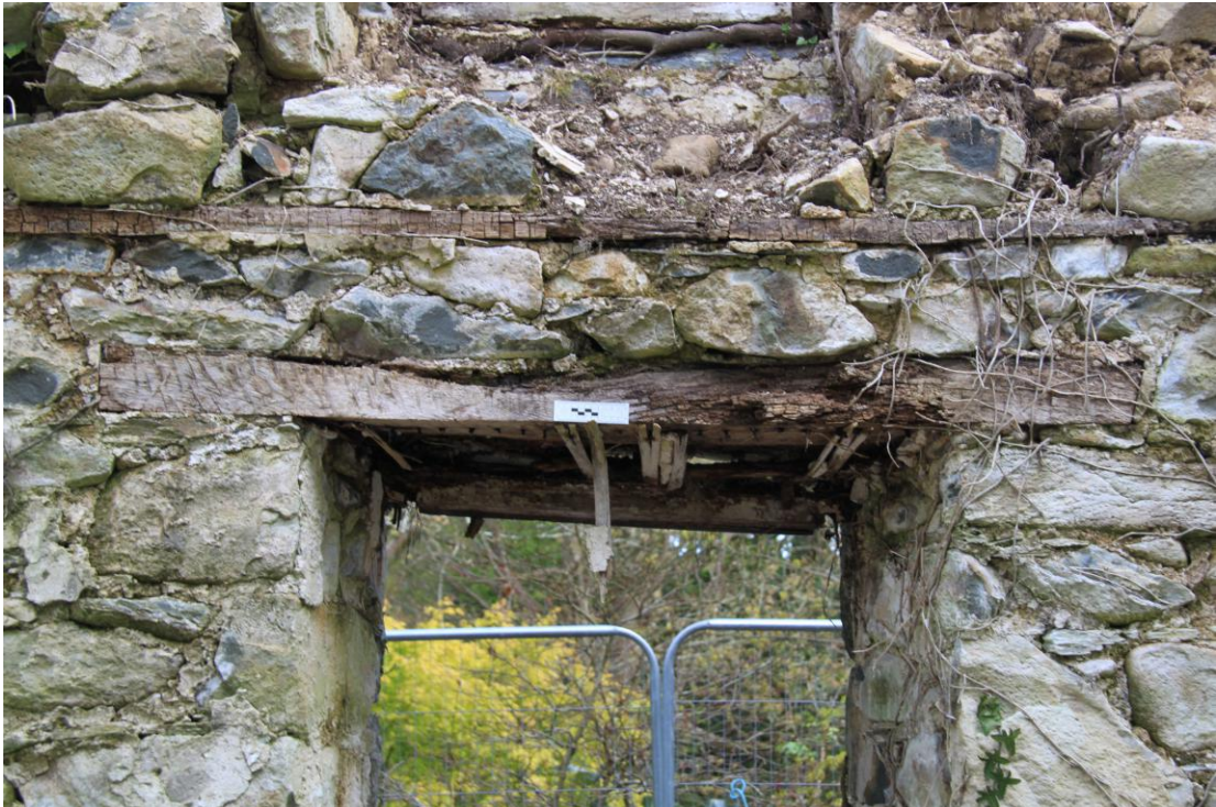
Plate 16 - AD010-BR-016 - Oak window lintel, internal, north wall.
