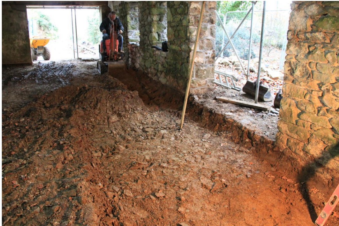
Plate 48 - AD010-D1-001 - Internal excavations for poring of concrete slab, view north-west.
