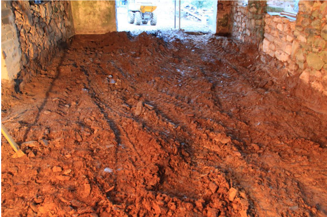
Plate 50 - AD010-D1-003 - Internal excavations for poring of concrete slab, view west.
