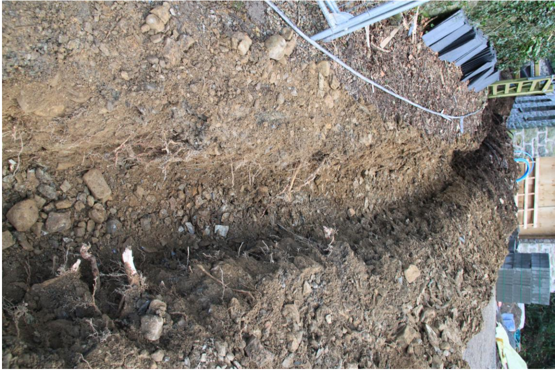
Plate 58 - AD010-D2-011 - Service trench 1 at west end of Former Coach House
