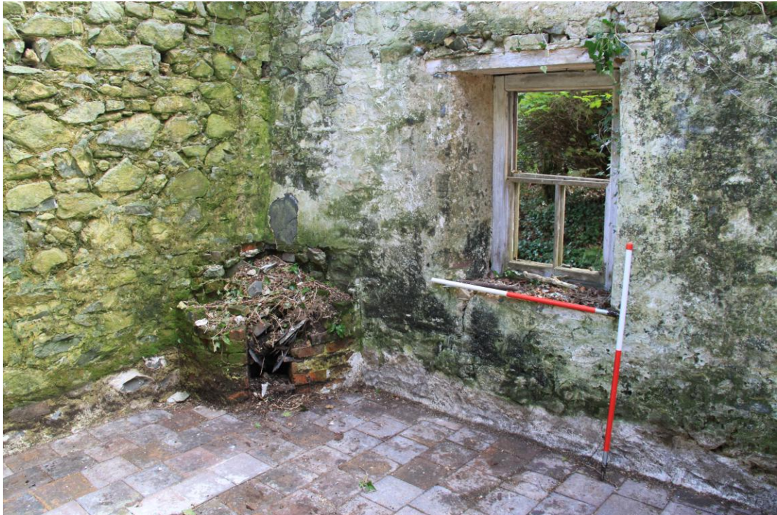
Plate 40 - AD010-BR-040 - Internal view of Extension B towards the east.
