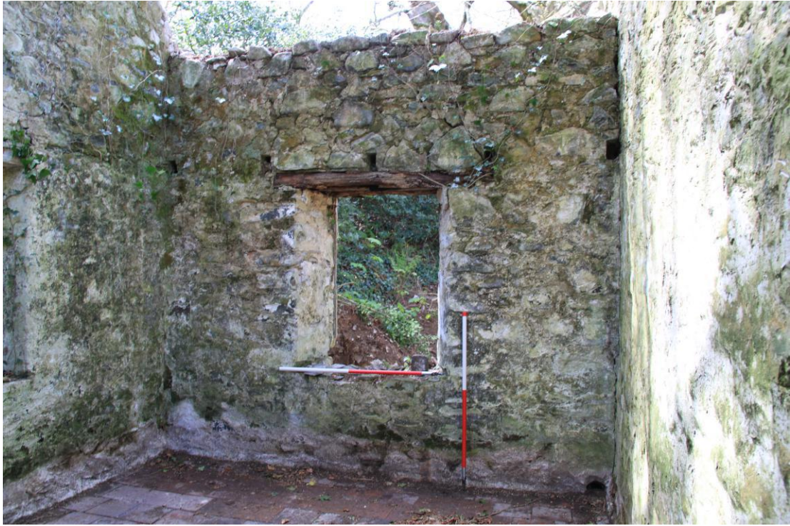
Plate 39 - AD010-BR-039 - Internal view of Extension B towards the south.
