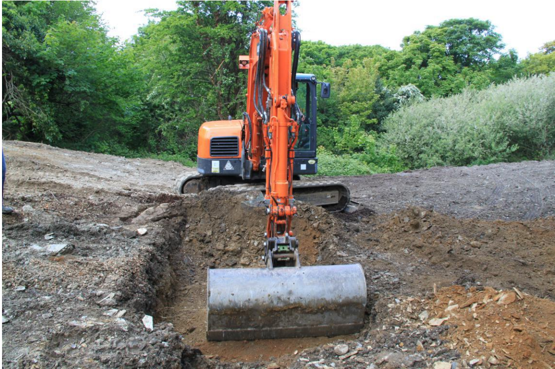
Plate 66 - AD010-D3-019 - Excavation of septic tank pit.
