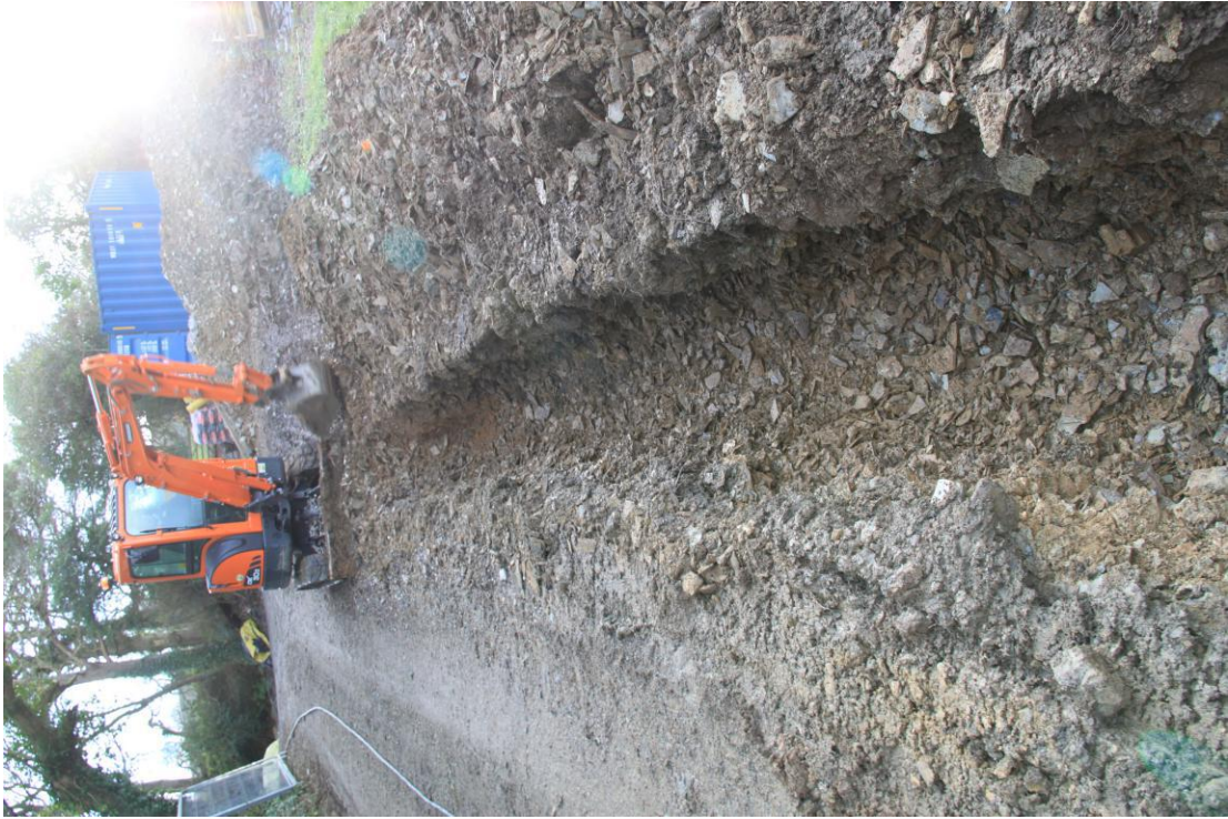
Plate 54 - AD010-D1-007 - Service trench 1 at half way along track.
