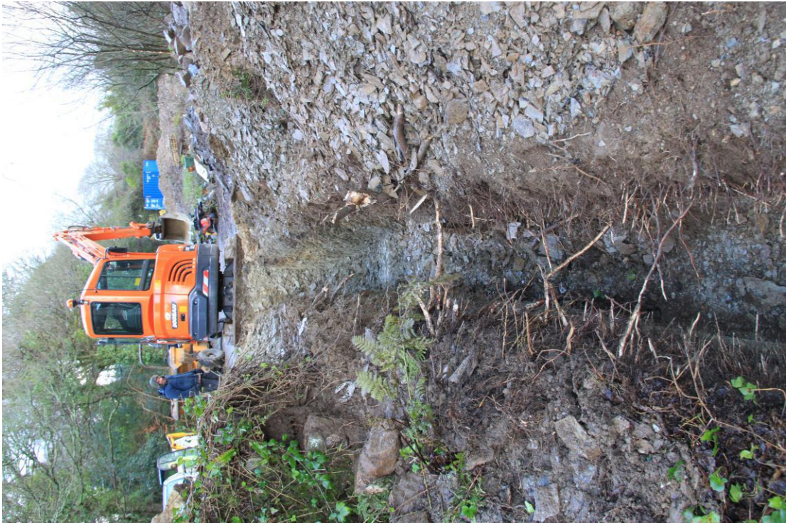
Plate 55 - AD010-D1-008 - Service trench 1 cutting through disused leaf.
