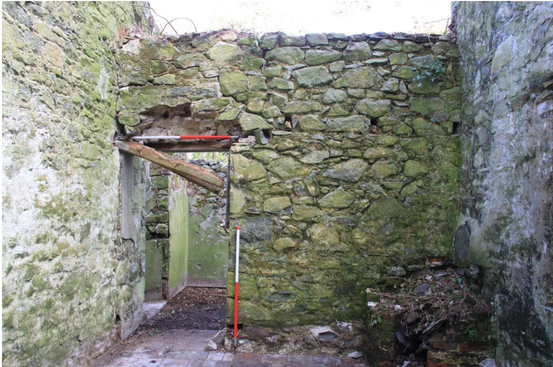
Plate 42 - AD010-BR-042 - Internal view of Extension B towards the north.
