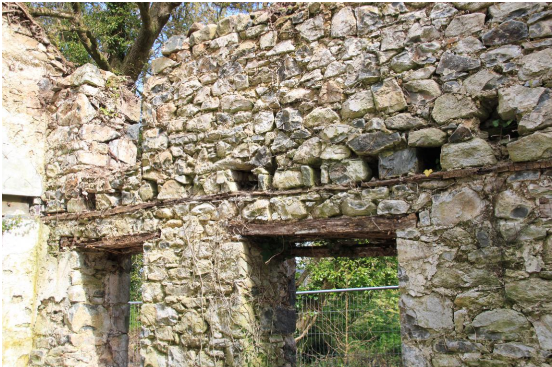
Plate 18 - AD010-BR-018 - Joist sockets, internal, north wall.
