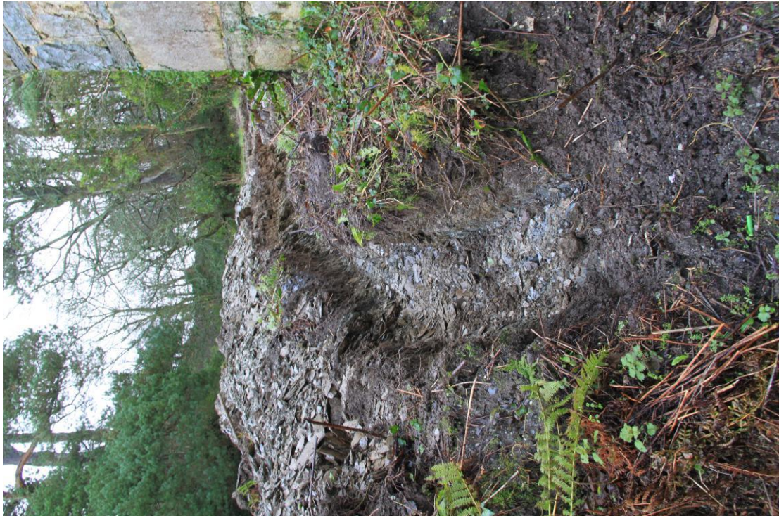
Plate 51 - AD010-D1-004 - Service trench 1 starting at Castle Mill, view south-east.
