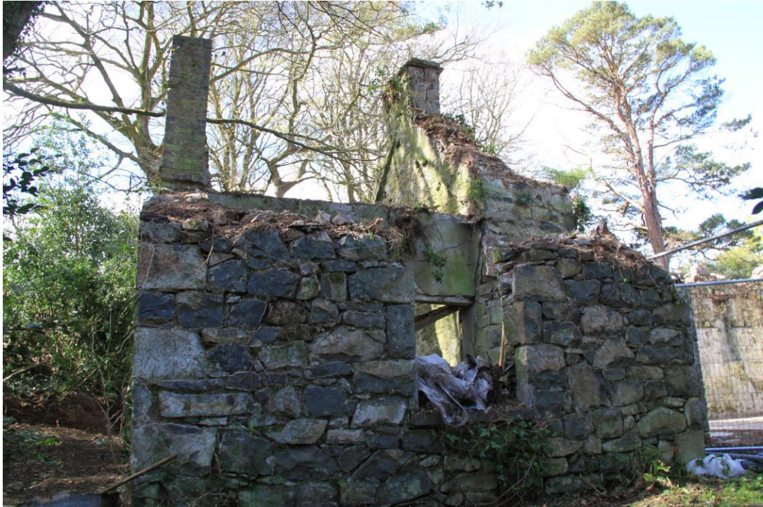
Plate 9 - AD010-BR-009 - North elevation, east end.
