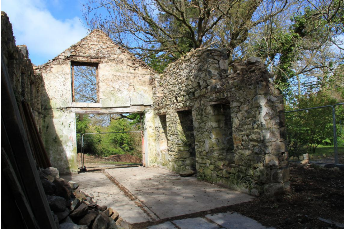
Plate 23 - AD010-BR-023 - Internal view of Former Coach House towards the west.
