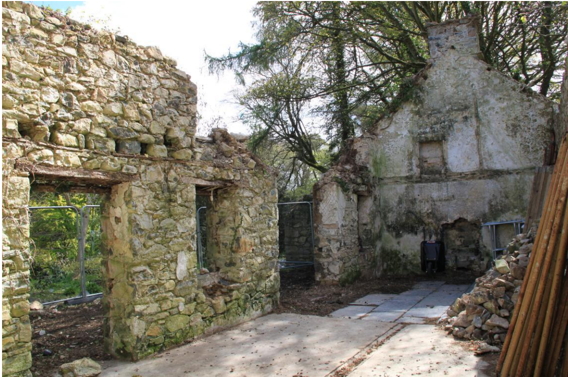
Plate 20 - AD010-BR-020 - Internal view of Former Coach House towards the east.
