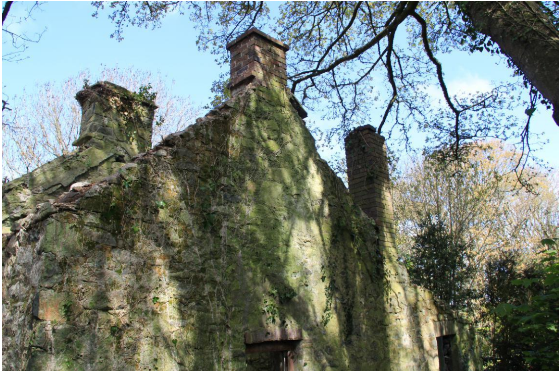
Plate 6 - AD010-BR-006 - East elevation, upper section.
