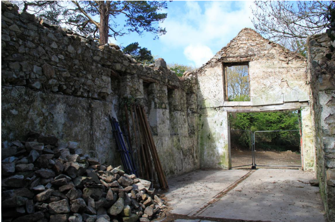
Plate 22 - AD010-BR-022 - Internal view of Former Coach House towards the west.
