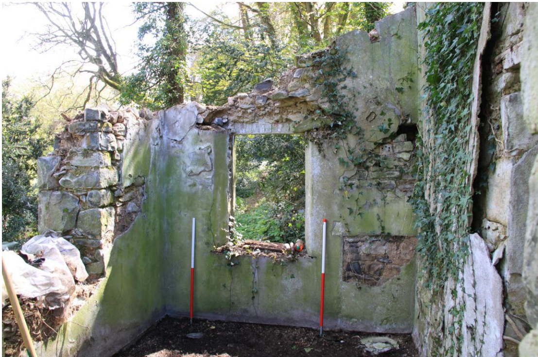
Plate 34 - AD010-BR-034 - Internal view of Extension B towards the east.
