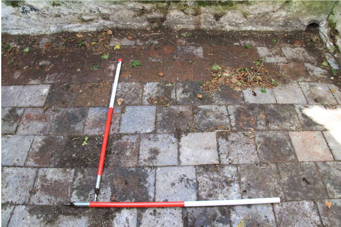
Plate 37 - AD010-BR-037 - Quarry tile floor to Extension A.
