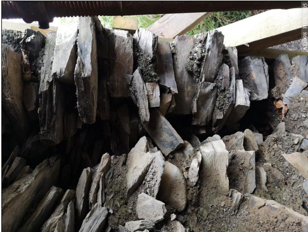
Plate 5 – View east, showing encasing modern retaining wall. Photo rotated 90° anticlockwise.
