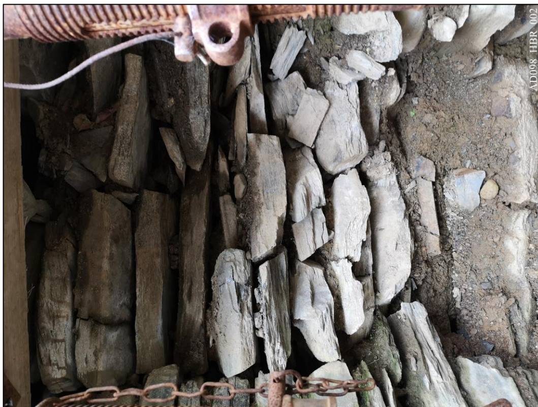
Plate 2 – View north, showing coursed rubble fill of wall core, with earth-clay bedding mortar. Photo rotated 90° anticlockwise.
