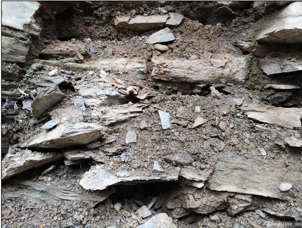
Plate 3 – View north, showing earth-clay mortar of bonding matrix of curtain wall.
