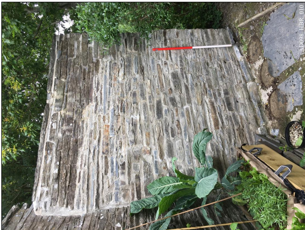
Plate 10 – View north, showing completed rebuild or retaining wall. Photo rotated 90° anticlockwise. Photo courtesy of Joseph Cliff, Cadw.
