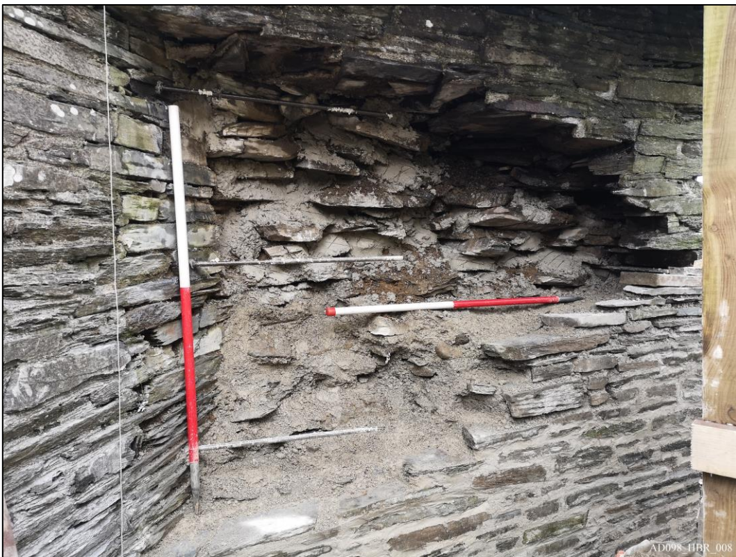
Plate 8 – View north, showing full width of rebuild, including stainless steel ties.
