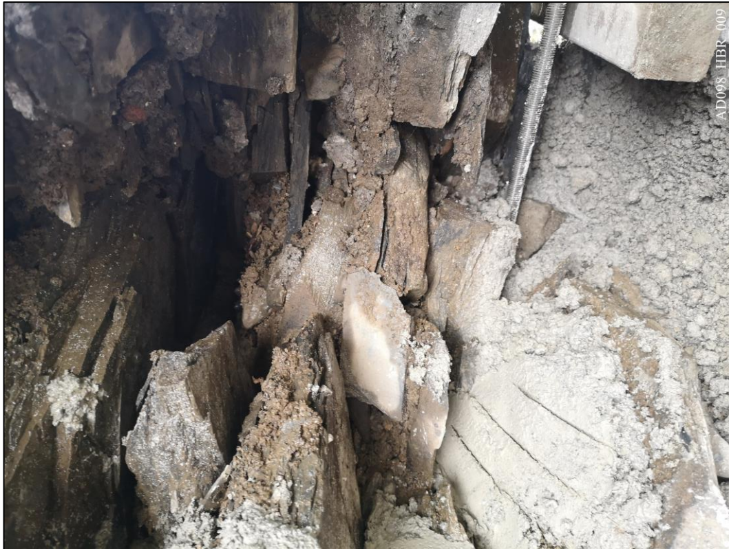
Plate 9 – View north-west, showing insertion of stainless-steel tie and introduction of lime mortar. Photo rotated 90° anticlockwise.
