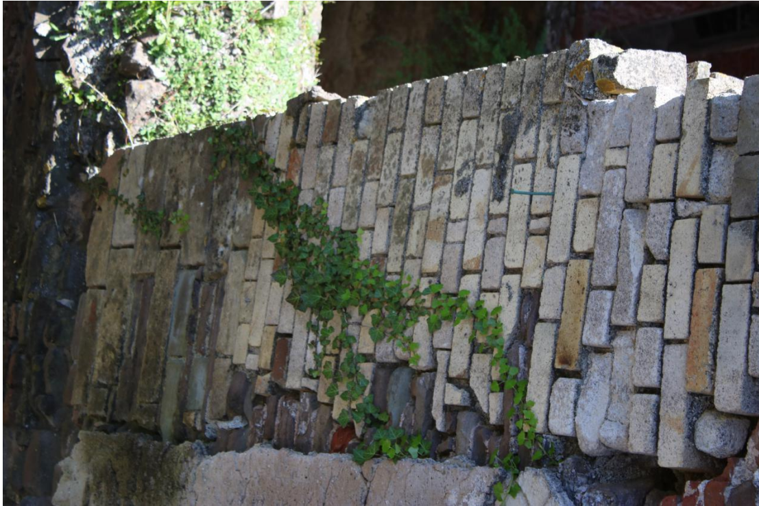
Plate 51 - AD042_WB_051 - East elevation, showing latter flue (5) addition in white brick.
