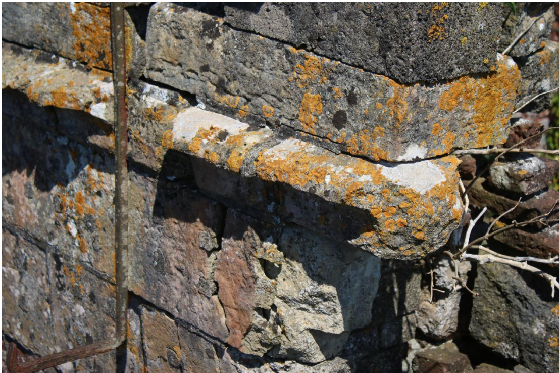
Plate 6 - AD042_WB_006 - West chimney elevation, showing string course.
