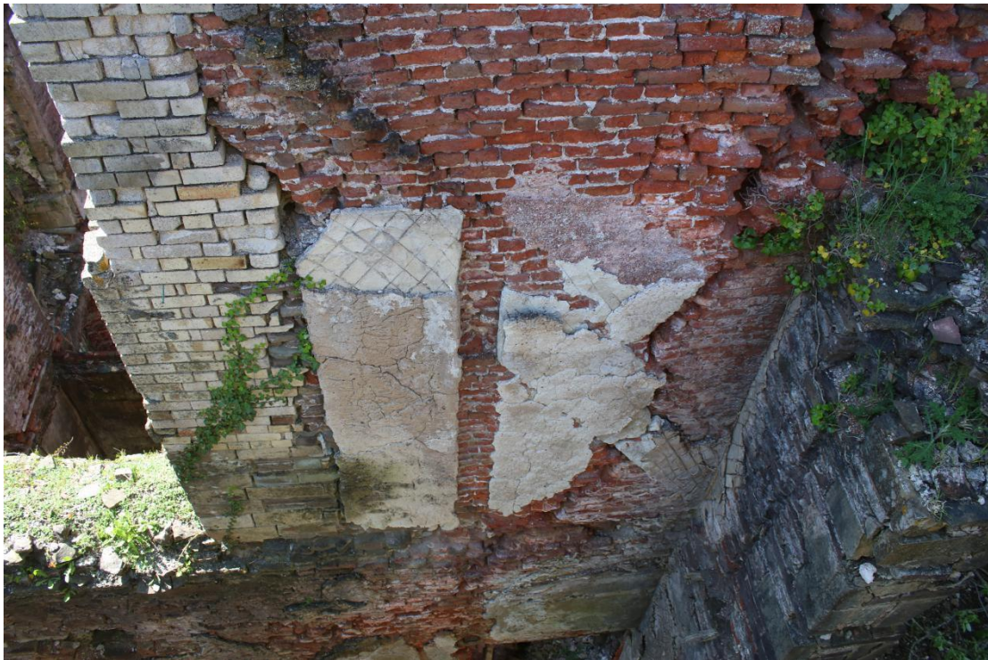
Plate 46 - AD042_WB_046 - East elevation, showing 1626 roofline and surviving lime plasterwork.
