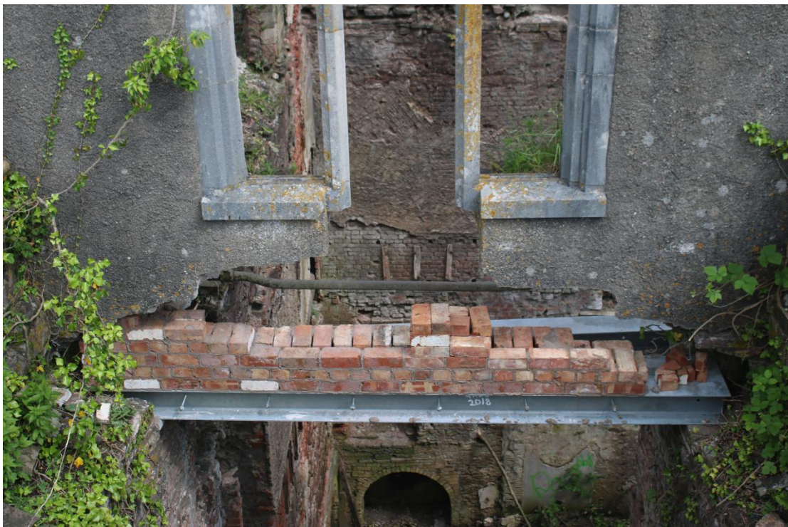
Plate 155 - AD042_WB_155 - South window, showing start of supporting brickwork.
