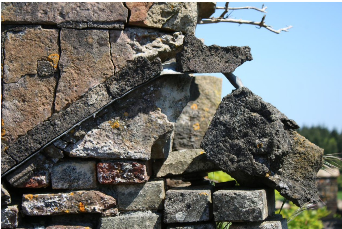
Plate 10 - AD042_WB_010 - West elevation, showing line of lead flashing.
