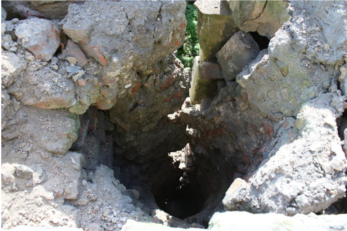
Plate 69 - AD042_WB_069 - Chimney after removal of row 4, showing flue 2.
