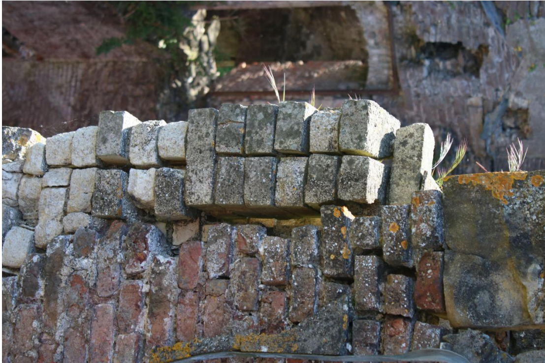
Plate 53 - AD042_WB_053 - East elevation, showing later flue brickwork in white.
