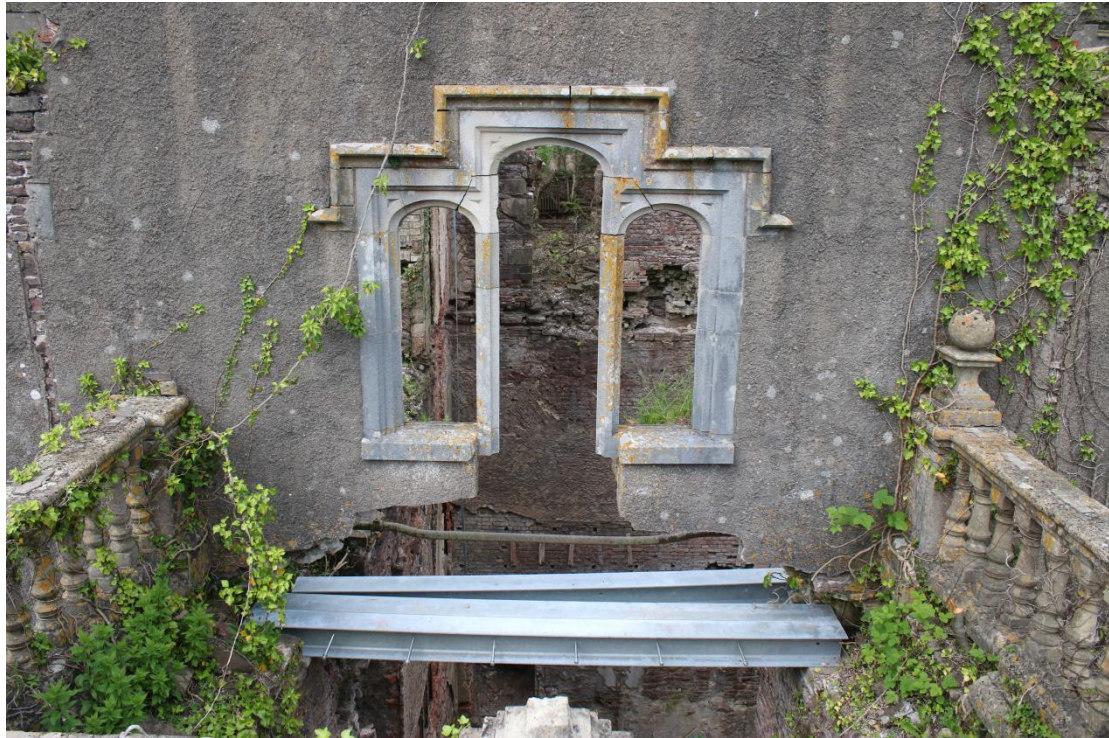
Plate 121 - AD042_WB_121 - South window exterior, showing rolled steel joists (RSJ).
