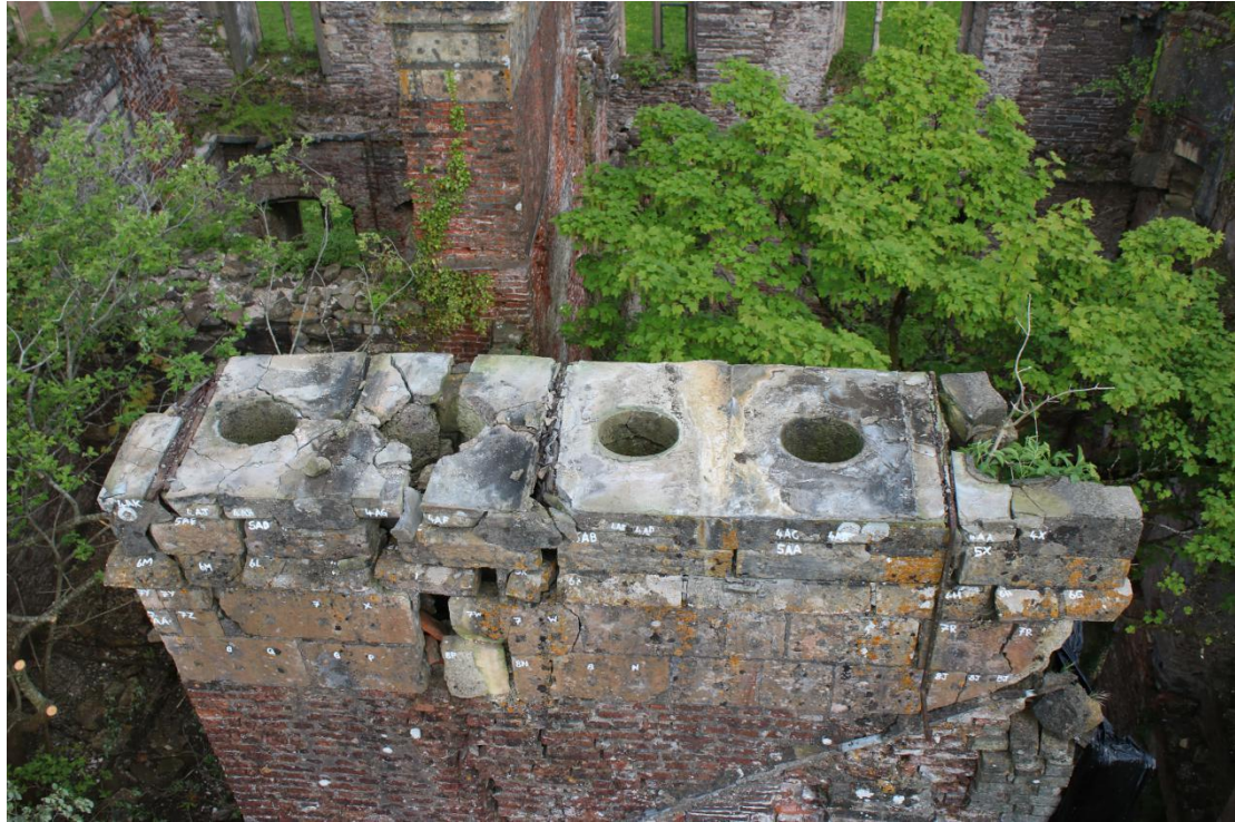
Plate 67 - AD042_WB_067 - Chimney after removal of row 3.
