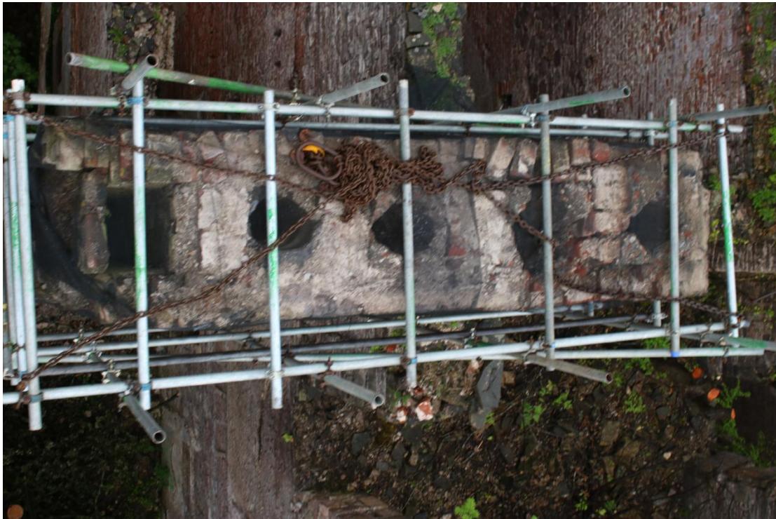
Plate 117 - AD042_WB_117 - Chimney after removal of row 8.
