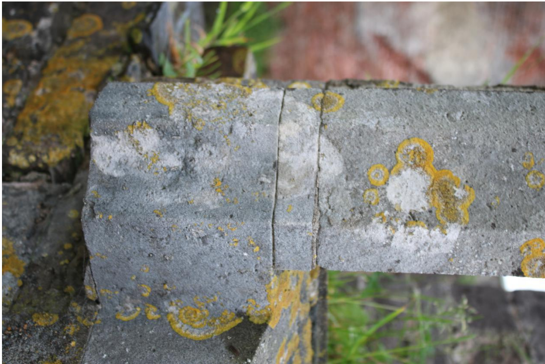
Plate 150 - AD042_WB_150 - South window, showing hollow mould of mullion, east.
