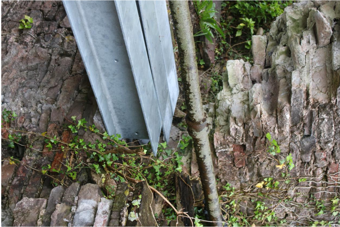
Plate 133 - AD042_WB_133 - South window interior, showing RSJ temporary siting.
