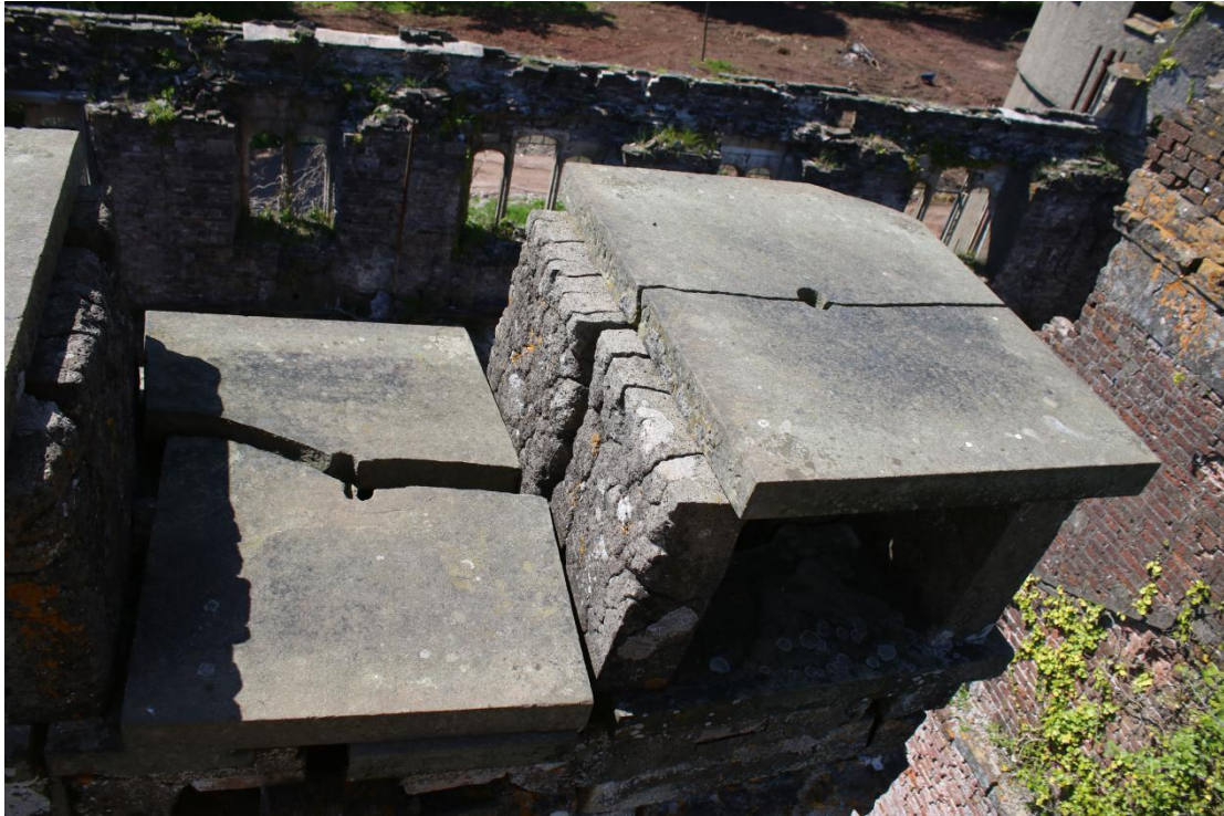
Plate 37 - AD042_WB_037 - East elevation, showing cap stones to flues 1 and 2.
