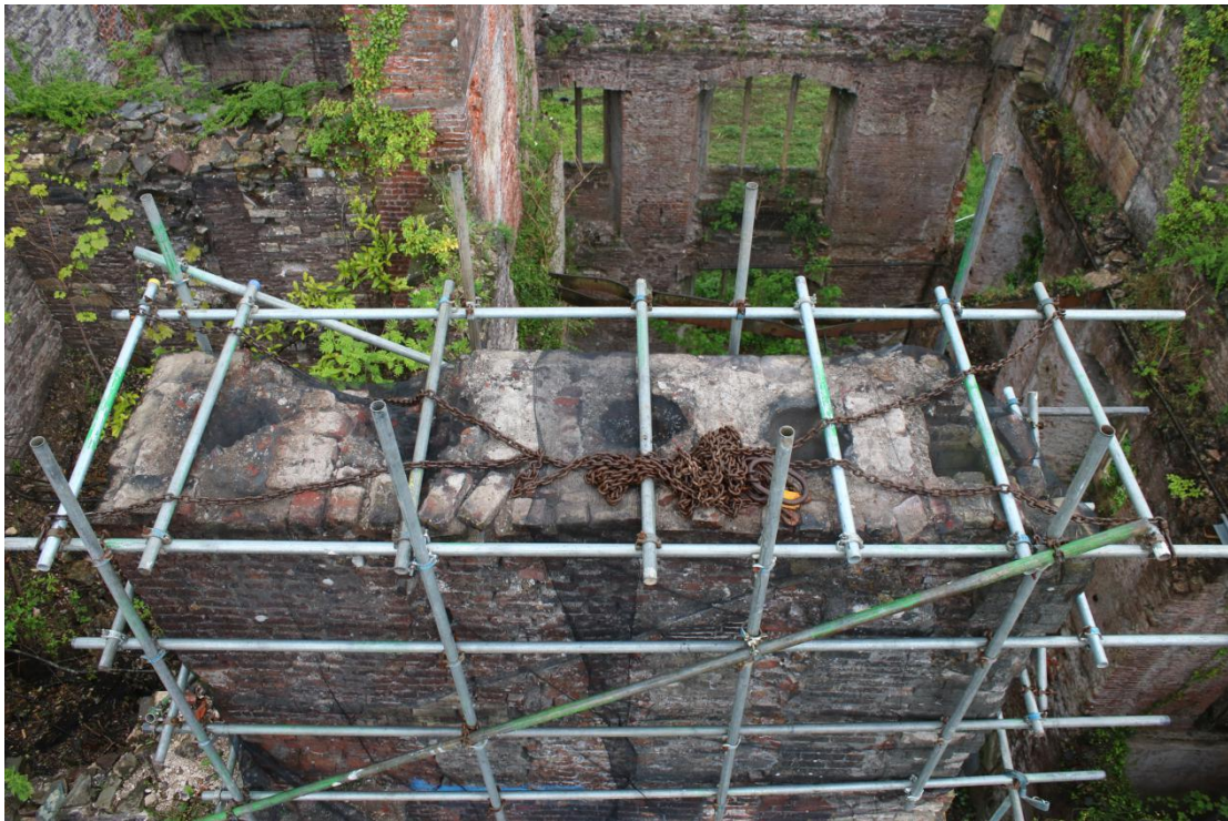
Plate 112 - AD042_WB_112 - Chimney after removal of row 8.
