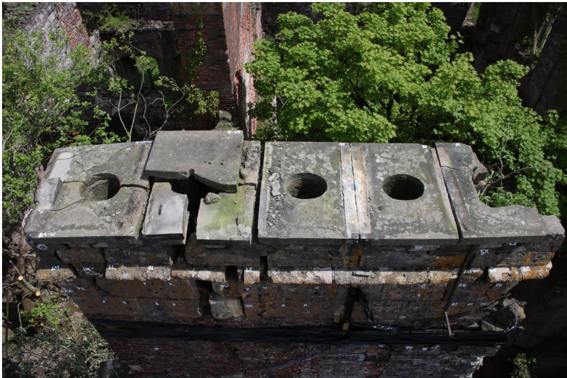
Plate 62 - AD042_WB_062 - Chimney after removal of rows 1 and 2, showing flue stones.
