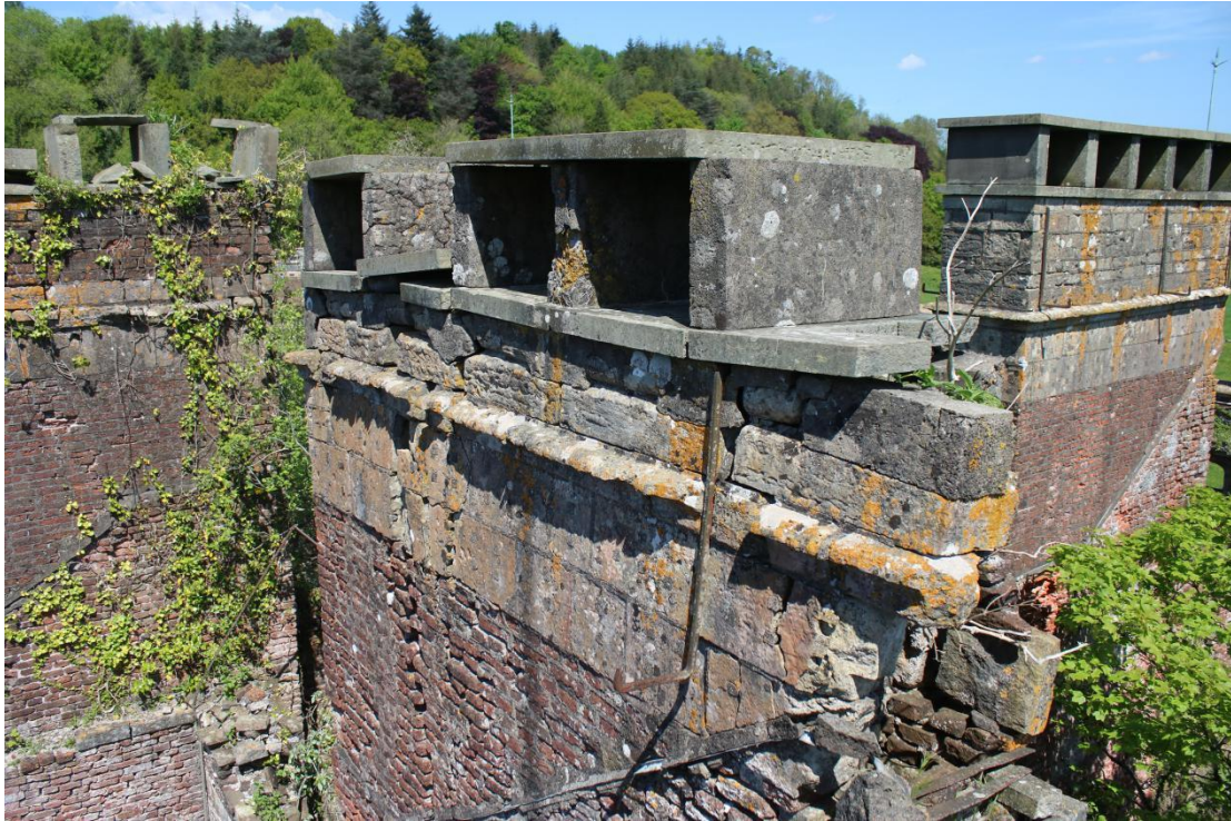
Plate 5 - AD042_WB_005 - West chimney elevation, showing capstones and sandstone coursing.
