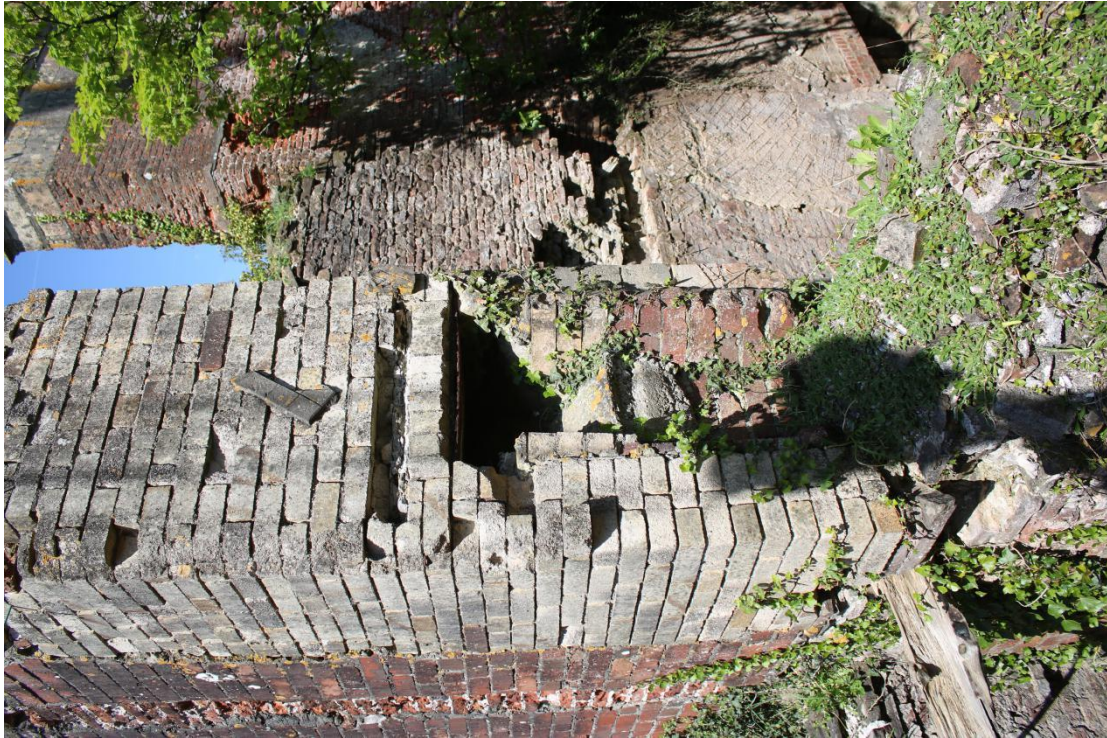
Plate 59 - AD042_WB_059 - South elevation, showing former first floor fireplace.
