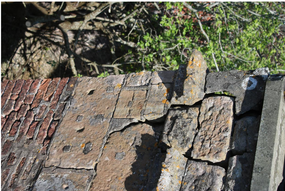
Plate 22 - AD042_WB_022 - West elevation, showing sandstone and concrete fill to north-west corner.
