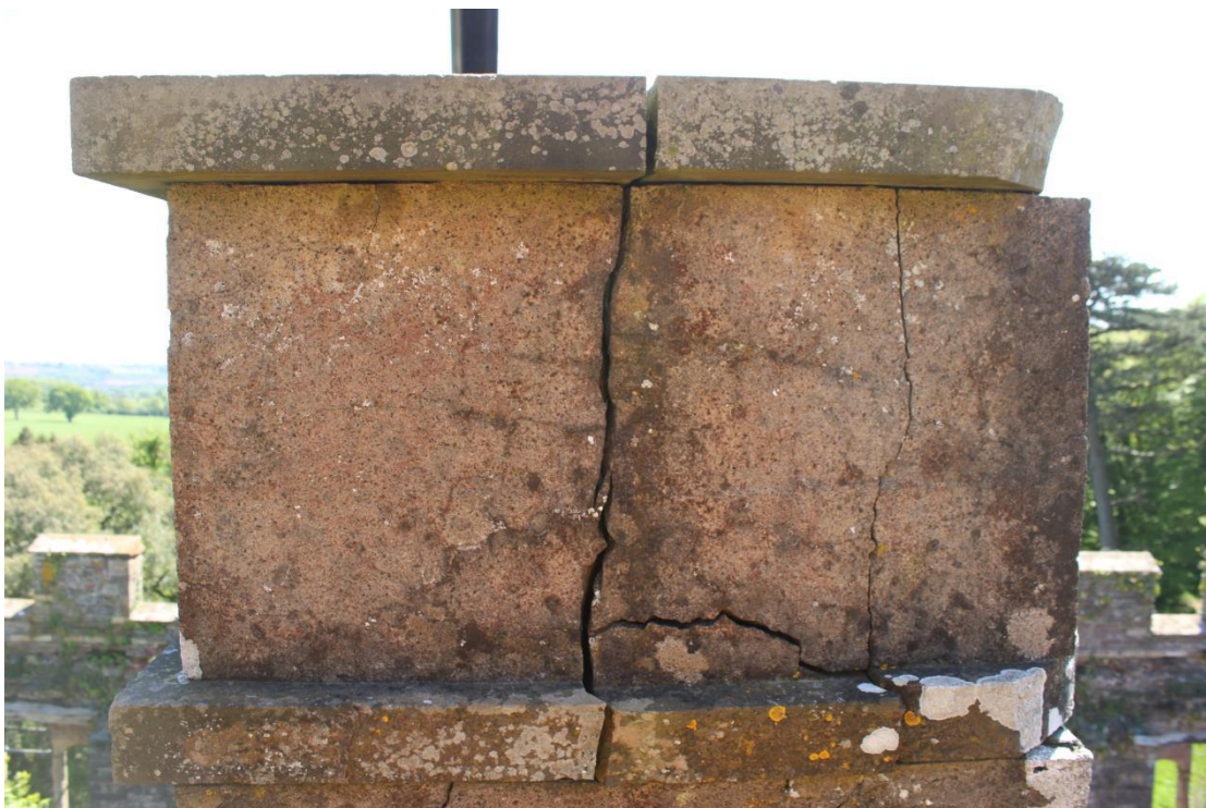
Plate 32 - AD042_WB_032 - North elevation, showing capstone, cast concrete uprights and flue stone.
