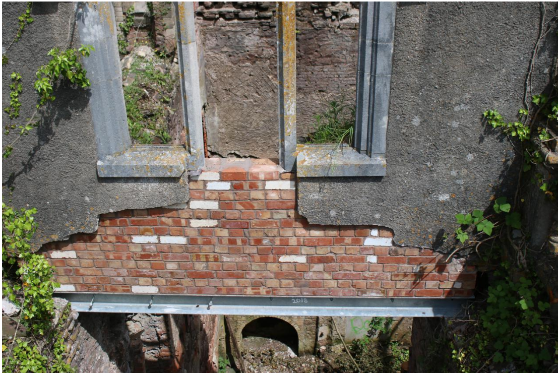
Plate 156 - AD042_WB_156 - South window, showing supporting brickwork complete to exterior.
