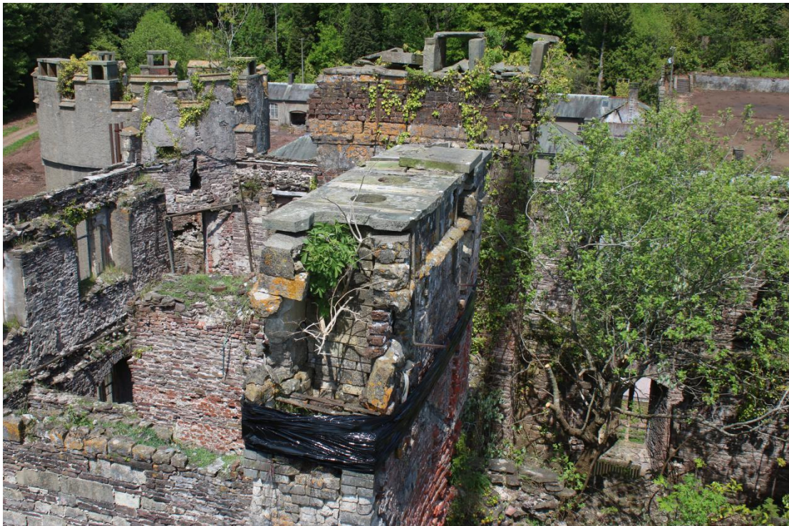
Plate 60 - AD042_WB_060 - Chimney after removal of rows 1 and 2, showing flue stones.
