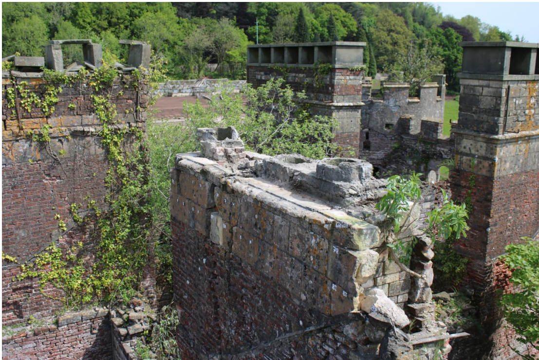
Plate 74 - AD042_WB_074 - Chimney after removal of row 5.
