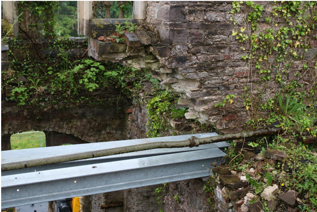
Plate 127 - AD042_WB_127 - South window interior, showing RSJ pad.
