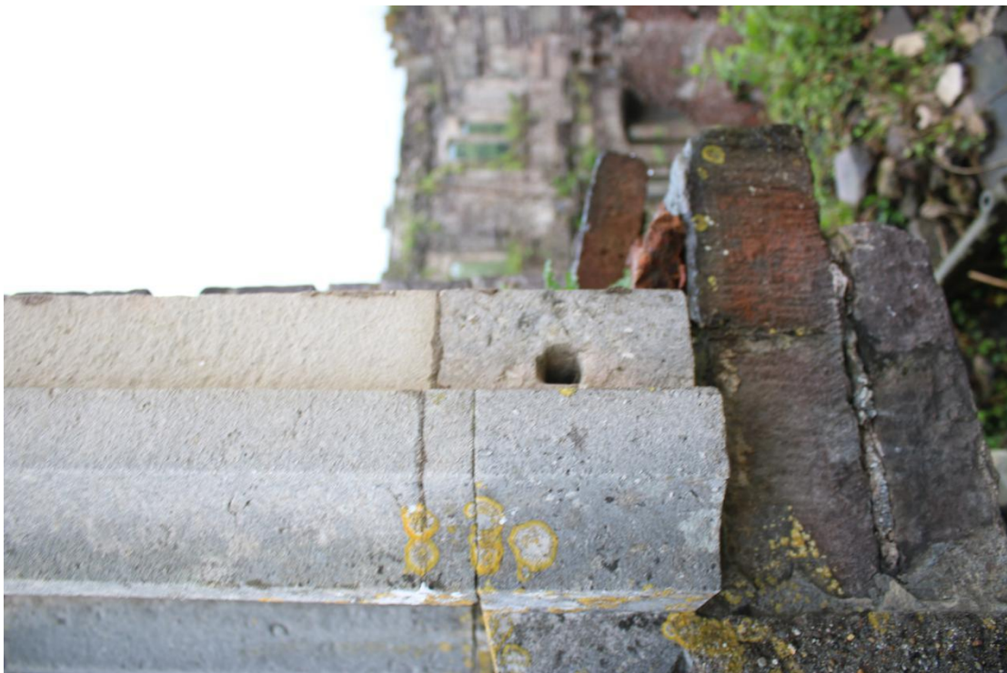
Plate 149 - AD042_WB_149 - South window, showing glazing bar socket, west.
