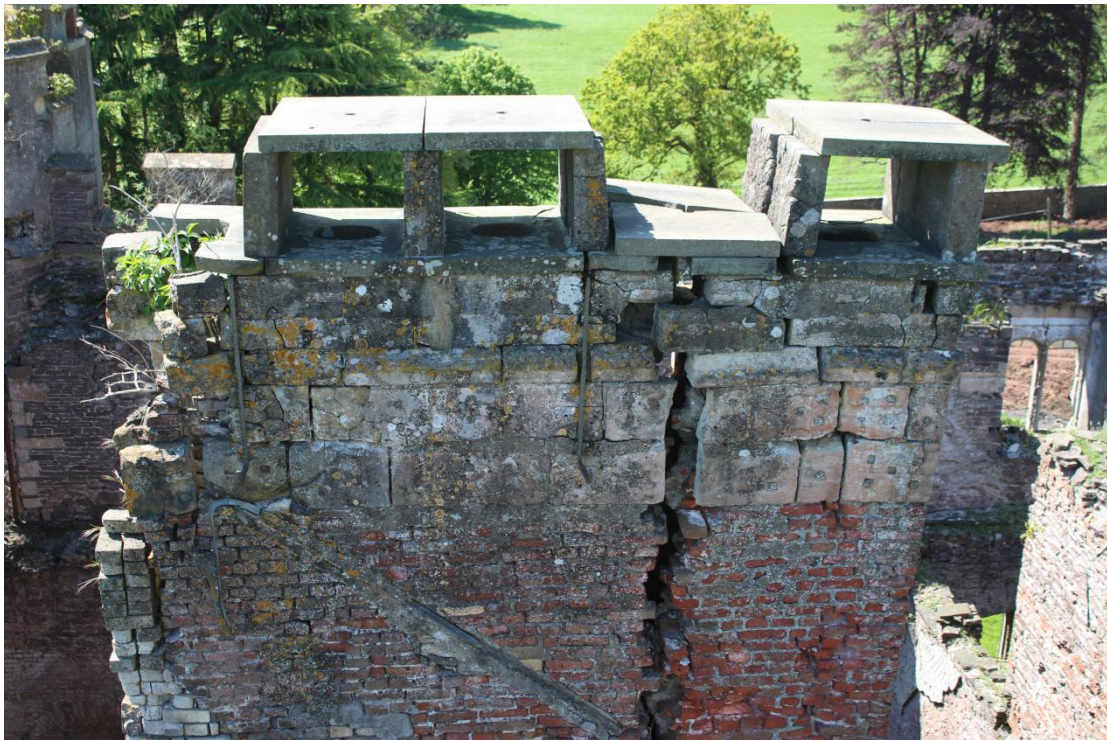
Plate 40 - AD042_WB_040 - East elevation.
