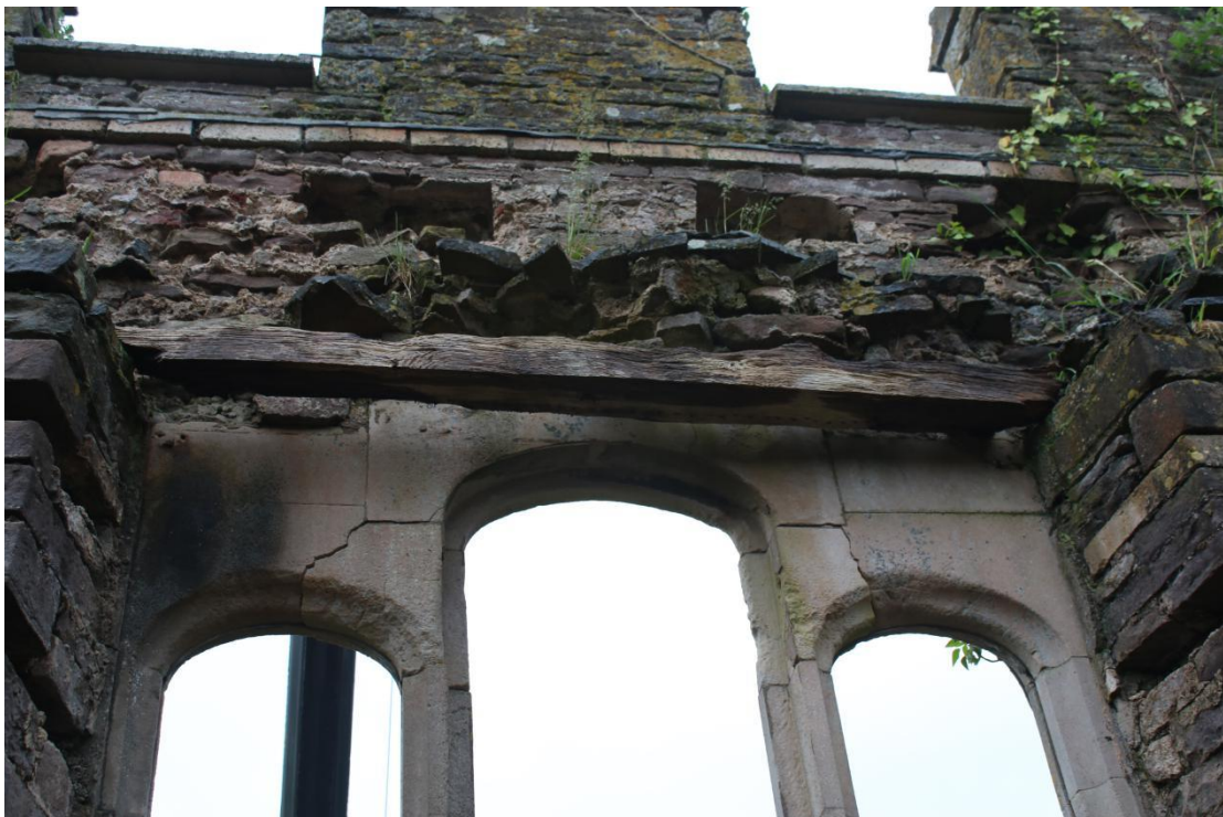
Plate 134 - AD042_WB_134 - South window interior, showing surviving timber lintel.
