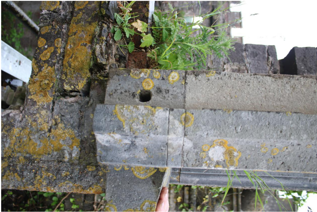
Plate 148 - AD042_WB_148 - South window, showing glazing bar socket, east.
