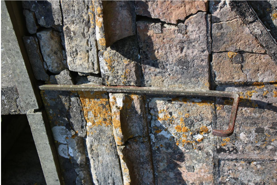
Plate 9 - AD042_WB_009 - West elevation, showing iron hook/strap.
