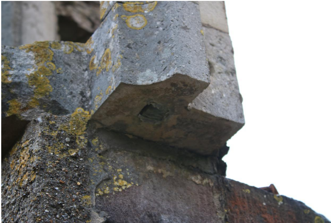
Plate 146 - AD042_WB_146 - South window, showing lead fixing joint, west.
