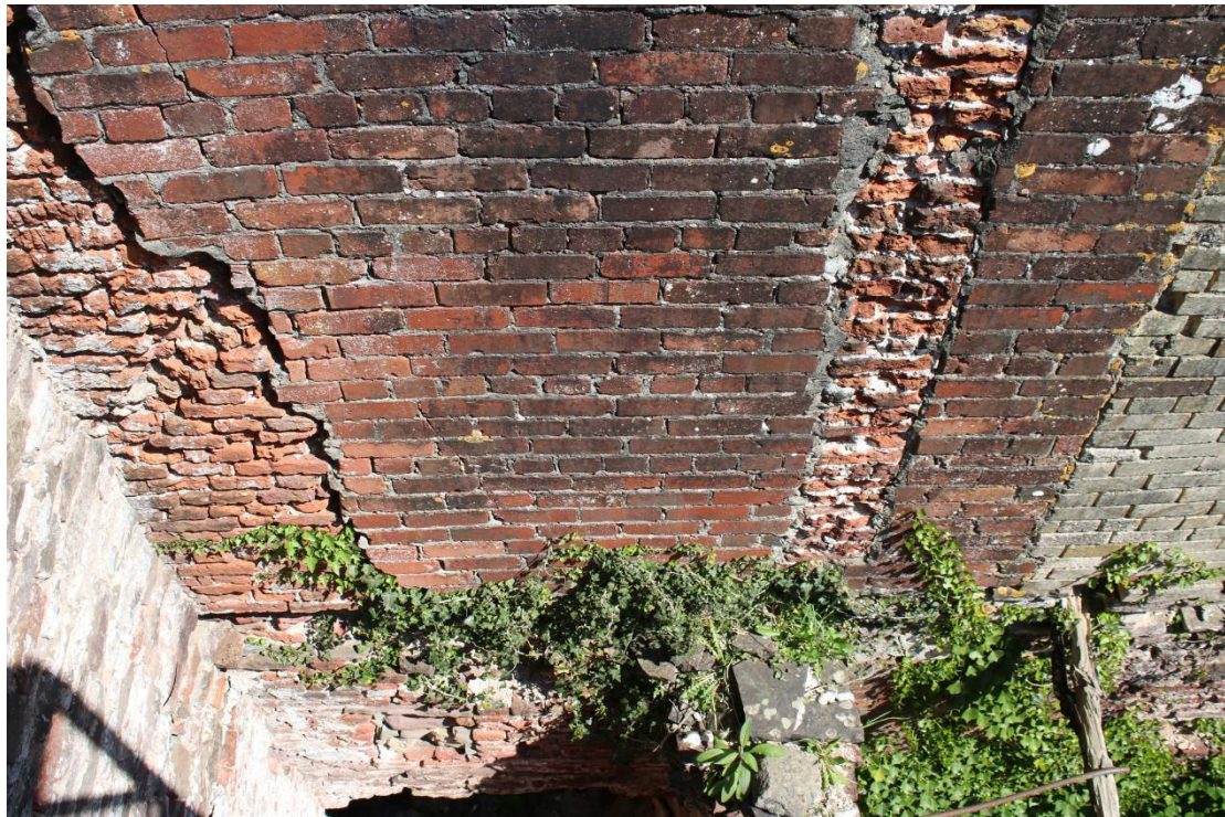
Plate 18 - AD042_WB_018 - West elevation, showing 20 th century red brickwork and wall scar.
