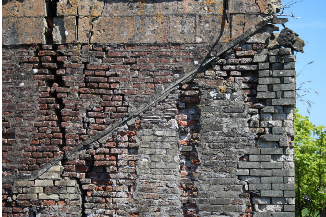
Plate 17 - AD042_WB_017 - West elevation, showing lead flashing to former roofline.
