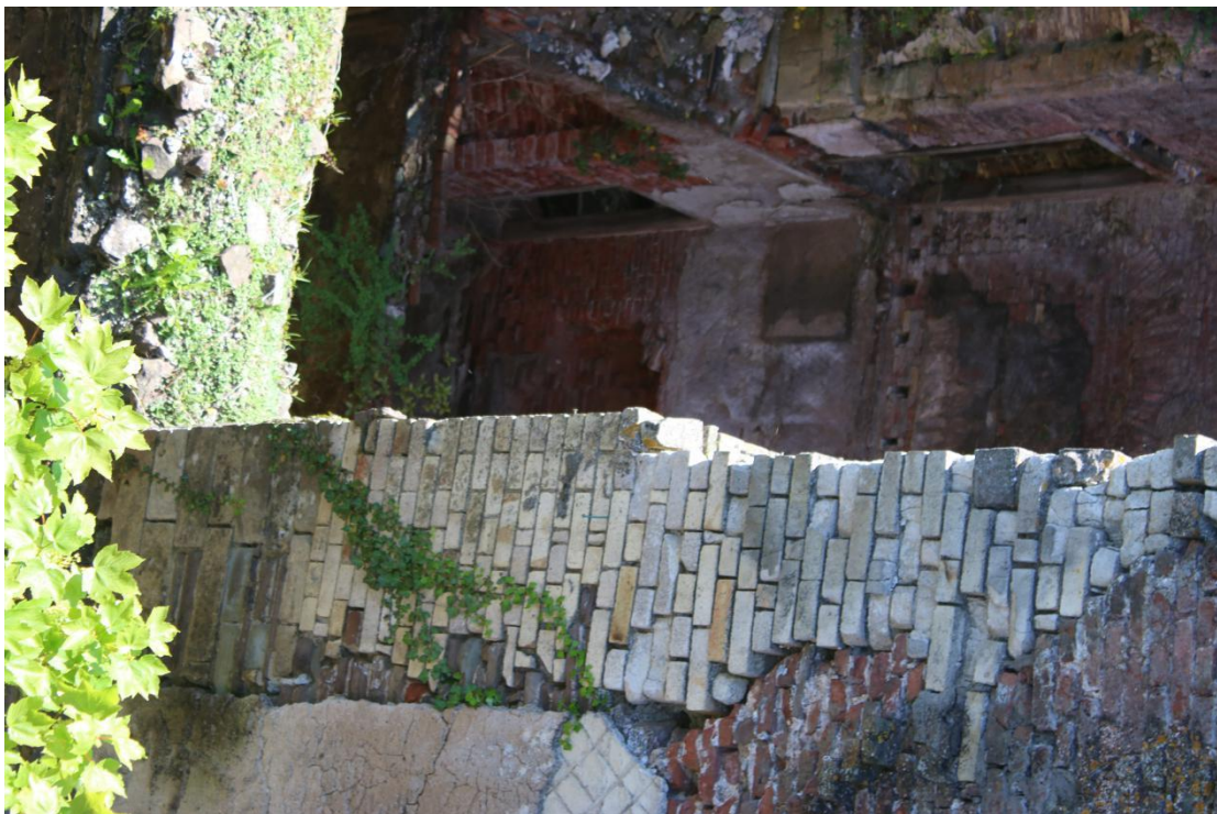
Plate 42 - AD042_WB_042 - East elevation, showing inserted flue (5; white brick).
