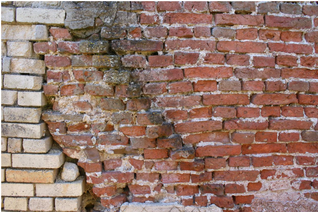
Plate 54 - AD042_WB_054 - East elevation, showing 1626 roofline.
