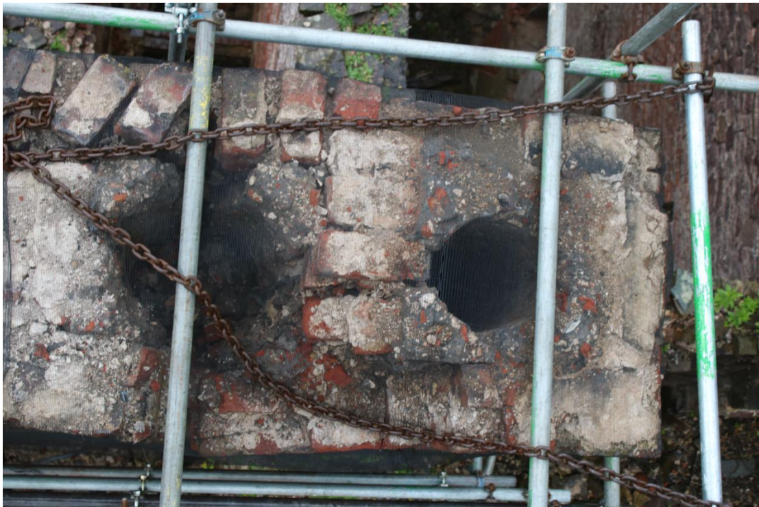
Plate 114 - AD042_WB_114 - Chimney after removal of row 8, showing flues 1 and 2.
