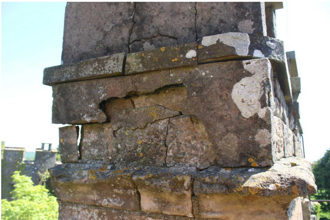
Plate 28 - AD042_WB_028 - North elevation, showing cementitious mortar fill.
