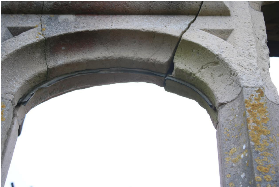
Plate 152 - AD042_WB_152 - South window, showing window head with glazing lead, west.
