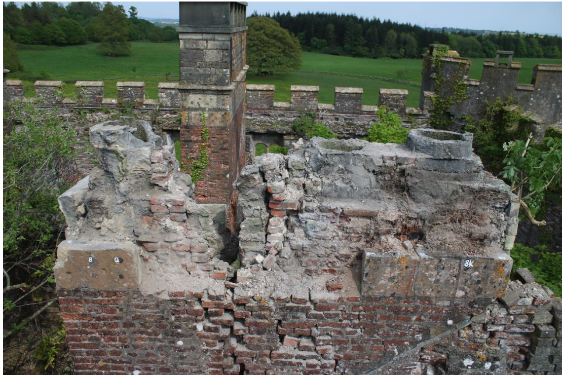
Plate 79 - AD042_WB_079 - Chimney after removal of row 7 and partial row 8.
