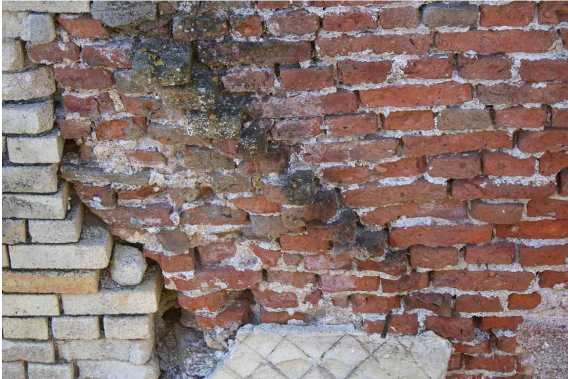
Plate 45 - AD042_WB_045 - East elevation, showing remaining evidence of 1626 roofline.
