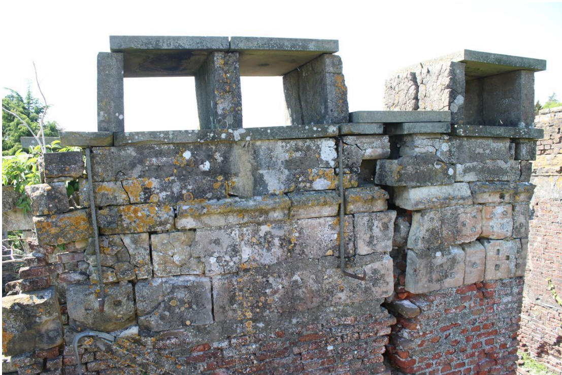
Plate 44 - AD042_WB_044 - East elevation, showing capstones to sandstone ashlar coursing.
