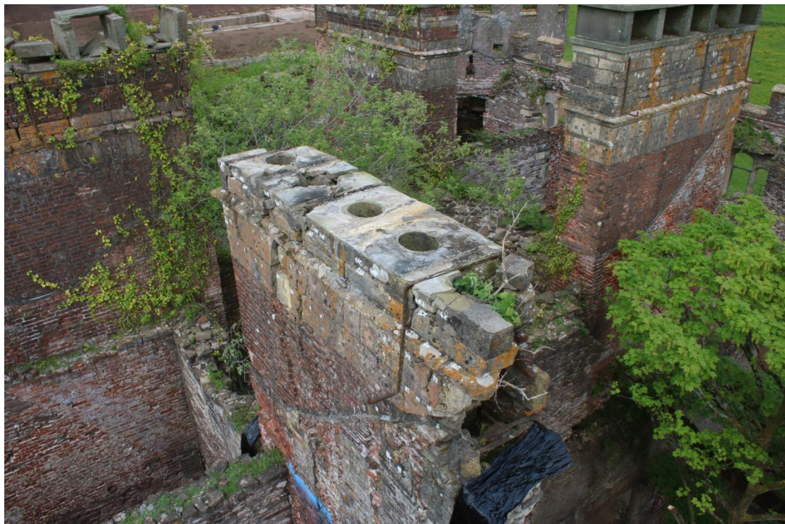
Plate 66 - AD042_WB_066 - Chimney after removal of row 3.
