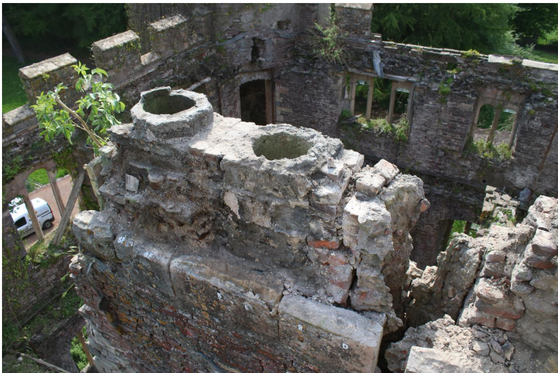
Plate 82 - AD042_WB_082 - Chimney after removal of row 7.
