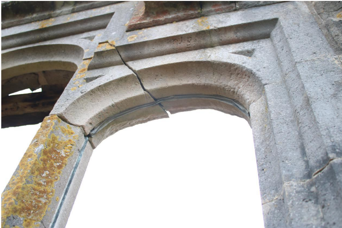
Plate 154 - AD042_WB_154 - South window, showing window head with glazing lead, east.
