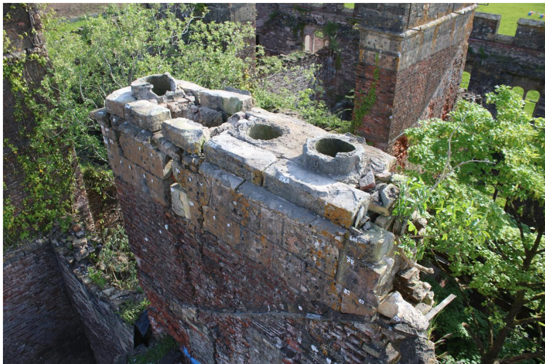
Plate 68 - AD042_WB_068 - Chimney after removal of row 4.
