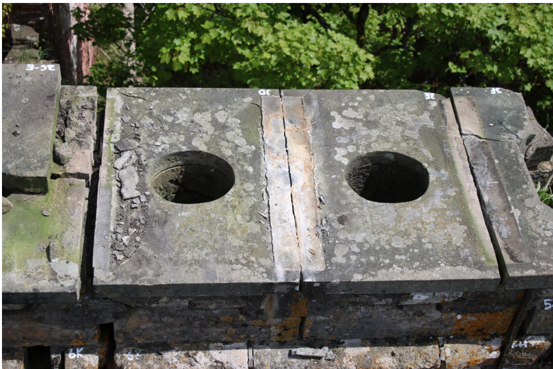
Plate 64 - AD042_WB_064 - Chimney after removal of rows 1 and 2, showing flue stones 3 and 4.
