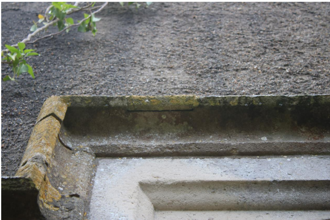
Plate 153 - AD042_WB_153 - South window, showing hood moulding.
