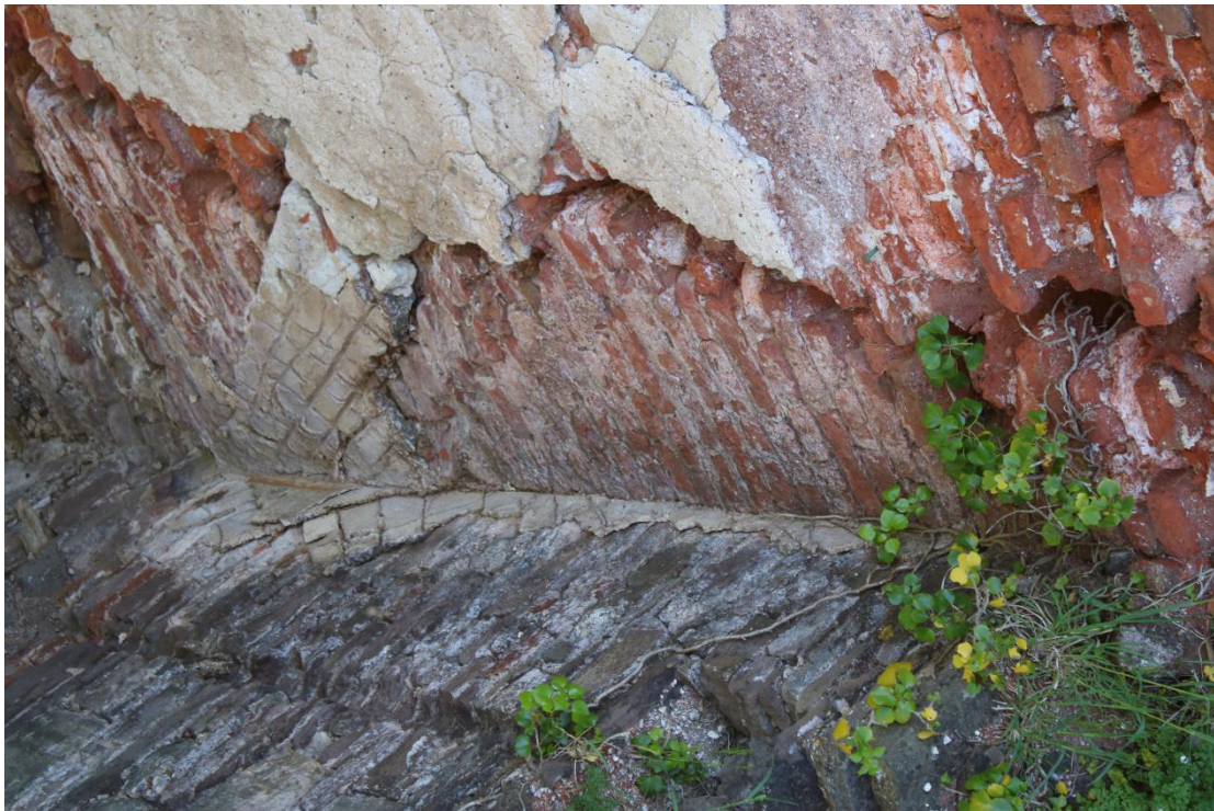
Plate 52 - AD042_WB_052 - East elevation, showing surviving lime plaster.
