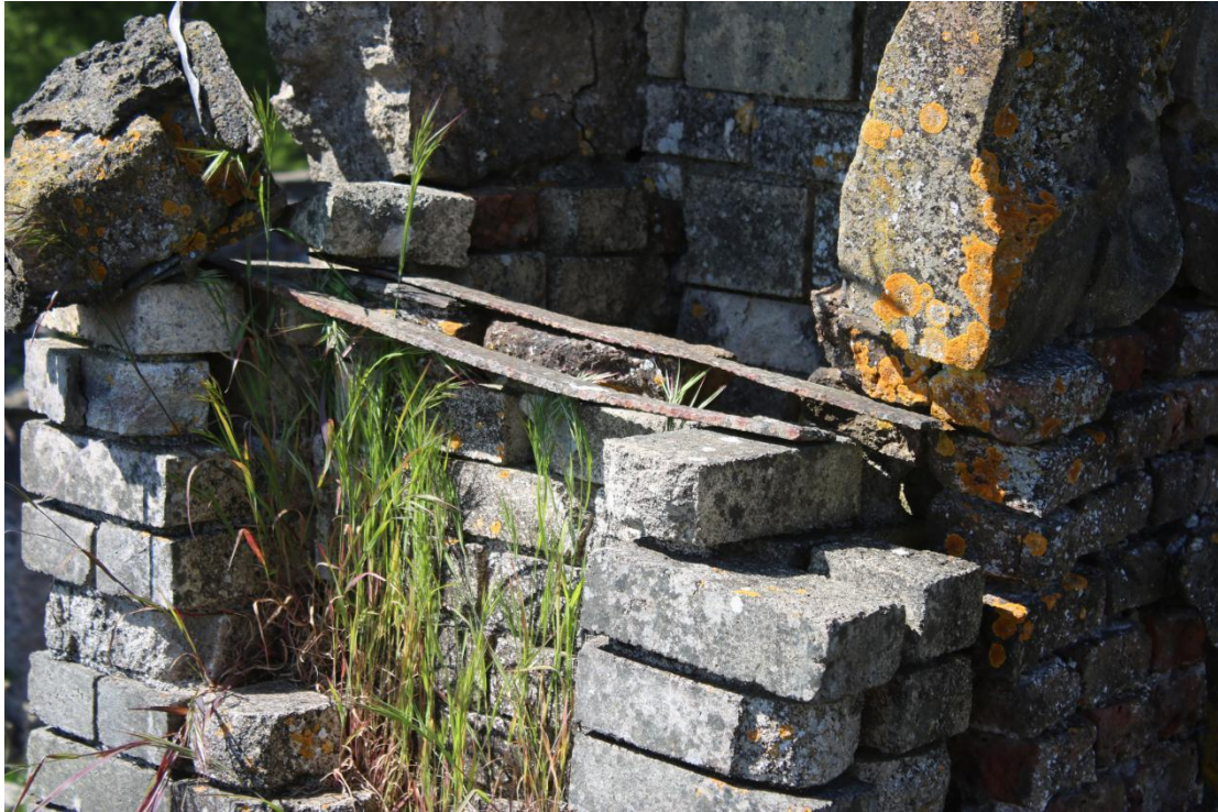
Plate 57 - AD042_WB_057 - South elevation, showing iron support to former 3 rd floor fireplace.
