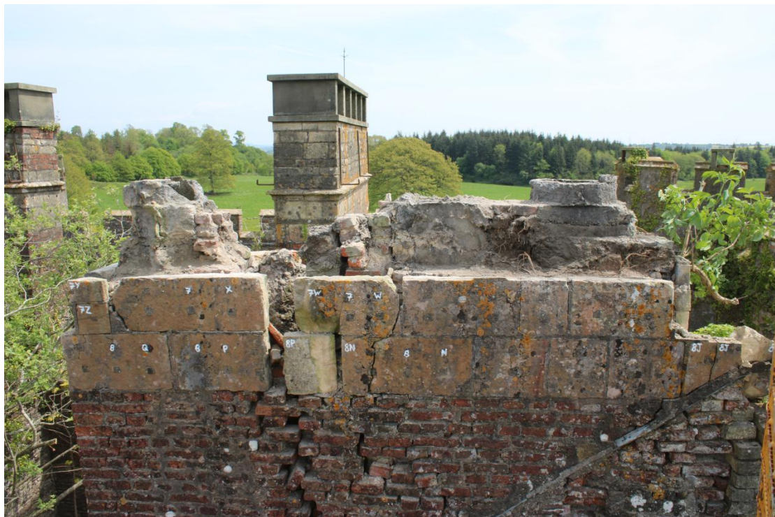
Plate 78 - AD042_WB_078 - Chimney after removal of row 6.
