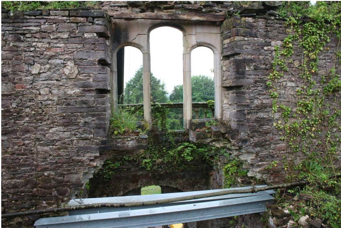
Plate 125 - AD042_WB_125 - South window interior.
