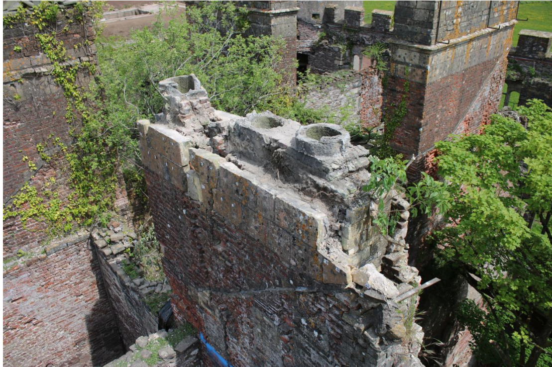
Plate 77 - AD042_WB_077 - Chimney after removal of row 6.
