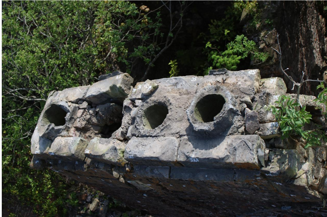
Plate 71 - AD042_WB_071 - Chimney after removal of row 4.
