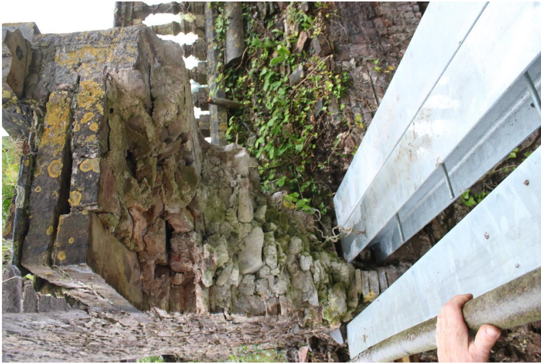
Plate 135 - AD042_WB_135 - South window interior, showing wall masonry section, east.
