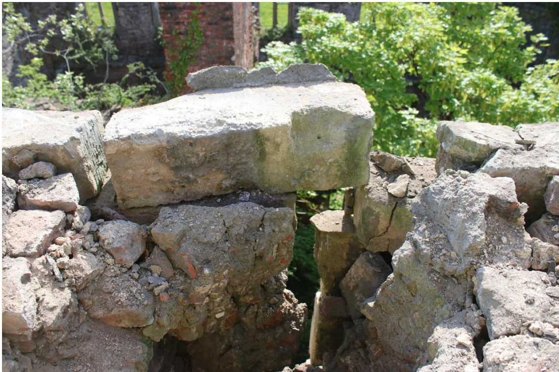
Plate 70 - AD042_WB_070 - Chimney after removal of row 4, showing flue 2.
