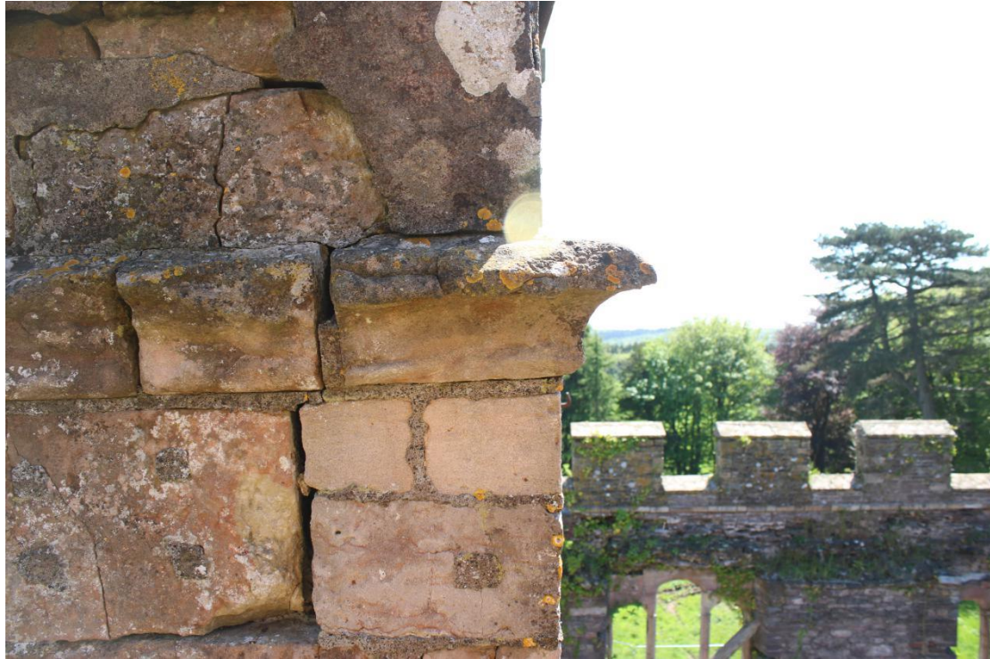
Plate 29 - AD042_WB_029 - North elevation, showing string course profile.
