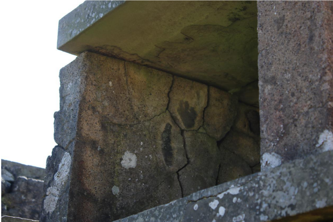
Plate 33 - AD042_WB_033 - East elevation, showing evidence of mud-casting to concrete upright.
