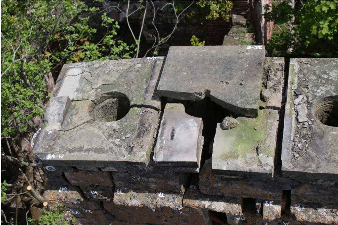
Plate 63 - AD042_WB_063 - Chimney after removal of rows 1 and 2, showing flue stones 1 and 2.
