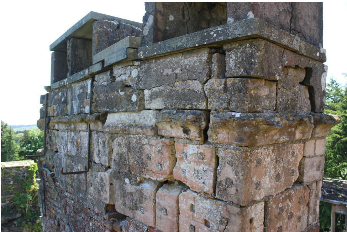
Plate 34 - AD042_WB_034 - 3/4 view of north and east elevations, showing string course.
