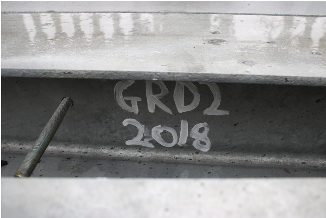
Plate 144 - AD042_WB_144 - South window, showing GRD2 - middle.
