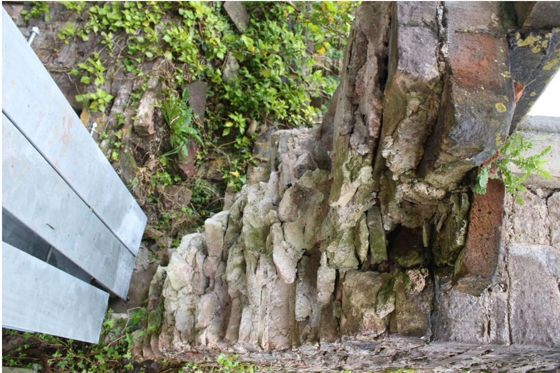
Plate 137 - AD042_WB_137 - South window, showing wall masonry cross section, west.
