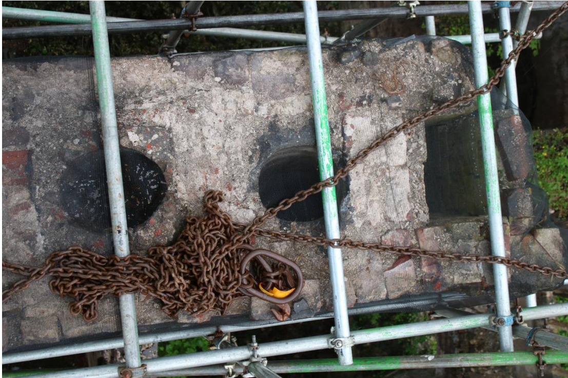
Plate 113 - AD042_WB_113 - Chimney after removal of row 8, showing flues 3 to 5.
