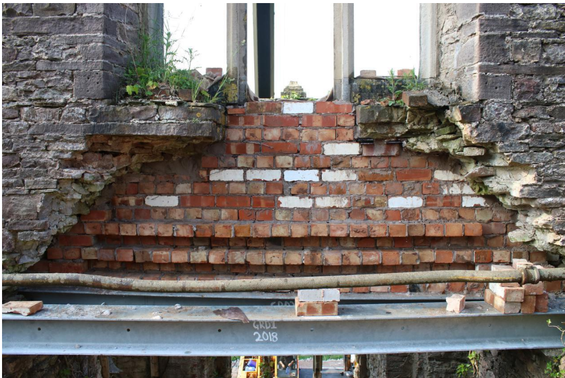
Plate 157 - AD042_WB_157 - South window, showing supporting brickwork exterior skin, inner face.
