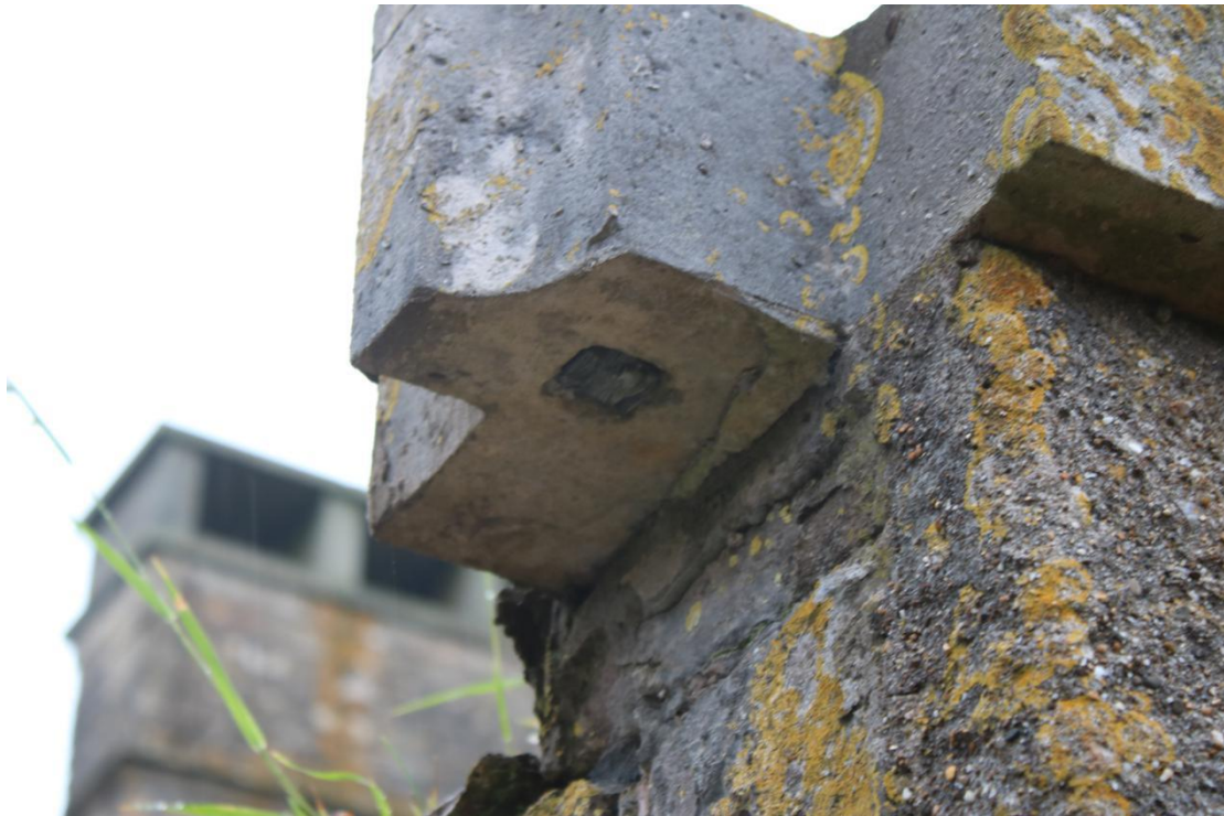
Plate 147 - AD042_WB_147 - South window, showing lead fixing joint, west.
