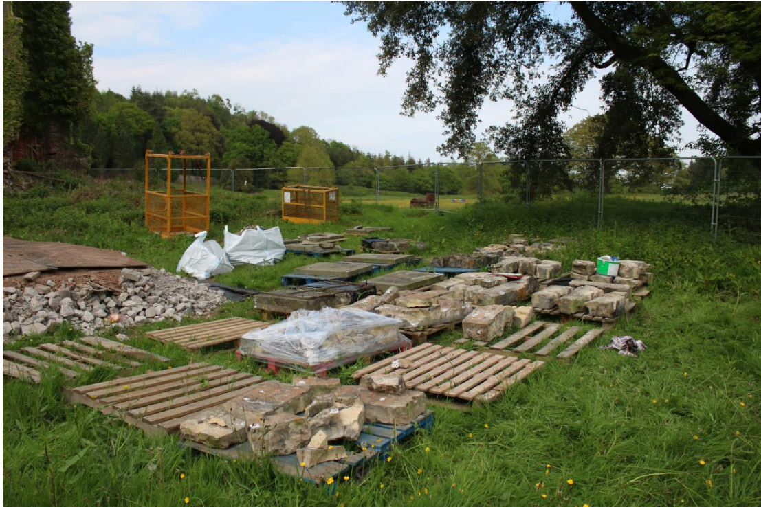
Plate 111 - AD042_WB_111 – General view of palletised masonry.
