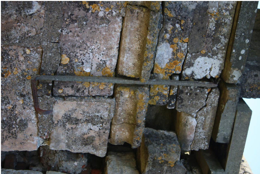
Plate 48 - AD042_WB_048 - East elevation, showing iron hook/strap.
