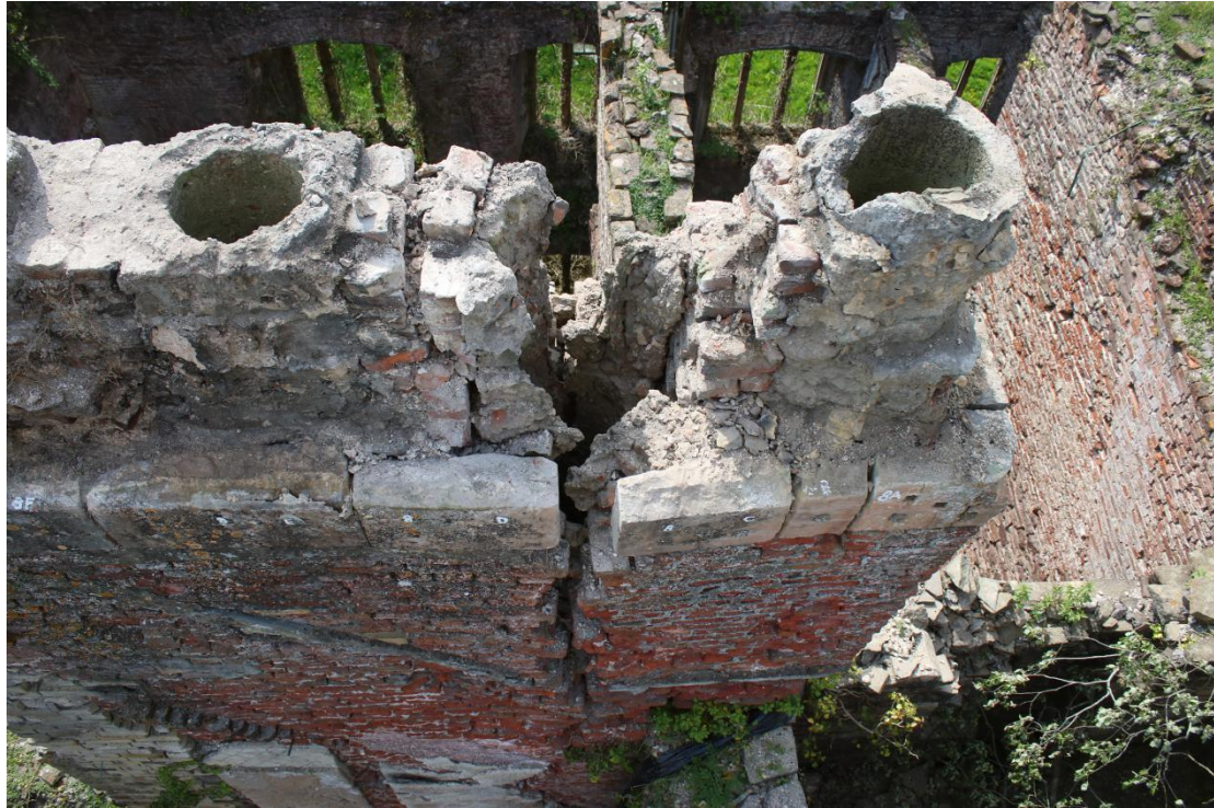
Plate 83 - AD042_WB_083 - Chimney after removal of row 7, showing flues 1, 2 and 3.
