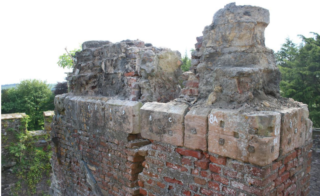
Plate 81 - AD042_WB_081 - Chimney after removal of row 7.
