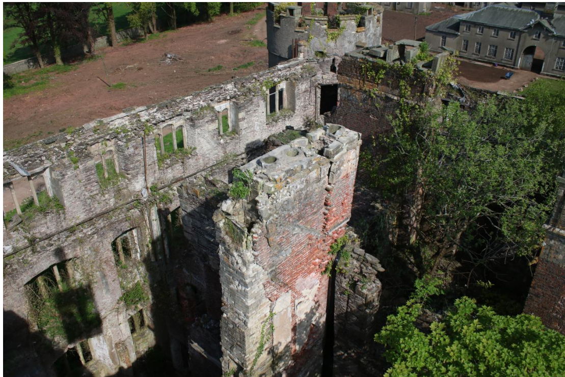
Plate 72 - AD042_WB_072 - Chimney after removal of row 4.
