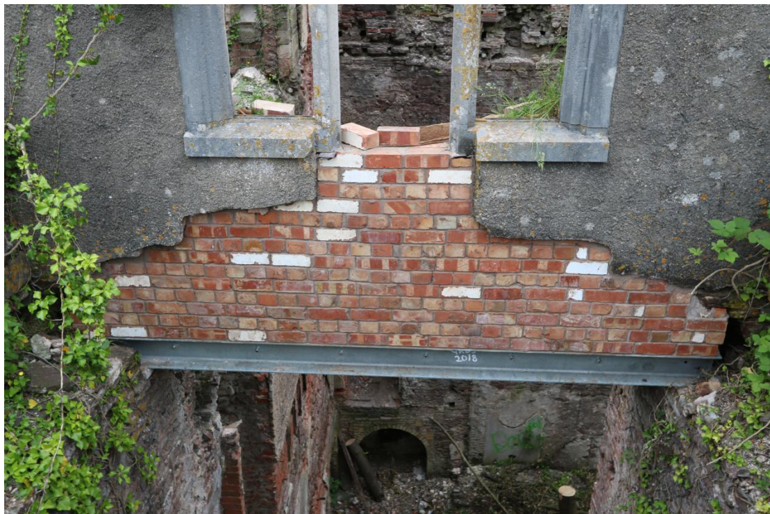
Plate 159 - AD042_WB_159 - South window, showing supporting brickwork complete to exterior.
