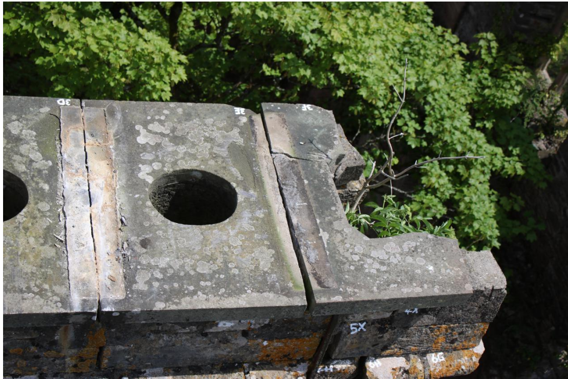
Plate 65 - AD042_WB_065 - Chimney after removal of rows 1 and 2, showing flue stones 4 and 5.
