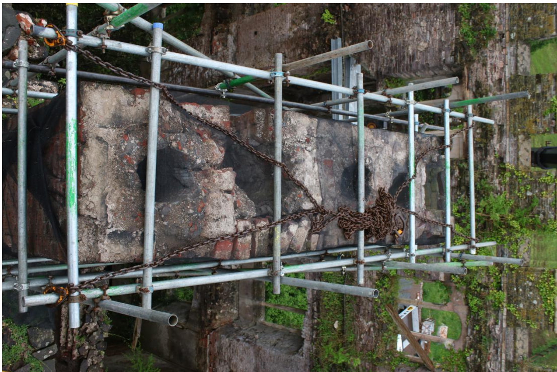
Plate 116 - AD042_WB_116 - Chimney after removal of row 8.
