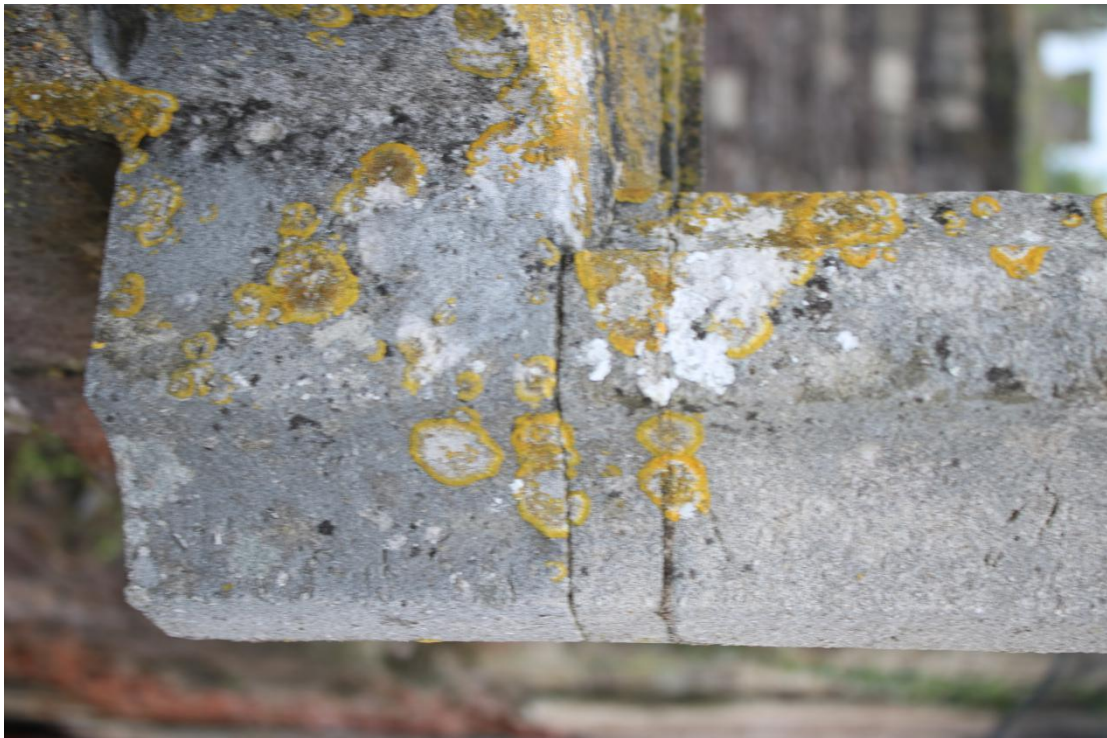
Plate 151 - AD042_WB_151 - South window, showing showing hollow mould of mullion, west.
