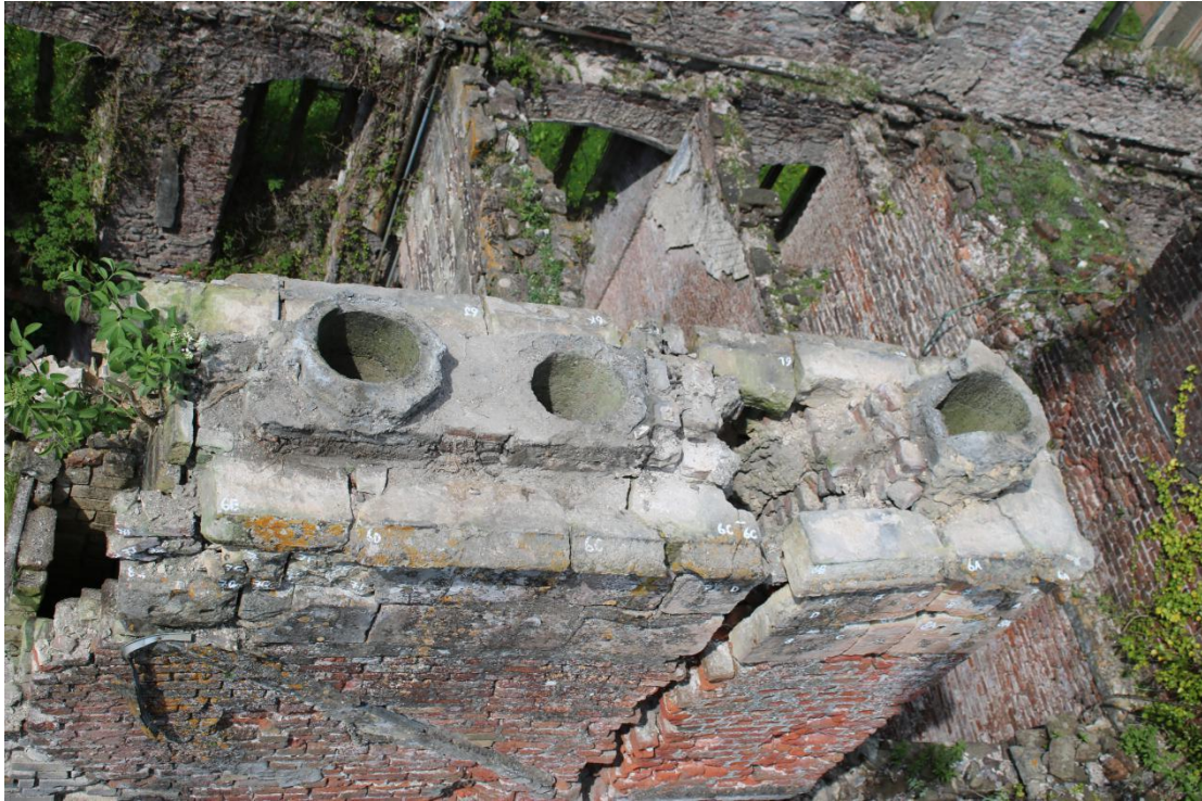
Plate 75 - AD042_WB_075 - Chimney after removal of row 5.
