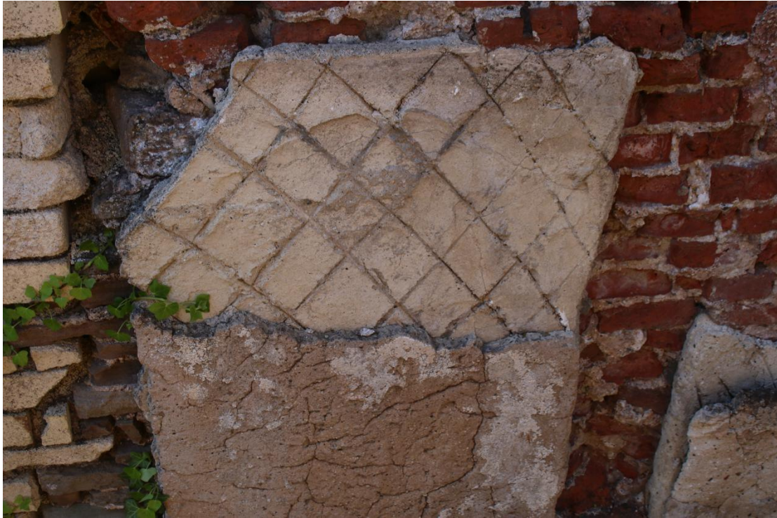
Plate 55 - AD042_WB_055 - East elevation, showing surviving plasterwork scratch and float coat.
