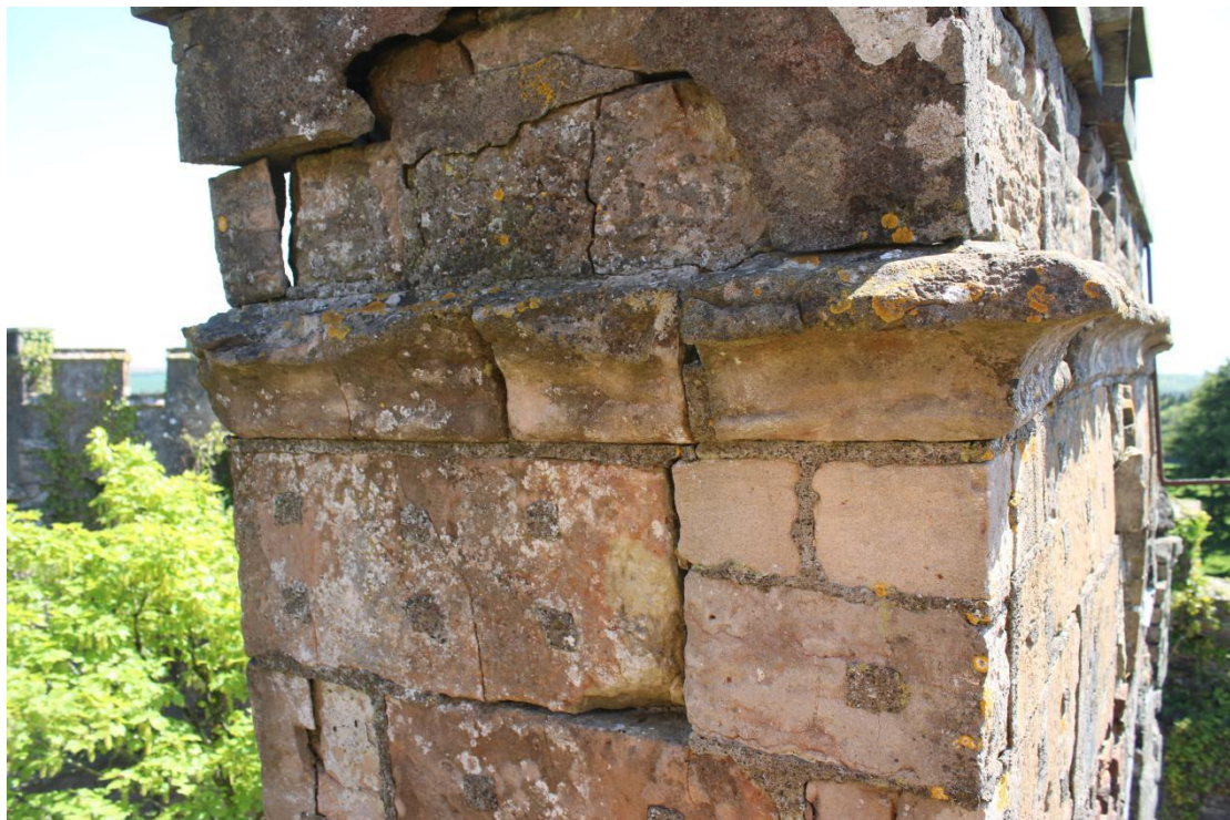
Plate 30 - AD042_WB_030 - North elevation, showing string course.
