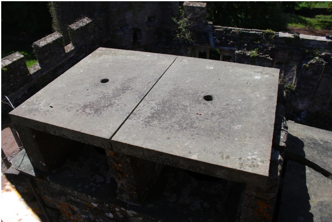
Plate 38 - AD042_WB_038 - East elevation, showing cap stones to flues 3 and 4.
