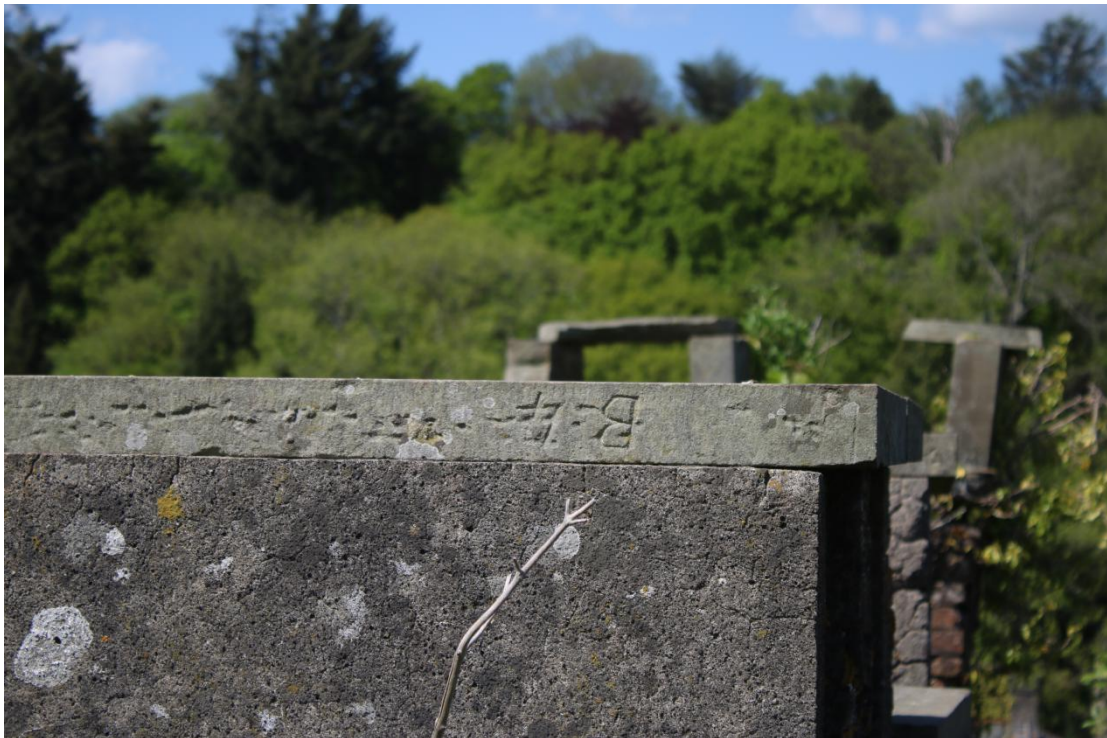
Plate 58 - AD042_WB_058 - South elevation, showing numbering to limestone flue cap.
