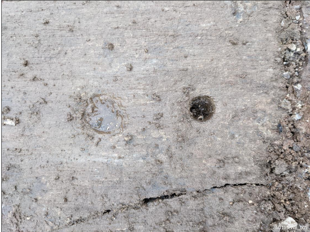
Plate 35 – View showing bolt holes in flagstones of porch.
