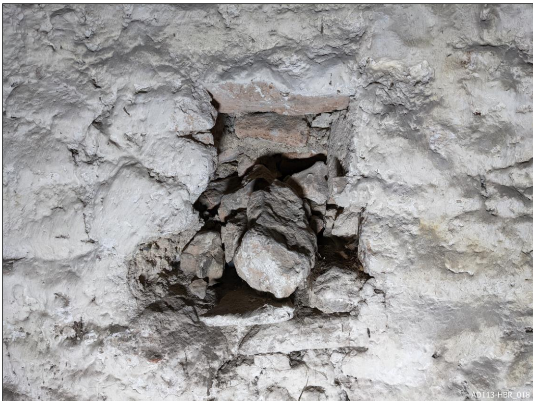
Plate 18 – View west, showing socket in masonry.
