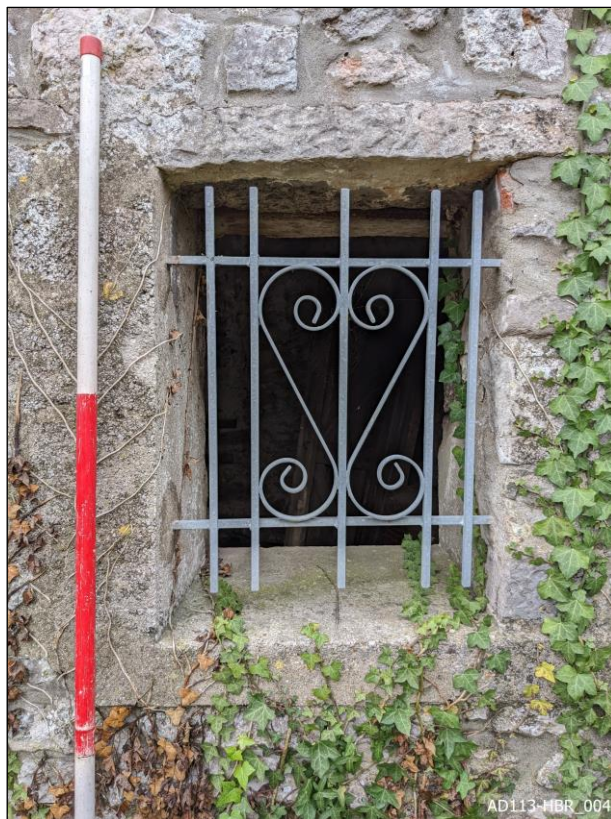
Plate 4 – View west, showing window to east elevation.
