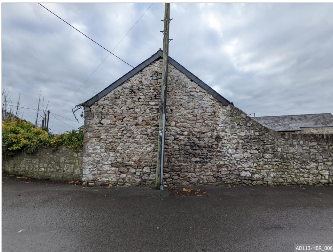
Plate 6 – View south, showing north elevation and flanking yard walls.
