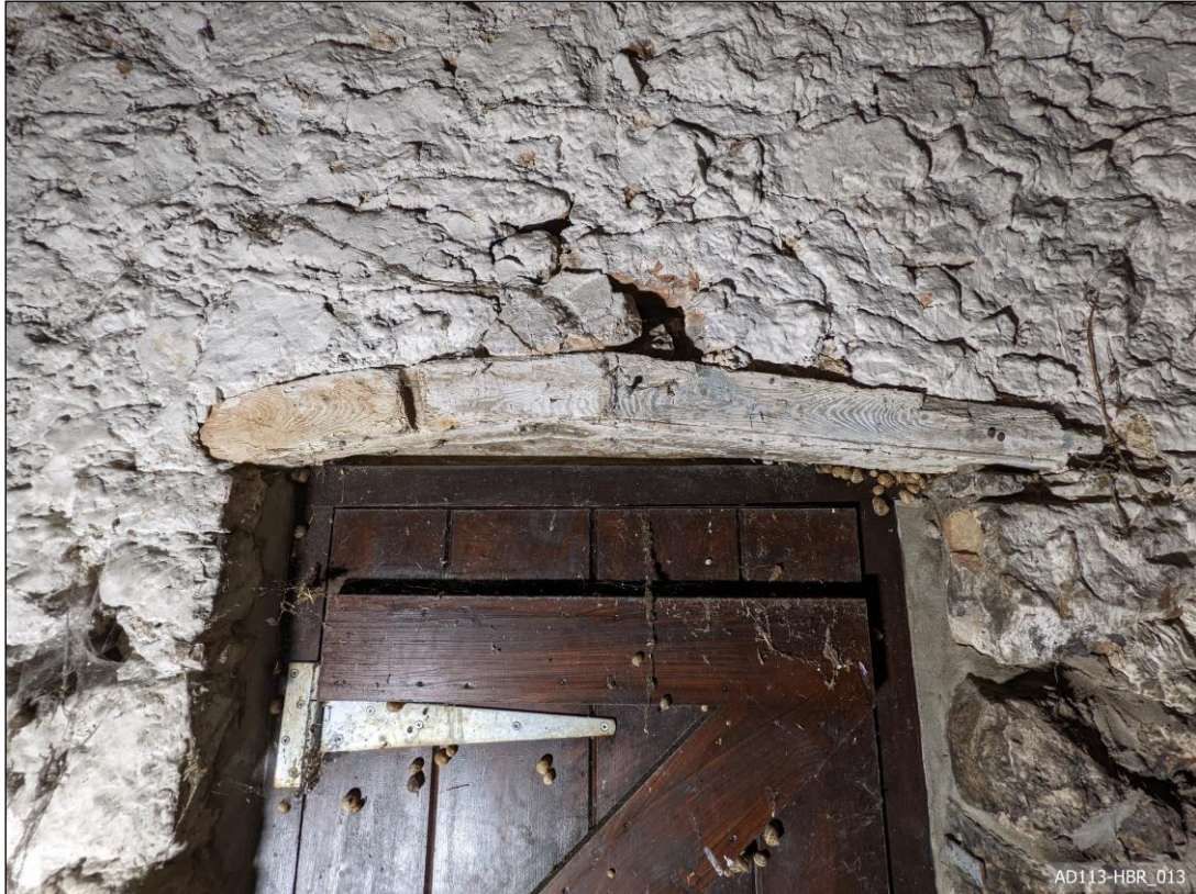
Plate 13 – View east, showing reused joist as lintel.
