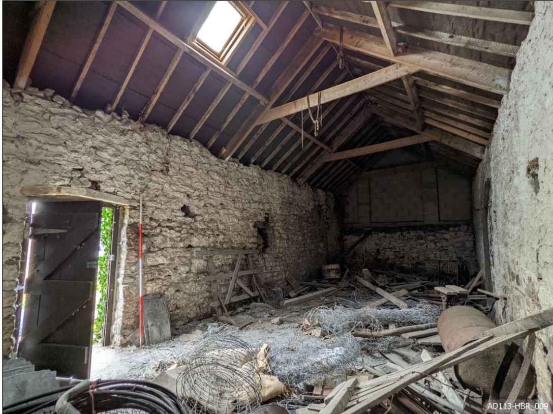
Plate 9 – View south, showing barn internal space.
