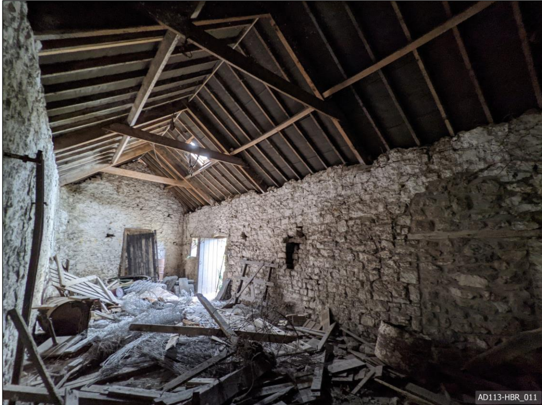
Plate 11 – View north, showing barn internal space.
