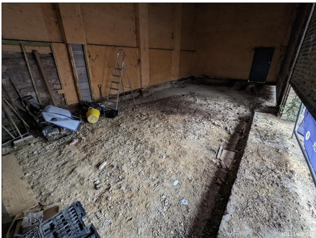
Plate 42 – View south-west, showing Area 2.
