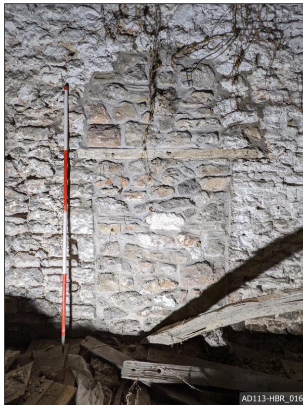
Plate 16 – View east, showing blocked doorway to bay 3.
