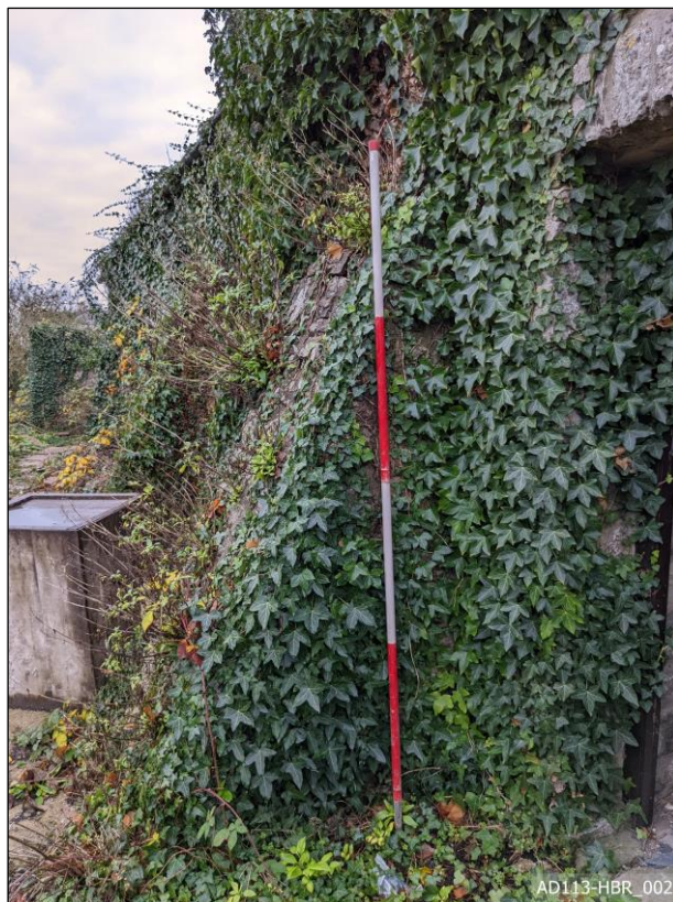
Plate 2 – View south, showing buttress to west elevation.
