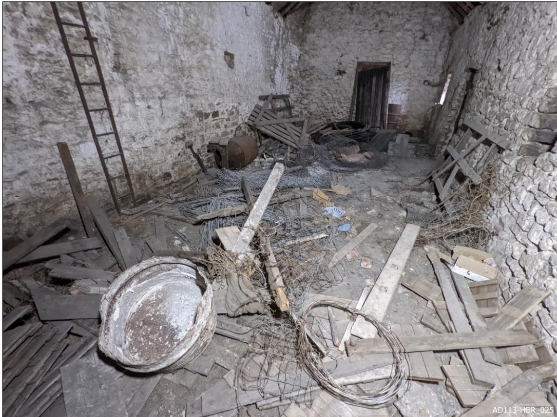
Plate 25 – View north-west, showing stored materials and items.
