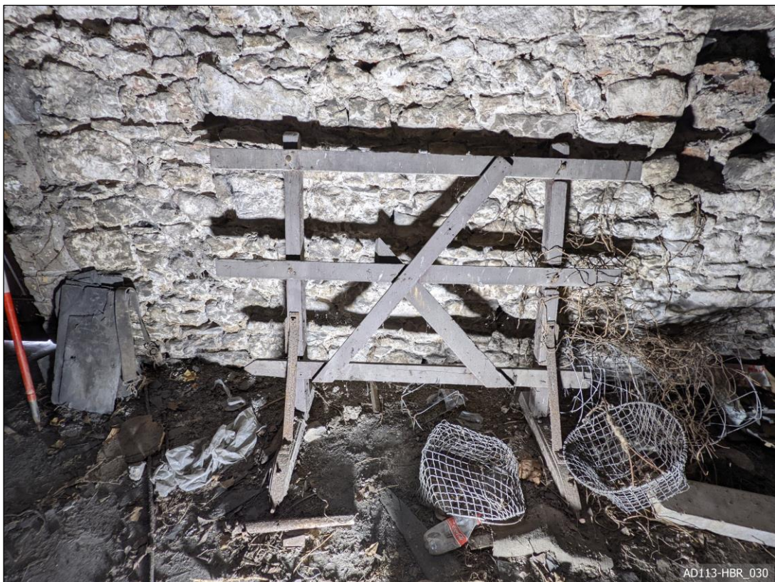
Plate 30 – View east, showing railway station platform barrier.
