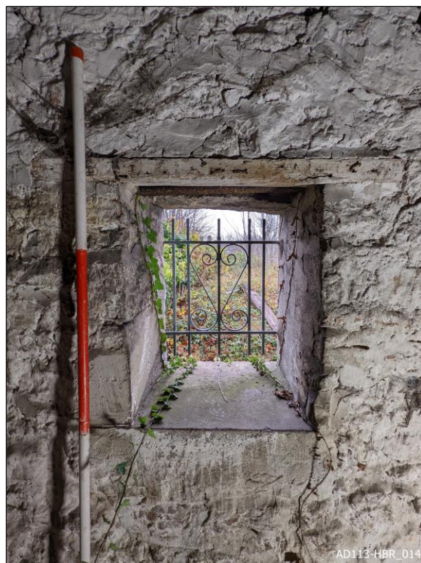
Plate 14 – View east, showing window.
