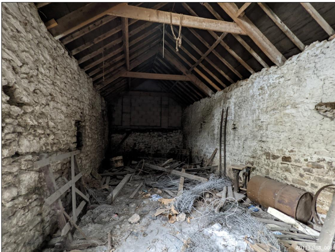
Plate 8 – View south, showing barn internal space.
