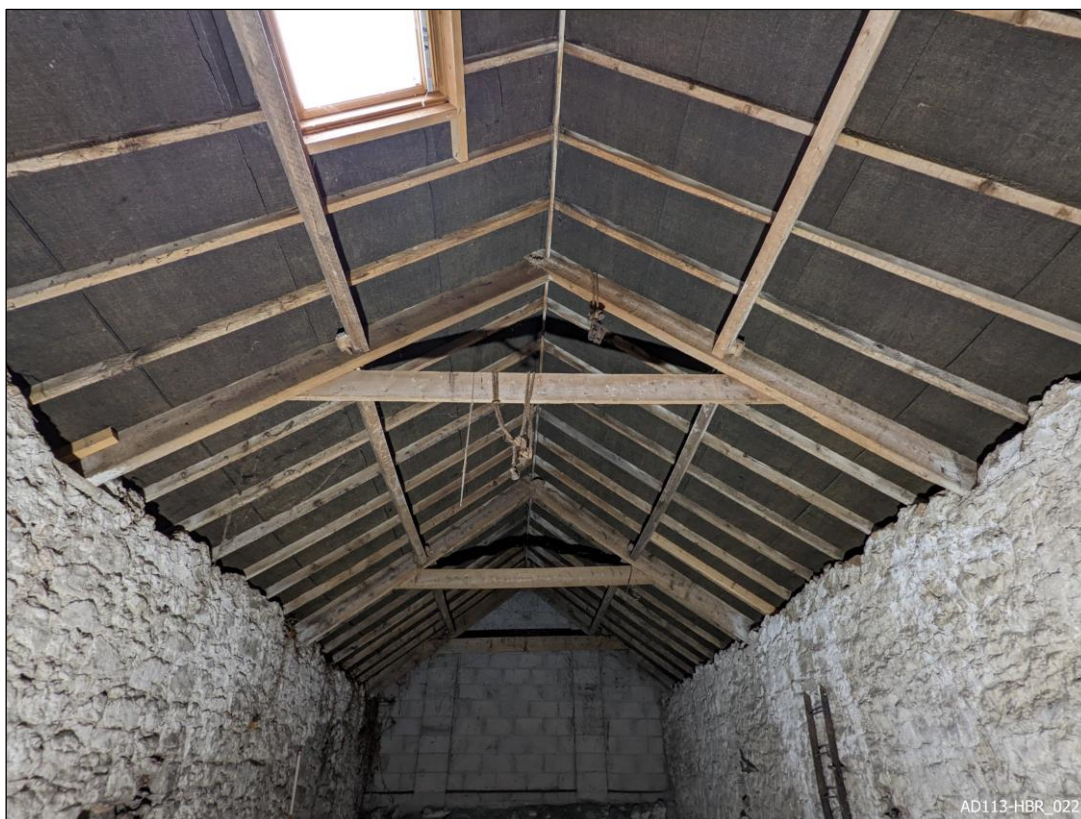
Plate 22 – View south, showing exemplar roof truss.
