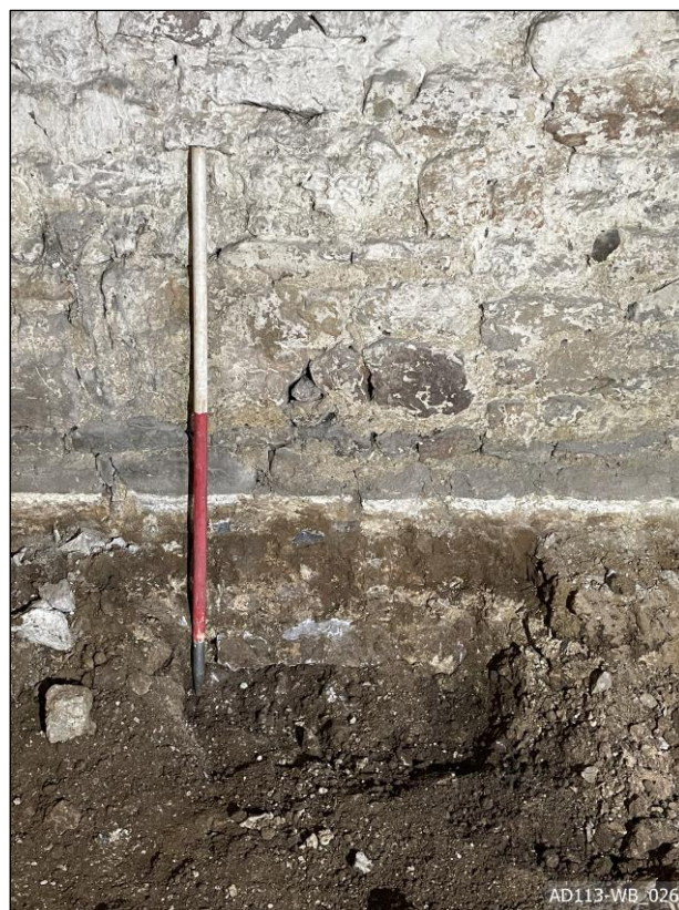
Plate 56 – View west, showing wall footing.
