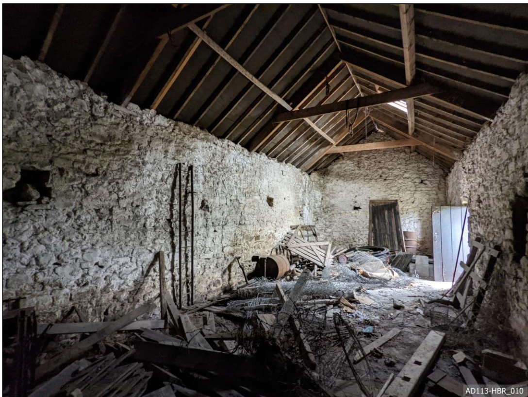
Plate 10 – View north, showing barn internal space.
