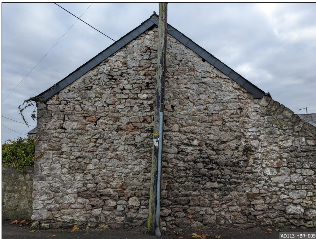
Plate 5 – View south, showing north elevation.
