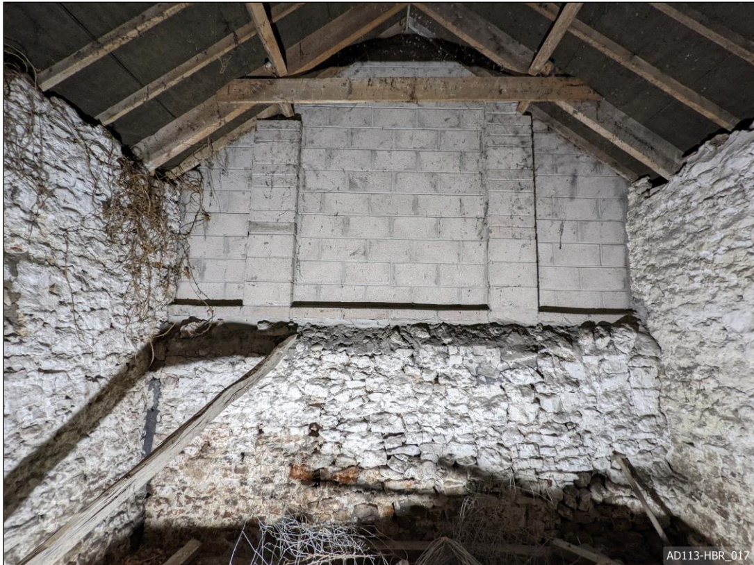
Plate 17 – View south, showing partition wall, with concrete block upper wall.
