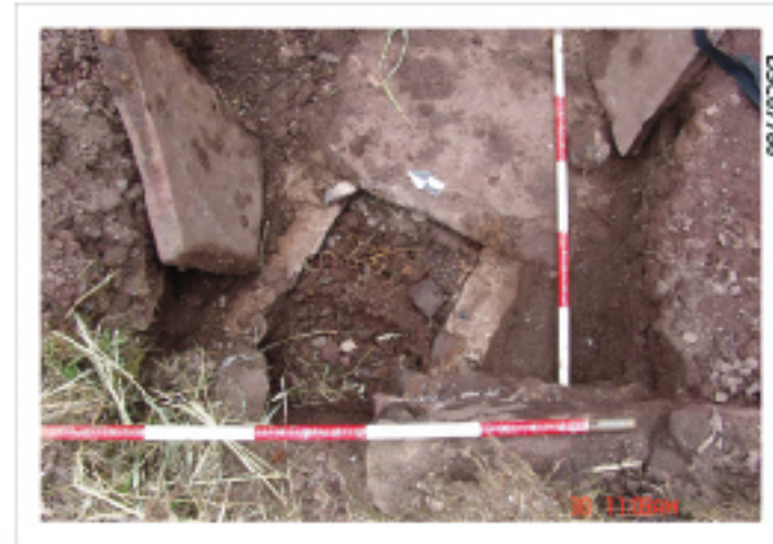
Plate 40: Upper covered culvert. Capstone removed showing lining and fill
