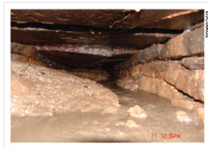
Plate 57: Eastern culvert from the wheelpit hutch. Silt level and broken capstones
