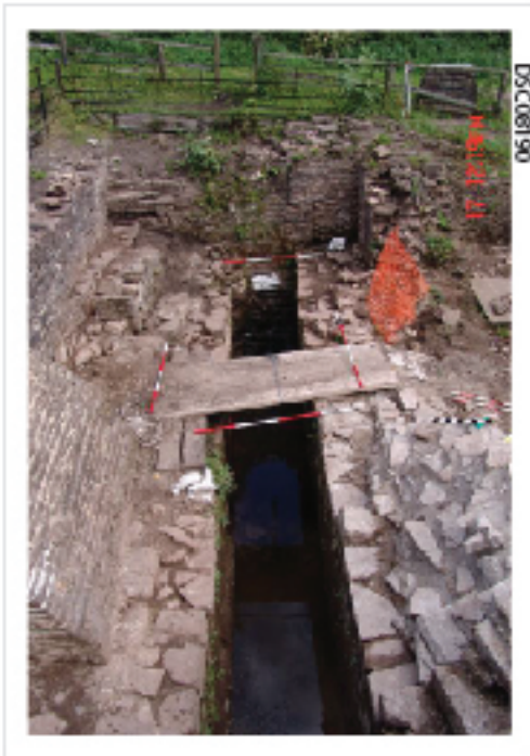
Plate 61: Wheelpit. Measured photographic recording.
