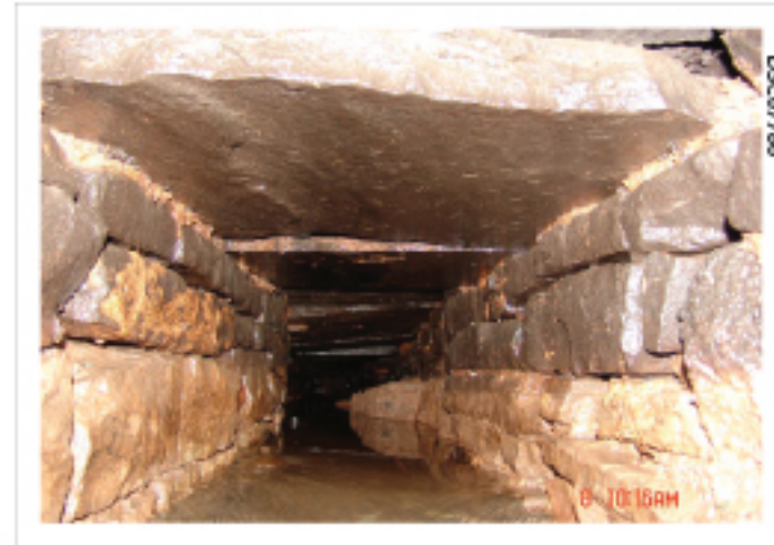
Plate 27: Main Culvert, excavation in K. View towards wheelpit. Silt on left
