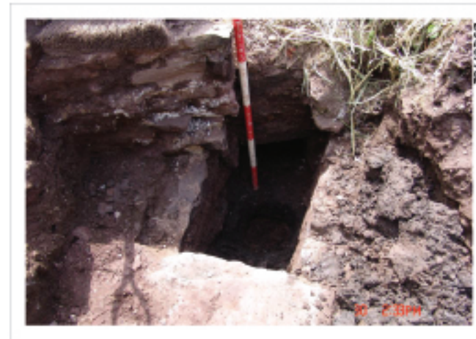
Plate 15: Upper culvert at join under 198 after clearing of silt
