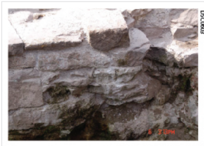
Plate 59: Wheel pit water wheel rub marks
