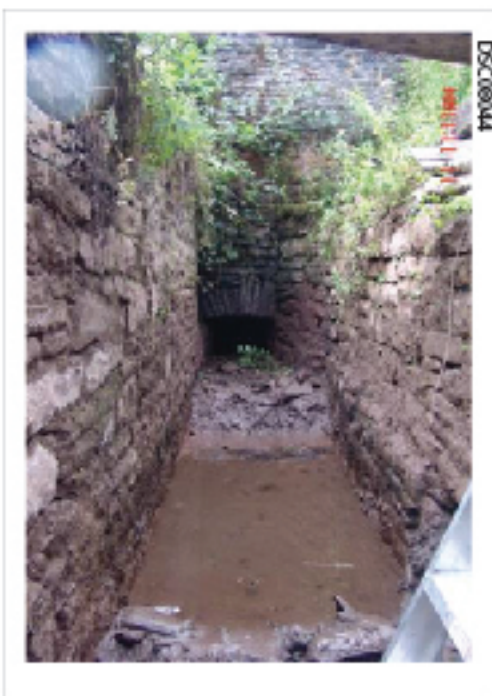
Plate 20: Drained wheelpit showing hutch under rear furnace wall
