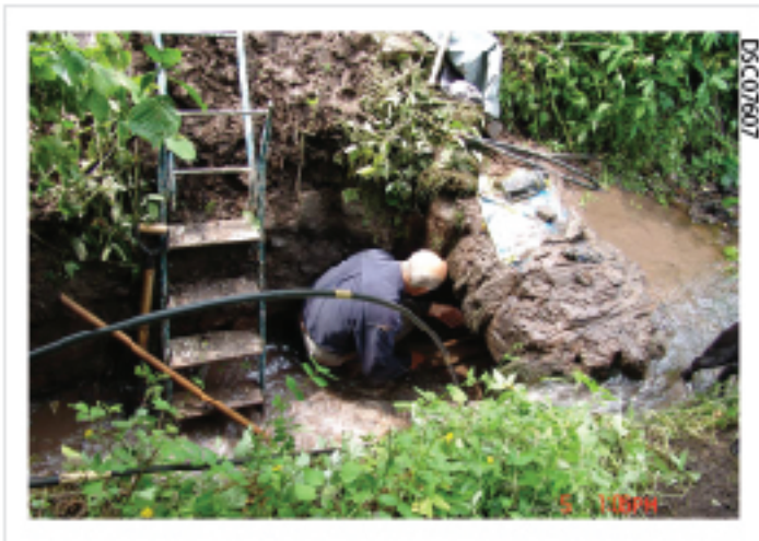
Plate 04: Rodding out the culvert after further de-silting (WB/JB/10).
