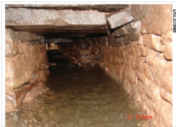
Plate 30: View down culvert below cottage, from open capstone area
