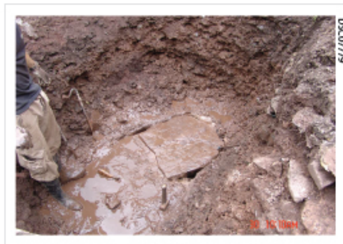
Plate 44: Excavation in K. Main covered culvert
