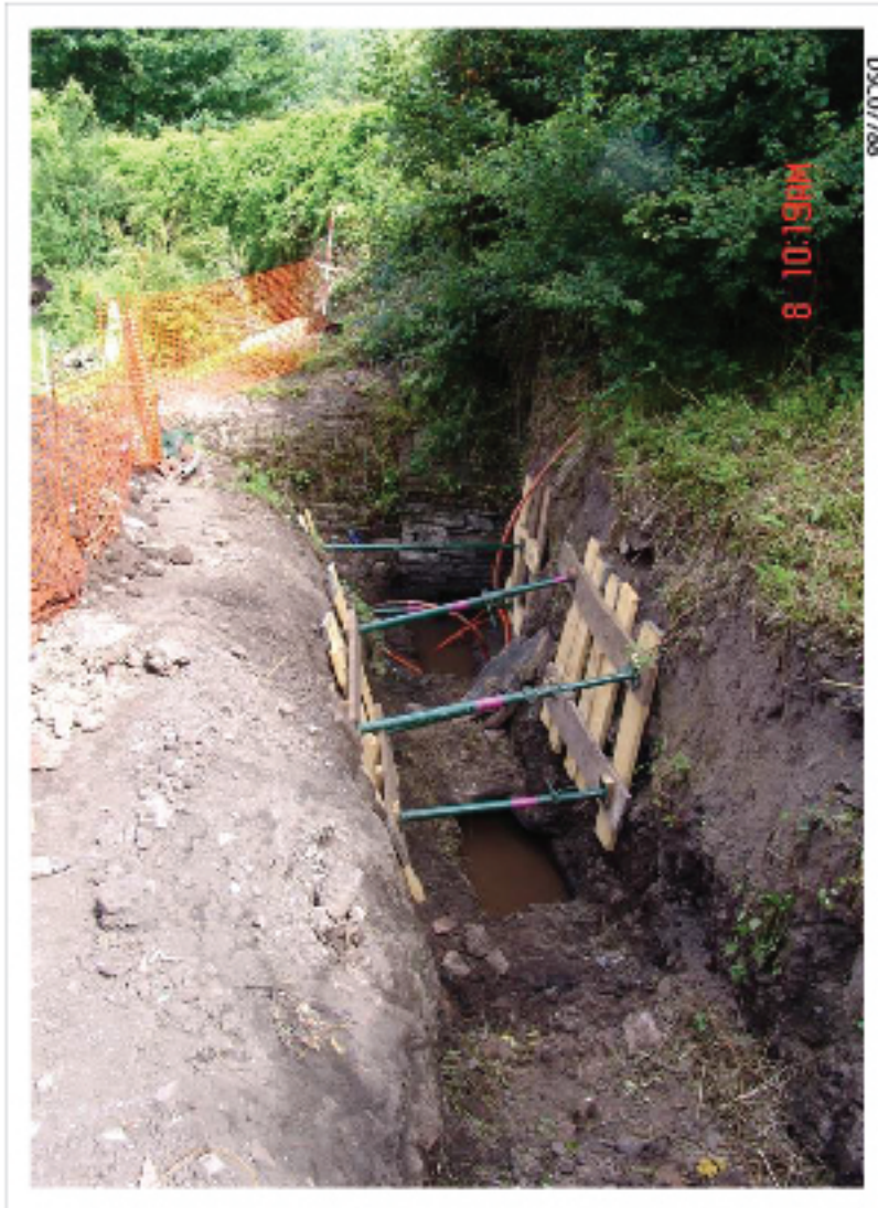
Plate 11: View along culvert at cottage, with partial removal of capstones
