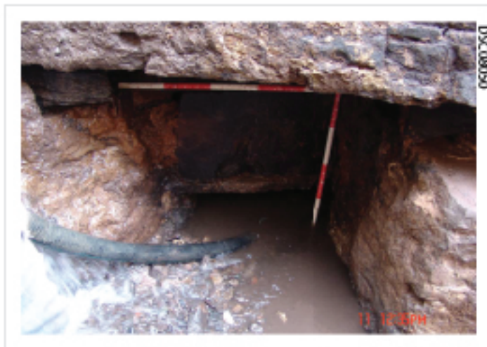
Plate 56: Eastern hutch in drained wheelpit showing wooden lintel and socket.
