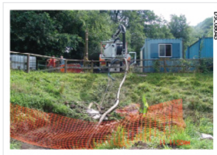
Plate 16: Desilting through sump: 204 (Pickin1982)
