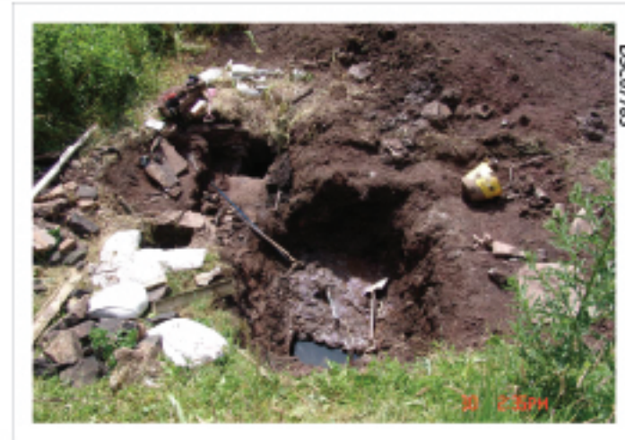
Plate 12: Overview of excavation in K showing both culverts
