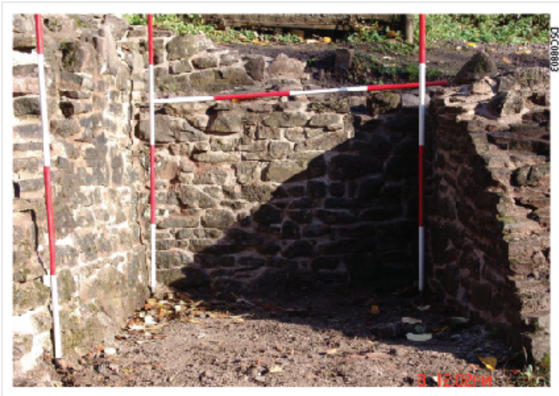
Plate 82: Enclosure behind blowing house after consolidation
