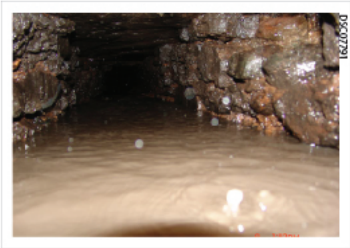
Plate 46: View along culvert from test pit 1
