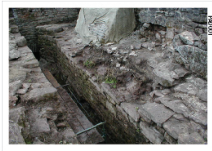
Plate 78: Wheelpit. Upperwall, clearing
