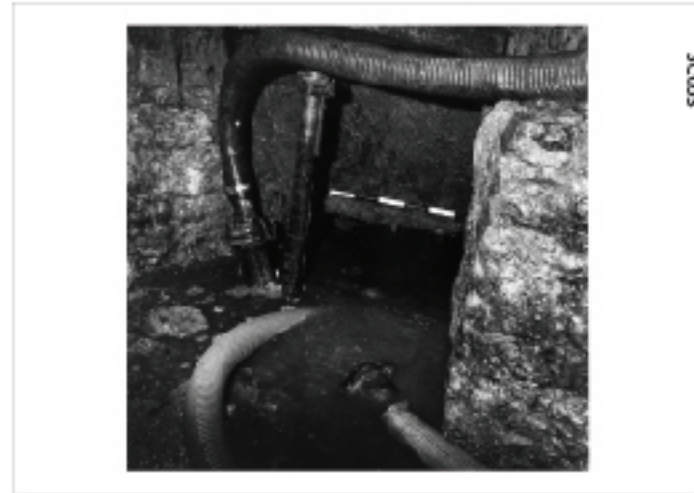
Plate 55: Wheelpit hutch 207 internal view during excavation summer 1979
