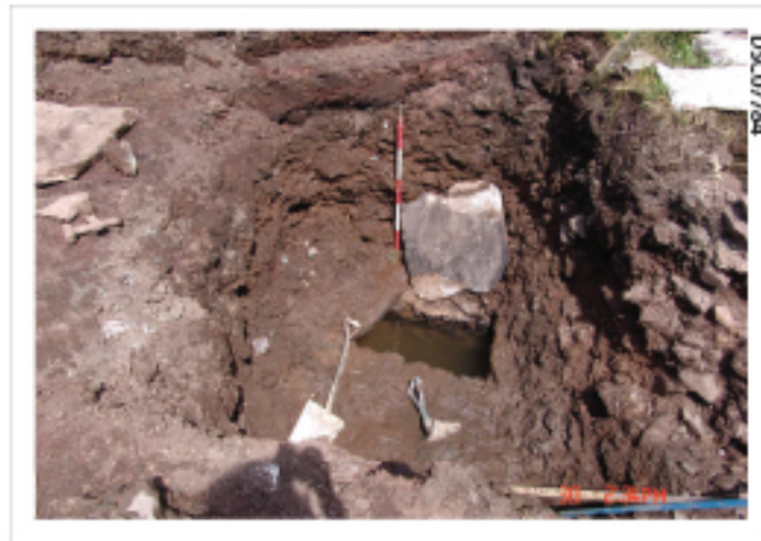
Plate 14: Main Culvert, excavation in K with capstone lifted
