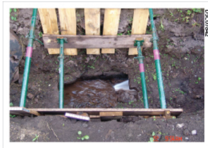
Plate 32: Jetting operation in Cottage outfall, culvert
