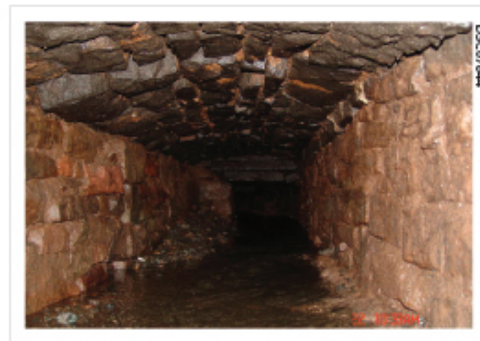
Plate 28: Cottage outflow at south end of covered culvert. Internal details
