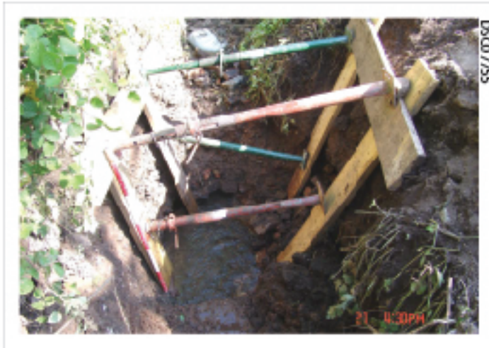
Plate 08: Culvert beside cottage, water levels reduced.
