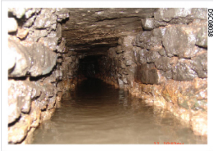
Plate 47: Test pit 1 culvert after de silting. View along culvert, towards wheelpit.
