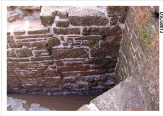
Plate 54: Phasing detail, wheelpit after repointing
