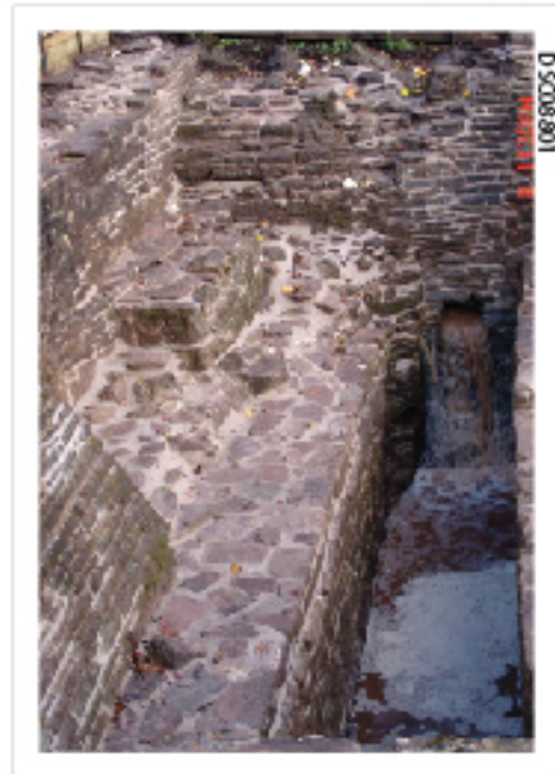
Plate 63: Overview of wheelpit after consolidation
