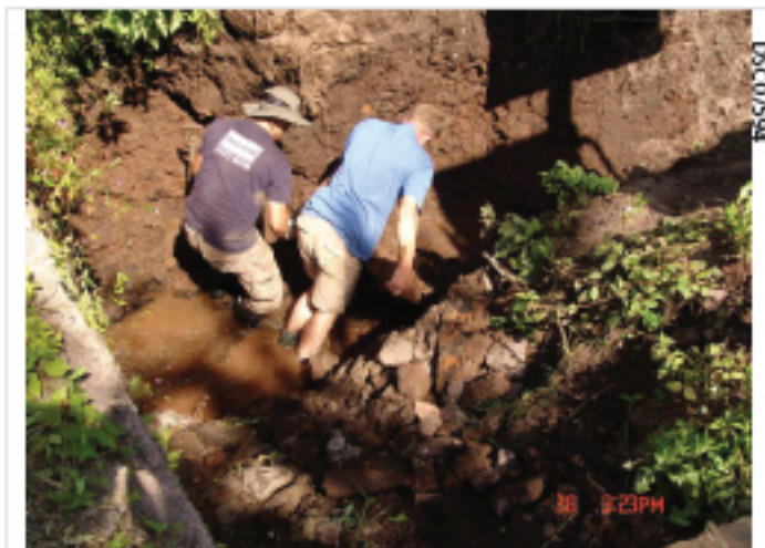
Plate 09: Lifting of capstone from culvert close to the cottage wall
