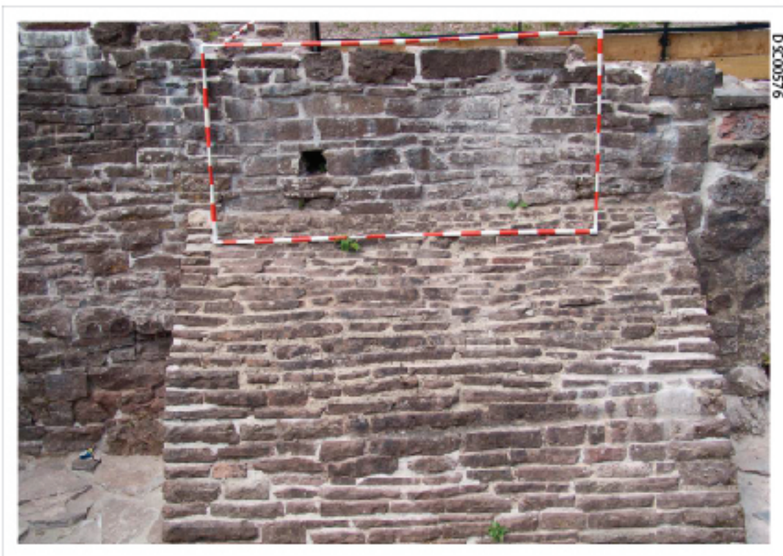
Plate 62: Final elevation record, Upper wheel pit 5
