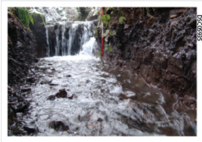
Plate 02: View of culvert resurgence after 1m de-silting (WB/ACNB2/09)
