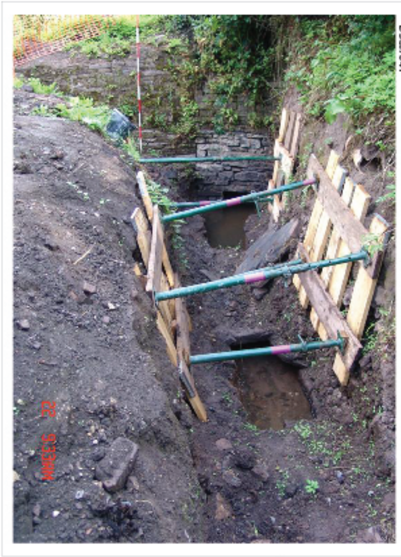
Plate 31: Later view along culvert at cottage, prior to jetting
