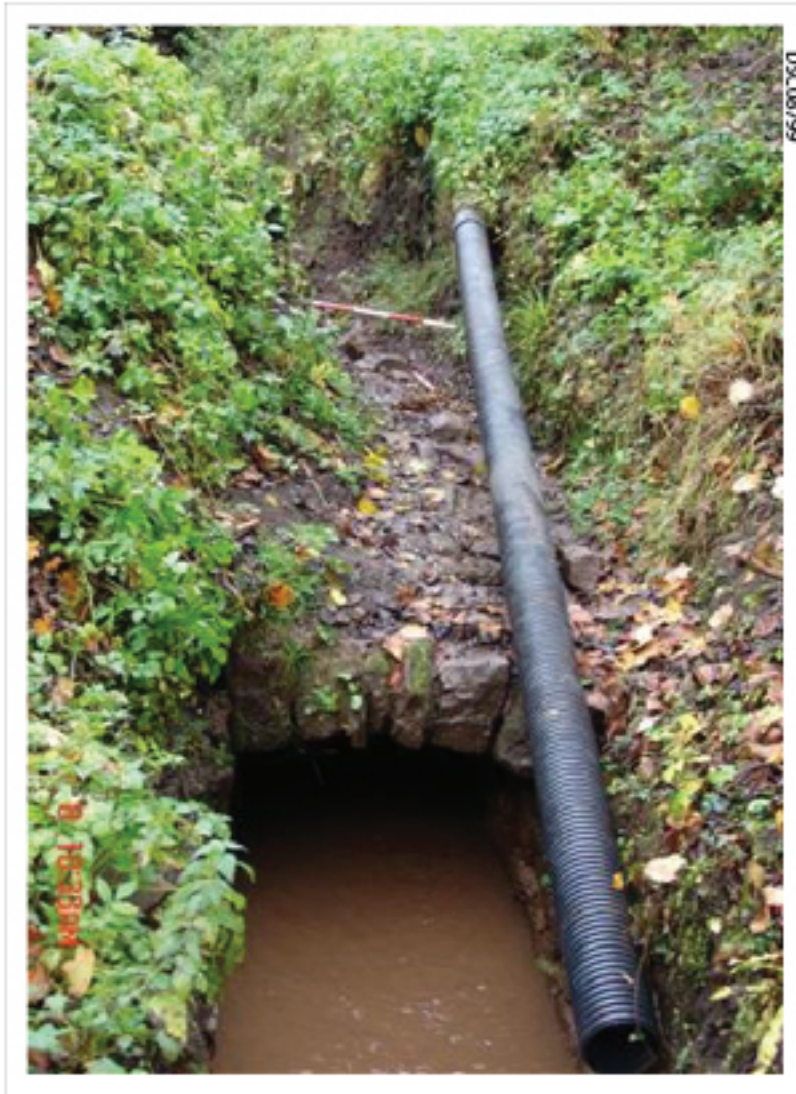
Plate 26: Culvert prior to back fill.
