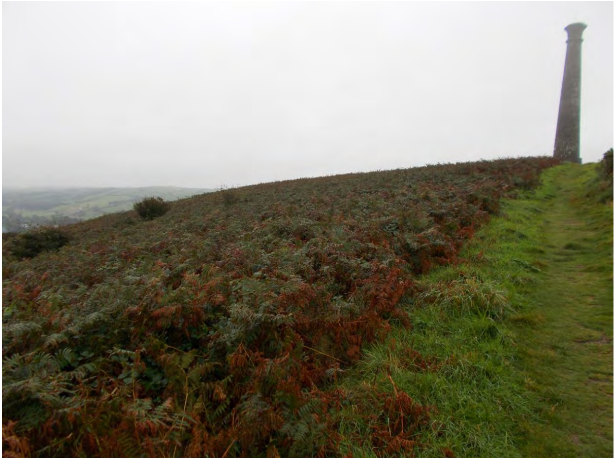
Photo 3: The main area of the 'South Fort' prior to vegetation clearance, looking south.
