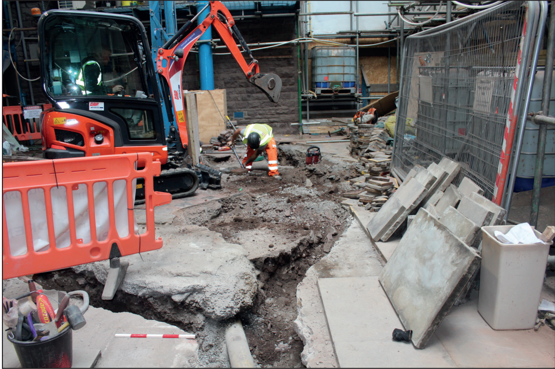
Trenches 13, 14 and 15 during groundworks, looking north-west (0.5m scale)
