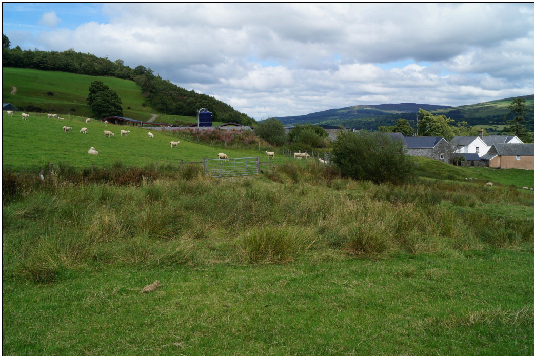
Plate 24: TYF2020_024. Looking northeast. A view towards Tyfos Farm showing the farmhouse, the older buildings on the farmyard, and the newer structures to the northwest.
