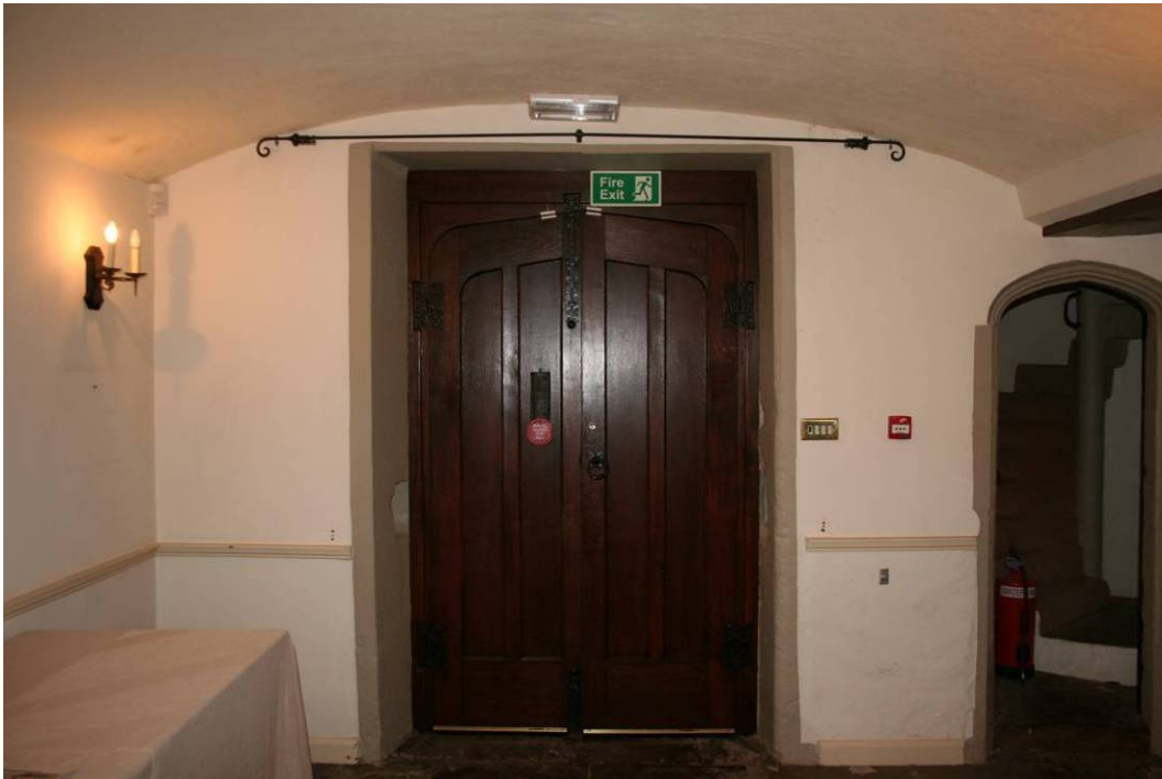
Photo 64: Main doorway from the inside of Entrance Lobby 014
