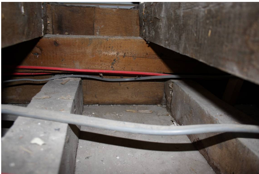
Photo 41: The Chapel Lounge 121 showing joist attachments to cross-beam
