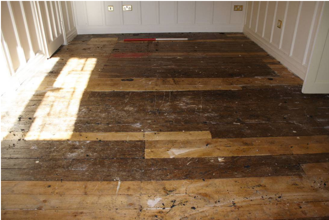
Photo 24: Room 103 before floorboards were removed
