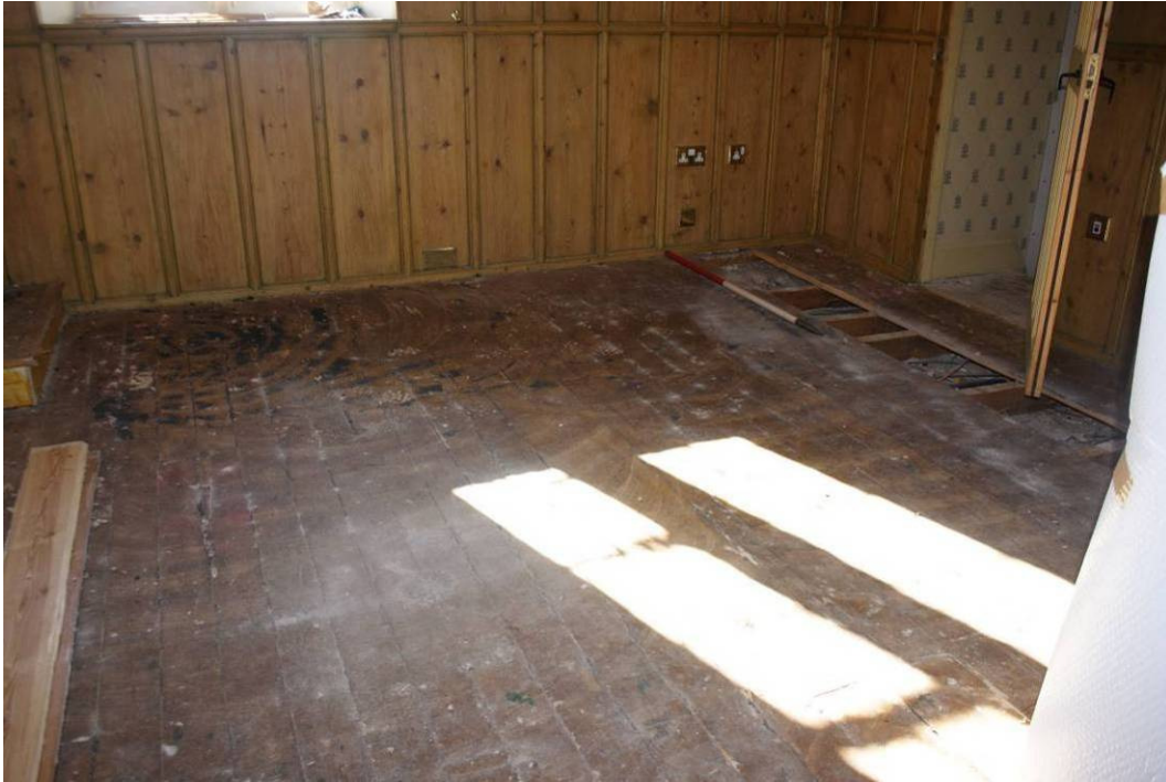
Photo 81: Bedroom 109, floorboards prior to removal
