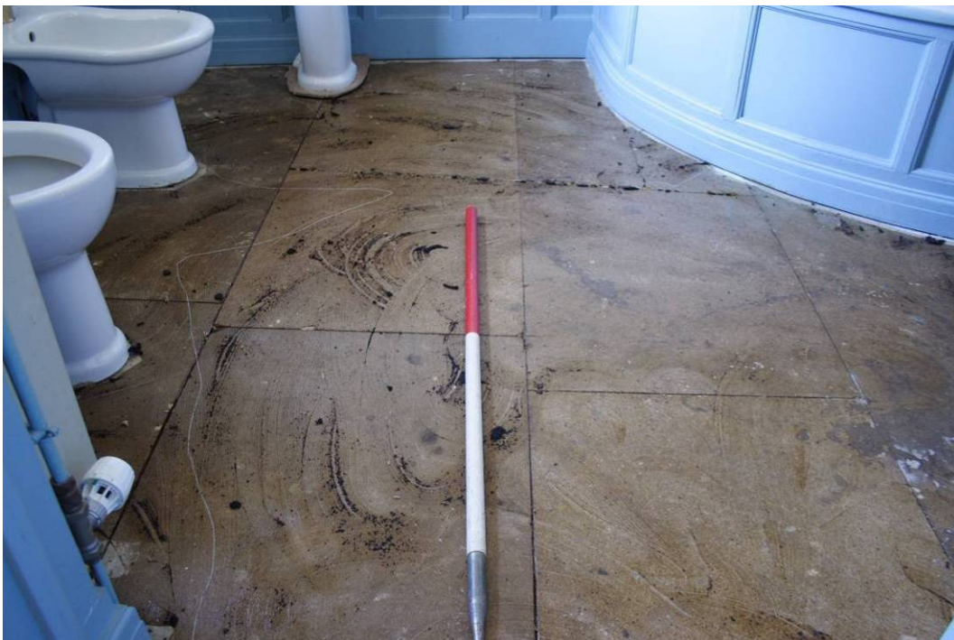
Photo 31: Bathroom 107 showing chipboard flooring
