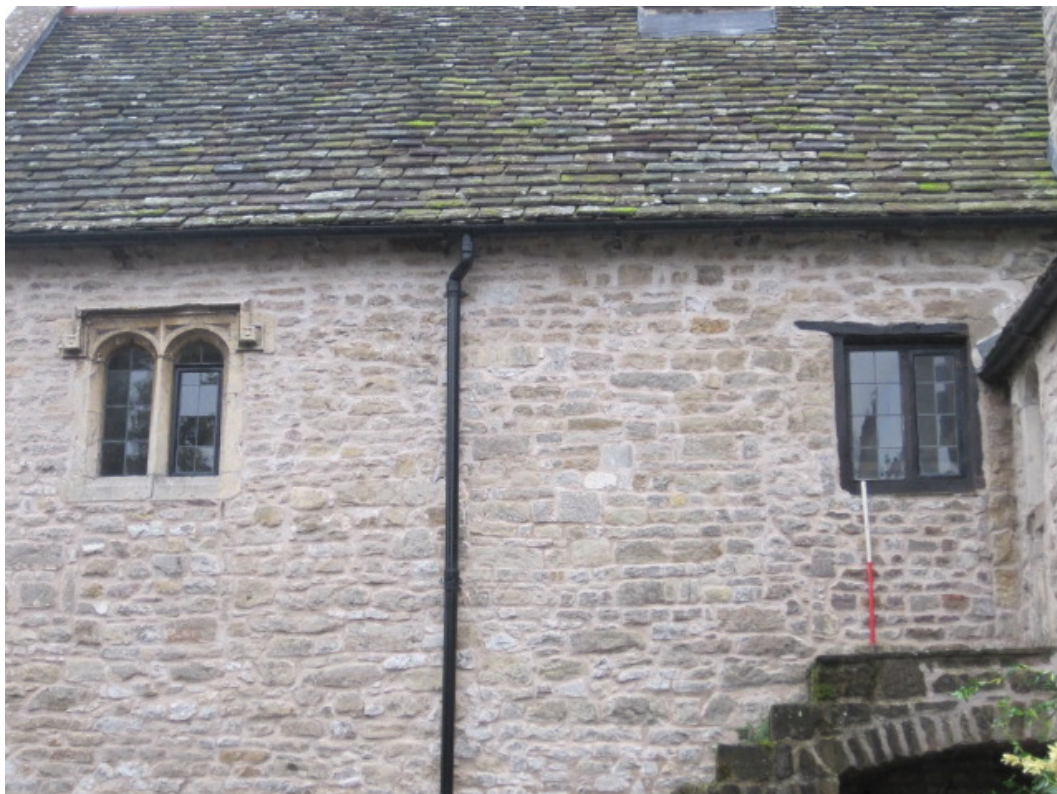
Photo 11: Window opening and blocked doorway before commencement of works
