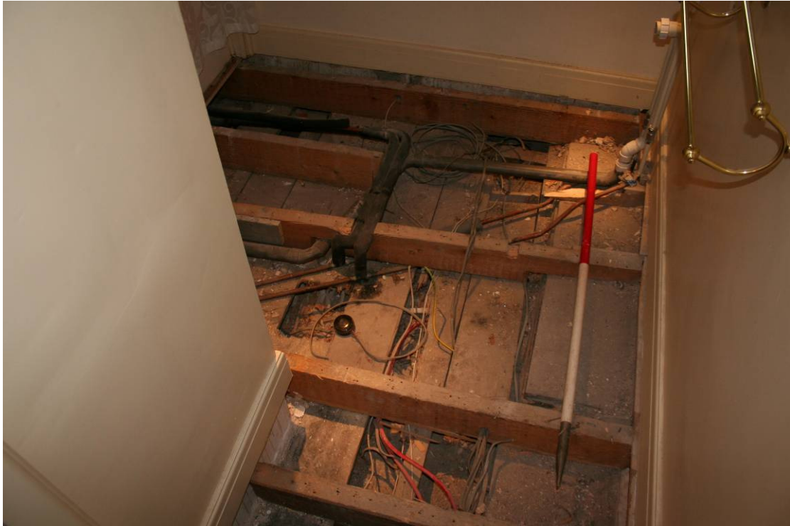
Photo 50: Bathroom 117 following removal of floorboards, viewing NE
