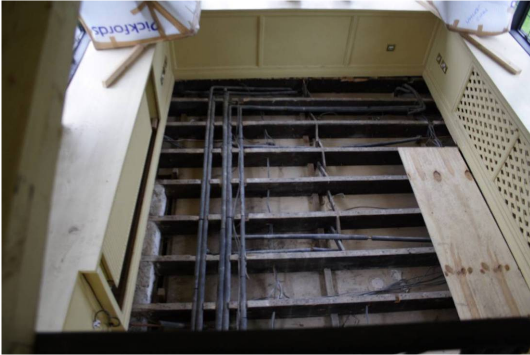
Photo 20: The Gazebo Lounge 101, following removal of floorboards
