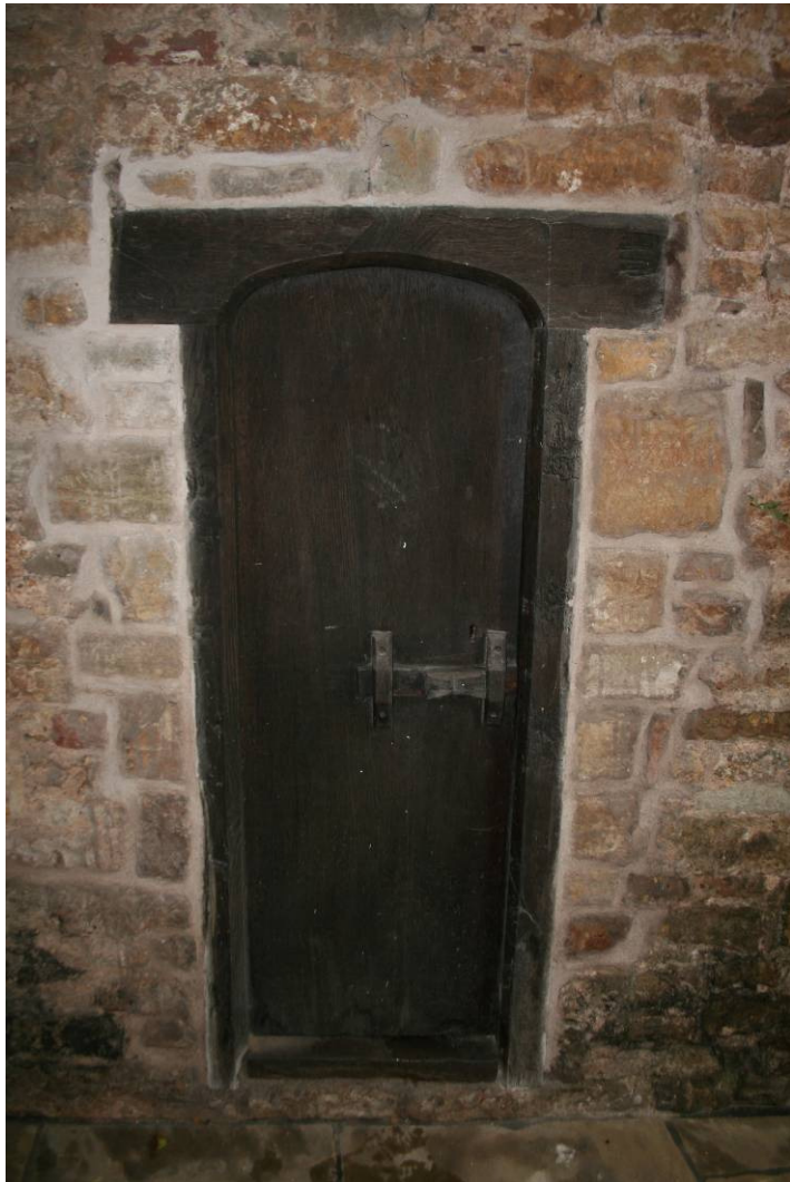
Photo 68: Doorway in exterior passage to Room 035
