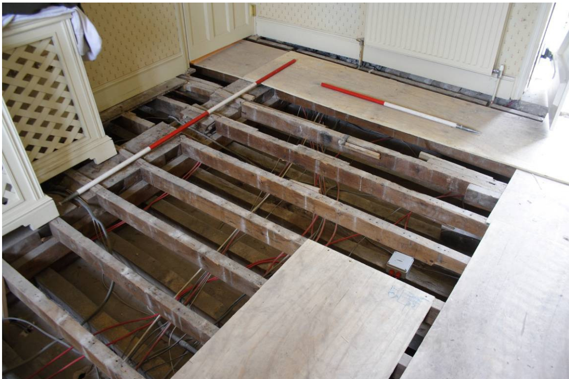
Photo 40: The Chapel Lounge 121 following removal of floorboards, showing underlying joist arrangement
