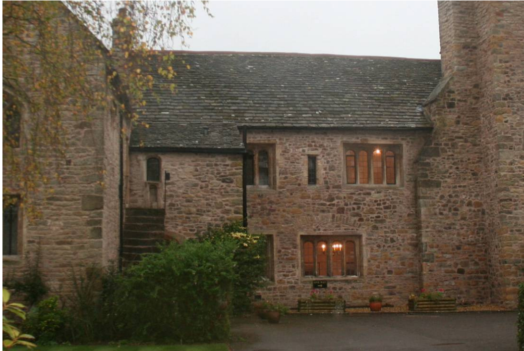
Photo 7: NE facade of central section from NE
