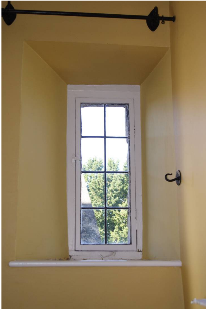
Photo 93: Window in NW wall of Bedroom 201
