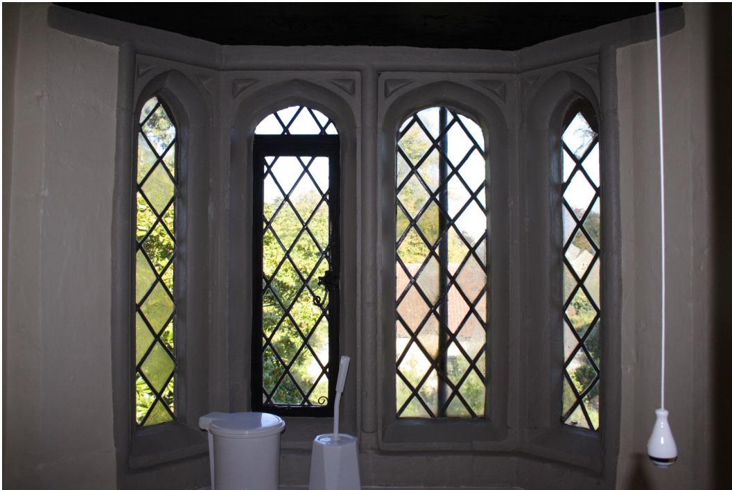
Photo 112: Four light, bayed window in Bathroom 204
