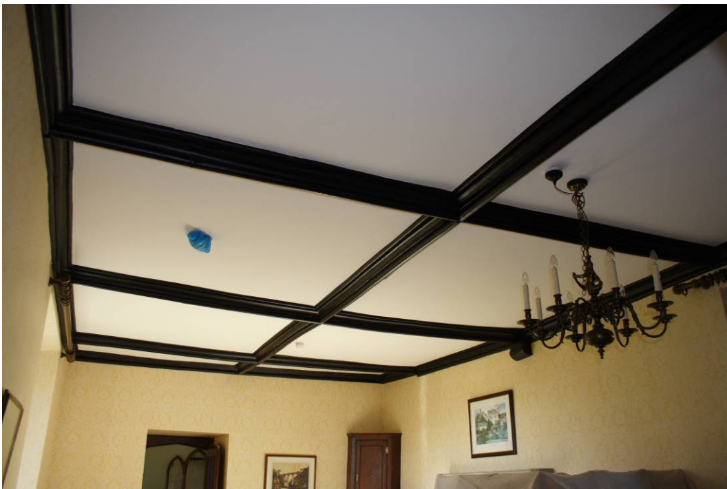
Photo 59: Ceiling of Lounge 015, viewing NW, showing ornate beams
