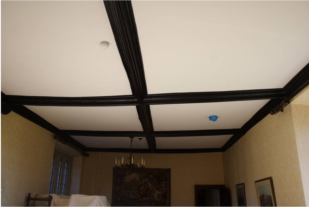
Photo 60: Ceiling of Lounge 015, viewing SE, showing ornate beams
