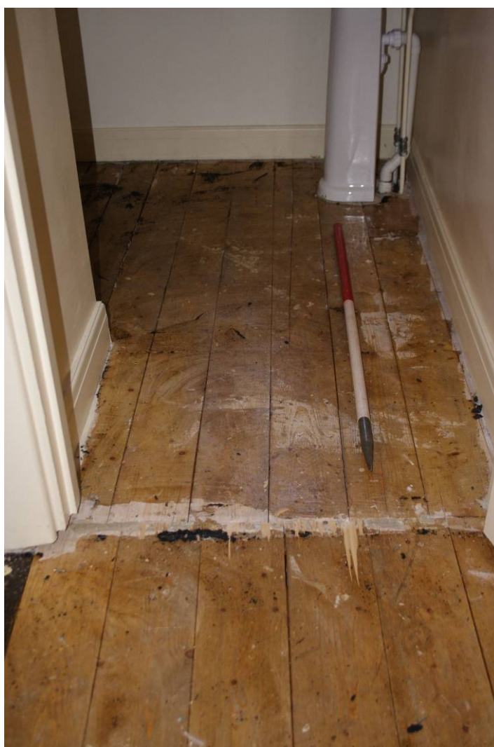
Photo 49: Bathroom 117 prior to removal of floorboards, viewing NE
