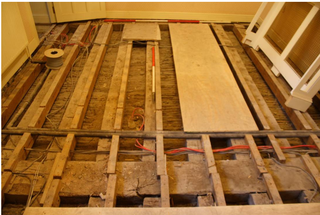
Photo 48: Bishop Miles Godwin Bedroom 116 following removal of floorboards, viewing SE
