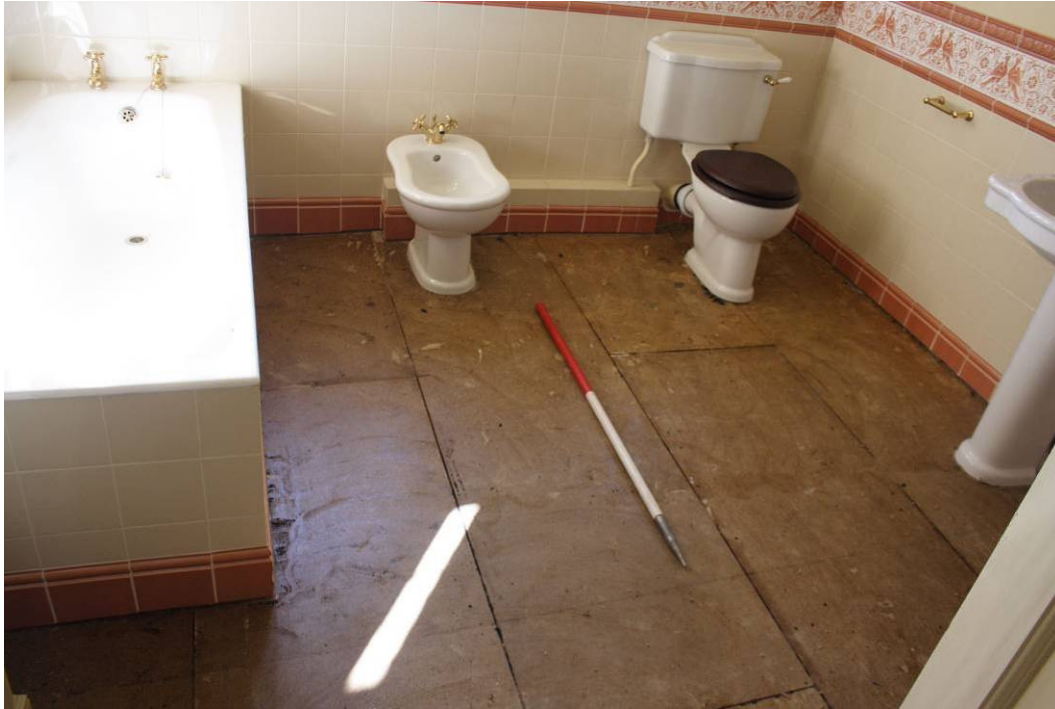
Photo 42: The Chapel Suite Bathroom 120, before removal of flooring
