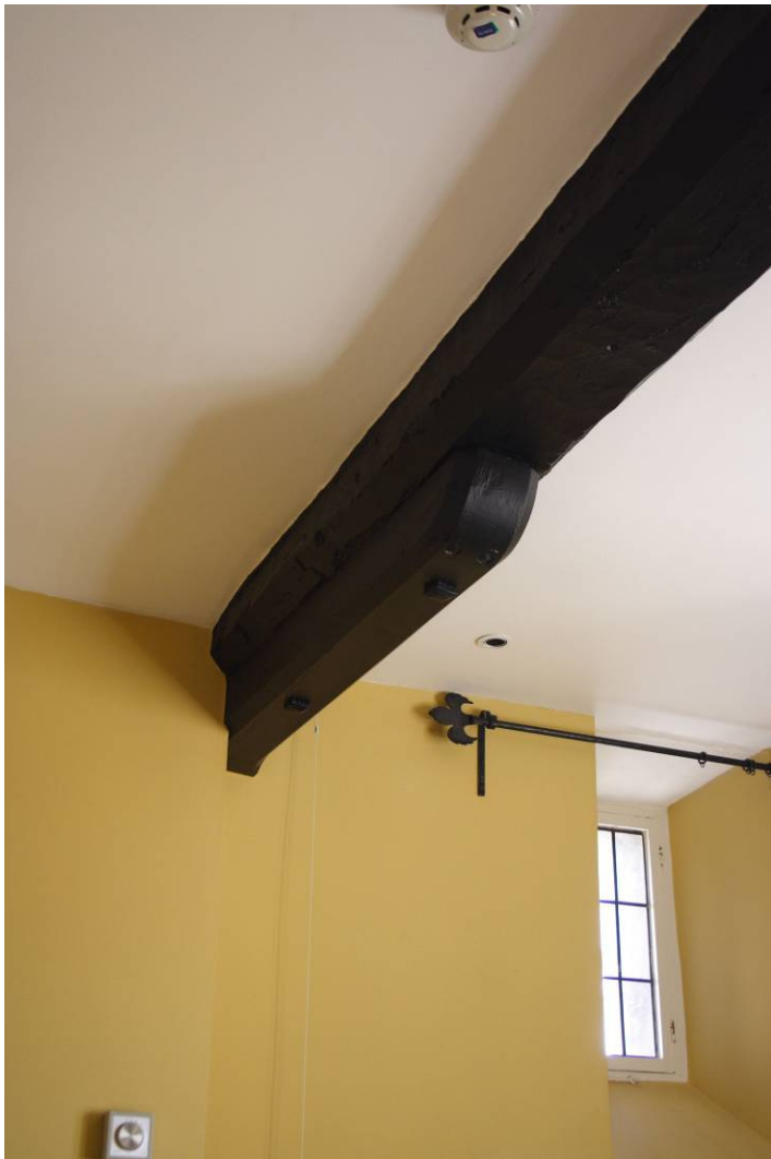
Photo 113: SW beam in ceiling of Bedroom 203, with more recent support beneath
