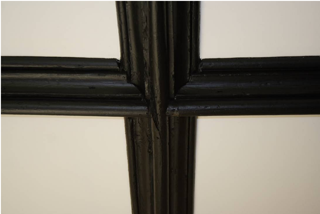
Photo 61: Detail of beams in ceiling of Lounge 015, showing ornate moulding
