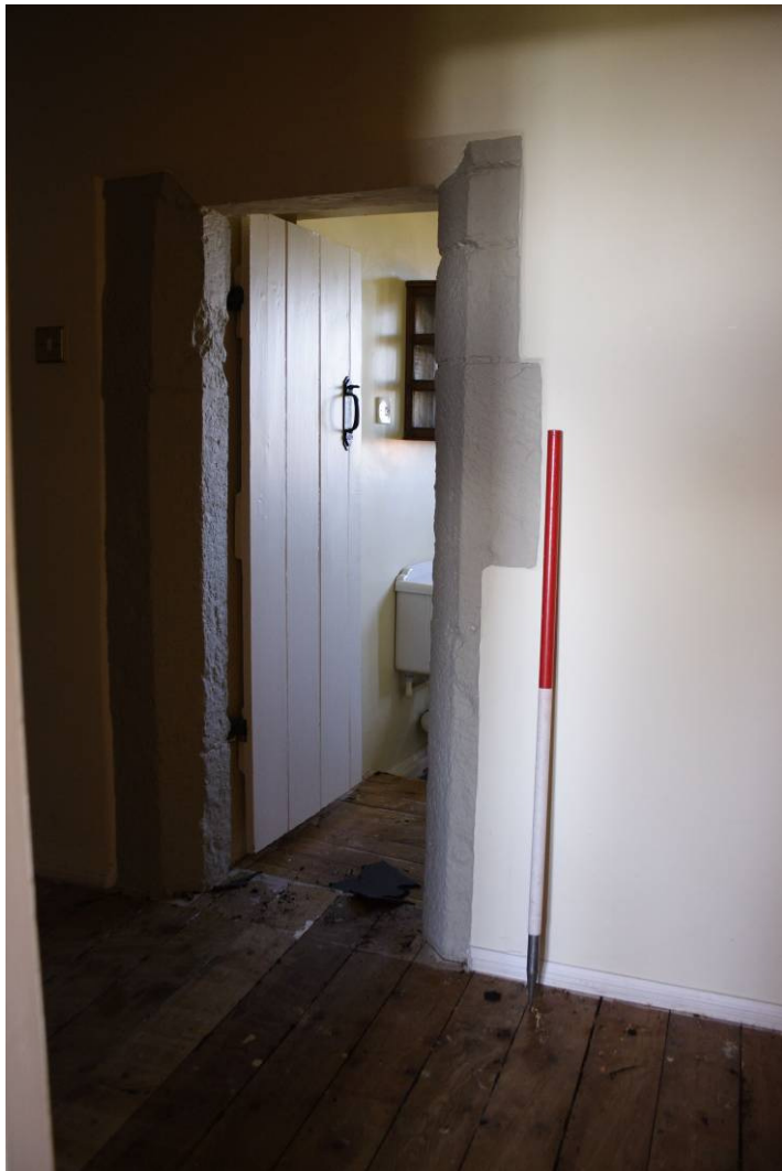
Photo 100: Corridor 205 looking towards Bathroom 205 showing stone framed doorway
