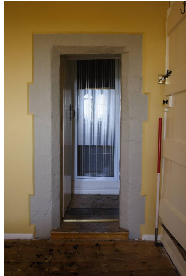
Photo 90: Stone framed doorway to Bathroom 202
