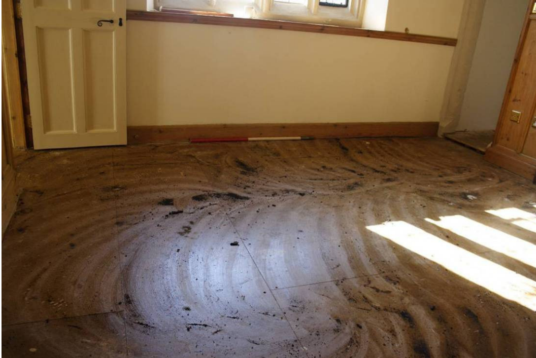
Photo 73: Bishop de La Zouche Lounge 111, ply-board sheet flooring
