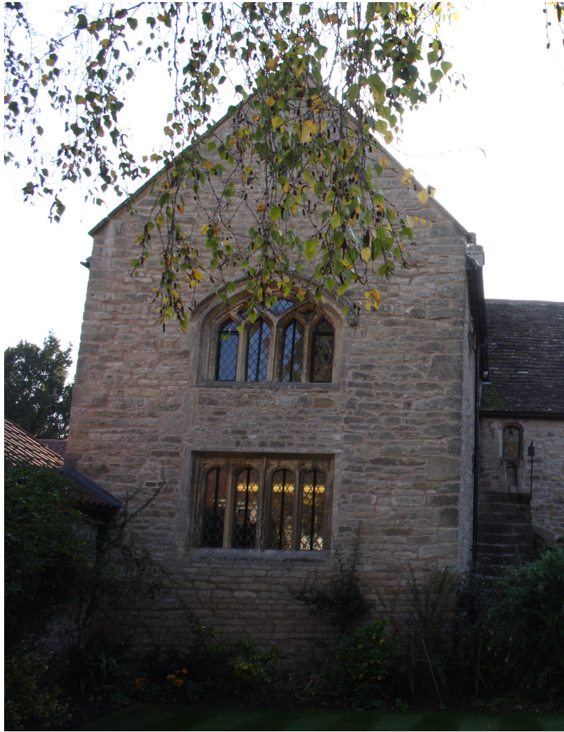
Photo 10: SE facade of SE wing showing original mullioned windows of chapel
