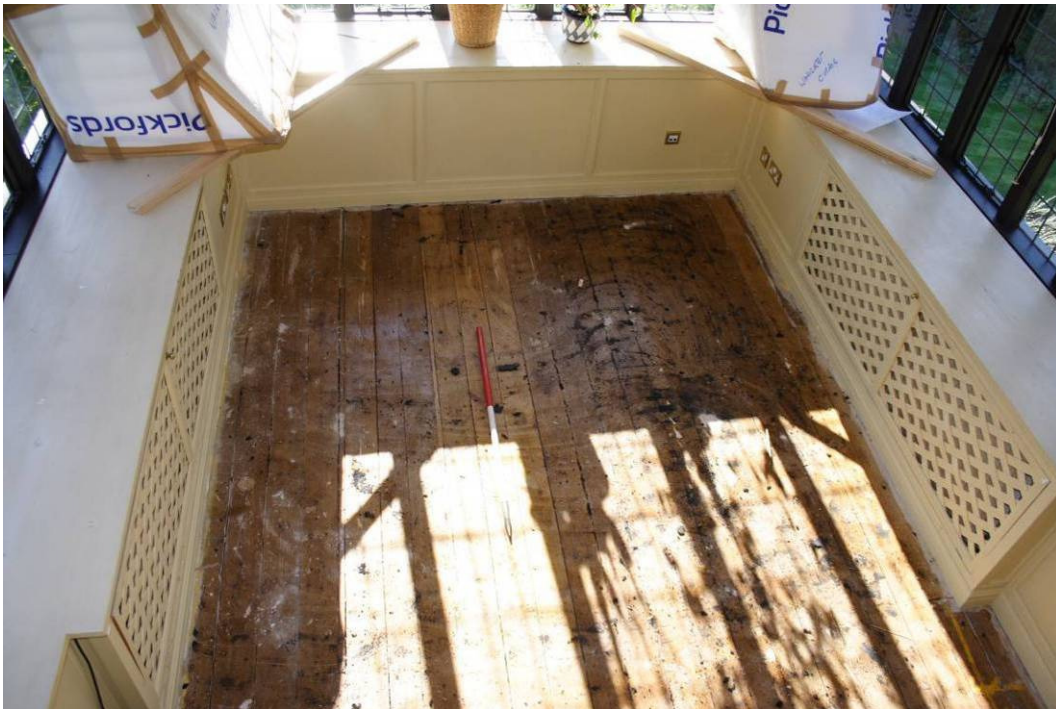
Photo 19: The Gazebo Lounge 101, floorboards prior to removal
