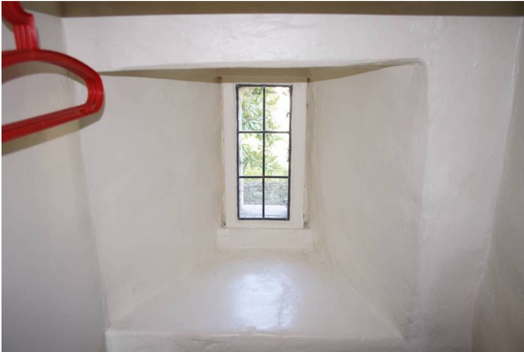
Photo 85: Window in NE wall of Store 110
