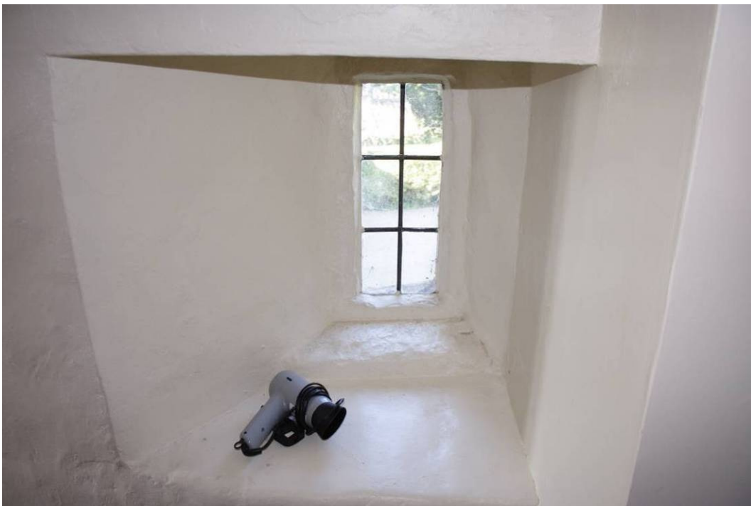
Photo 86: Window in NW wall of Store 110
