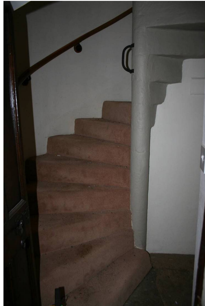
Photo 72: Spiral stone stairs in Stair 036
