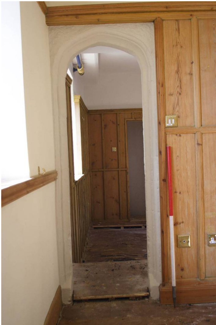
Photo 75: Stone framed doorway to Bedroom 109
