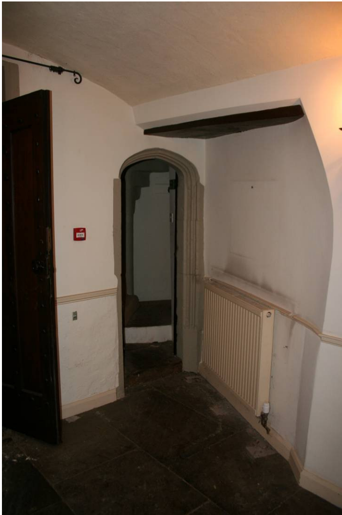
Photo 66: Doorway to Stair 035 in ground floor of Tower and adjacent recess
