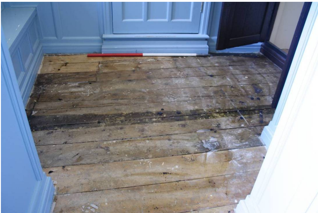
Photo 29: Lobby 106 viewing NE prior to removal of floorboards
