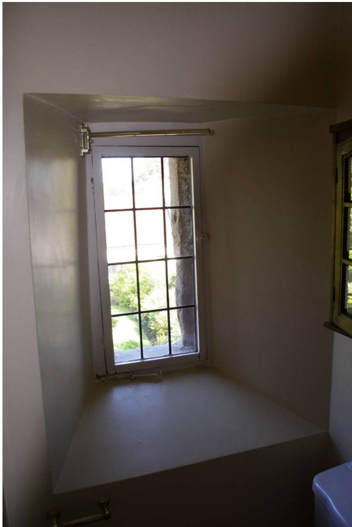
Photo 95: Window in NE wall of Bathroom 202
