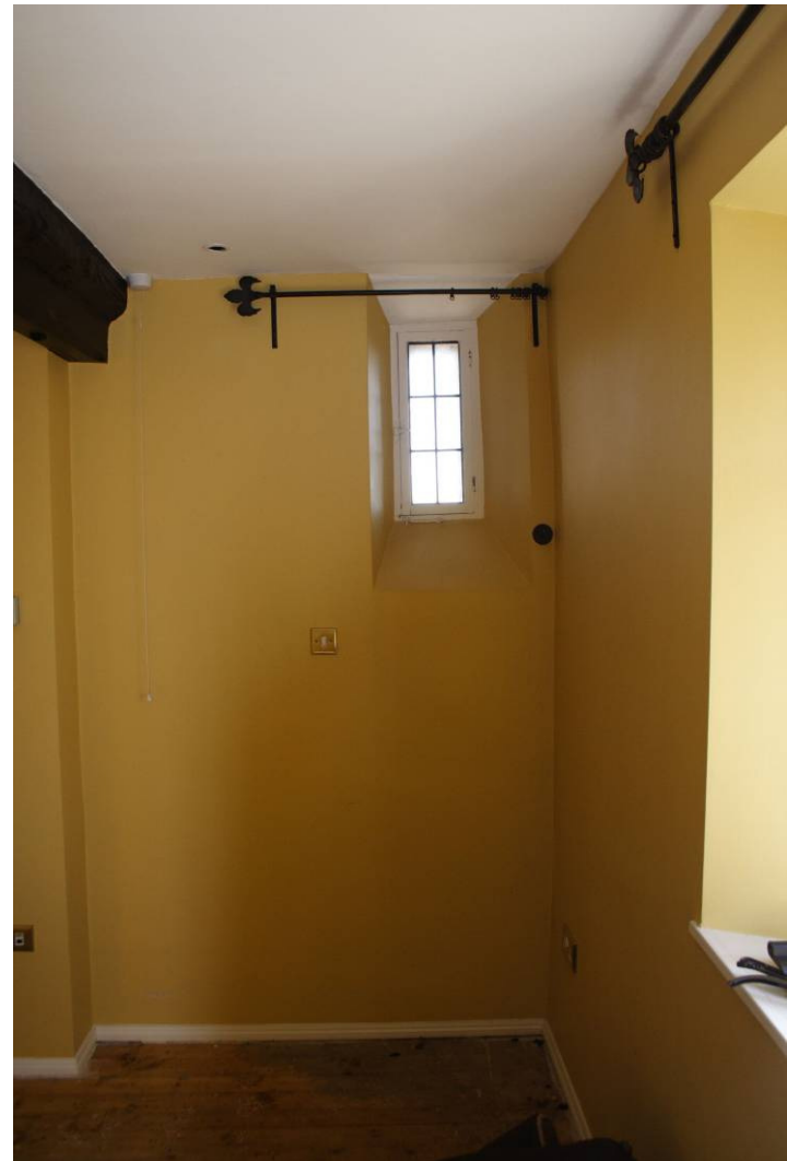
Photo 108: Window in SE wall of Bedroom 203
