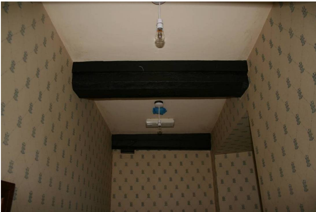
Photo 70: Exposed beams in ceiling of Room 012 in ground floor of Tower
