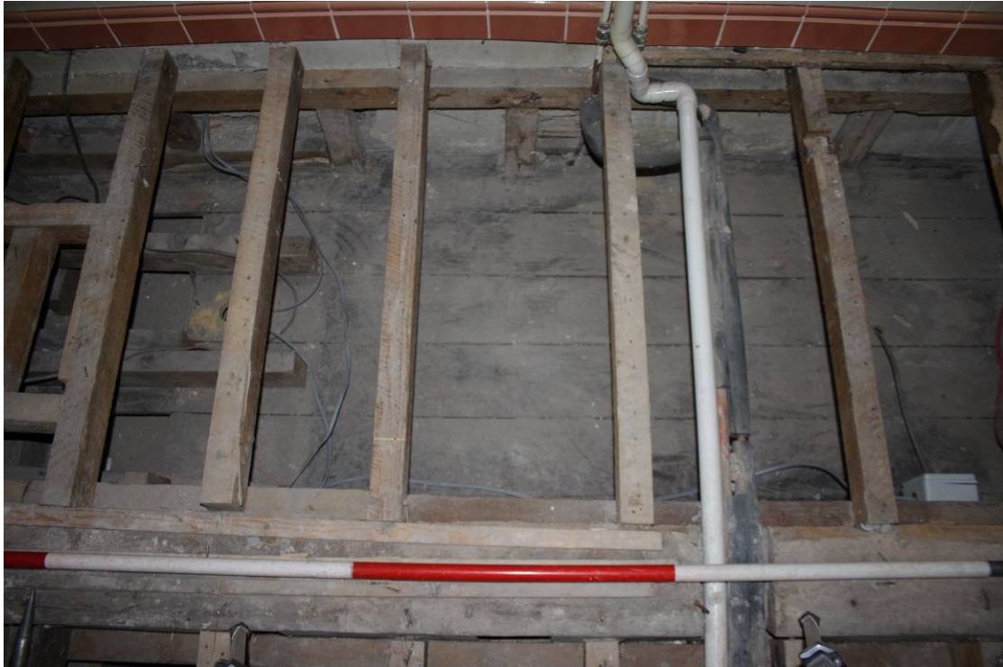
Photo 44: Bathroom 121 showing area of lower floorboards
