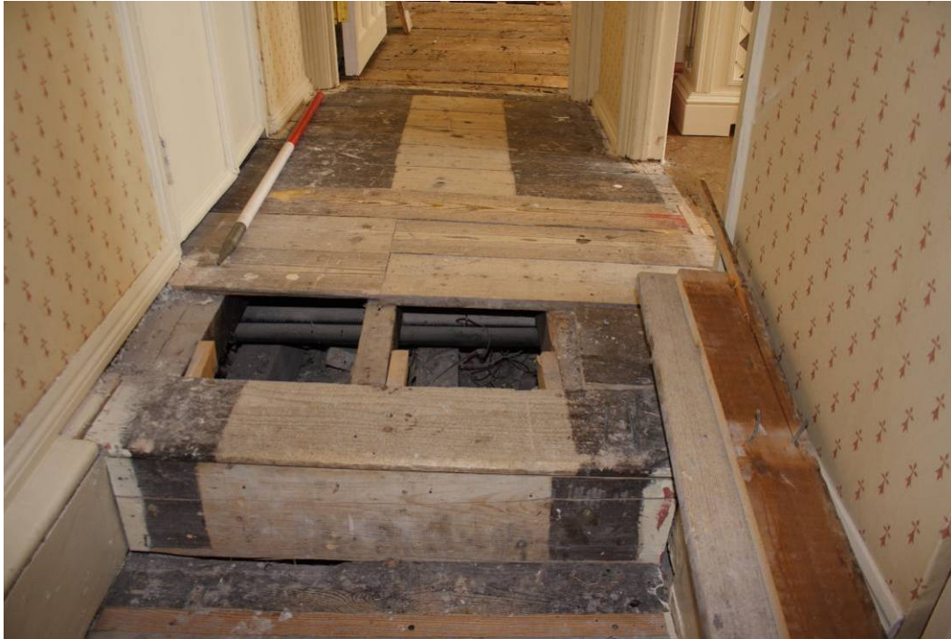
Photo 45: Corridor 119, showing start of stairs prior to floorboard removal
