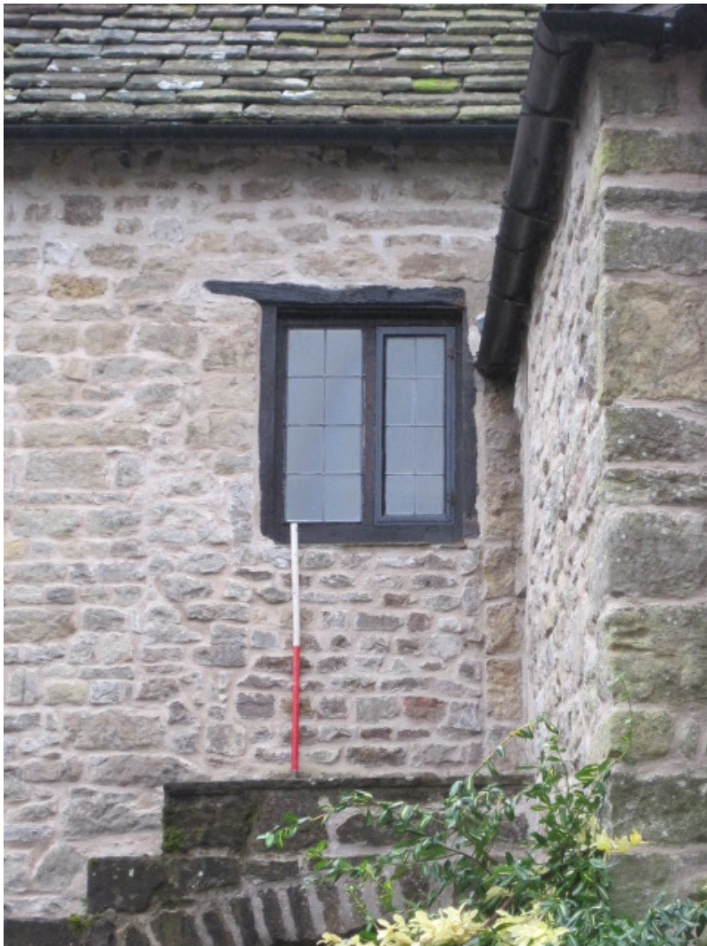
Photo 12: Detail of blocked doorway before opening
