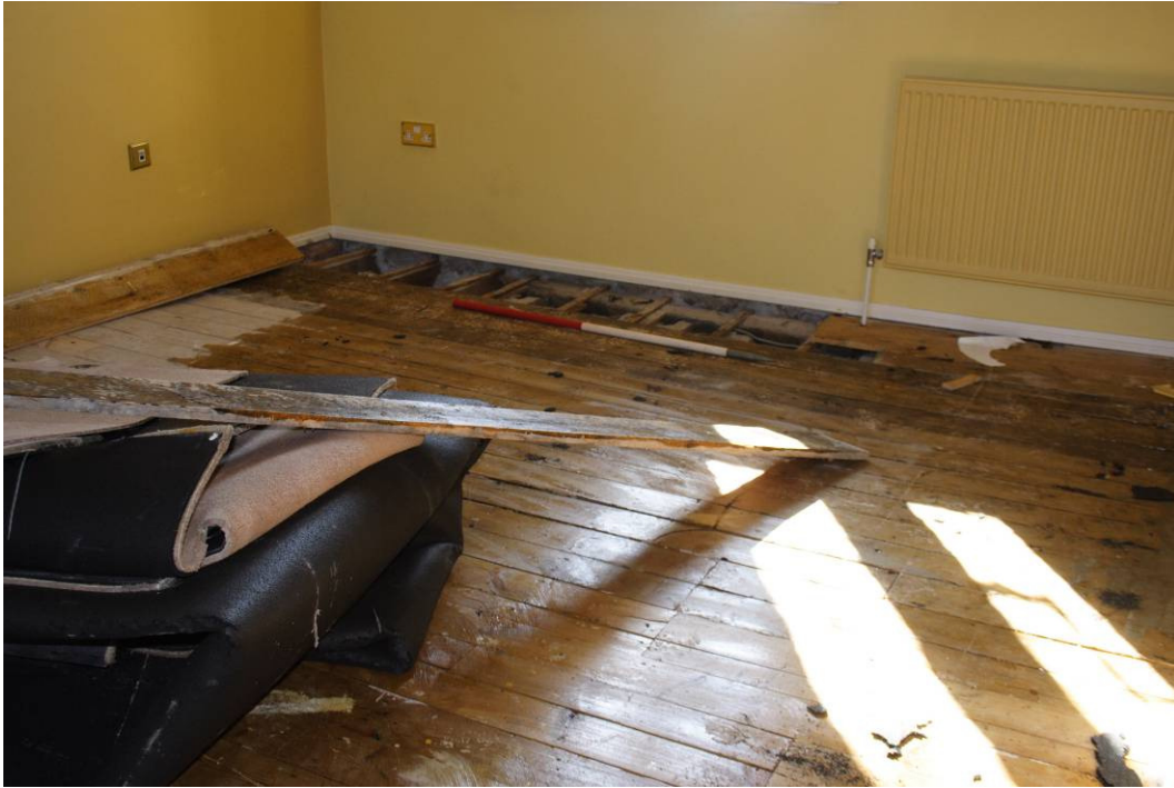
Photo 87: Bishop Morgan Bedroom 201 prior to removal of floorboards
