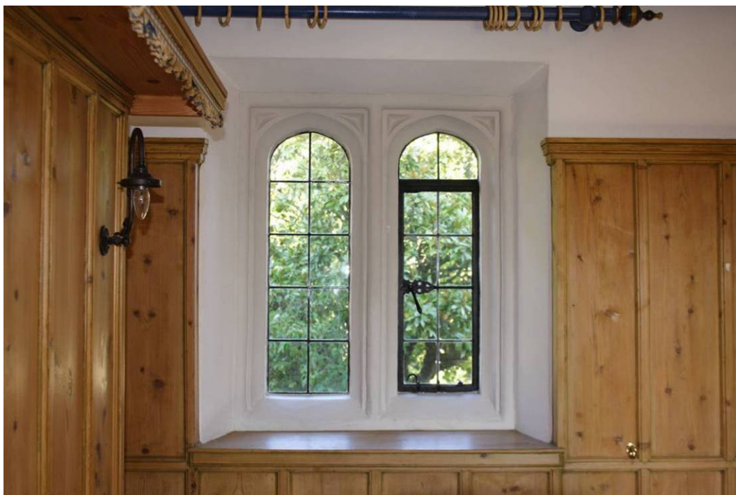
Photo 83: Window in NE wall of Bedroom 109
