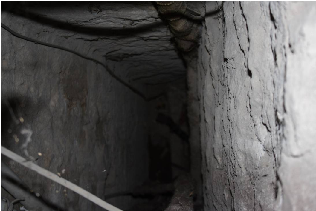
Photo 97: Probable garderobe chute within Bathroom 202 showing stone work
