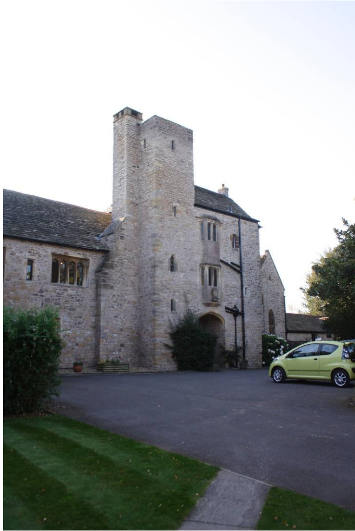
Photo 4: NE facade of the three-storey Tower from east
