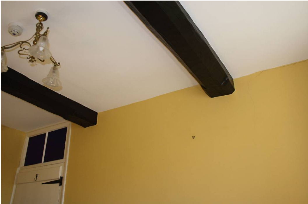
Photo 115: The two beams in the ceiling of Bedroom 201
