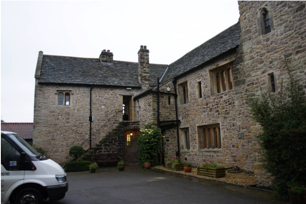
Photo 9: NE facade of SE wing (with Central Section on right hand side of photograph)
