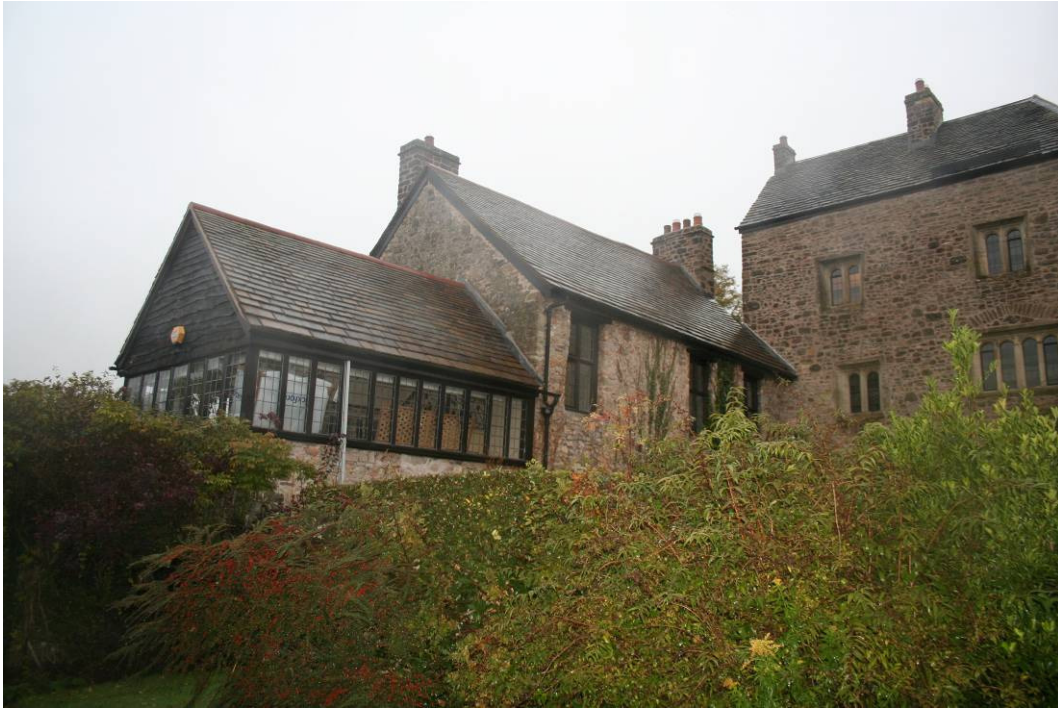
Photo 3: SW elevation of NW wing
