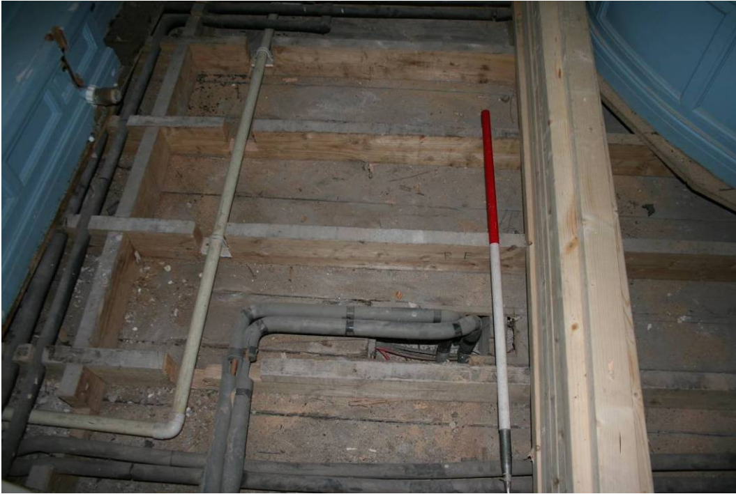
Photo 32: Bathroom 107 following removal of floorboards
