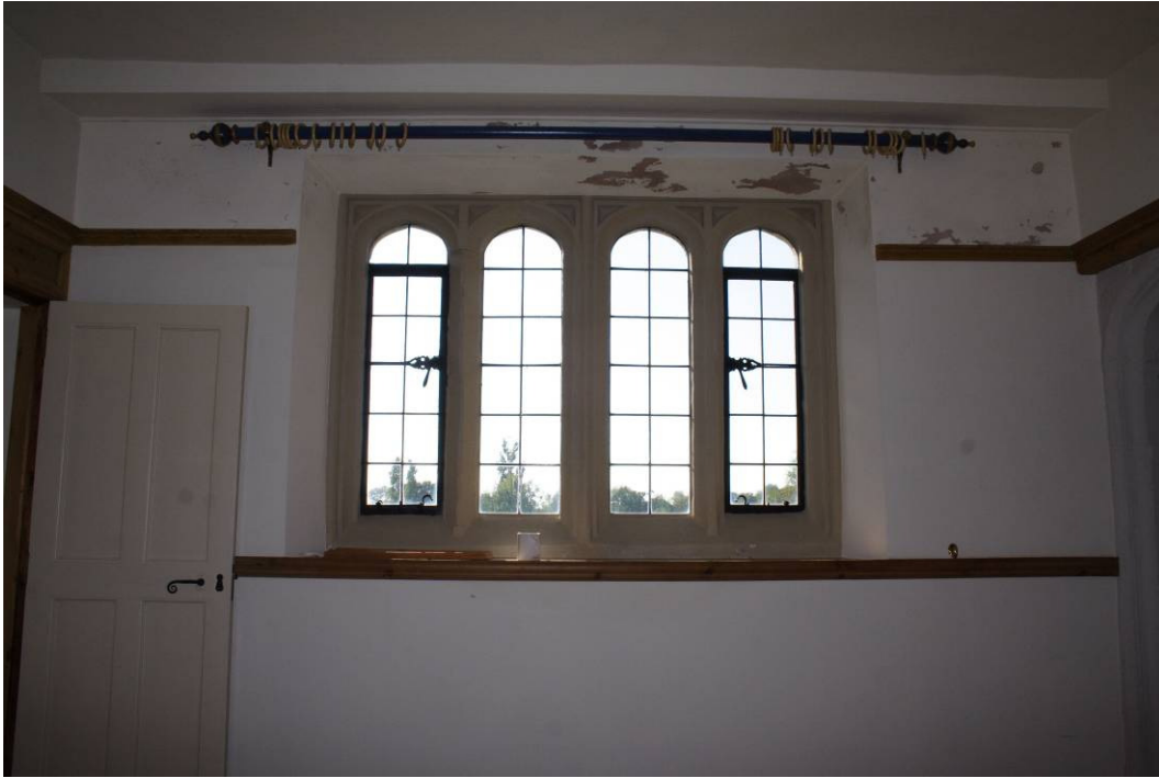
Photo 78: Stone mullioned window in SW wall of Lounge 111
