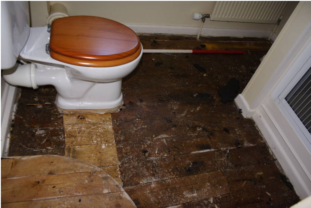
Photo 110: Bathroom 204 prior to removal of floorboards
