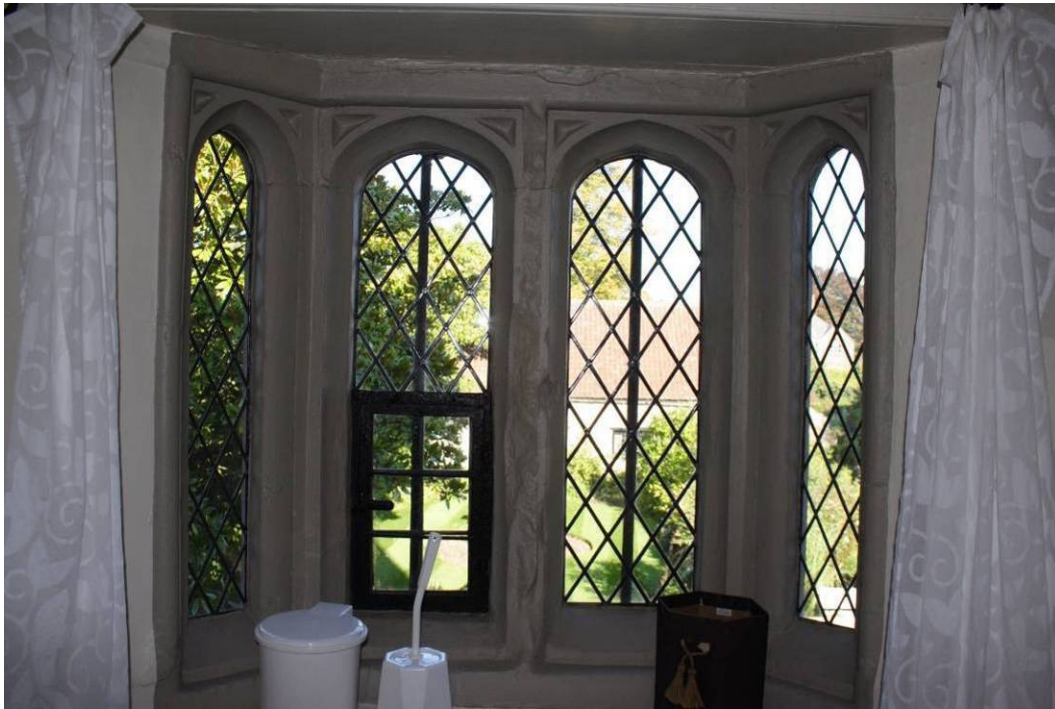
Photo 80: Stone mullioned window in NE wall of Bathroom 112
