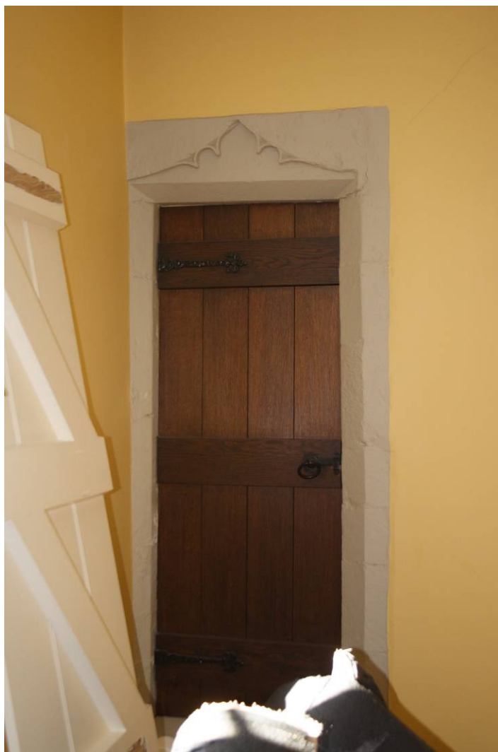
Photo 109: Stone surround doorway, now blocked, between Bedrooms 203 and 201
