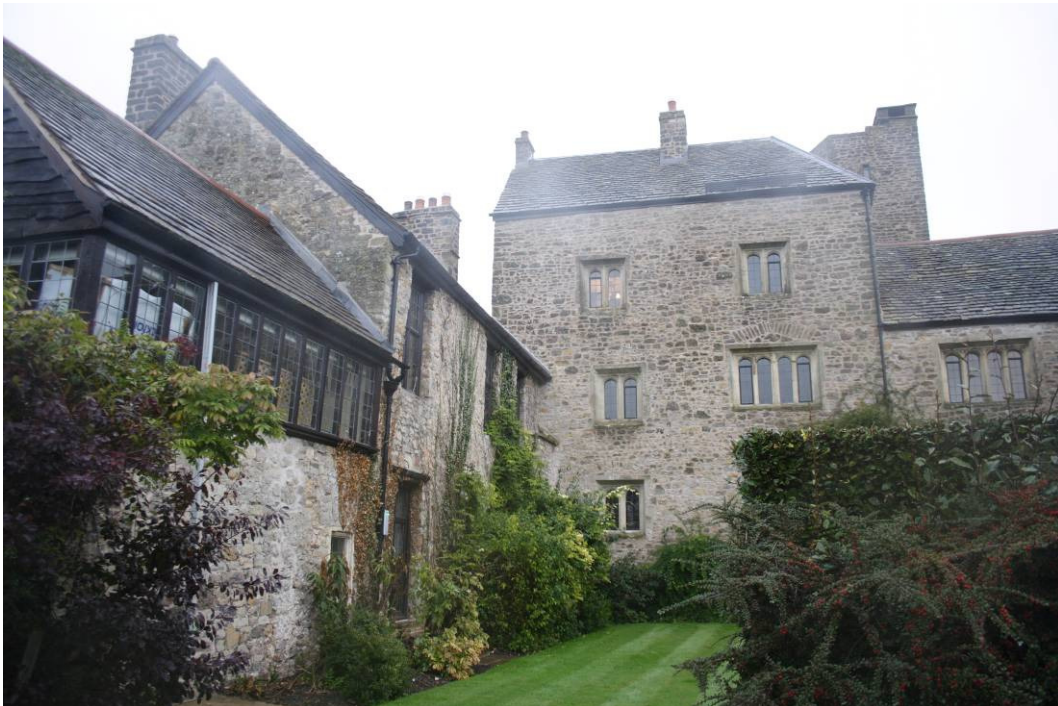
Photo 6: SW facade of three storey Tower from SW
