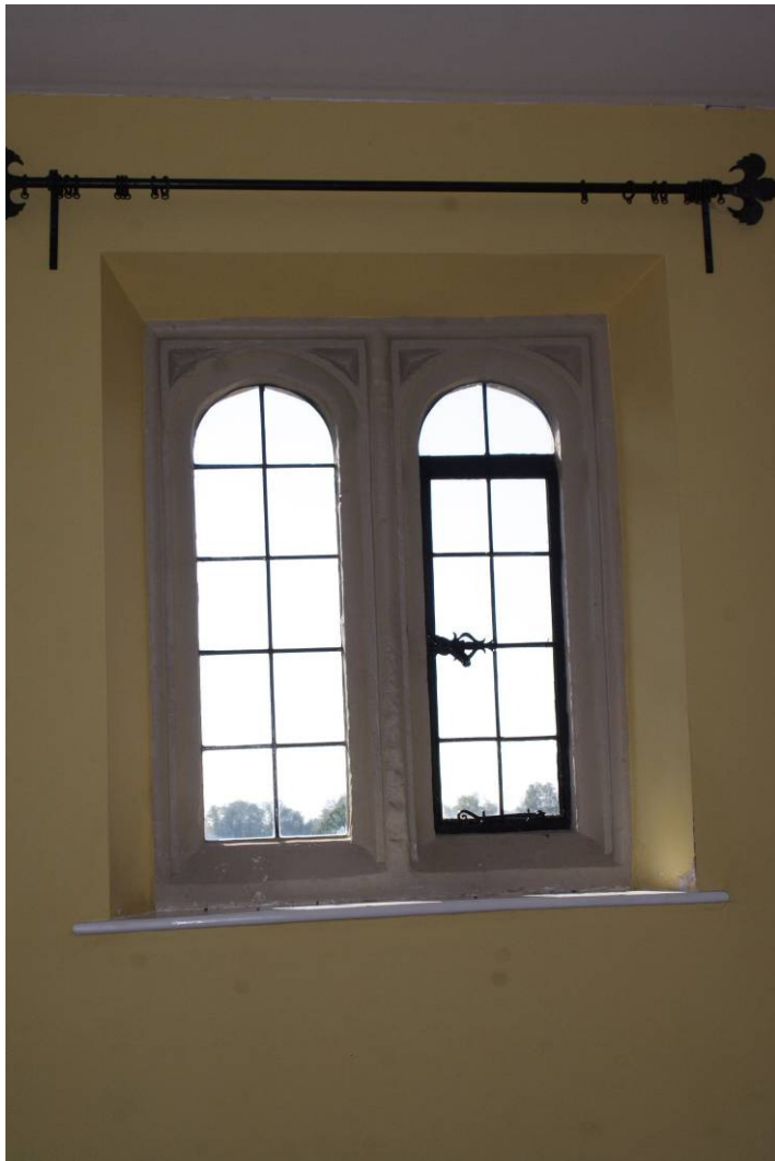
Photo 91: Window in SW wall of Bedroom 201
