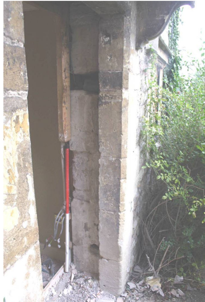
Photo 18: Right side of the internal door frame
