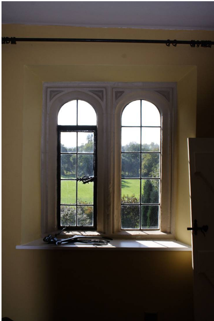
Photo 107: Window in SW wall of Bedroom 203
