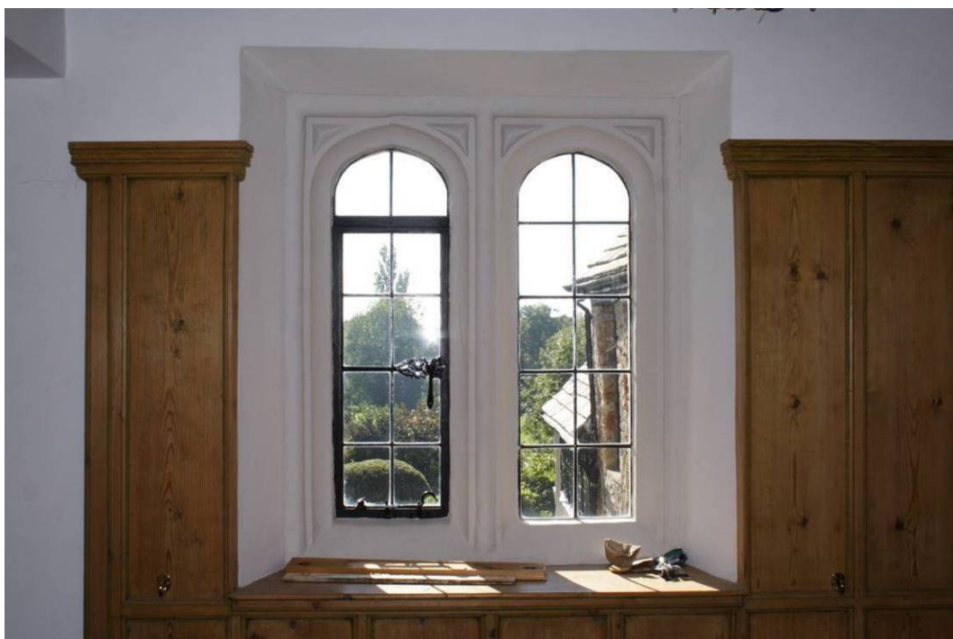
Photo 84: Window in SW wall of Bedroom 109
