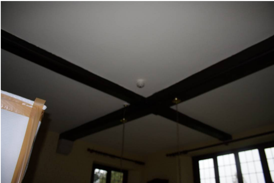
Photo 33: Ceiling of Snooker Room 006 showing exposed crossing beams
