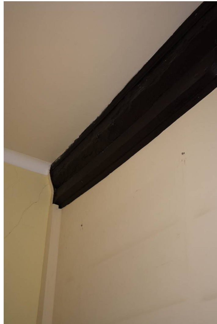
Photo 114: NE beam in ceiling of Bedroom 203, showing underlying partition wall
