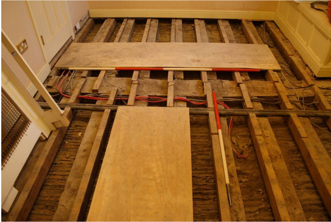
Photo 47: Bishop Miles Godwin Bedroom 116 following removal of floorboards, viewing NW
