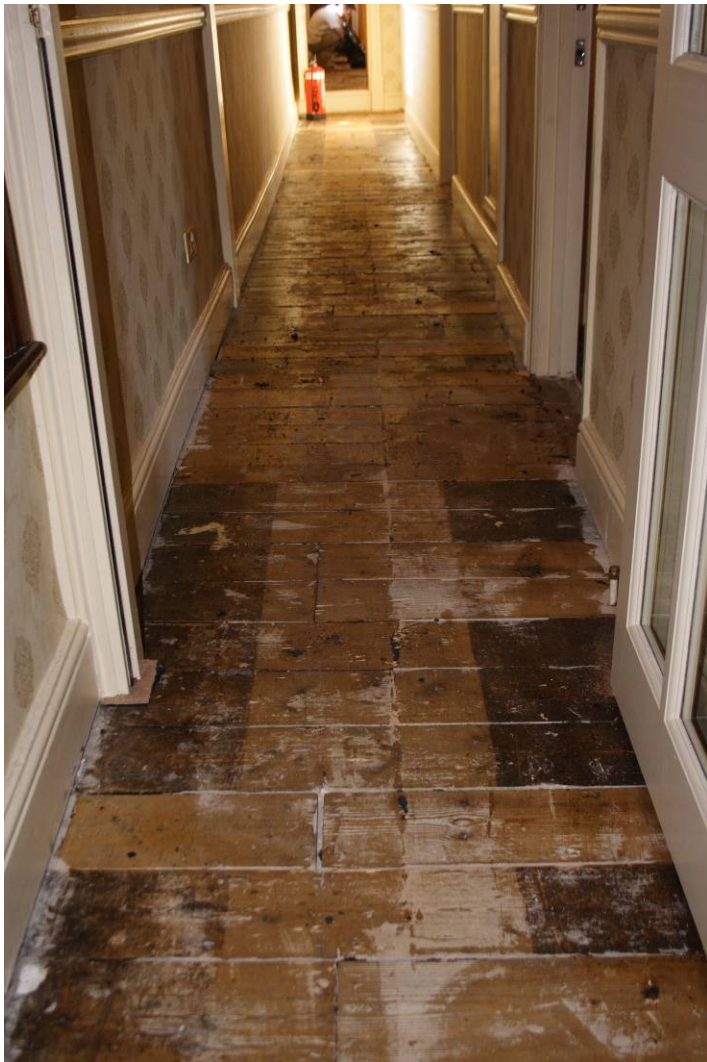
Photo 56: Corridor 113 prior to removal of floorboards, viewing NW
