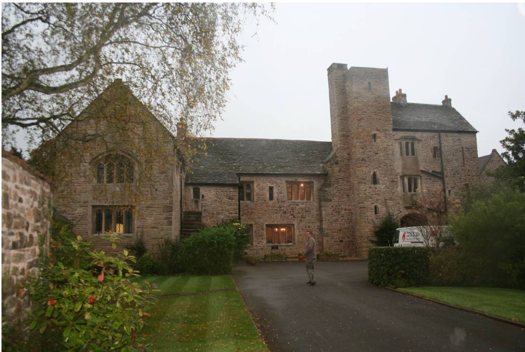
Photo 1: Main NE elevation of Mathern Palace from SE
