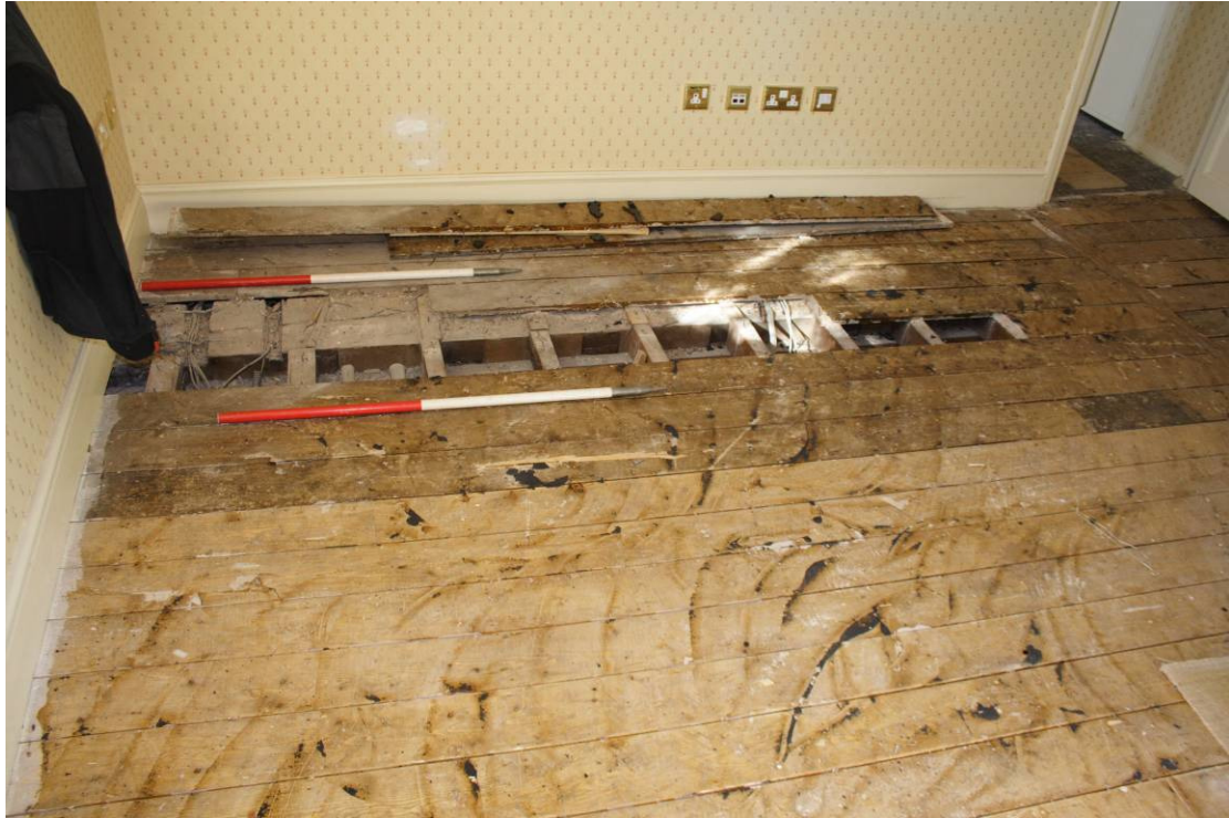
Photo 39: The Chapel Lounge 121 prior to total removal of floorboards
