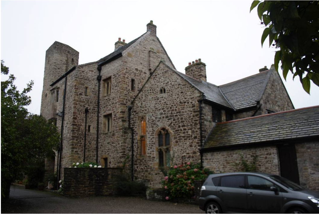
Photo 5: NE facade of the three-storey Tower from the north
