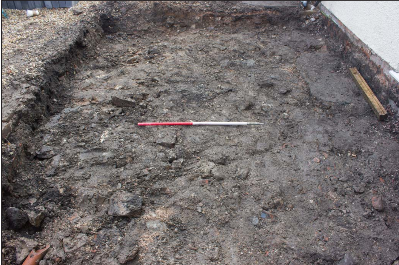
Plate 02: Post ground reduction for extension footprint to rear of Longton, Parliament Street, Rhuddlan, Denbighshire - from the southeast - 1.00m scale
