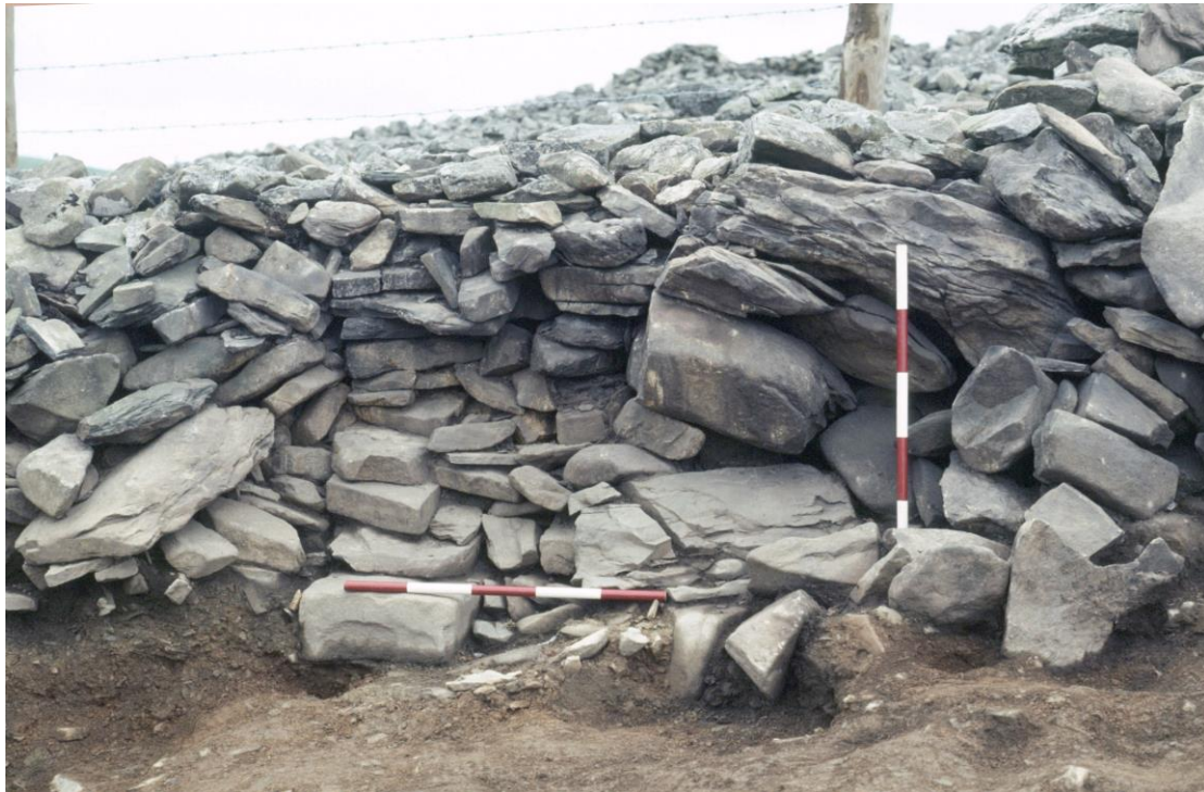
FIGURE 2.13: Relationship of coursed slab wall [13] to original boulder face [34] as evidenced in south section
