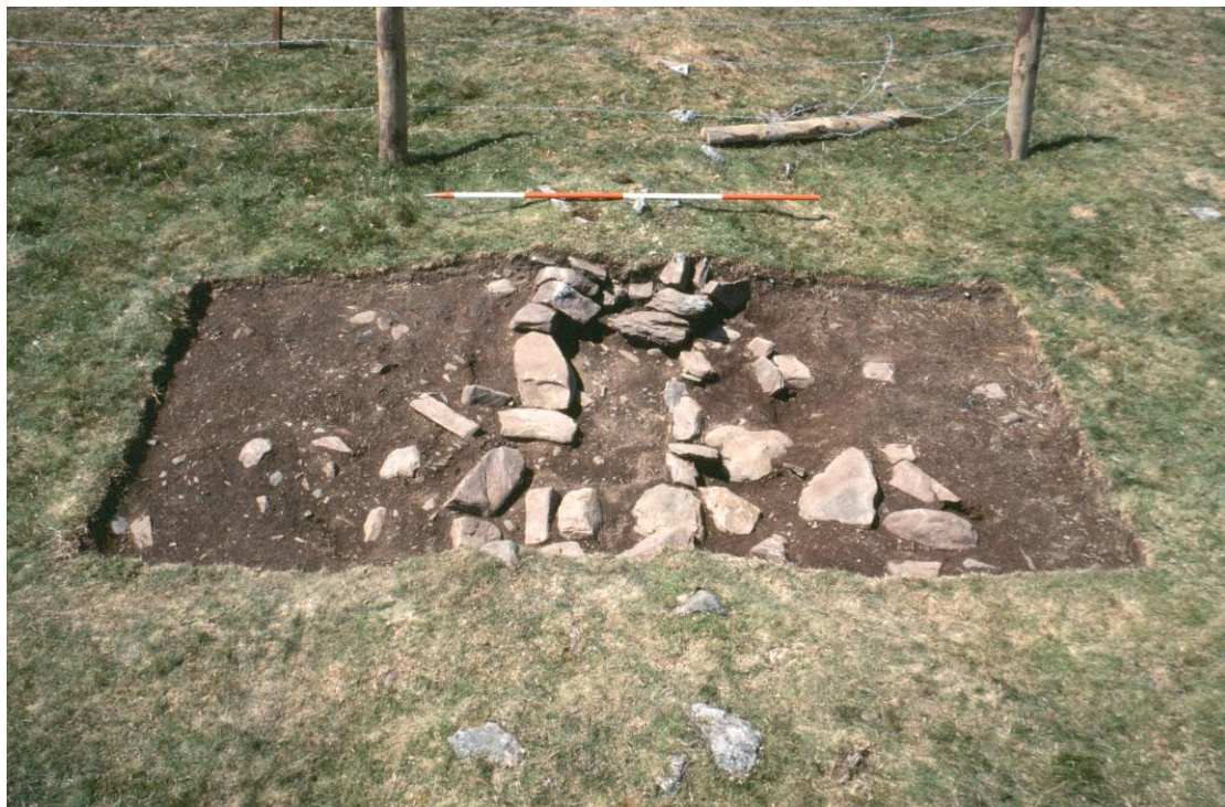
FIGURE 4.2: Detail of drystone wall faces [105 and 106]
