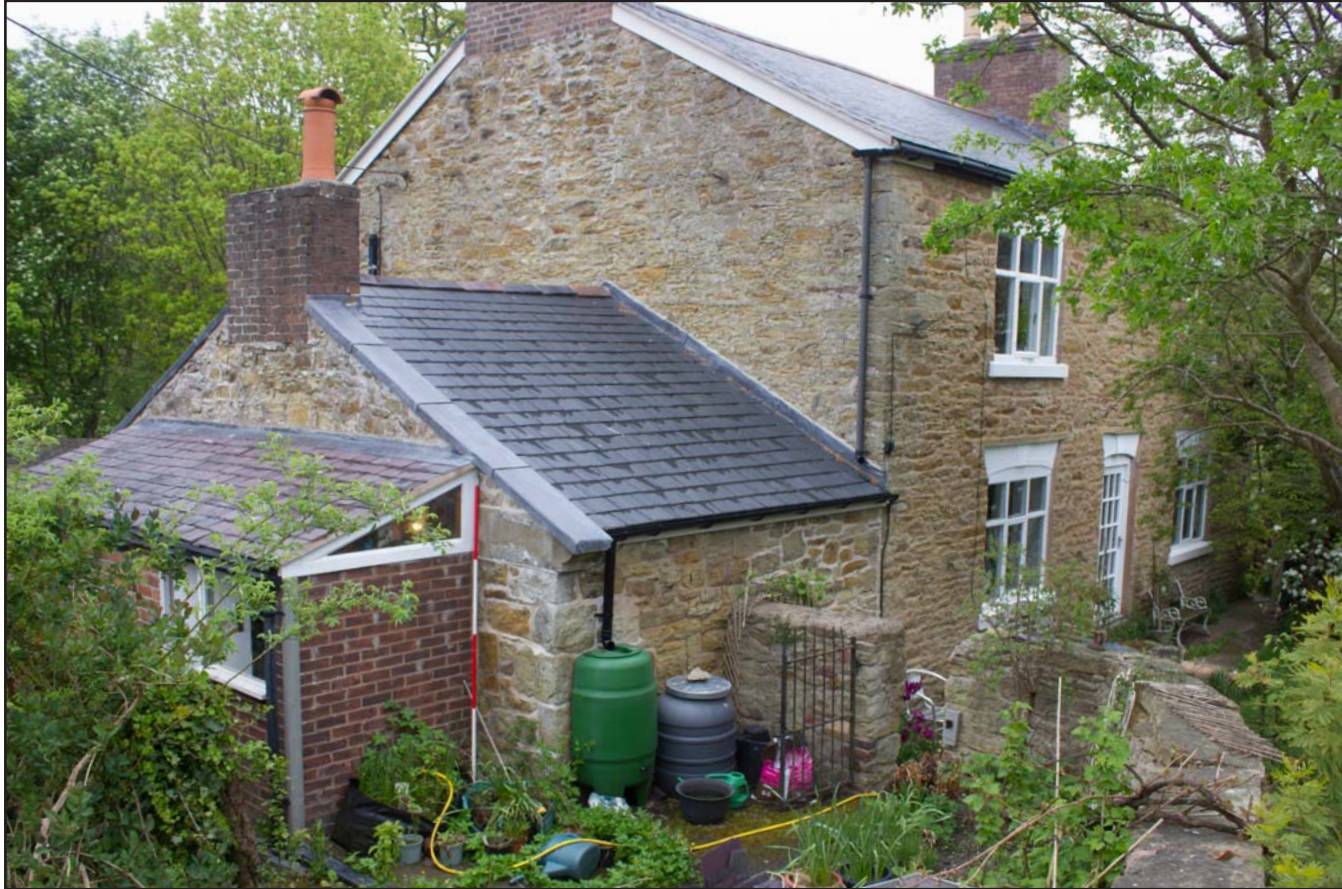
Plate 07: Oblique shot of northwest & southwest elevations of Ty Carreg, Northop, Mold, Flintshire - from the southwest - 2.00m scale
