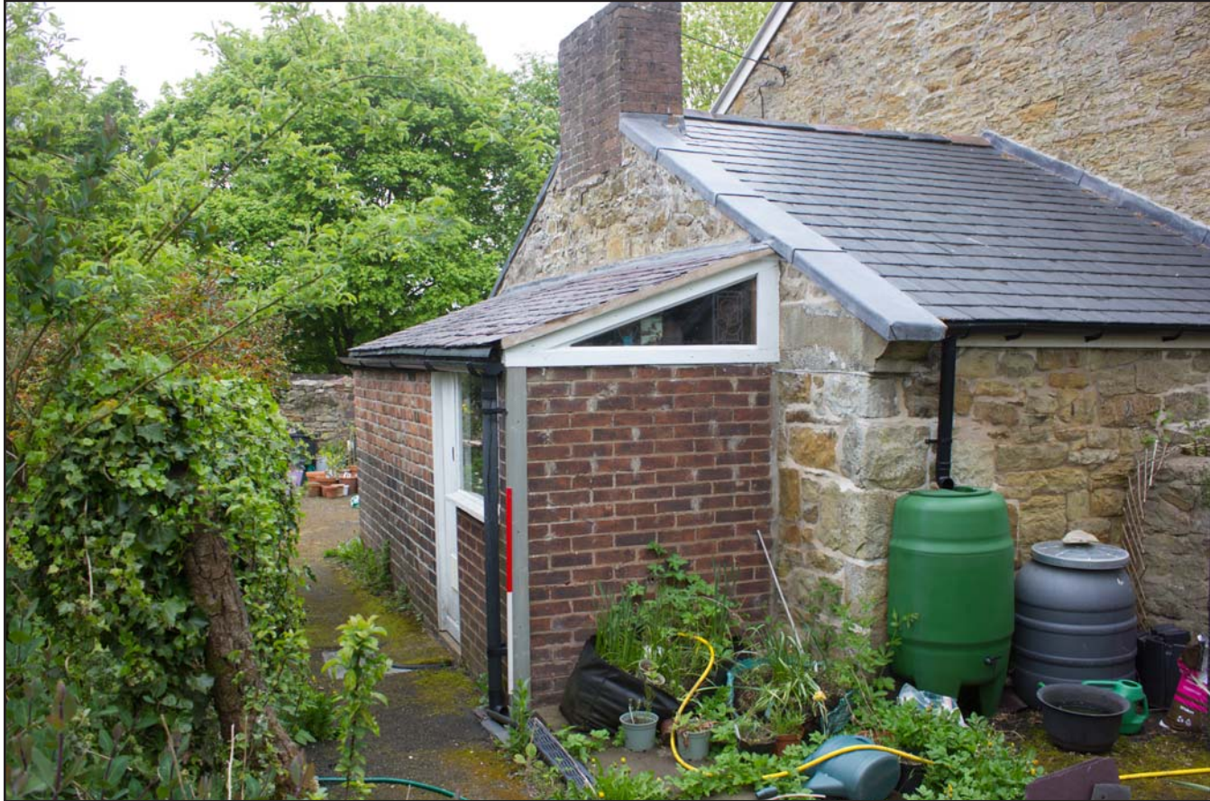
Plate 21: External shot of brick out building at Ty Carreg, Northop, Mold, Flintshire - from the southwest - 1.00m scale
