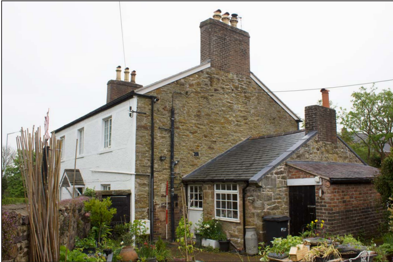
Plate 10: Oblique shot of northwest elevation of Ty Carreg, Northop, Mold, Flintshire - from the northwest - 2.00m scale
