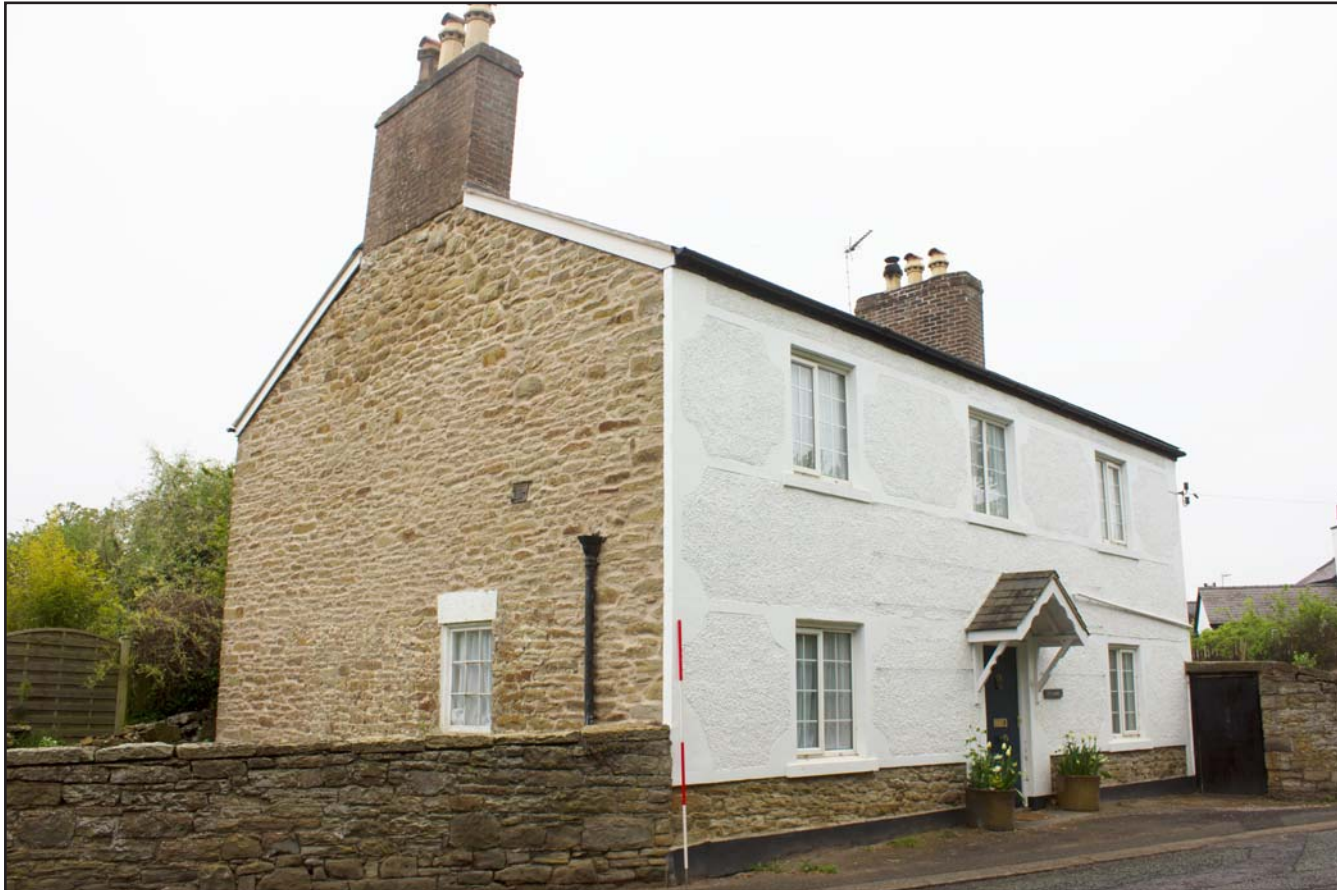
Plate 02: Oblique shot of northeast & southeast elevations of Ty Carreg, Northop, Mold, Flintshire - from the northeast - 2.00m scale
