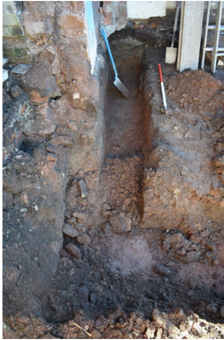
Figure 6 The trench at the northern part. Viewed from the west. CPAT photo 4961-0007
