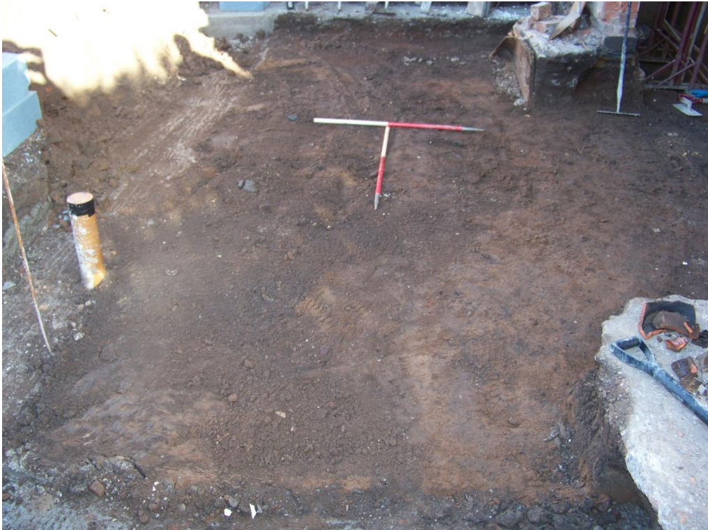
Figure 9 Completed excavation. Viewed from the south. CPAT photo 4961-0016
