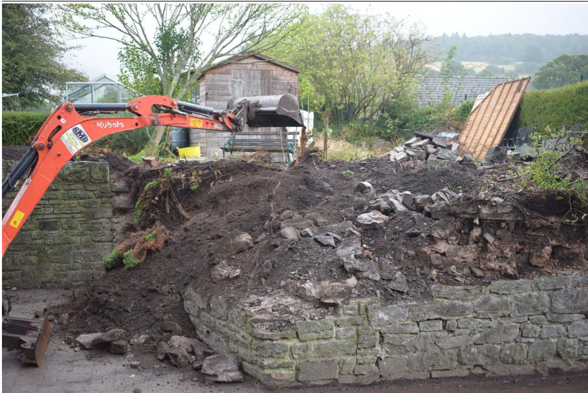
Fig. 5 Mechanical excavation of the soil. CPAT photo 4945-0004
