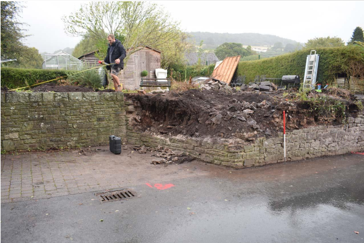
Fig. 4 The original height of the garden soil, visible upon removal of wall. Viewed from the southwest. Edited, CPAT photo 4945-0002
