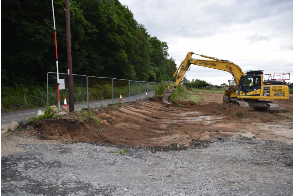
Fig. 4 Removal of roadside hedgerow, working shot. Photo CPAT 4934-0006
