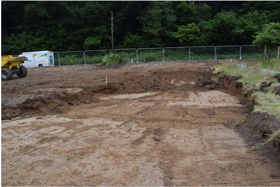
Fig. 4 Glacial till present in car park area, looking west. Photo CPAT 4934-0006
