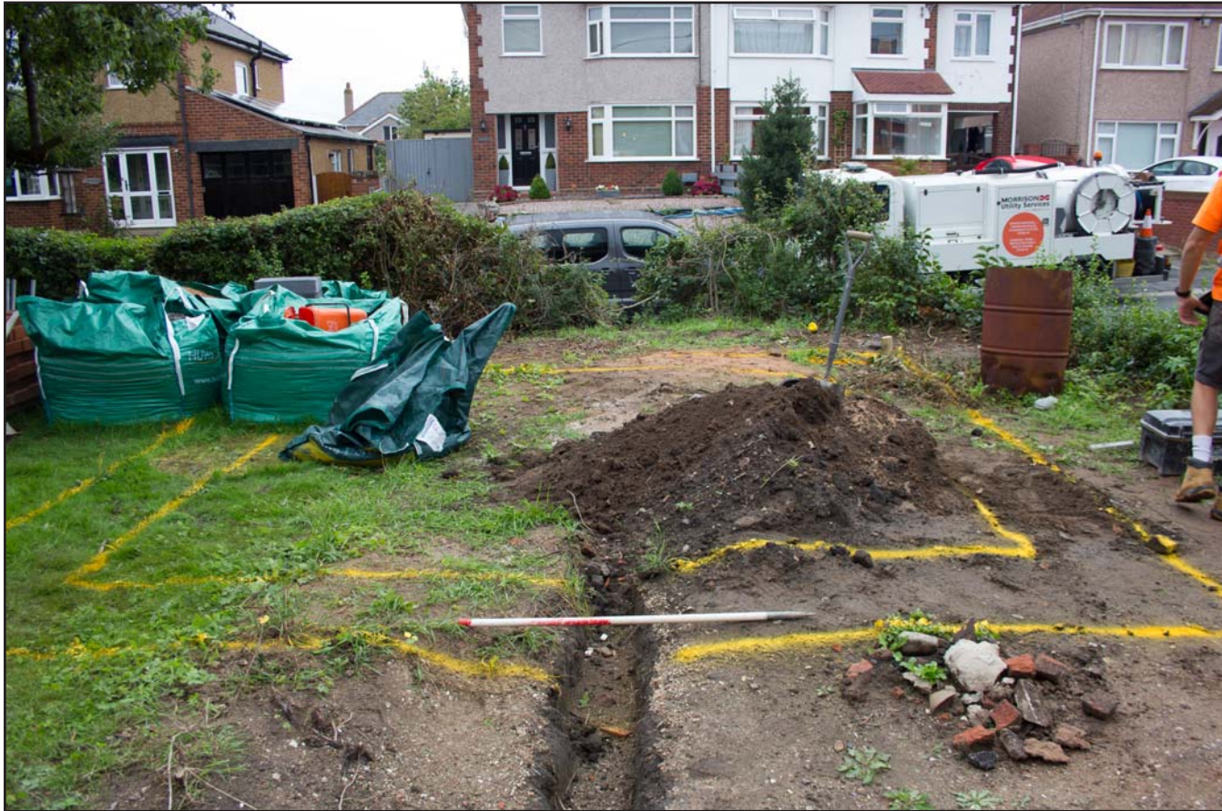
Plate 06: Pre excavation shot of store area at Plas Llewelyn, Hylas Lane, Rhuddlan, Denbighshire - from the west - scale 1m
