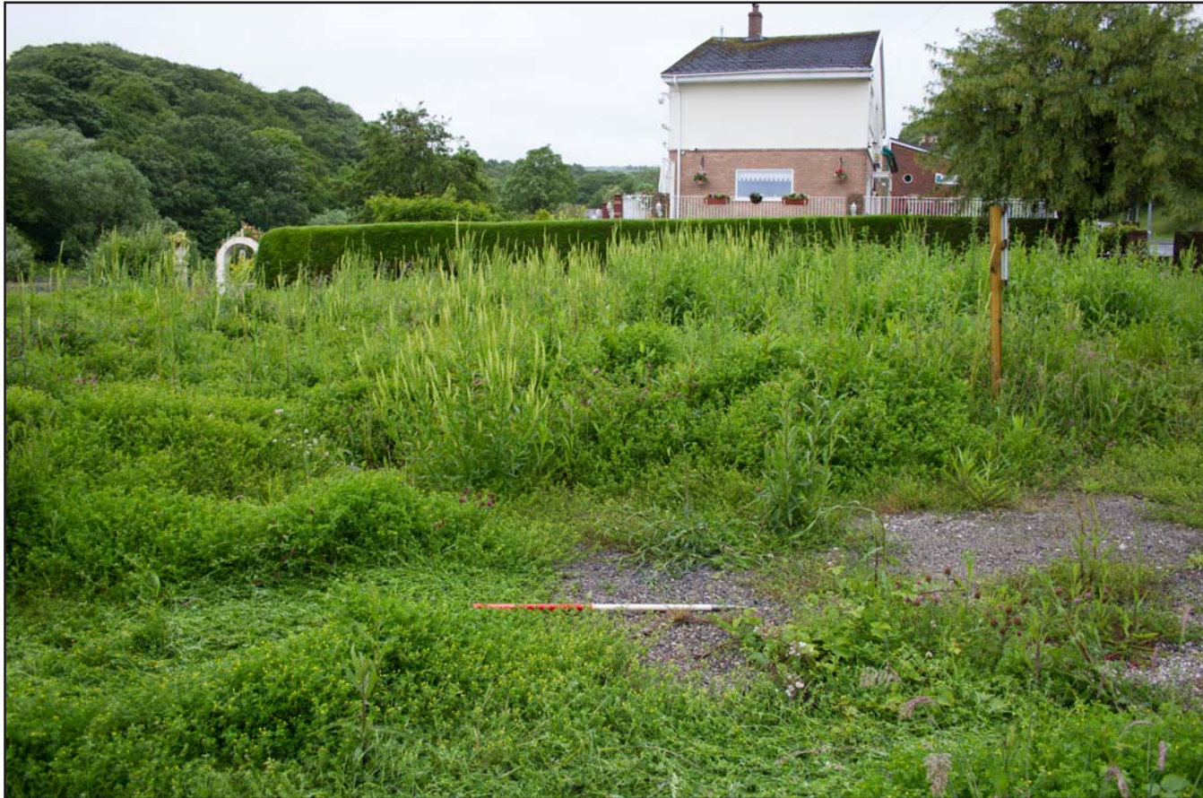
Plate 01: Pre excavation shot of land adjacent to Italia Residence, Greenfield - from the north - scale 1m
