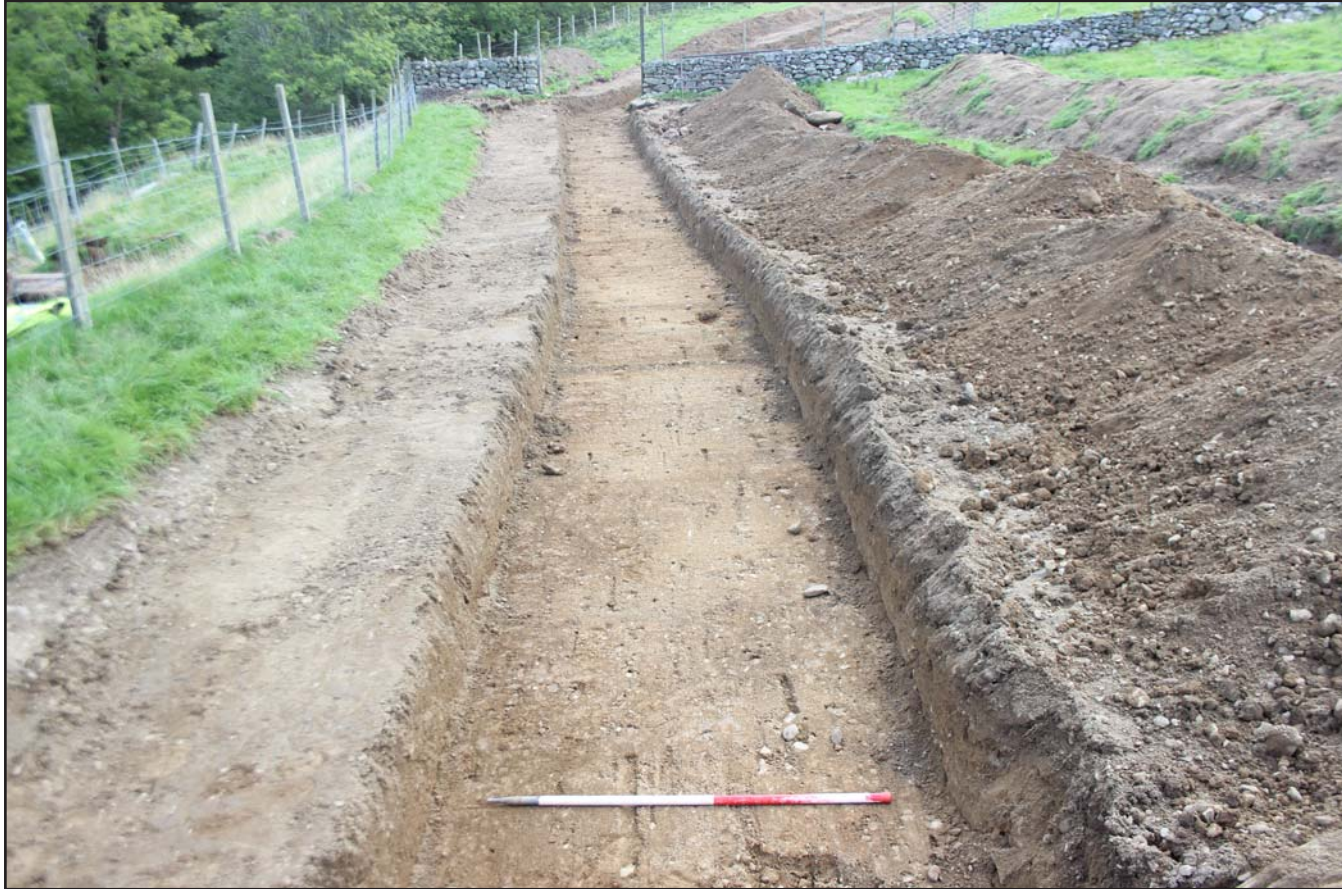
Plate 11: Pipe trench in Field C - from the west- scale 1m
