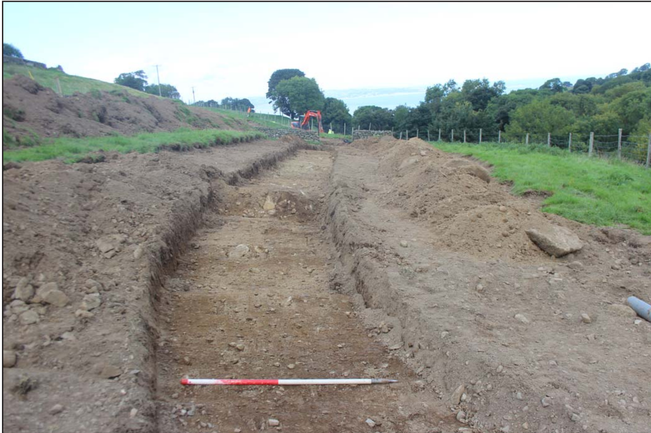
Plate 10: Pipe trench in Field B - from the southeast - scale 1m
