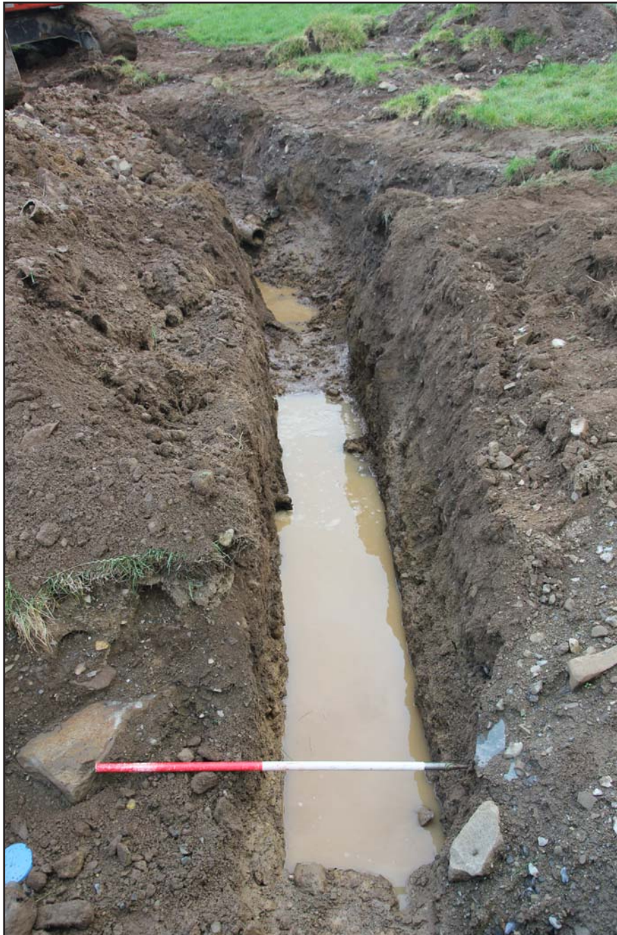
Plate 68: Launch pit 3 - from the west - scale 1m
