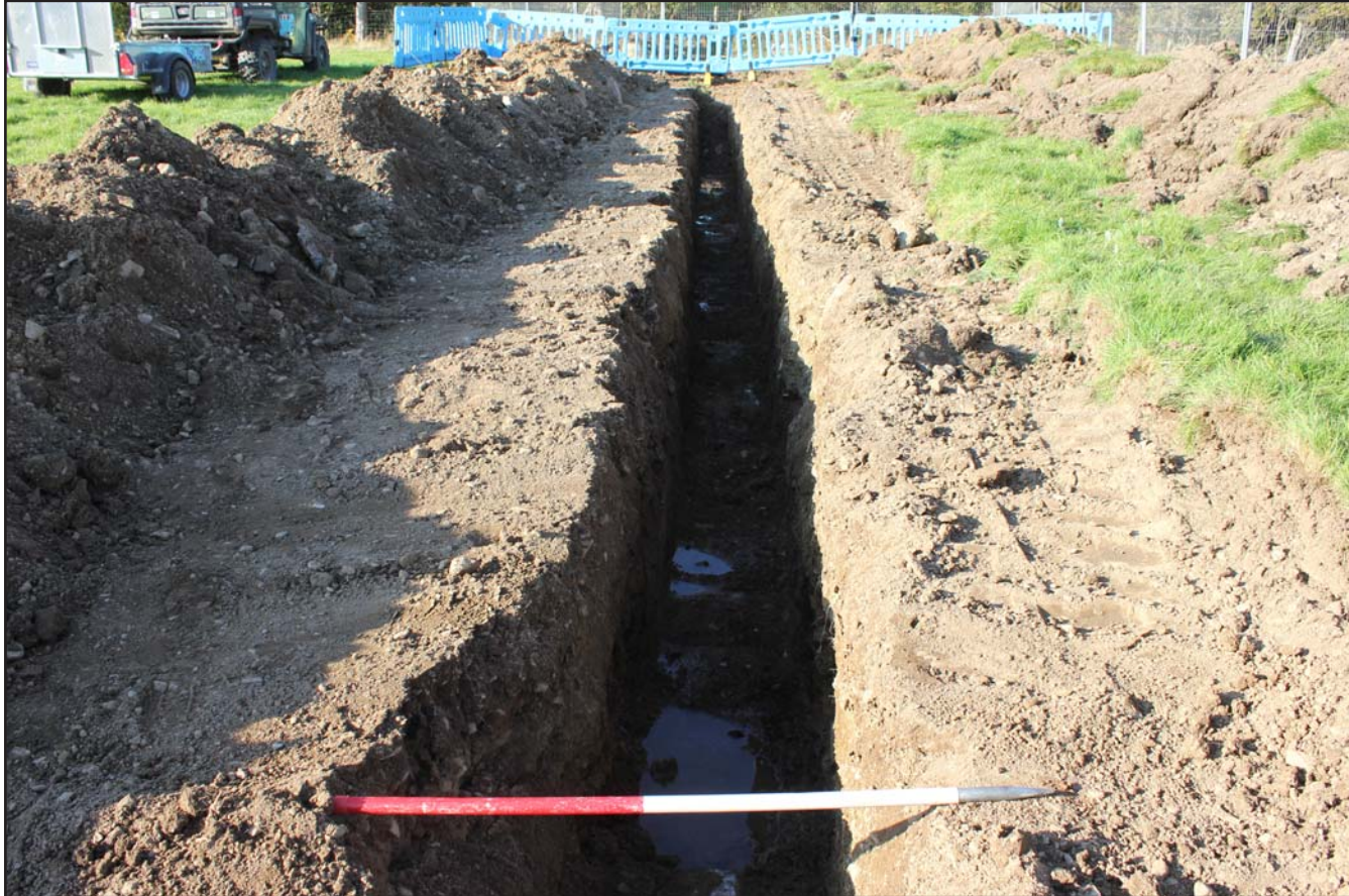
Plate 76: Pipe trench within Field K - from the southeast - 1m scale
