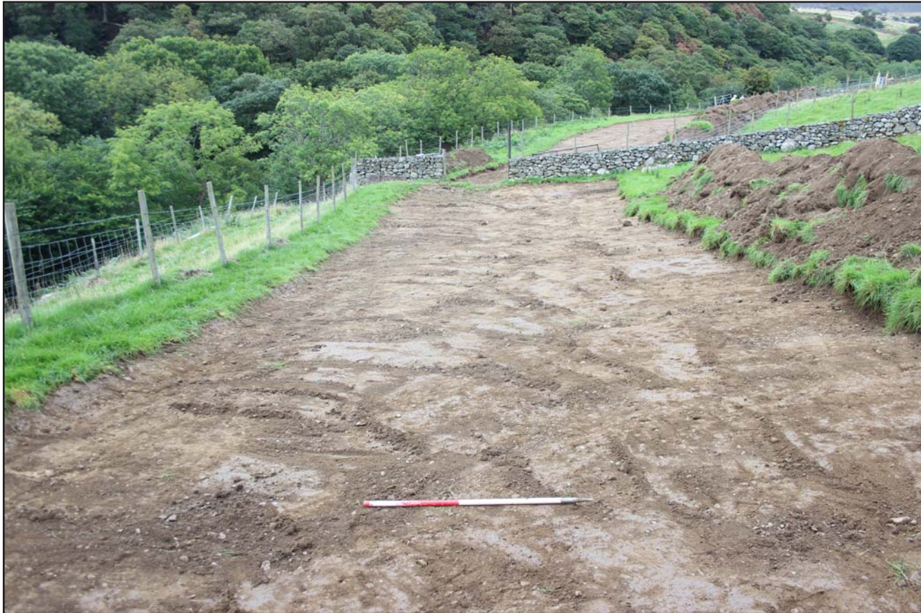
Plate 06: Topsoil strip within Field C - from the west - scale 1m
