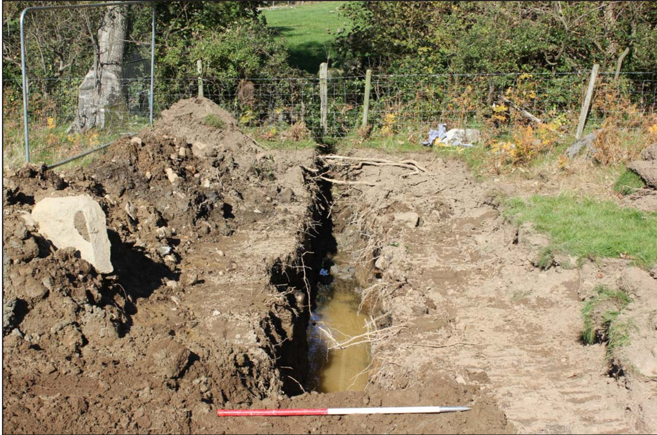
Plate 77: Pipe trench within Field K - from the north - 1m scale
