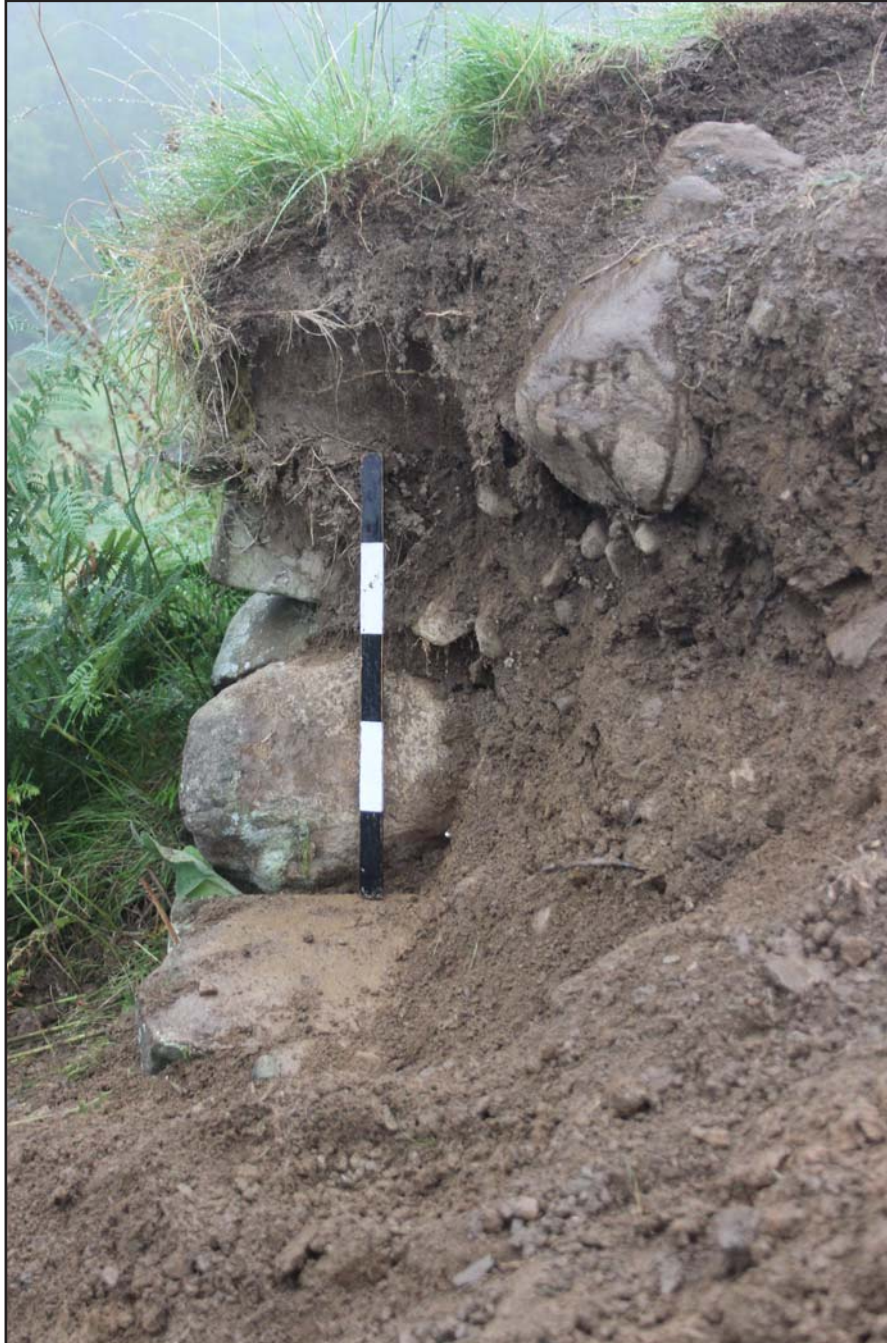
Plate 14: Section of trackway showing retaining wall for track (Field D) - from the west - scale 0.5m
