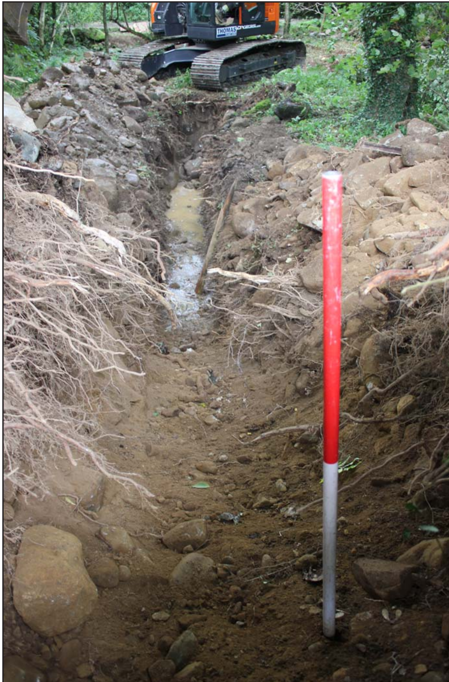
Plate 23: Pipe trench within river basin - from the north - scale 1m
