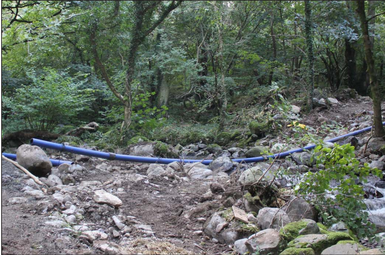
Plate 25: Pipe crossing Afon Llanfairfechan - from the northwest - scale n/a
