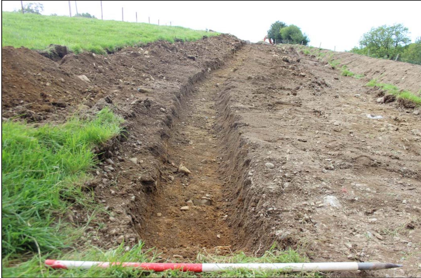
Plate 08: Pipe trench in Field A - from the southeast - scale 1m
