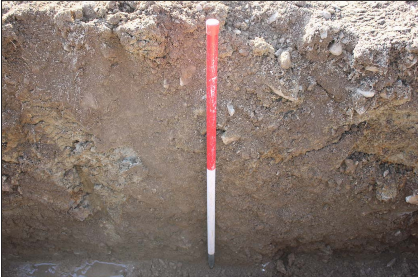
Plate 78: Section of pipe trench within Field K - from the southeast - 1m scale
