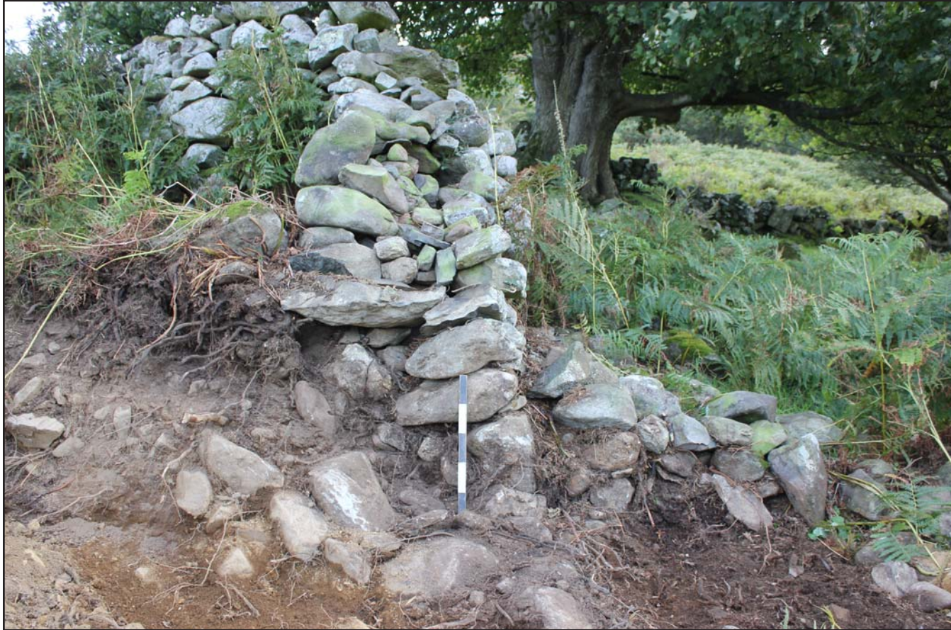
Plate 51: Section of breached wall (between Fields F & G) - from the west - scale 0.5m
