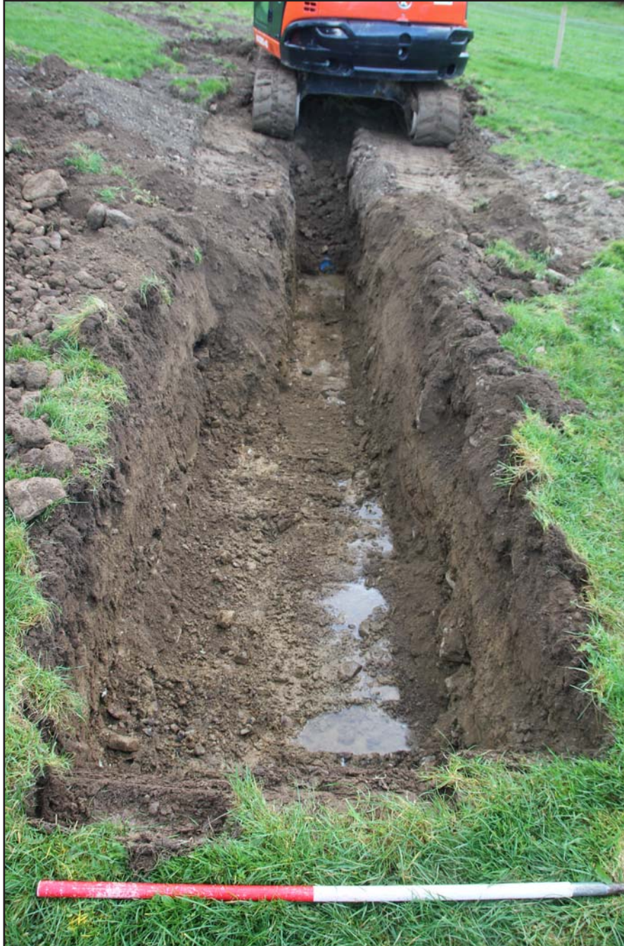
Plate 70: Reception pit 4 - from the northeast - scale 1m
