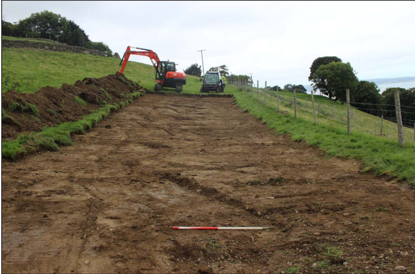
Plate 07: Topsoil strip within Field C - from the east - scale 1m
