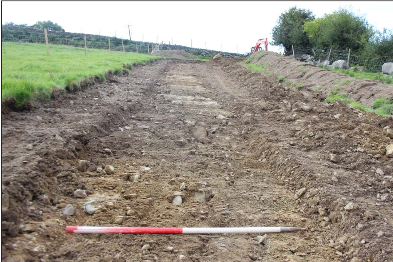
Plate 09: Pipe trench in Field A - from the southeast - scale 1m
