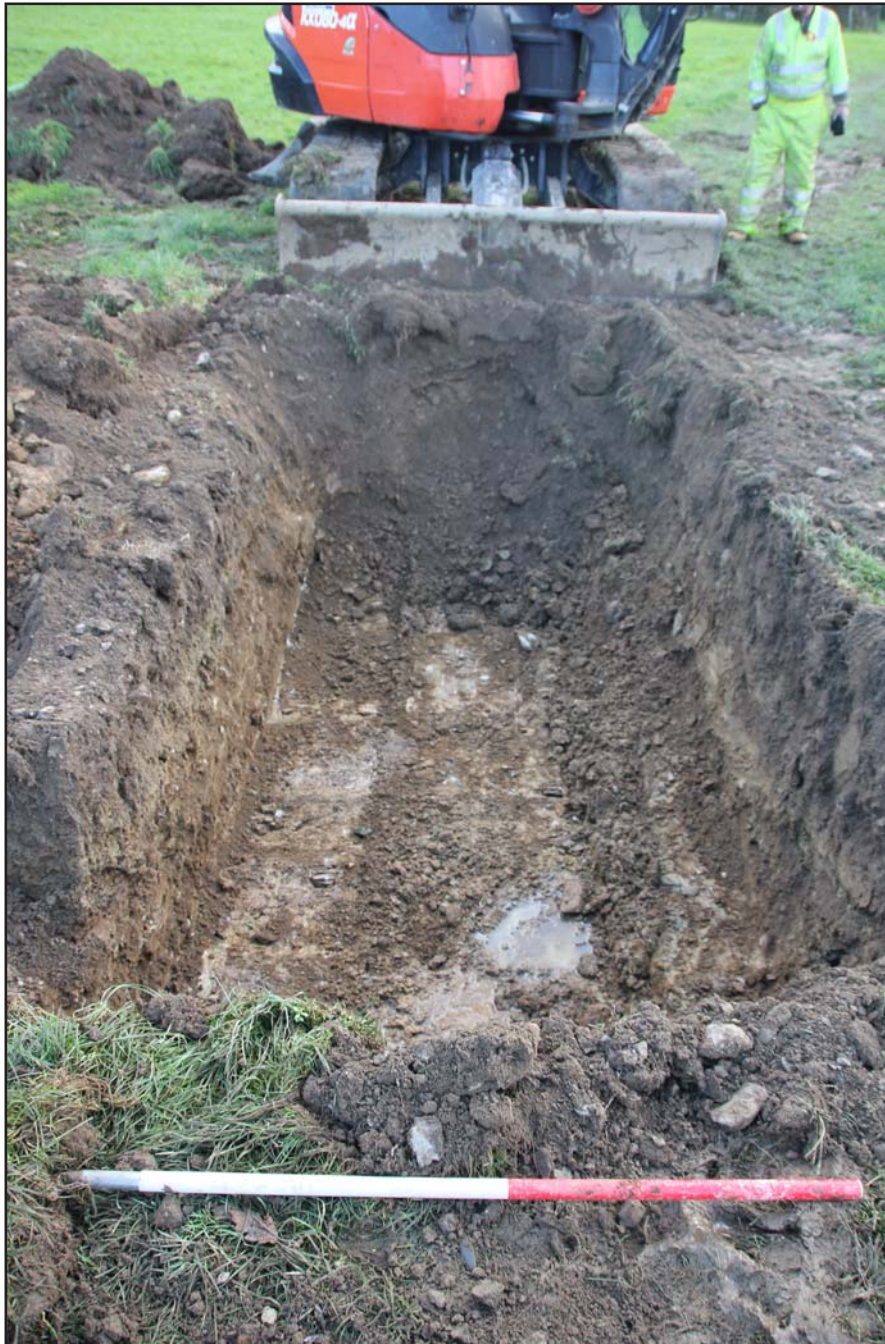
Plate 72: Launch pit 5 - from the east - 1m
