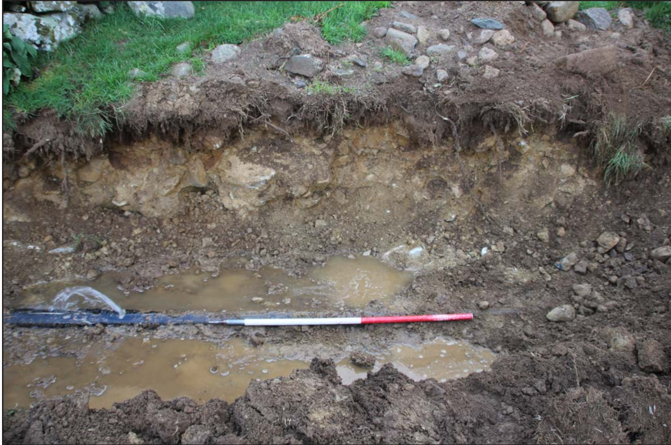
Plate 64: Launch pit 1 - from the west - scale 1m
