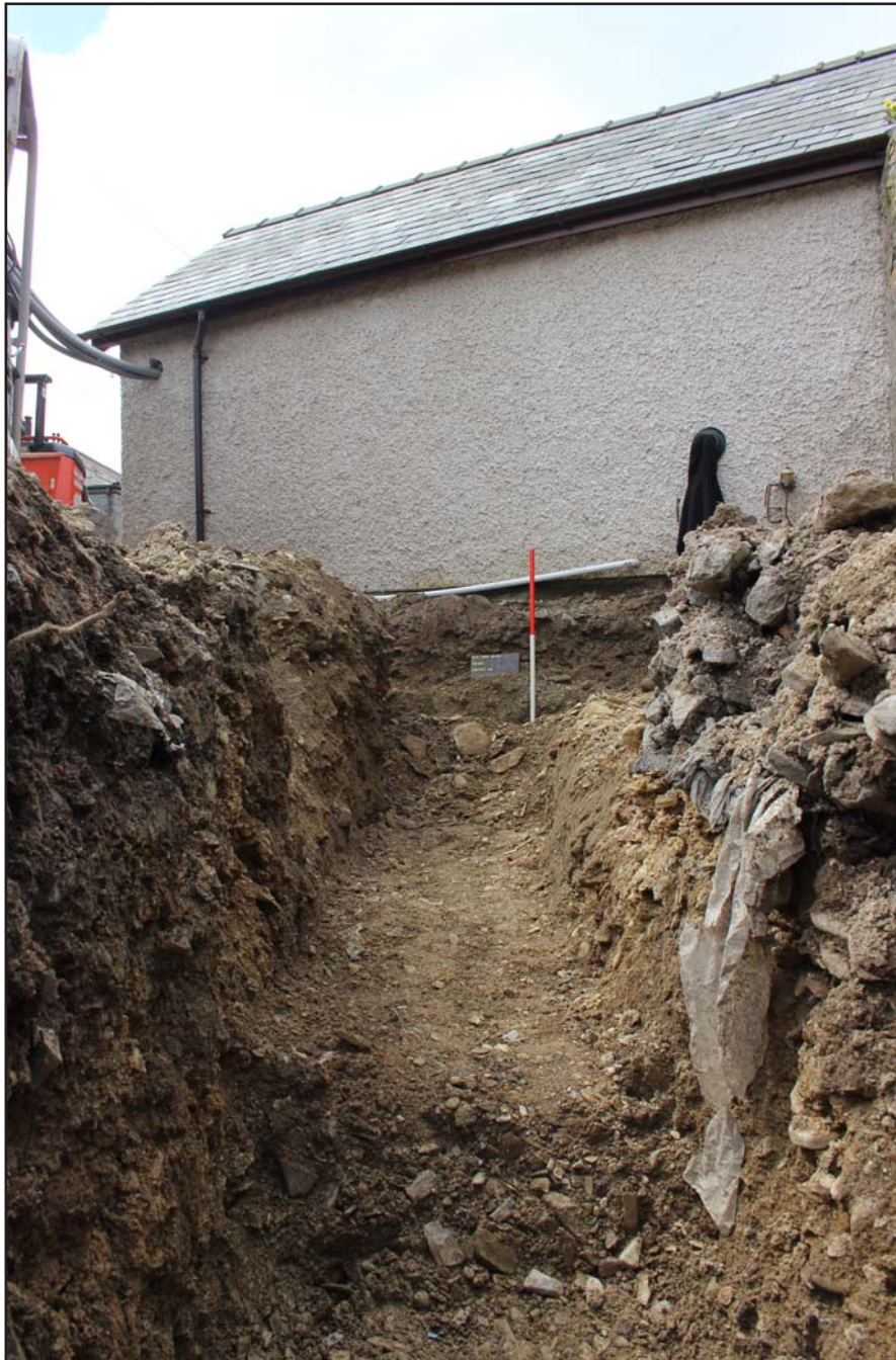
Plate 05: Western trench footing (aligned northeast - southwest) - from the northeast - scale 1.00m
