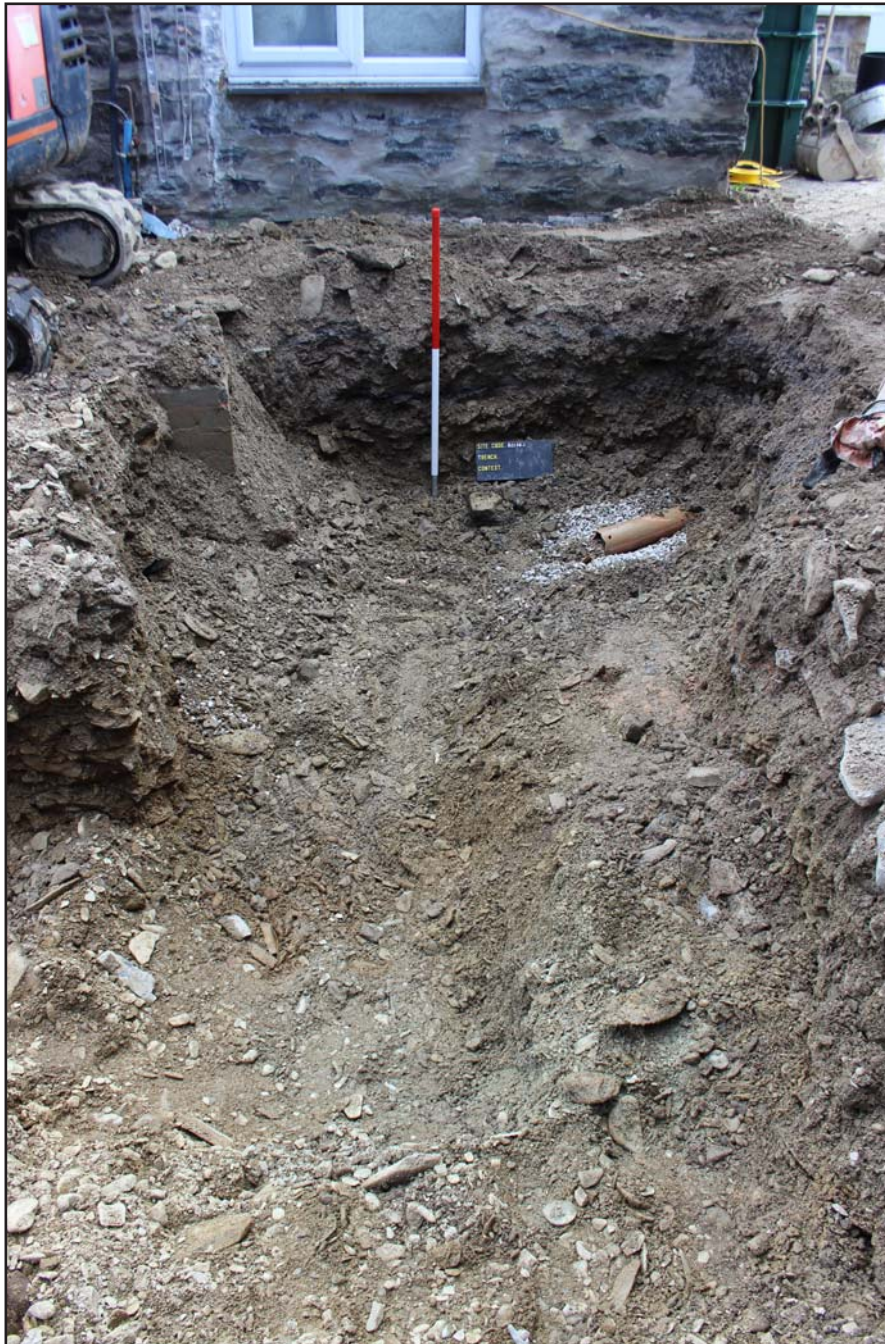
Plate 07: Southern trench footing (aligned northwest - southeast) - from the northwest - scale 1.00m
