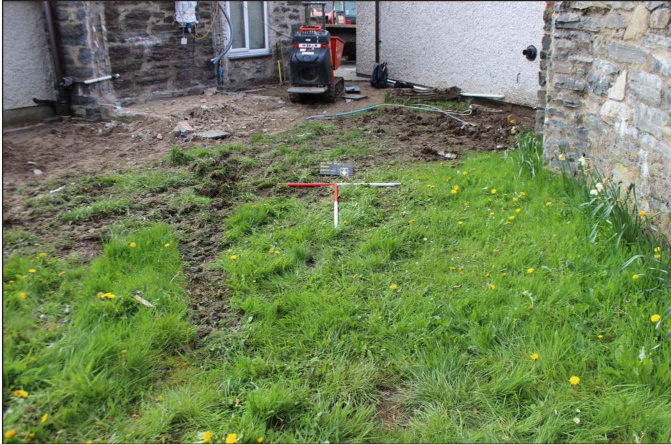
Plate 02: Pre excavation shot - from north - scale 2 x 1.00m
