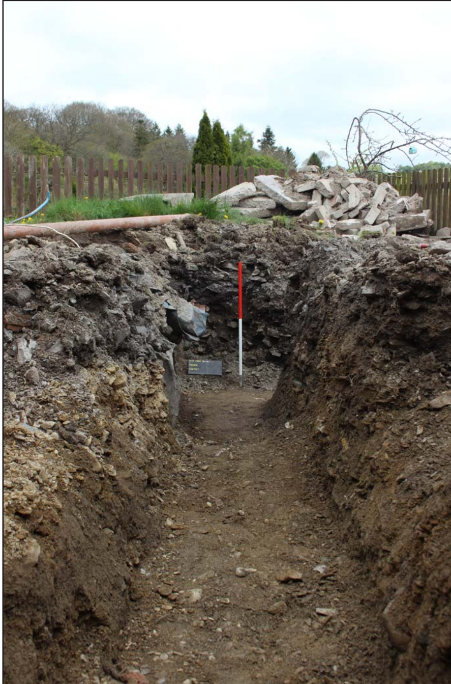
Plate 06: Western trench footing (aligned northeast - southwest) - from the southwest - scale 1.00m
