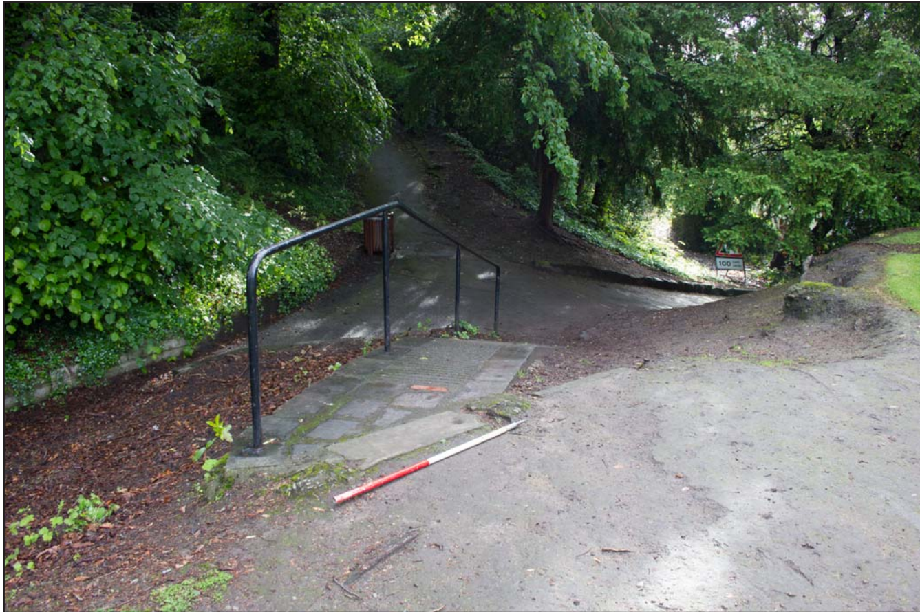
Plate 30: Pre excavation shot of evaluation area containing concrete ramp previously providing access to Outer Bailey ward, Bailey Hill, Mold, Flintshire - from the east - scale 1m
