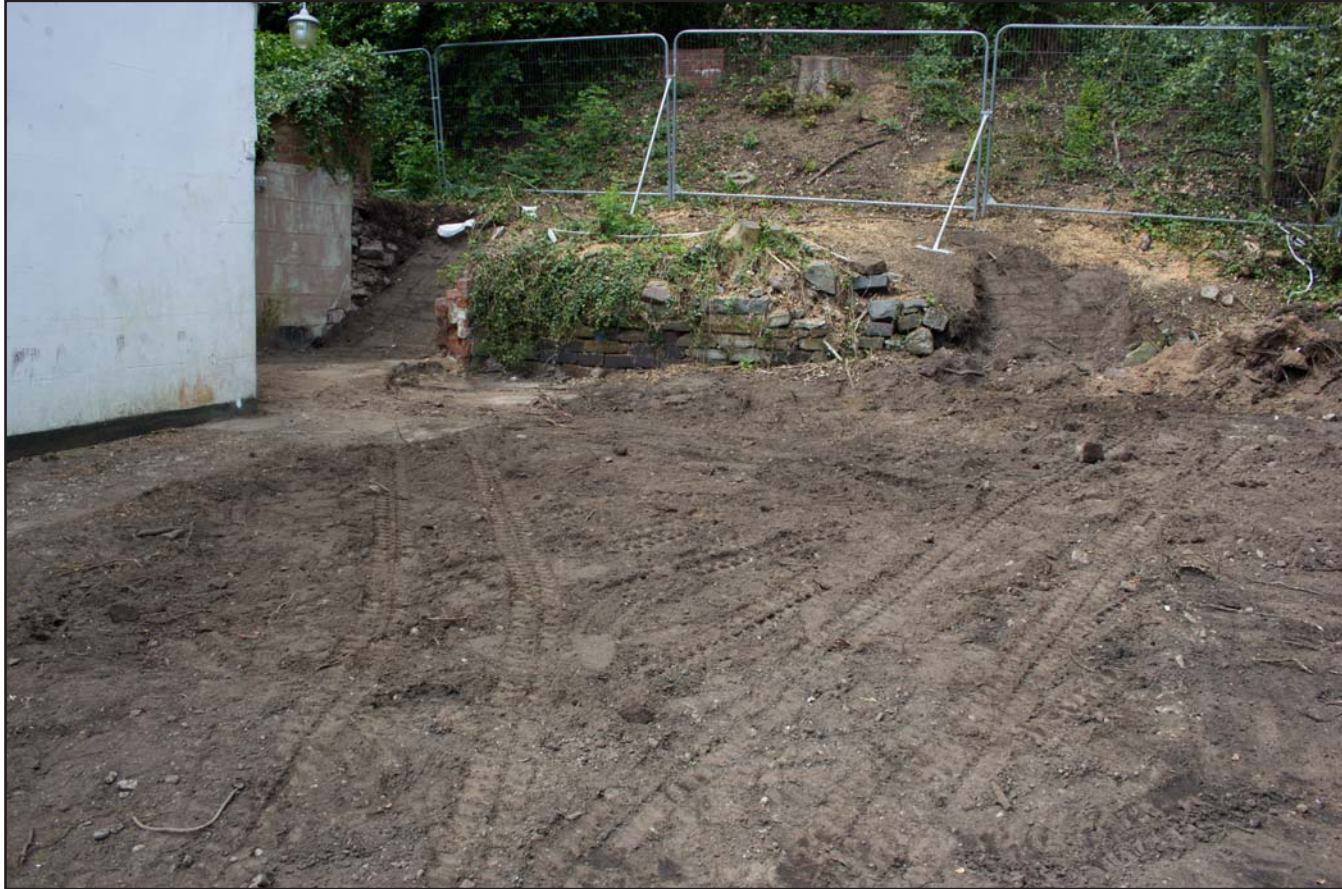
Plate 28: Evaluation Area (2) closed down and backfilled following archaeological work, Bailey Hill, Mold, Flintshire - from the southeast - no scale
