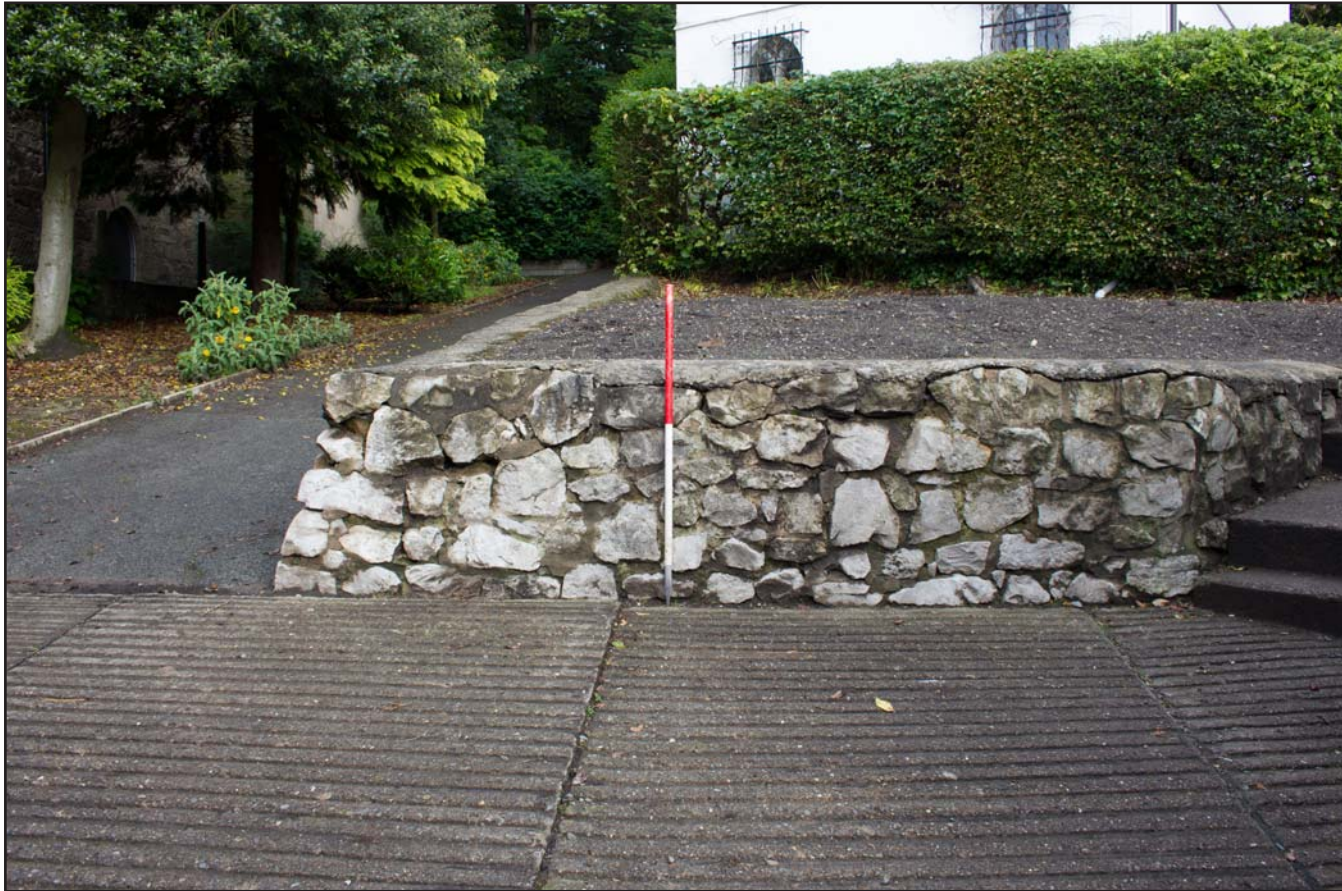
Plate 01: Pre excavation shot of Test Pit 1, Bailey Hill, Mold, Flintshire - from the southeast - scale 1m
