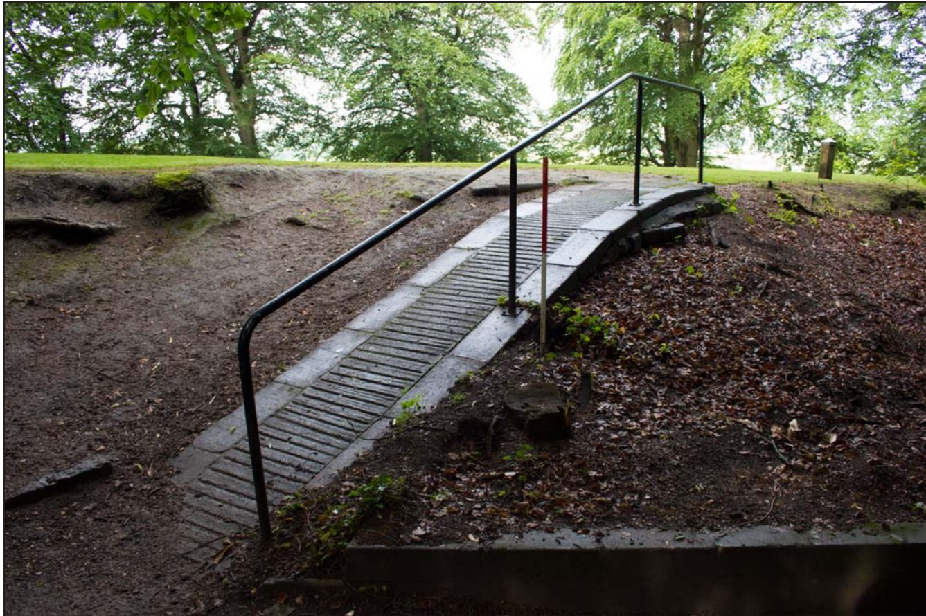
Plate 29: Pre excavation shot of evaluation area containing concrete ramp previously providing access to Outer Bailey ward, Bailey Hill, Mold, Flintshire - from the west - scale 1m
