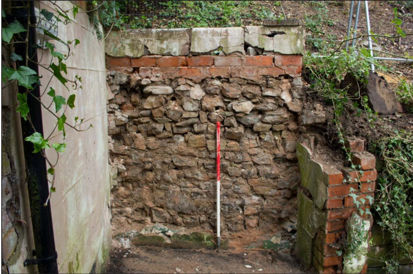
Plate 08: Removal of render from wall (406) in vicinity of Test Pit 4, Bailey Hill, Mold, Flintshire - from the southeast - scale 1m
