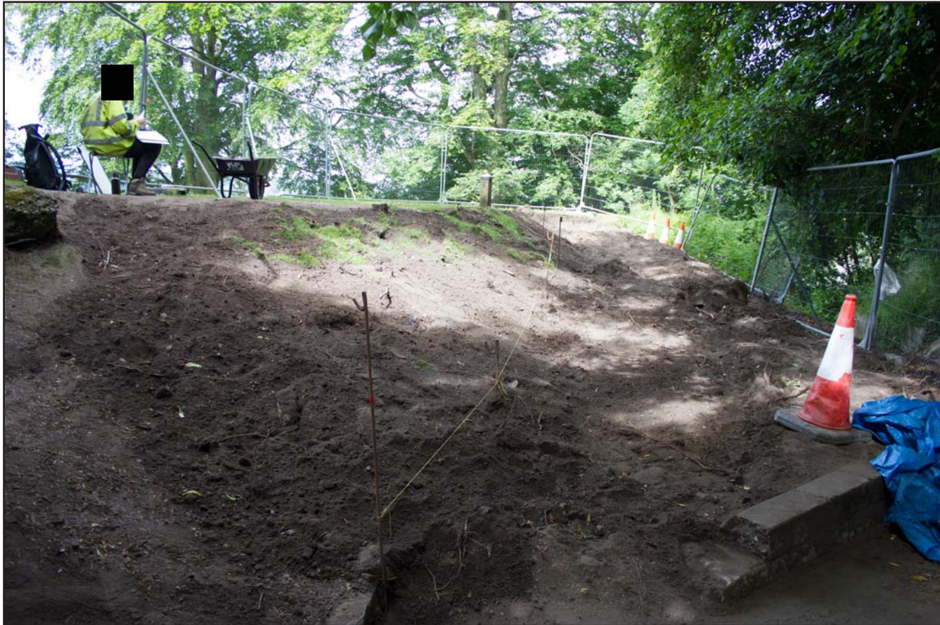
Plate 42: Reinstated soil and turf on the Outer Bailey access ramp - Bailey Hill, Mold, Flintshire - from the west - scale 1m
