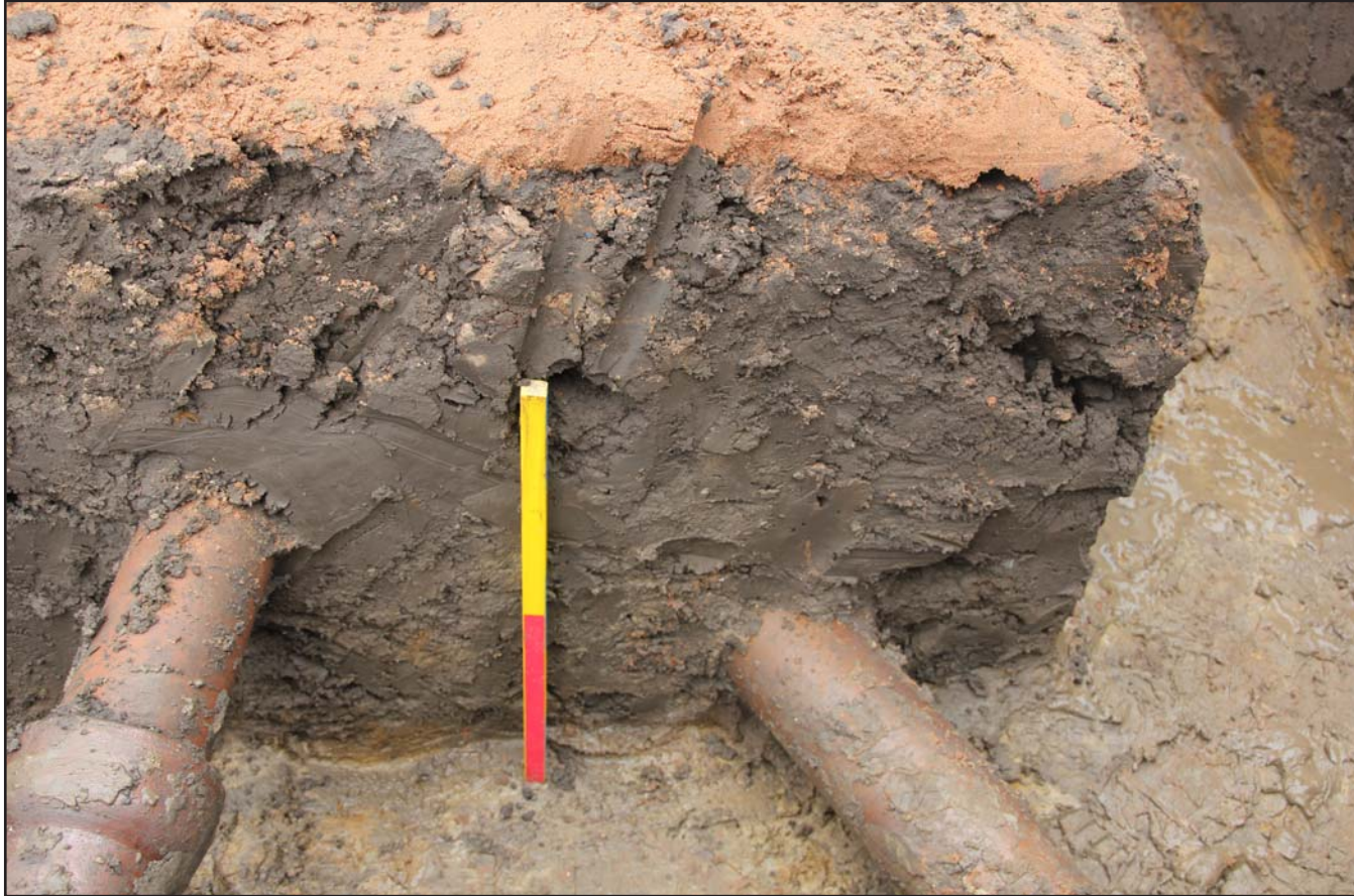
Plate 07: Section of extension southern foundation trench (running east-west), from the south. Scale 0.5m.
