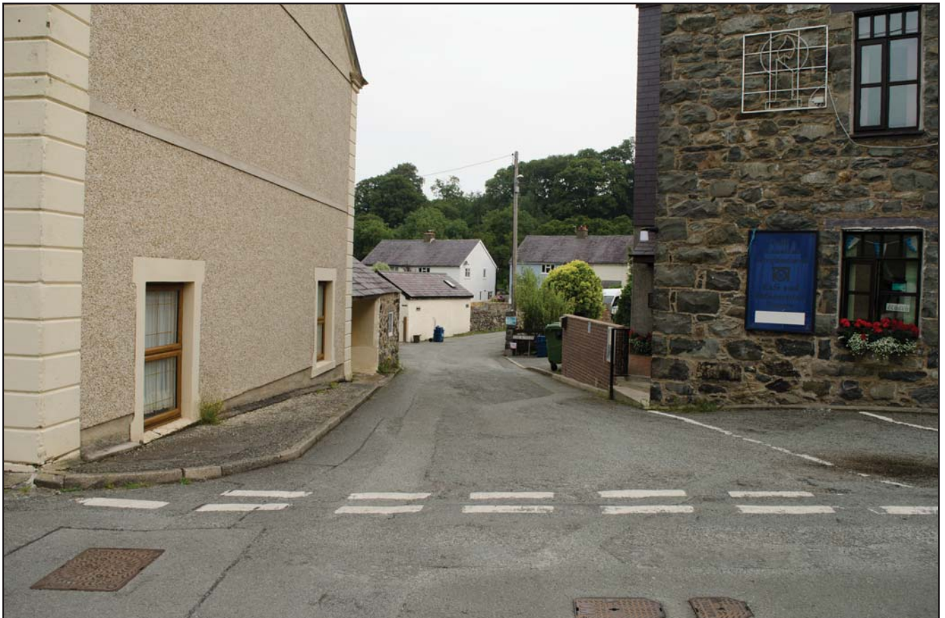
Plate 16: View towards the Enclosure and Associated Structures at Pen y Bryn (CN218) from the western end of the lane to the south of the proposed development site (Viewpoint 9), viewed from the southwest (archive ref G2651_004).
