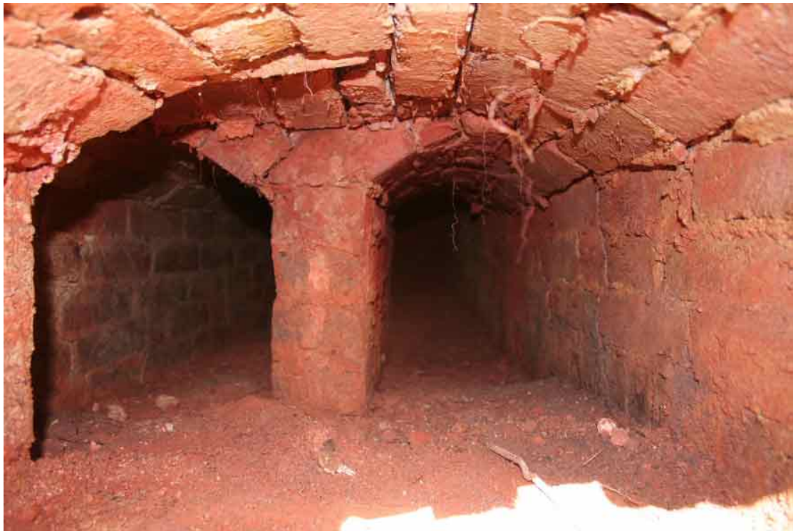
Photo 13: Trench 2C. Detail of flue structure beneath coke oven
