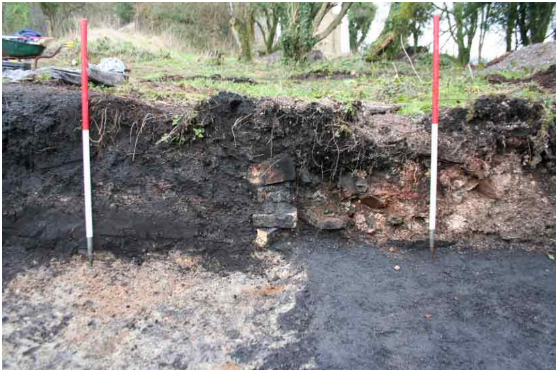
Photo 6: Trench 1A. Low brick wall (in section) separating the 'apron' (right) and 'platform' (left) working areas, looking west
