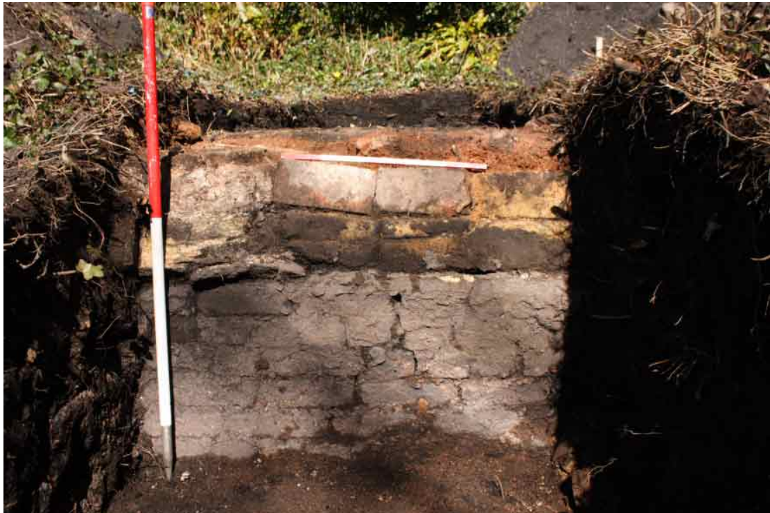
Photo 26: Trench 3A. North wall of box flue
