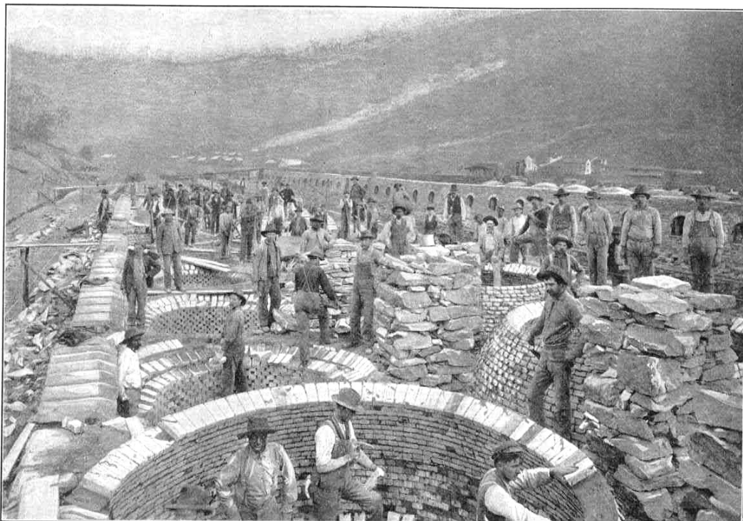
FIG. 9. CONSTRUCTING BEEHIVE OVENS
