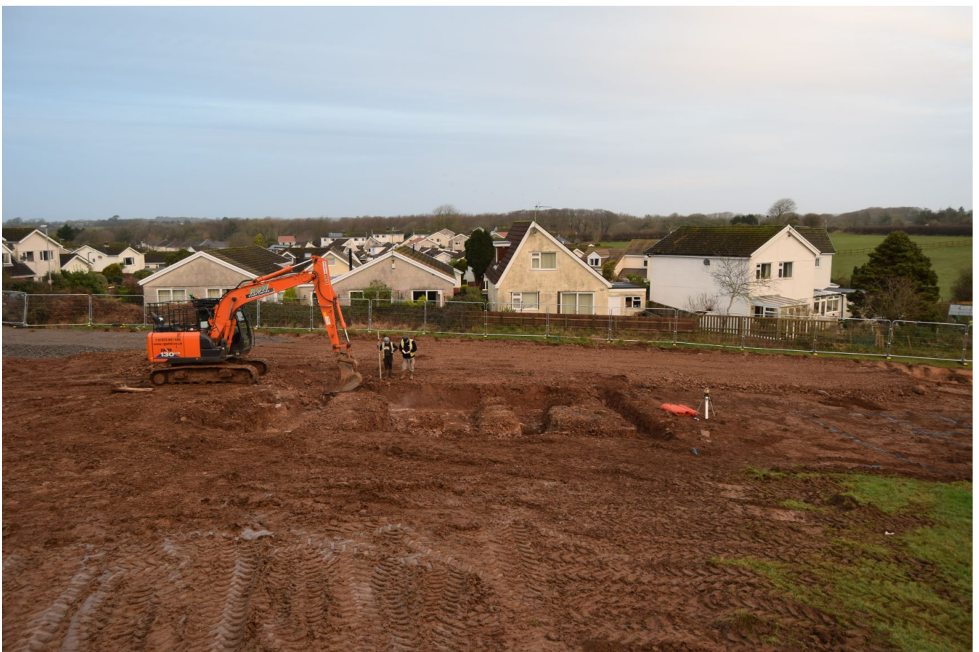
Plate 12. Excavation for foundations in northern area of site, facing north.
