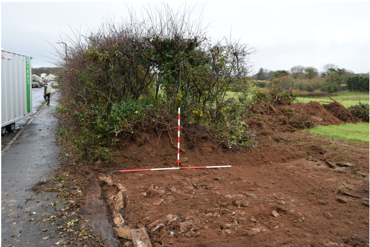
Plate 4. Removal of existing hedgerow, facing north, 1m & 2m scale.
