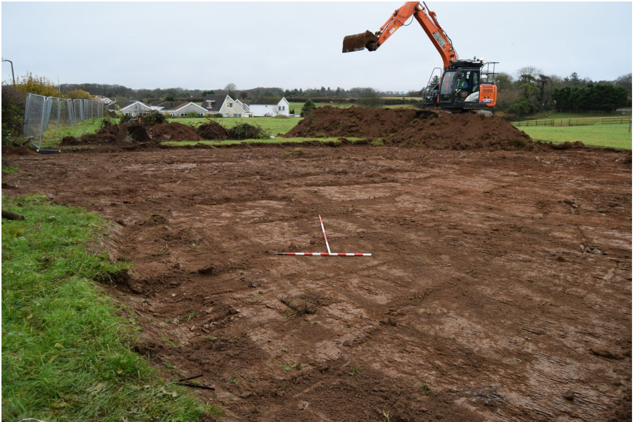
Plate 5. Topsoil (1000) removal, facing north-east, 1m & 2m scale.
