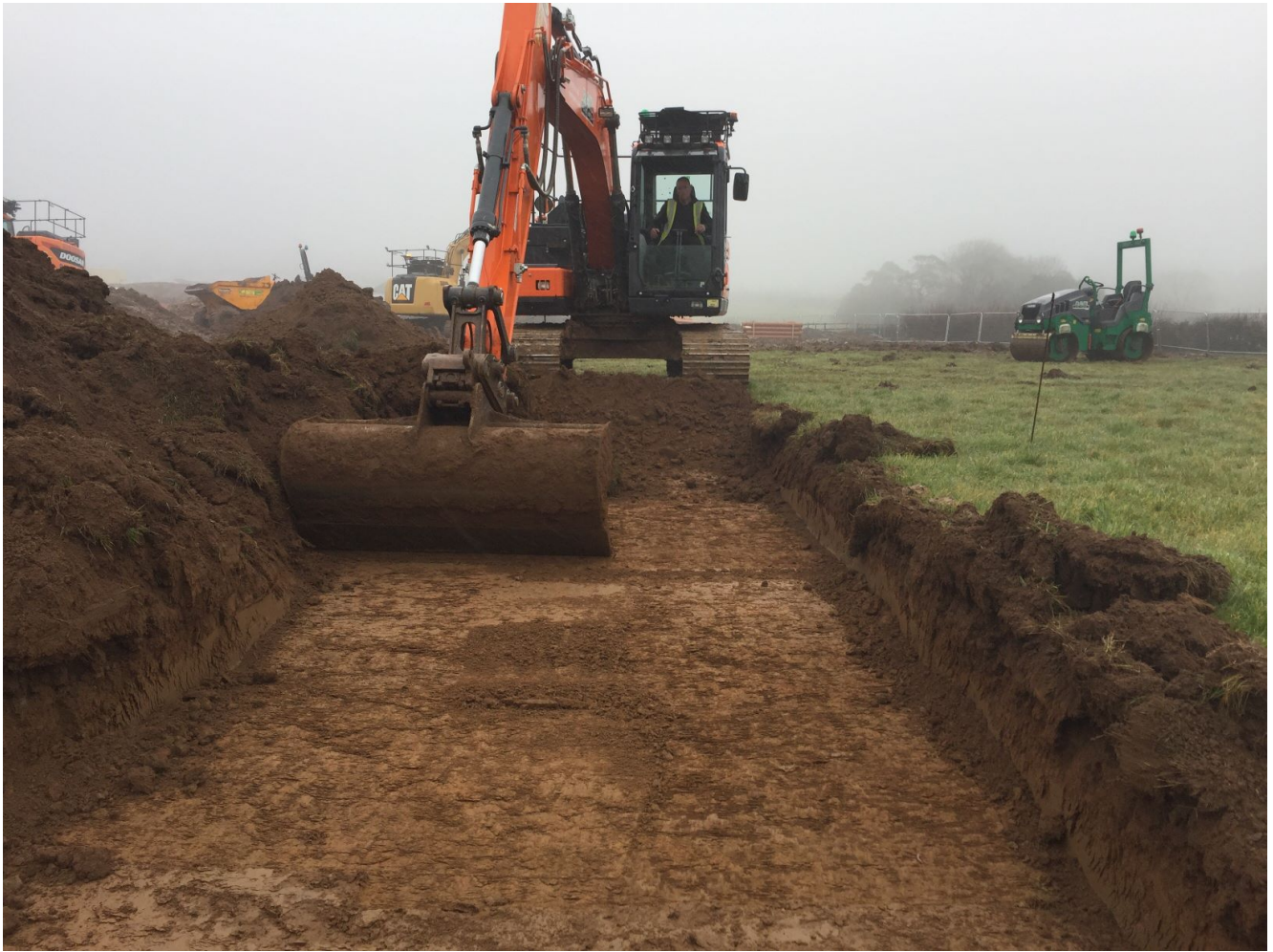
Plate 15. Topsoil (1000) removal in south-eastern area of site, facing north-east.
