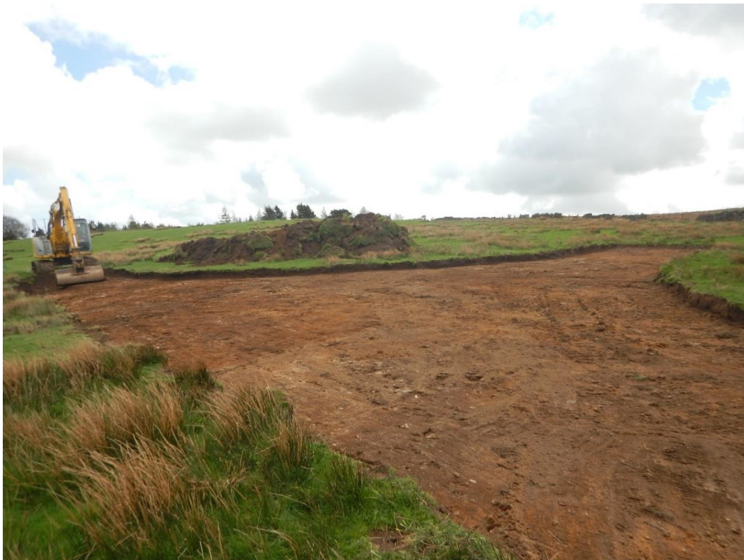
Photo 10: South facing shot of Phase 2 groundworks.
