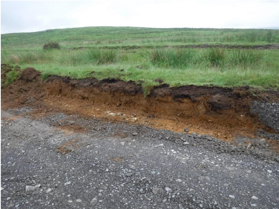
Photo 13: North facing shot of Phase 4 groundworks, showing deposits (006c), (005c) and (004c).
