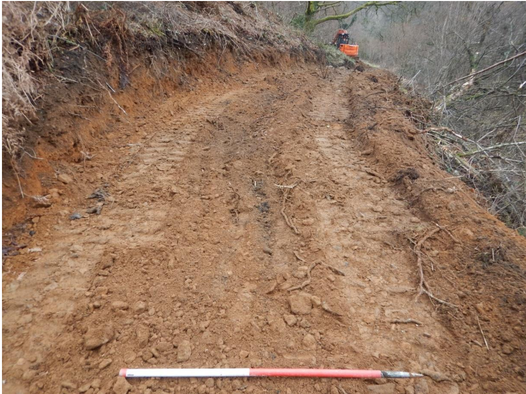
Photo 1: View west along the Phase 1 cabling route. 1m scale.
