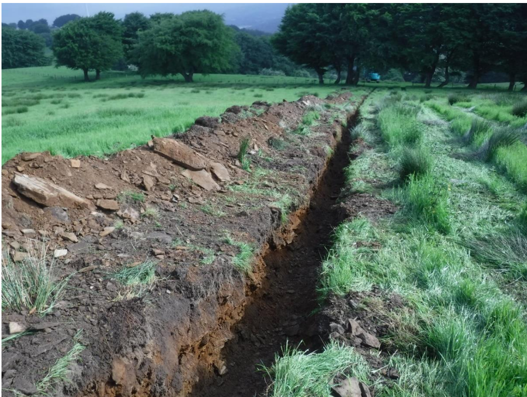
Photo 12: North facing shot of Phase 3 groundworks.
