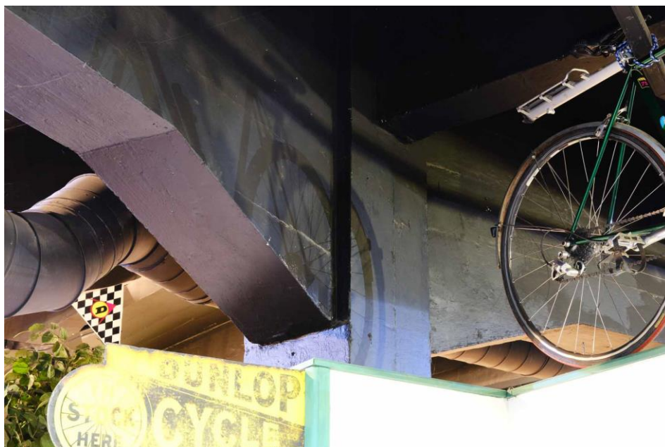
Figure 22. Detail of concrete pier and beam in room G.9.
