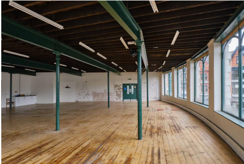
Figure 16. First floor of the original 1911 section of the building.
