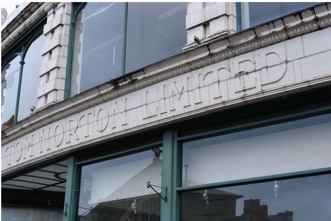
Figure 11. Fascia detail of the 1906-11 front to Temple Street.
