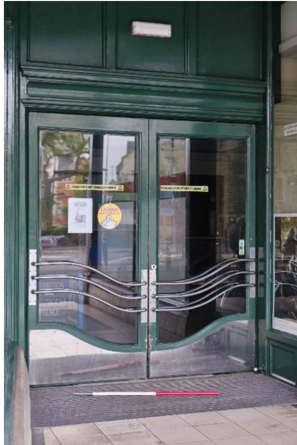
Figure 10. Doors to bay two, Temple Street.
