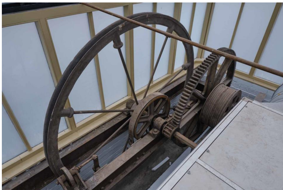
Figure 17. Hoist mechanism in room 2.1.
