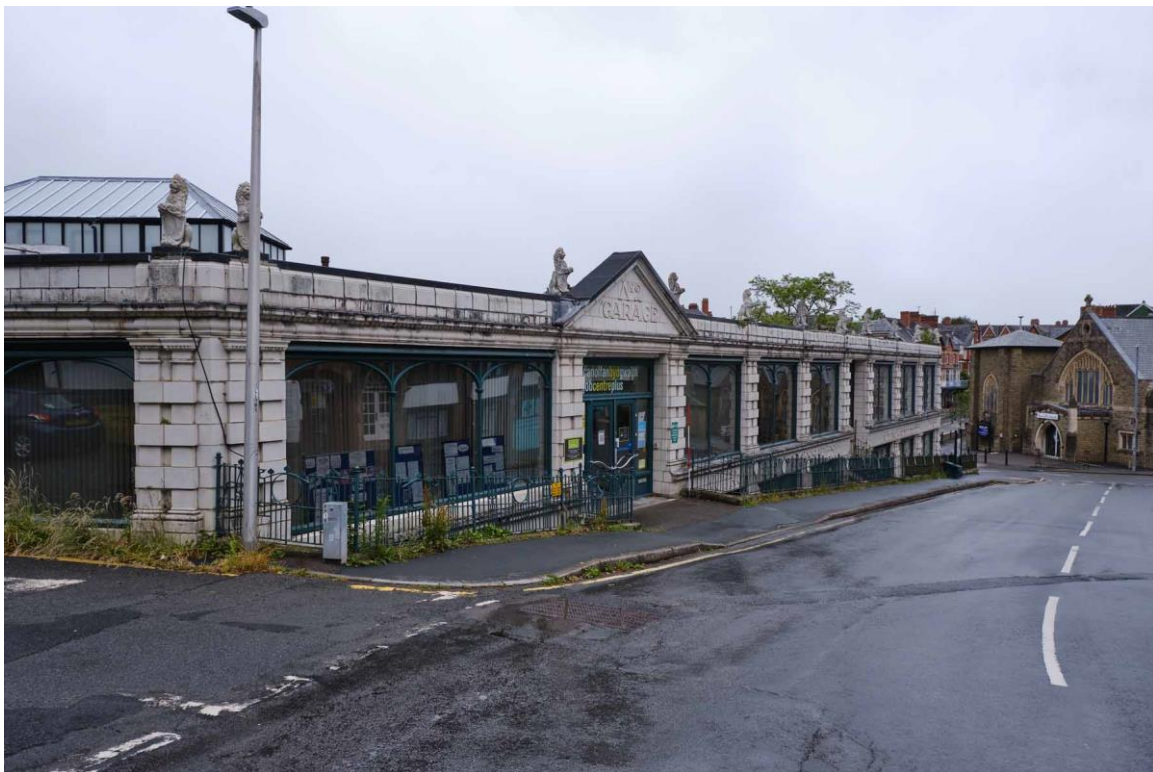
Figure 9. Princes Avenue front.
