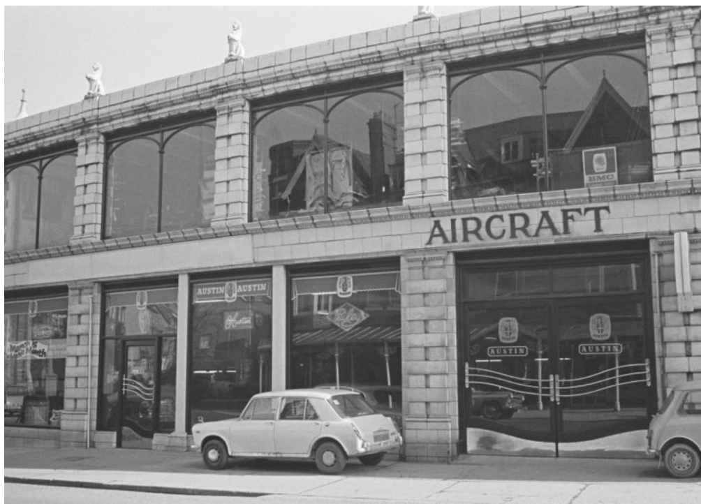
Figure 5. Entrances in bays 7-9 in 1969. (CC BY-NC-ND 2.0 UK)
