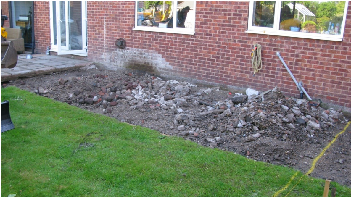
Site prior to excavation. Alan Wilmshurst
