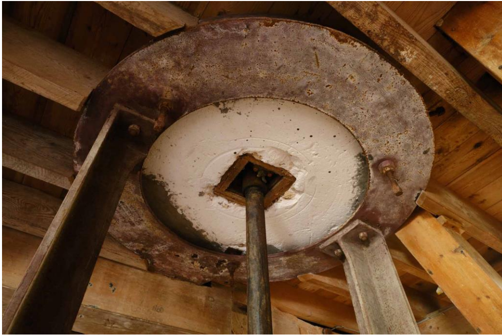
Figure 18. Hurst frame on the ground floor, supporting millstones.
