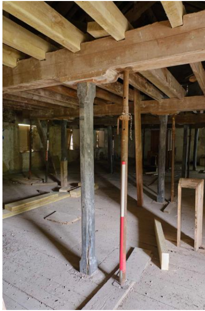
Figure 9. Timber post on third floor.
