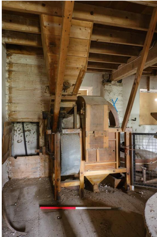
Figure 24. Howes smutter on first floor.
