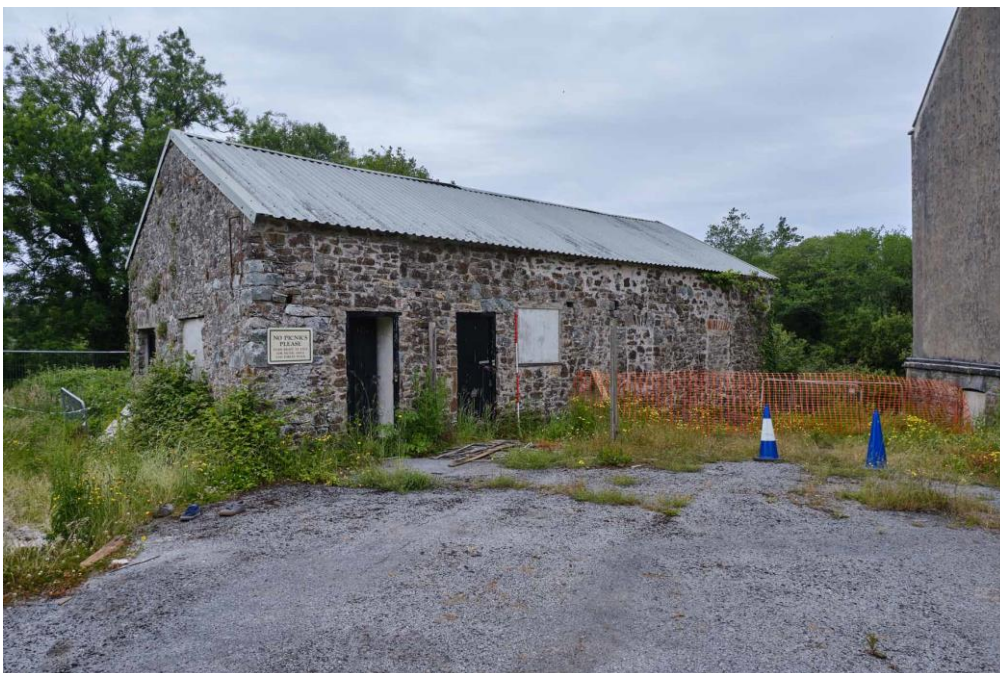
Figure 27. Store, looking north from the yard.
