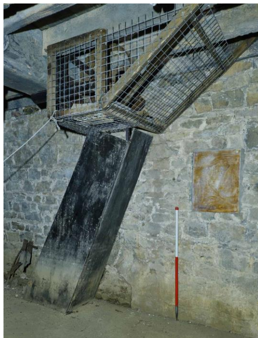
Figure 15. Drive from the secondary wheelpit in the basement.
